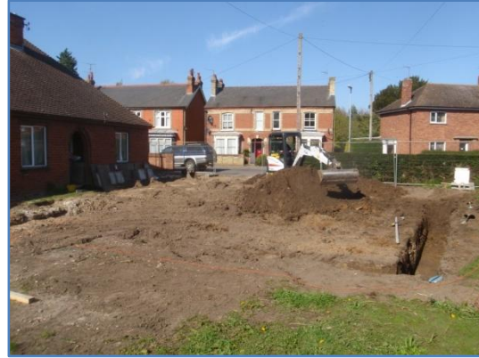
Plate 14: Ground reduction, from the south-west
