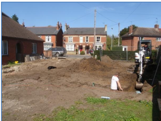
Plate 13: Excavation of the foundations, from the south-west
