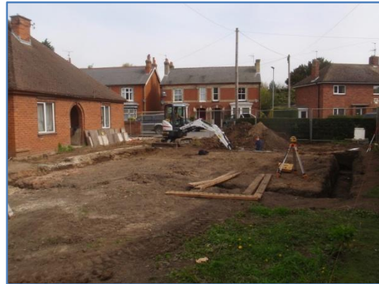
Plate 21: Excavation of the foundations, from the south-west
