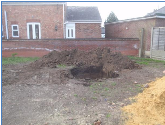
Plate 29: Completed excavation of the soakaway, from the north-west
