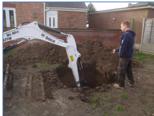
Plate 27: Excavation of the soakaway, from the north-west
