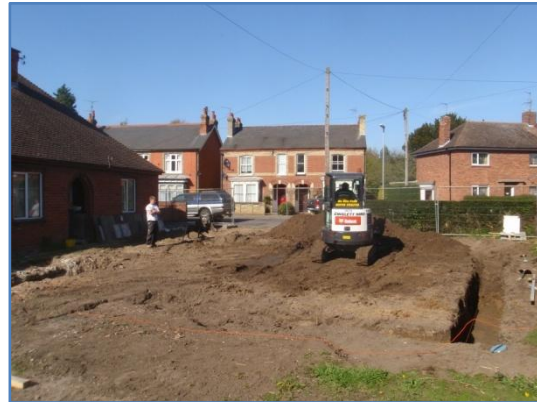
Plate 15: Ground reduction, from the south-west
