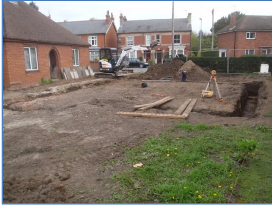
Plate 23: Excavation of the foundations, from the south-west
