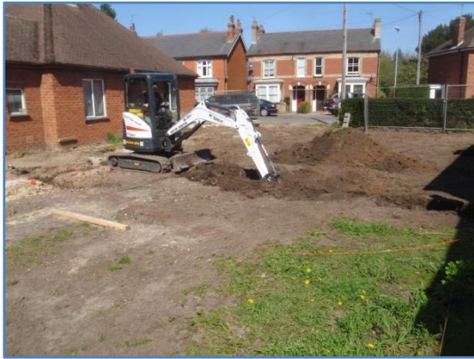
Plate 7: Excavation of the foundations, from the south-west
