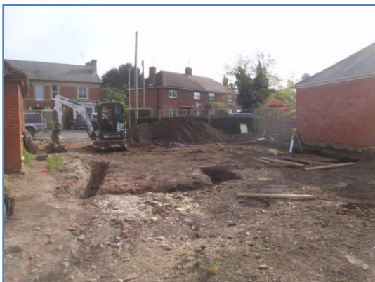
Plate 19: Excavation of the foundations, from the south-west
