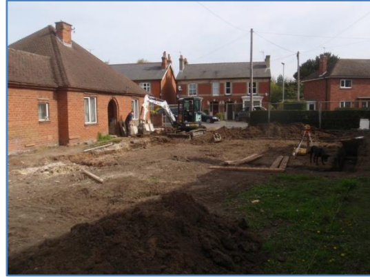
Plate 20: Excavation of the foundations, from the south-west
