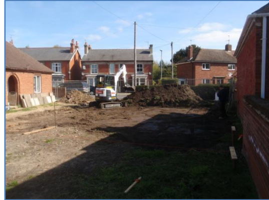
Plate 4: Ground reduction, from the south-west
