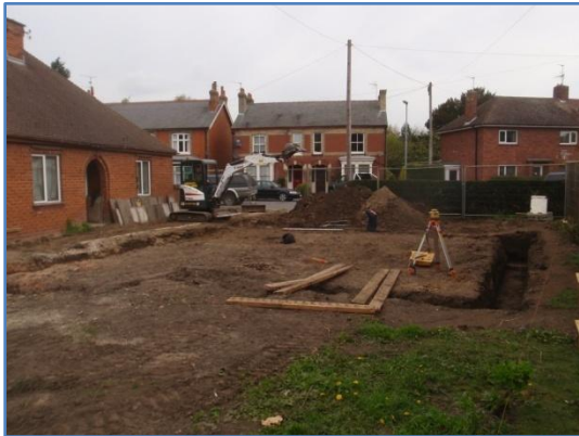
Plate 24: Completed foundation excavations, from the south-west
