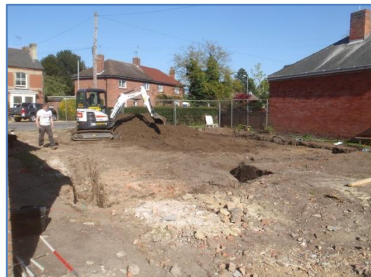
Plate 16: Ground reduction, from the south
