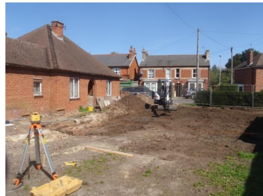
Plate 5: Ground reduction, from the south-west
