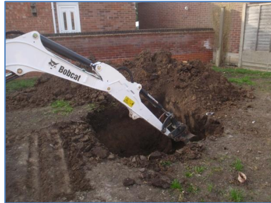
Plate 26: Excavation of the soakaway, from the north-west
