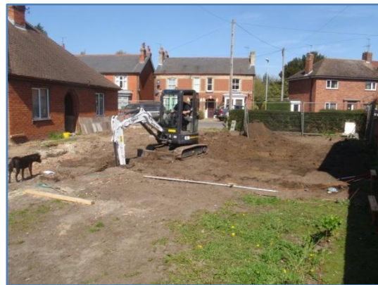
Plate 10: Excavation of the foundations, from the south-west
