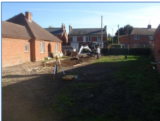
Plate 2: Ground reduction, from the south-west
