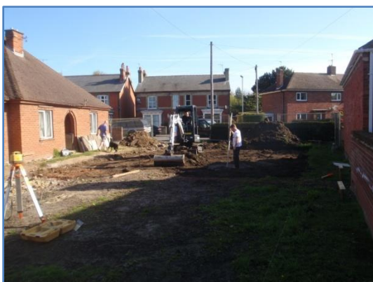
Plate 3: Ground reduction, from the south-west
