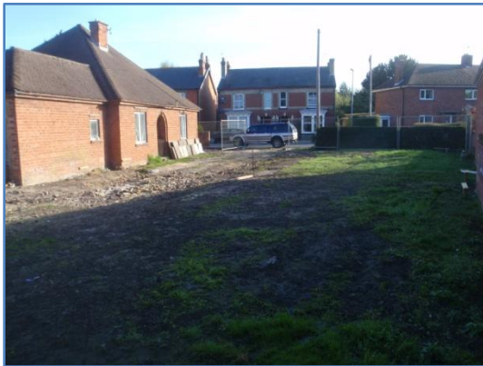
Plate 1: Pre-groundworks, from the south-west
