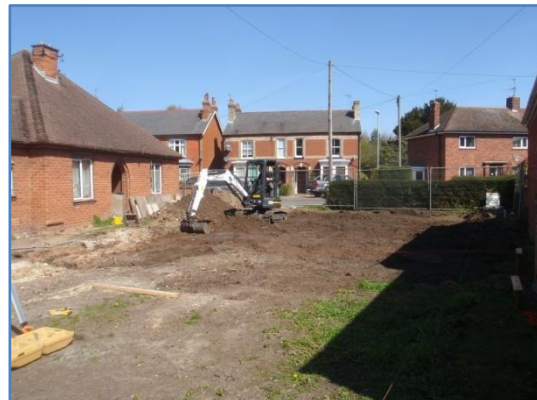
Plate 6: Ground reduction, from the south-west
