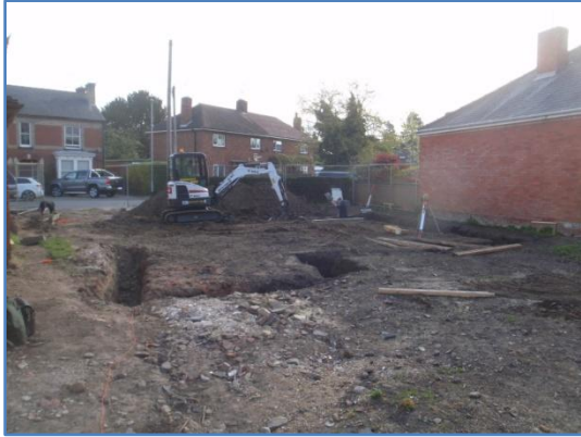
Plate 17: Excavation of the foundations, from the south-west
