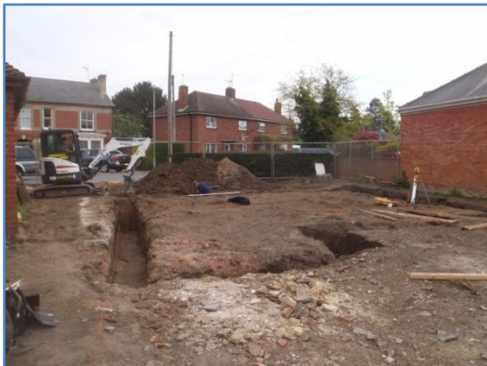
Plate 25: Completed foundation excavations, from the south-west
