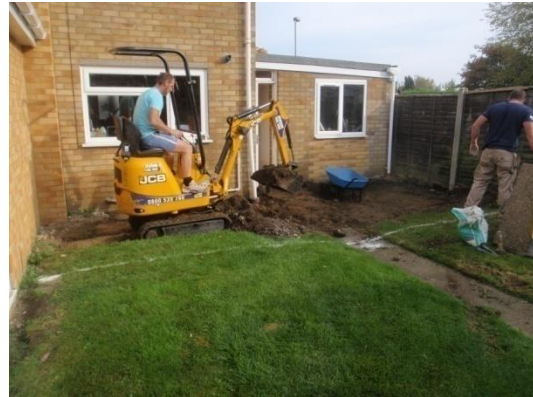
Plate 4: Initial ground reduction, from the south
