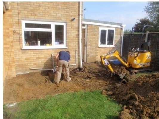
Plate 5: Initial ground reduction, from the south
