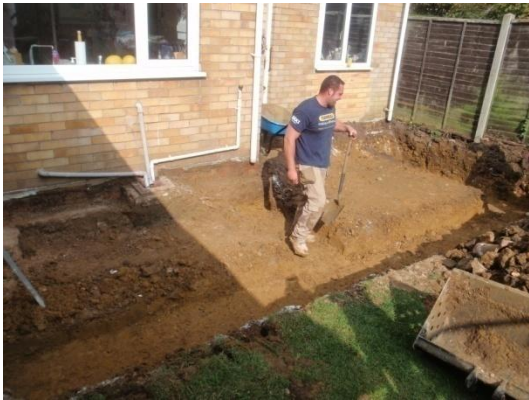
Plate 14: Completed excavation foundations, from the south-west
