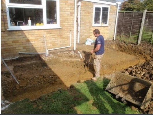
Plate 13: Excavation of the foundations, from the south-west
