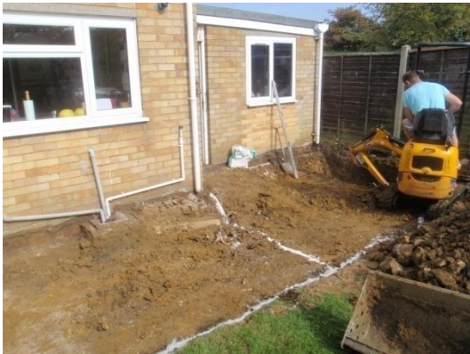
Plate 8: Excavation of the foundations, from the south-west
