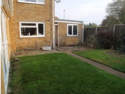
Plate 1: Pre-groundworks, from the south
