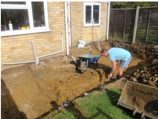
Plate 9: Excavation of the foundations, from the south-west
