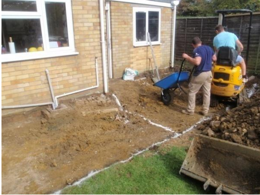
Plate 7: Excavation of the foundations, from the south-west
