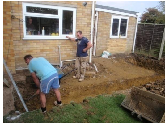
Plate 11: Excavation of the foundations, from the south-west
