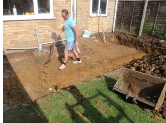
Plate 10: Excavation of the foundations, from the south-west
