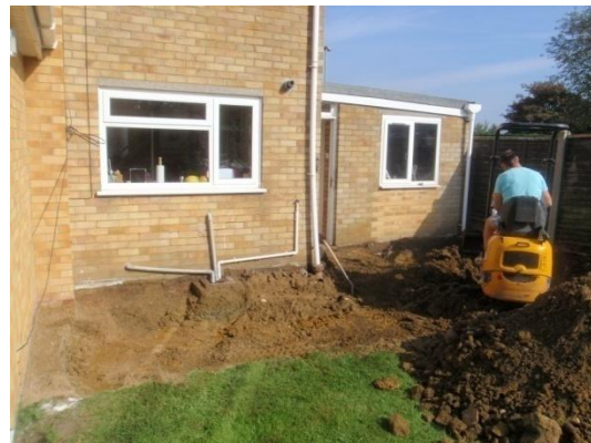
Plate 6: Initial ground reduction & excavation of the foundations, from the south
