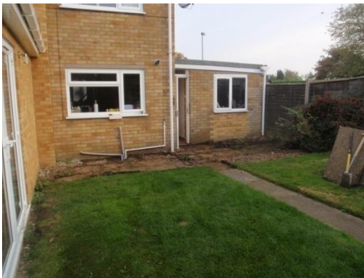
Plate 2: Paving slabs removed, from the south
