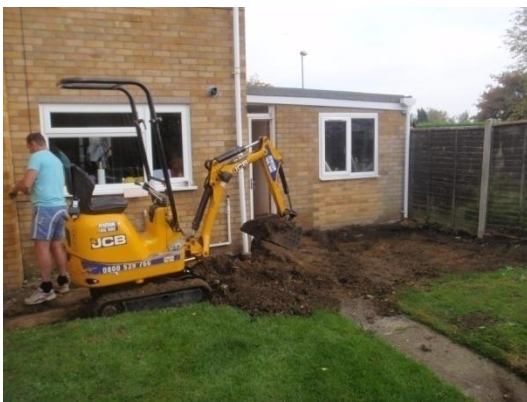
Plate 3: Initial ground reduction, from the south
