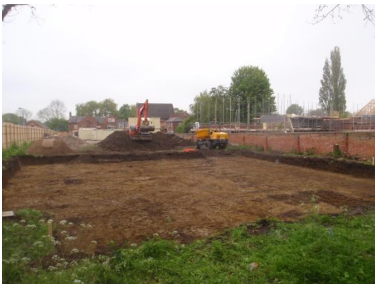
Plate 24: Ground reduction, from the north
