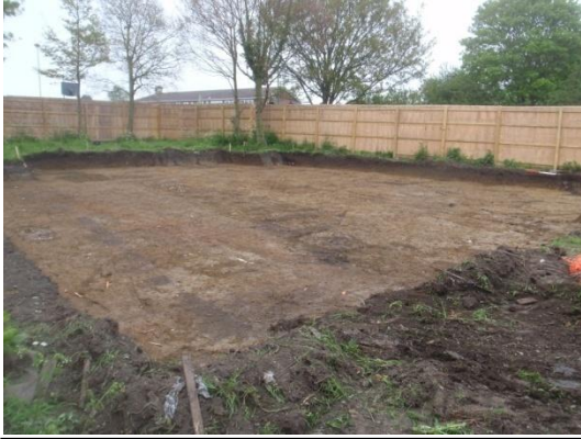
Plate 22: Ground reduction, from the south
