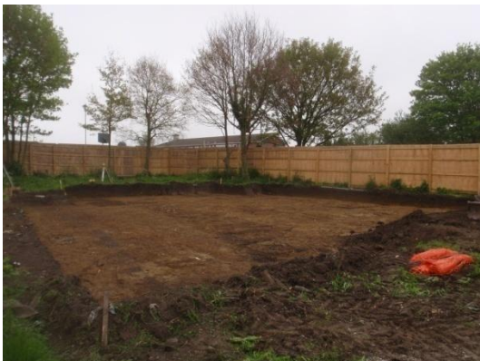
Plate 18: Ground reduction, from the south
