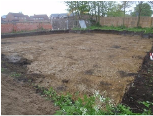
Plate 23: Ground reduction, from the south
