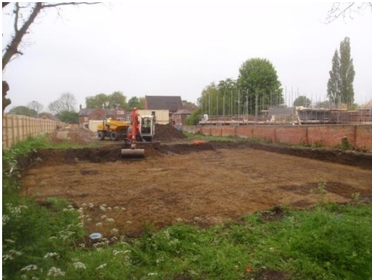
Plate 17: Ground reduction, from the north
