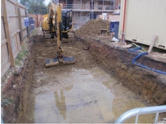
Plate 102: Excavation of the Service Trench 1 , from the north
