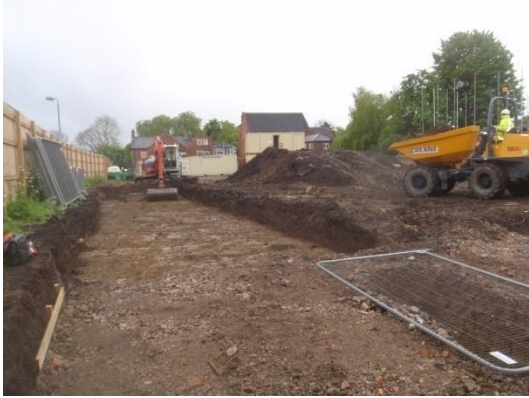
Plate 38: Ground reduction, from the north
