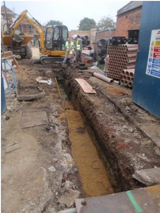
Plate 120: Excavation of the Service Trench 2 , from the south
