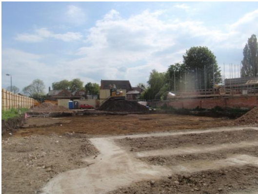
Plate 45: Ground reduction, from the north
