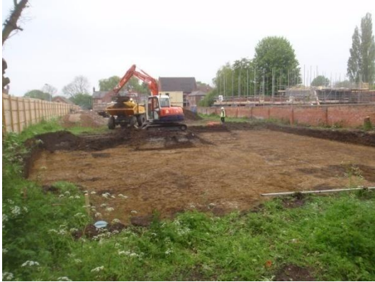
Plate 16: Ground reduction, from the north
