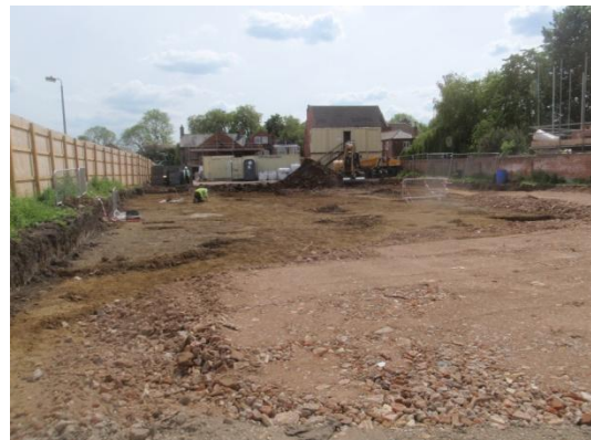
Plate 55: Ground reduction, from the north
