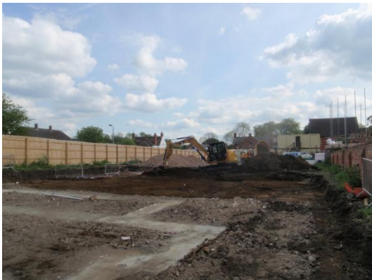
Plate 40: Ground reduction, from the north
