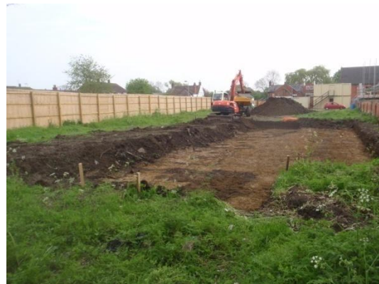
Plate 10: Ground reduction, from the north
