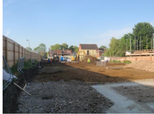
Plate 53: Ground reduction, from the north
