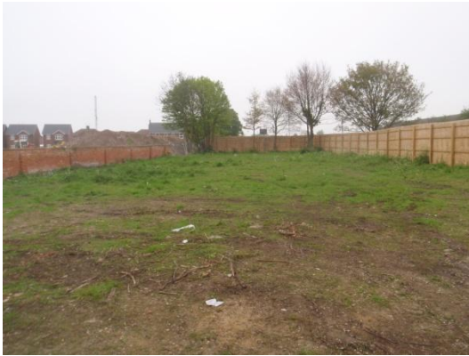
Plate 2: Pre-groundworks, from the south
