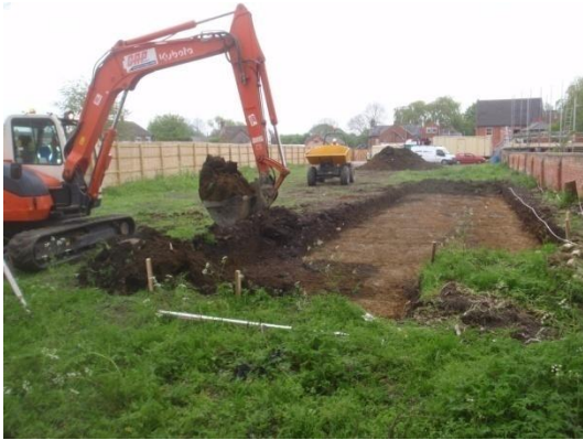
Plate 7: Ground reduction, from the north
