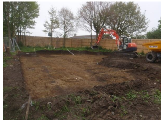
Plate 15: Ground reduction, from the south
