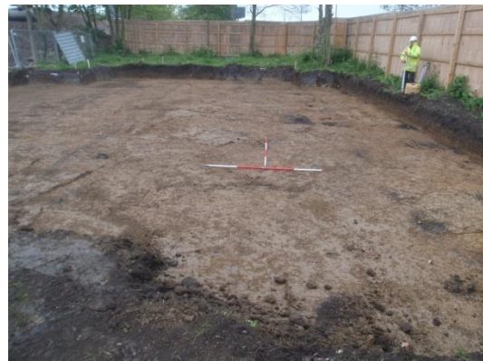
Plate 21: Ground reduction, from the south
