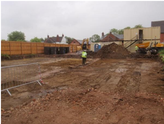
Plate 57: Ground reduction, from the north
