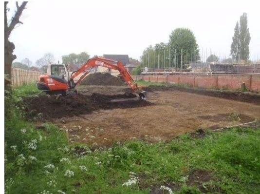
Plate 14: Ground reduction, from the north
