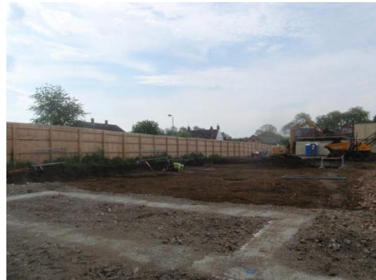
Plate 48: Ground reduction, from the north
