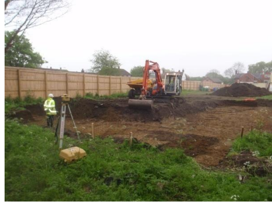
Plate 13: Ground reduction, from the north
