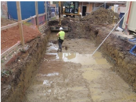
Plate 108: Excavation of the Service Trench 1 , from the north
