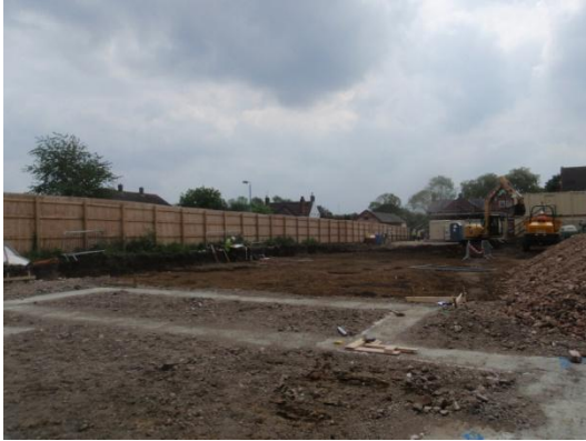
Plate 50: Ground reduction, from the north
