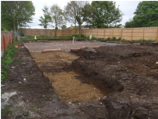
Plate 39: Ground reduction, from the south
