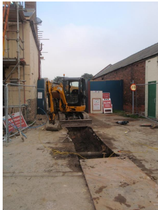
Plate 110: Excavation of the Service Trench 2 , from the south-east
