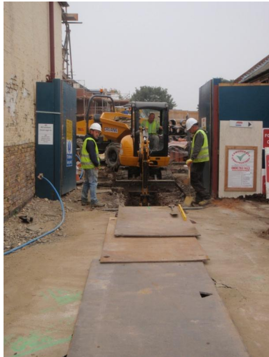
Plate 114: Excavation of the Service Trench 2, from the south
