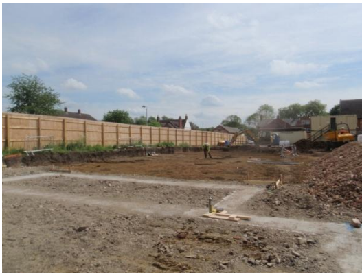
Plate 52: Ground reduction, from the north
