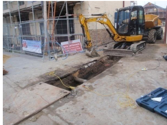
Plate 109: Excavation of the Service Trench 2 , from the south-east
