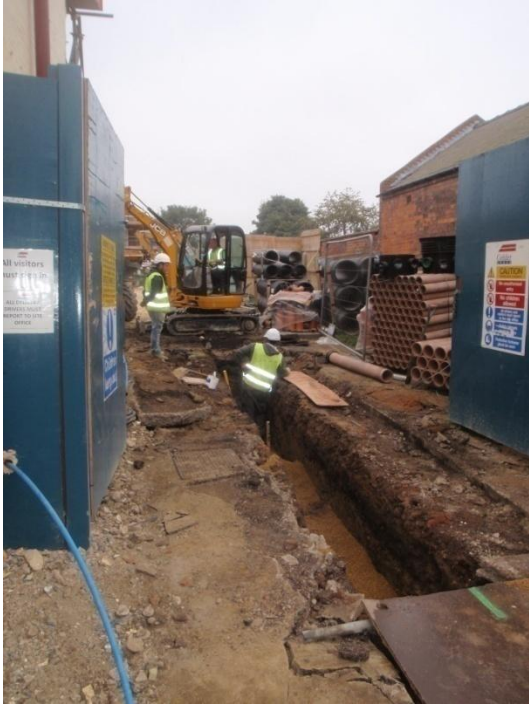
Plate 119: Excavation of the Service Trench 2 , from the south
