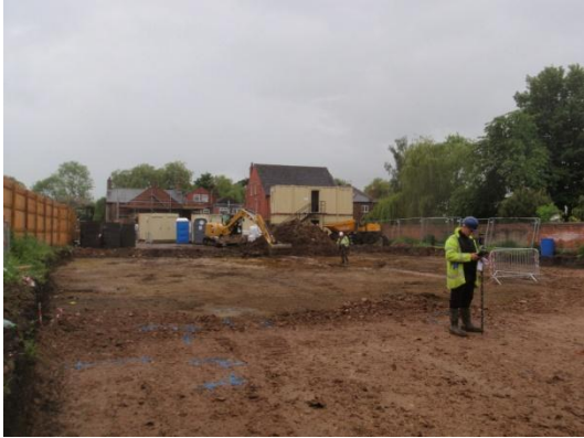
Plate 56: Ground reduction, from the north
