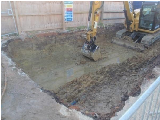
Plate 99: Excavation of the Service Trench 1 , from the north-west
