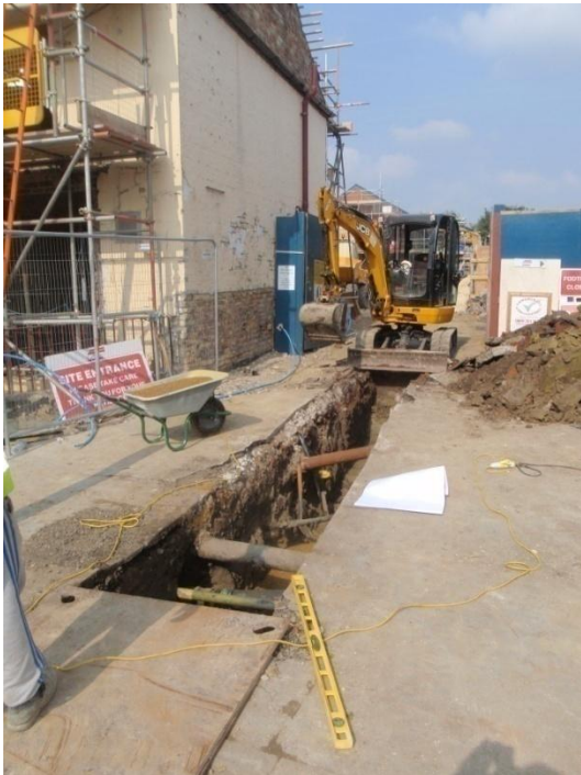
Plate 112: Excavation of the Service Trench 2, from the south
