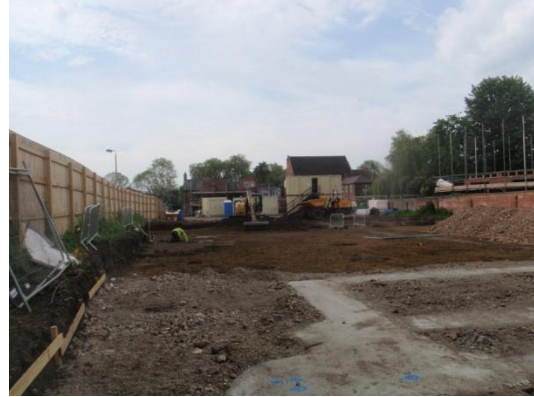
Plate 47: Ground reduction, from the north
