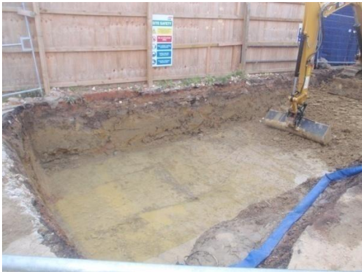
Plate 103: Excavation of the Service Trench 1 , from the north-west
