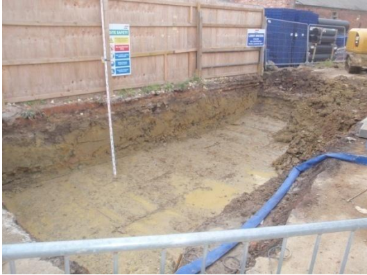
Plate 106: Excavation of the Service Trench 1 , from the north-west
