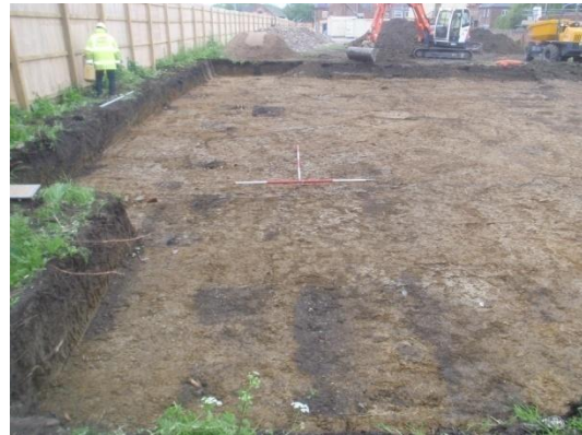
Plate 20: Ground reduction, from the south
