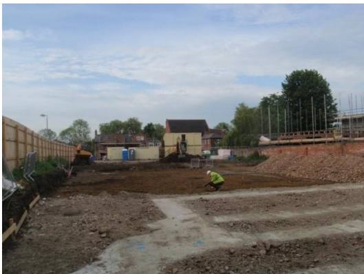
Plate 46: Ground reduction, from the north
