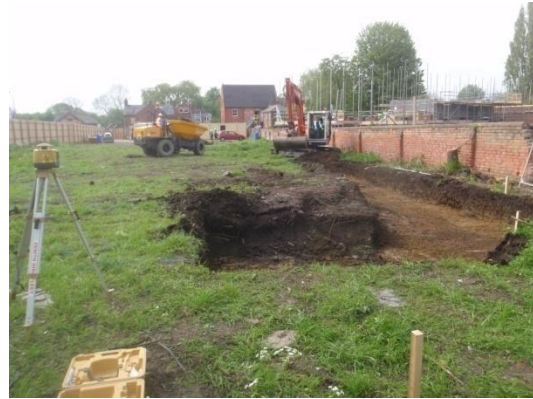
Plate 4: Ground reduction, from the north
