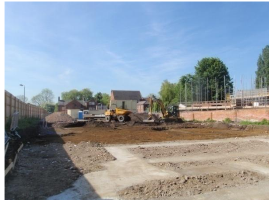
Plate 43: Ground reduction, from the north
