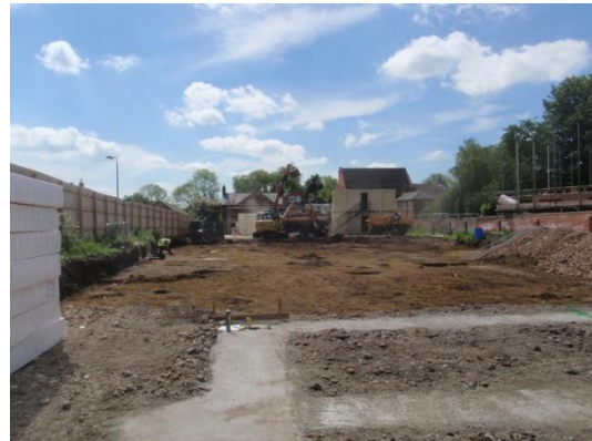
Plate 54: Ground reduction, from the north
