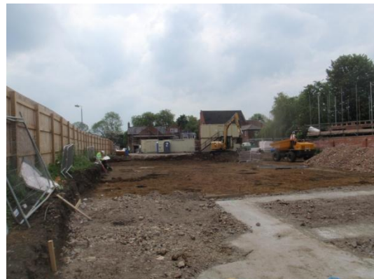
Plate 49: Ground reduction, from the north
