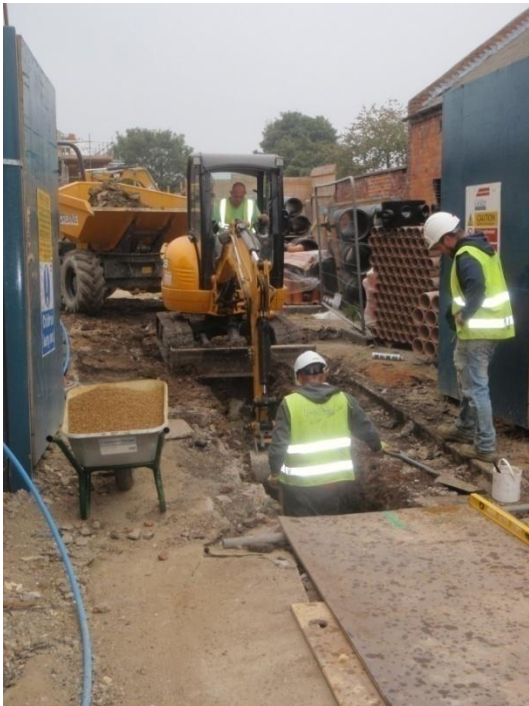
Plate 116: Excavation of the Service Trench 2, from the south
