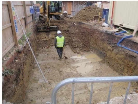
Plate 105: Excavation of the Service Trench 1 , from the north
