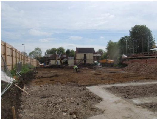
Plate 51: Ground reduction, from the north
