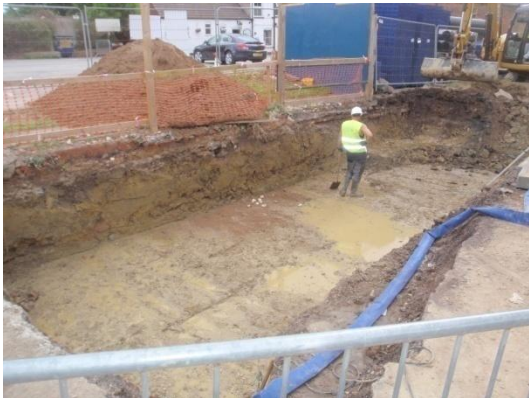
Plate 107: Excavation of the Service Trench 1 , from the north-west
