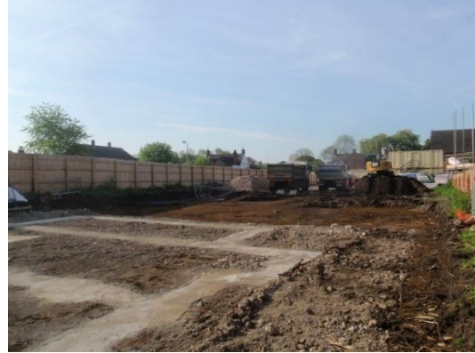
Plate 41: Ground reduction, from the north
