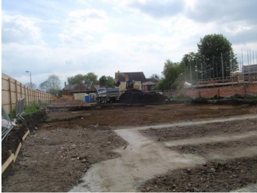
Plate 44: Ground reduction, from the north
