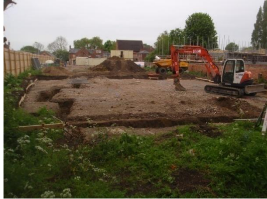
Plate 35: Area A, excavation of the foundations, from the north
