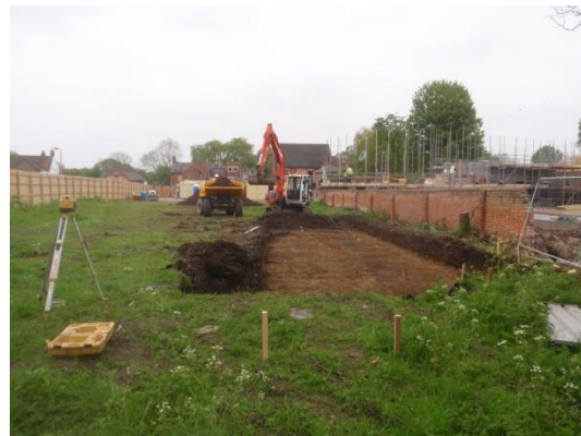
Plate 5: Ground reduction, from the north
