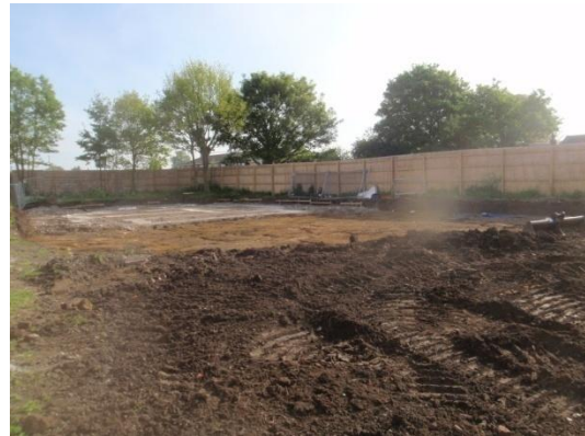
Plate 42: Ground reduction, from the south
