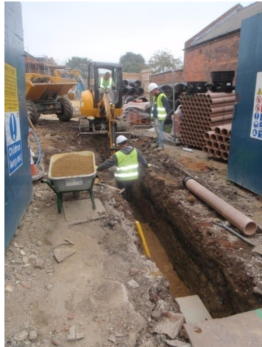
Plate 118: Excavation of the Service Trench 2, from the south
