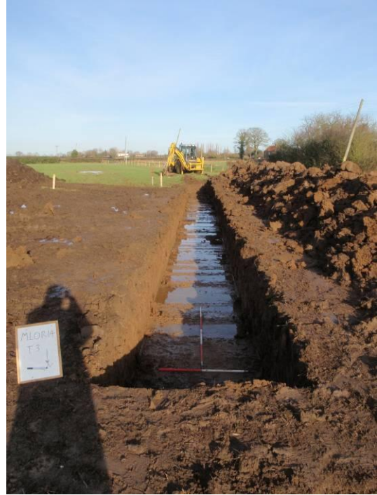
Plate 7: Trench 3, from the south-west
