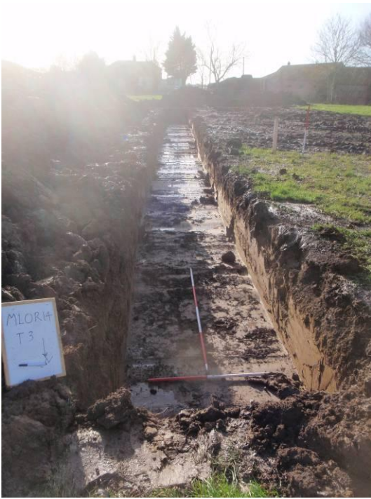
Plate 6: Trench 3, from the north-east
