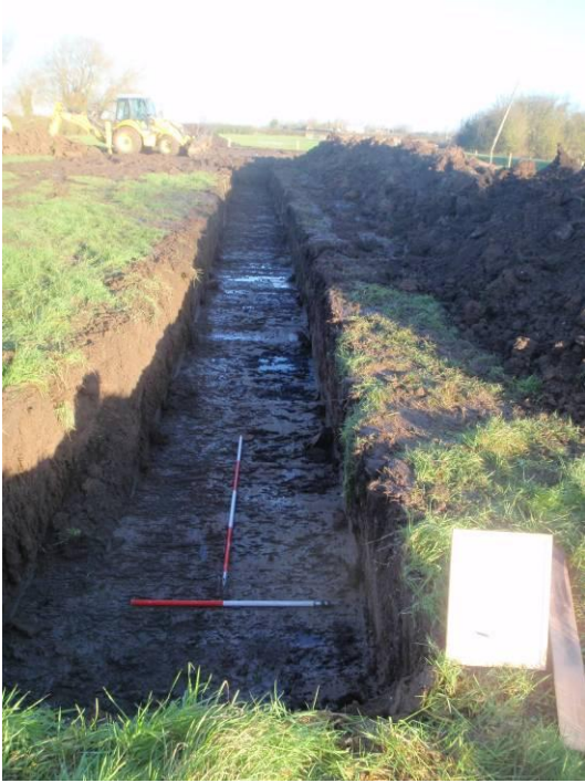
Plate 1: Trench 1, from the south
