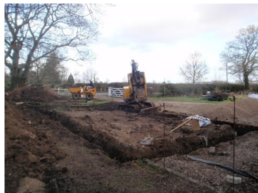
Plate 27: Excavation of the garage/workshop foundations, from the south-west
