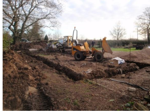
Plate 31: Excavation of the garage/workshop foundations, from the south-west
