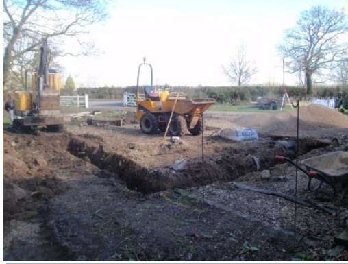
Plate 22: Excavation of the garage/workshop foundations, from the south-west
