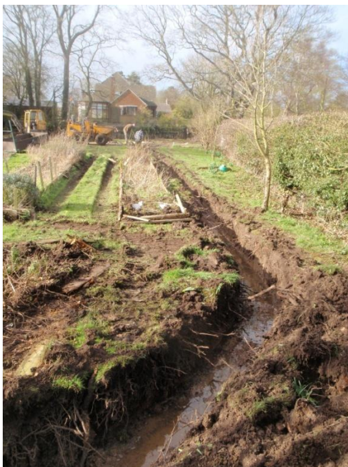
Plate 18: Excavation of the service trench, from the east
