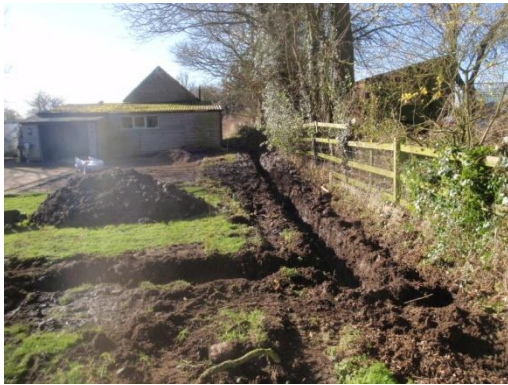
Plate 1: Excavations in the infilled drainage dyke, from the north
