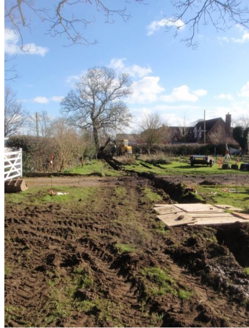
Plate 15: Excavation of the service trench, from the north-west
