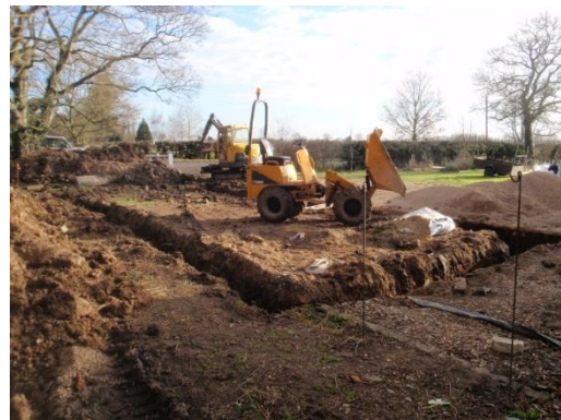
Plate 33: Excavation of the garage/workshop foundations, from the south-west
