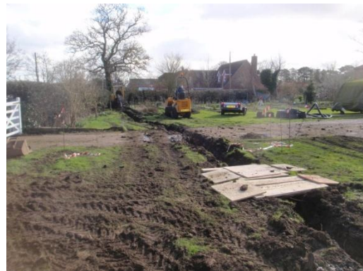
Plate 12: Excavation of the service trench, from the north-west
