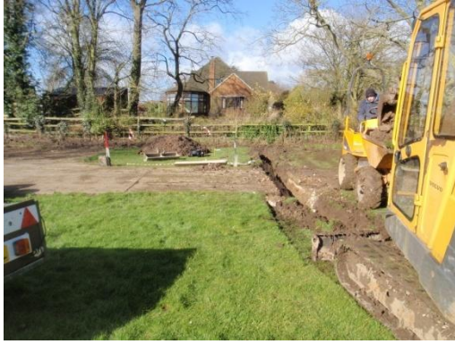
Plate 7: Excavation of the service trench, from the east
