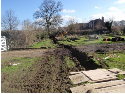
Plate 13: Excavation of the service trench, from the north-west
