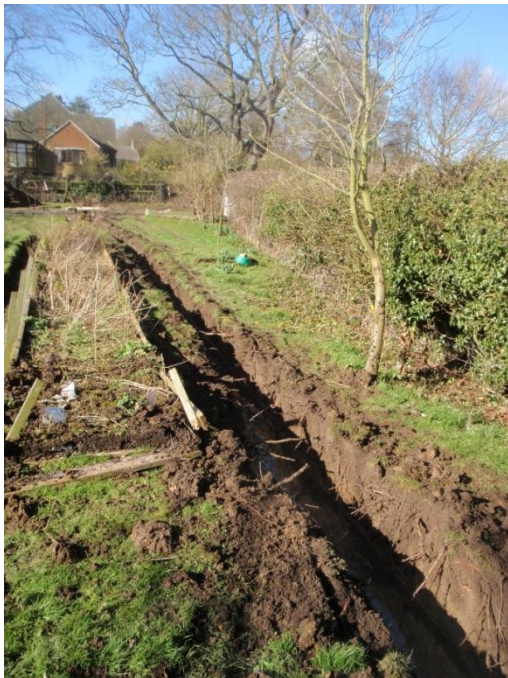
Plate 14: Excavation of the service trench, from the south-east
