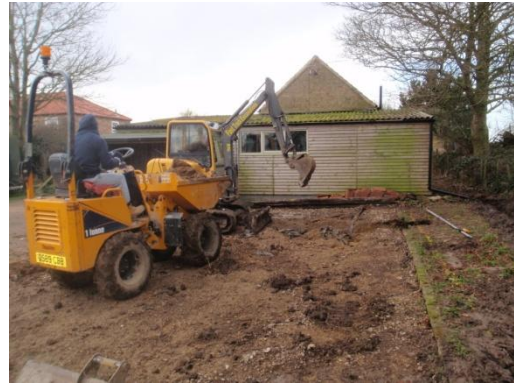
Plate 19: Excavation of the garage/workshop foundations, from the north-east
