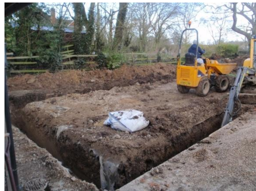
Plate 26: Excavation of the garage/workshop foundations, from the south-east
