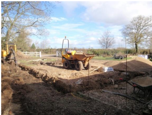
Plate 23: Excavation of the garage/workshop foundations, from the south-west
