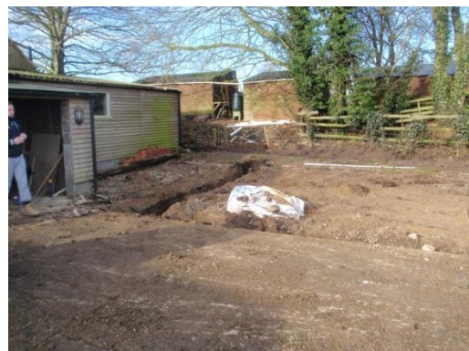
Plate 21: Excavation of the garage/workshop foundations, from the east
