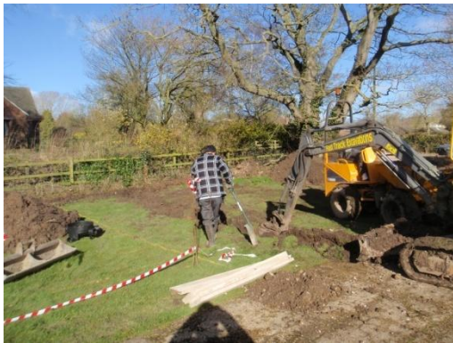
Plate 2: Excavation of the service trench, from the south-east
