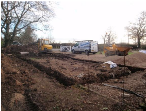
Plate 29: Excavation of the garage/workshop foundations, from the south-west
