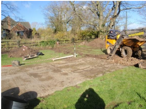
Plate 3: Excavation of the service trench, from the south-east
