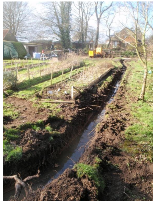
Plate 16: Excavation of the service trench, from the east
