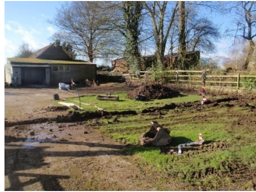
Plate 4: Excavation of the service trench, from the north
