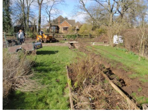
Plate 10: Excavation of the service trench, from the south-east
