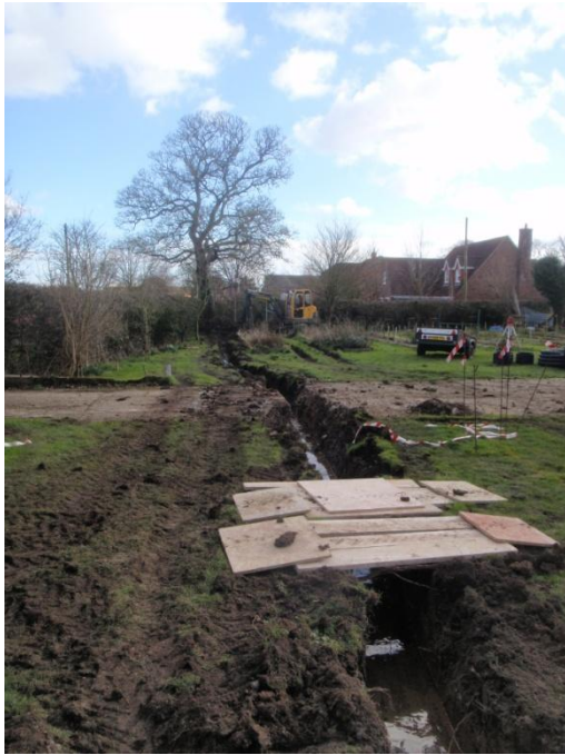
Plate 17: Excavation of the service trench, from the north-west
