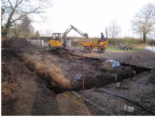
Plate 28: Excavation of the garage/workshop foundations, from the south-west
