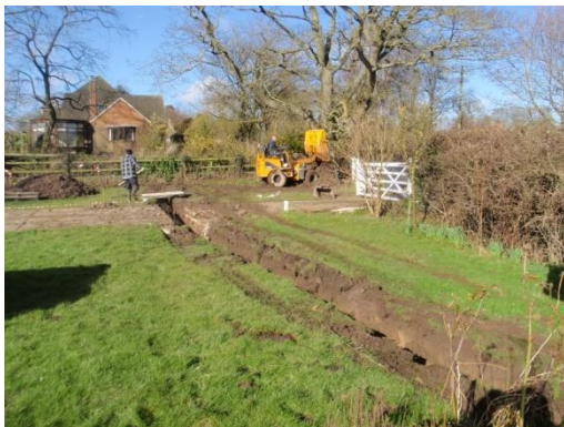
Plate 9: Excavation of the service trench, from the south-east
