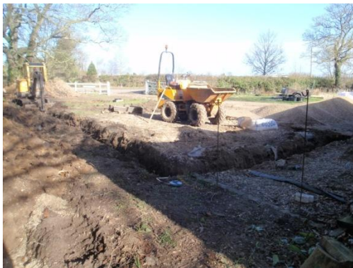
Plate 24: Excavation of the garage/workshop foundations, from the south-west
