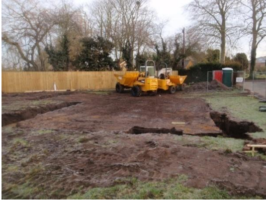
Plate 13: Excavation of the foundations, from the south
