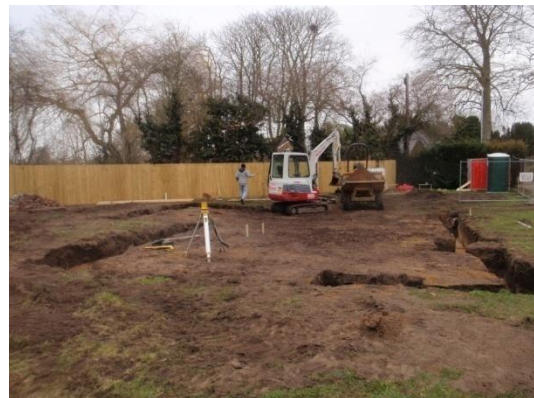
Plate 18: Excavation of the foundations, from the south
