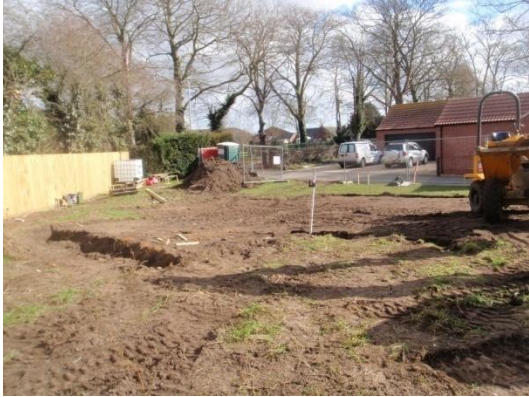
Plate 7: Excavation of the foundations, from the south-west
