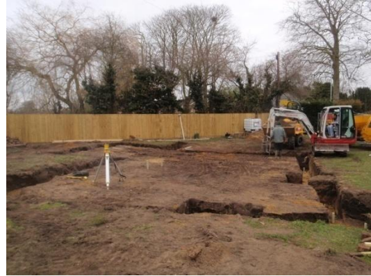
Plate 22: Excavation of the foundations, from the south
