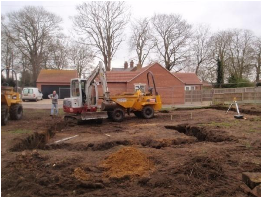
Plate 20: Excavation of the foundations, from the west
