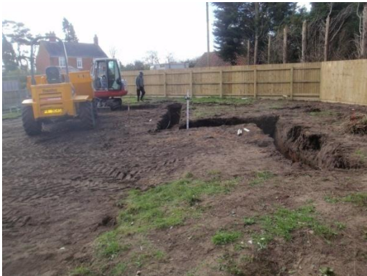
Plate 8: Excavation of the foundations, from the east
