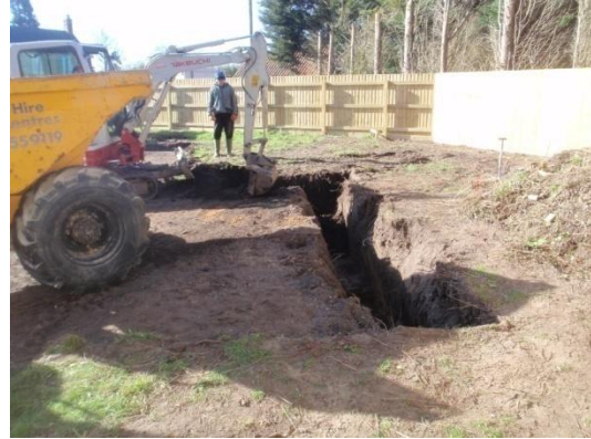
Plate 4: Excavation of the foundations, from the east
