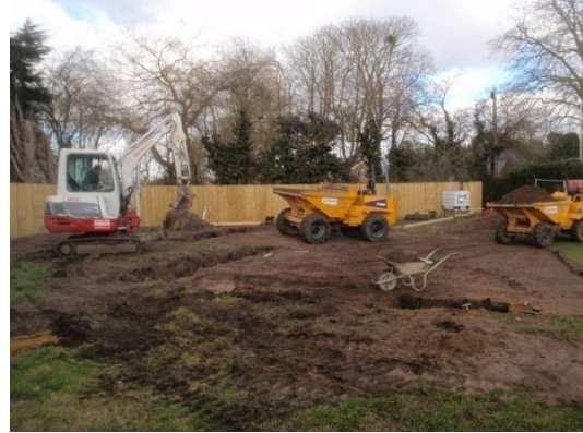
Plate 10: Excavation of the foundations, from the north-east
