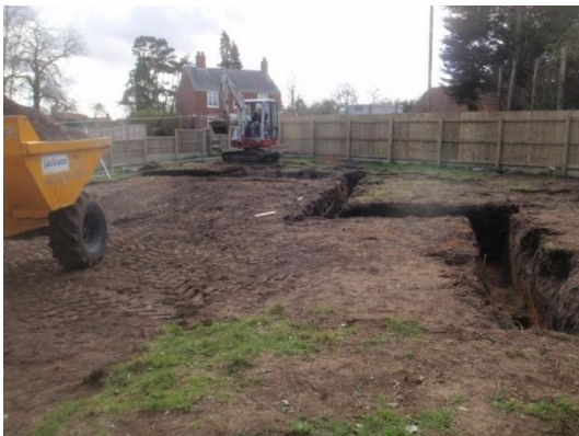
Plate 9: Excavation of the foundations, from the east
