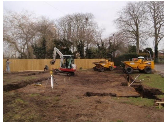
Plate 17: Excavation of the foundations, from the south
