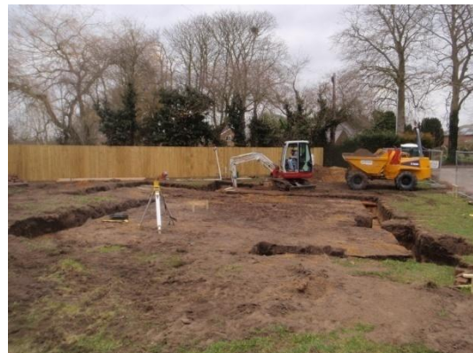
Plate 24: Excavation of the foundations, from the south
