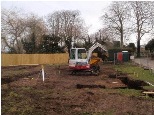
Plate 14: Excavation of the foundations, from the south
