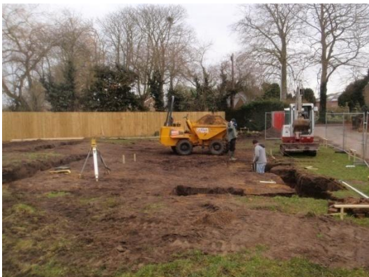
Plate 15: Excavation of the foundations, from the south
