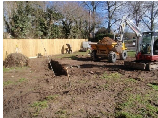
Plate 5: Excavation of the foundations, from the south
