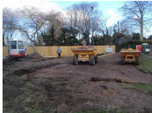
Plate 11: Excavation of the foundations, from the south
