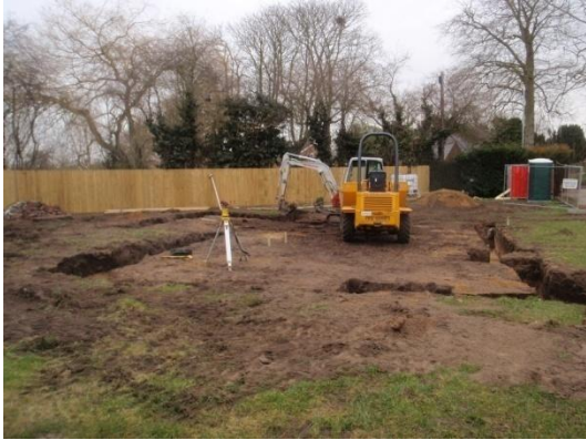
Plate 19: Excavation of the foundations, from the south
