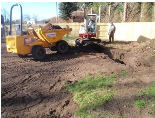
Plate 3: Excavation of the foundations, from the east
