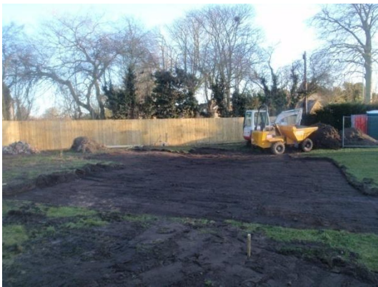
Plate 2: Initial ground reduction, from the south
