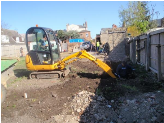
Plate 3: Excavation of the foundations, from the south
