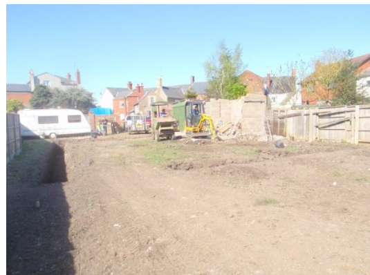
Plate 18: Excavation of the foundations, from the south
