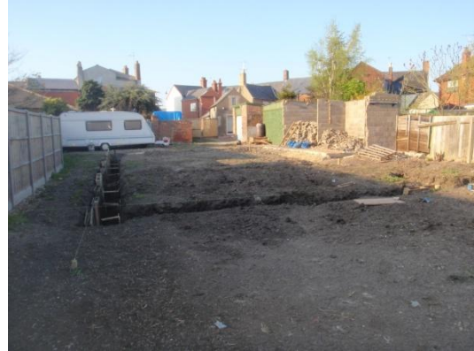
Plate 28: Excavated foundations, from the south
