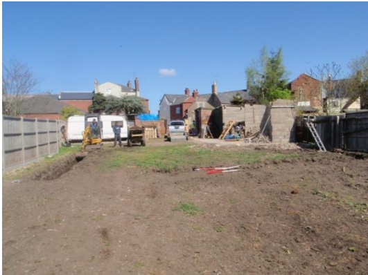
Plate 11: Excavation of the foundations, from the south
