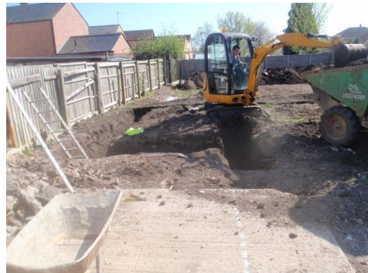
Plate 17: Excavation of the foundations, from the north
