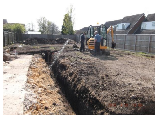
Plate 24: Excavation of the foundations, from the north
