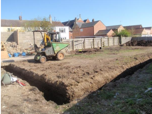
Plate 19: Excavation of the foundations, from the north-west
