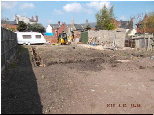
Plate 26: Excavation of the foundations, from the south
