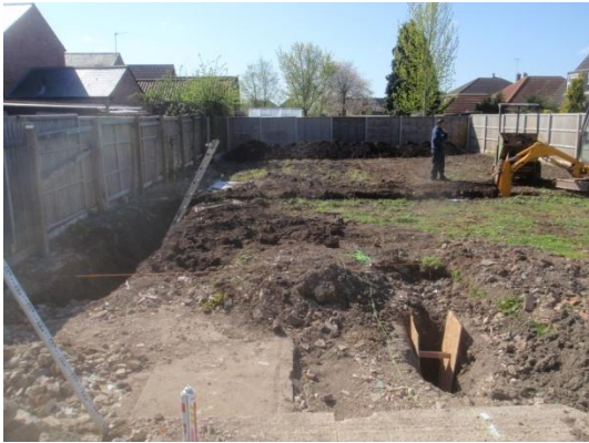
Plate 7: Excavation of the foundations, from the north
