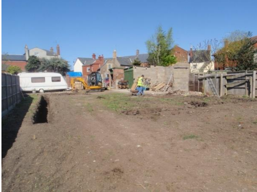
Plate 14: Excavation of the foundations, from the south
