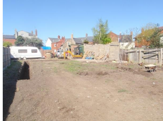
Plate 16: Excavation of the foundations, from the south
