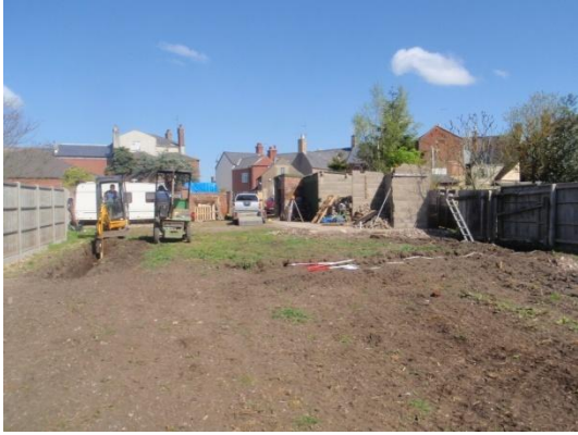
Plate 10: Excavation of the foundations, from the south
