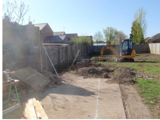
Plate 4: Excavation of the foundations, from the north
