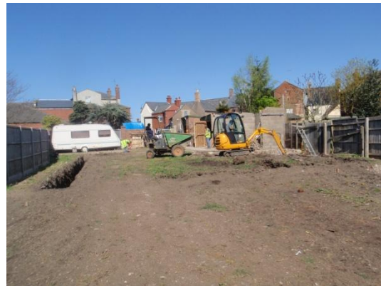
Plate 13: Excavation of the foundations, from the south
