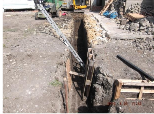
Plate 22: Excavation of the foundations, from the south
