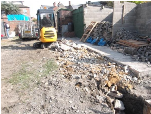
Plate 21: Breaking up of the concrete hardstanding, from the south
