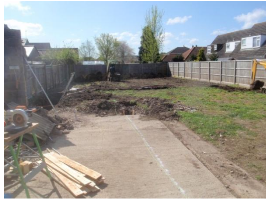
Plate 9: Excavation of the foundations, from the north
