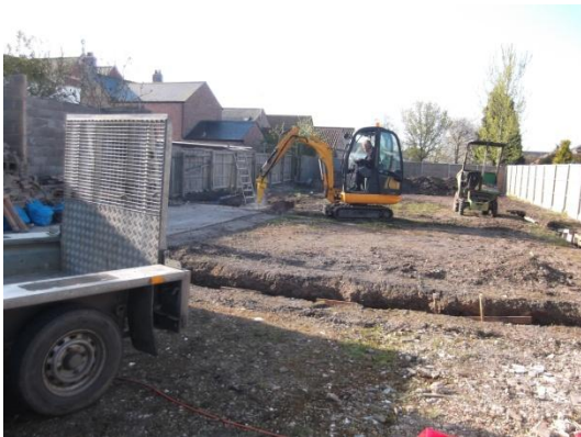
Plate 20: Breaking up of the concrete hardstanding, from the north
