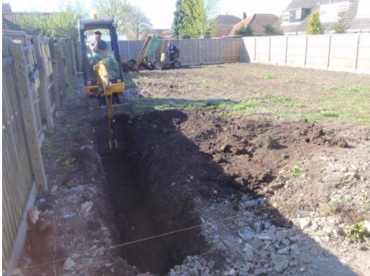
Plate 2: Excavation of the foundations, from the north
