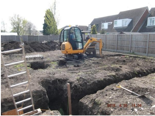
Plate 25: Excavation of the foundations, from the north
