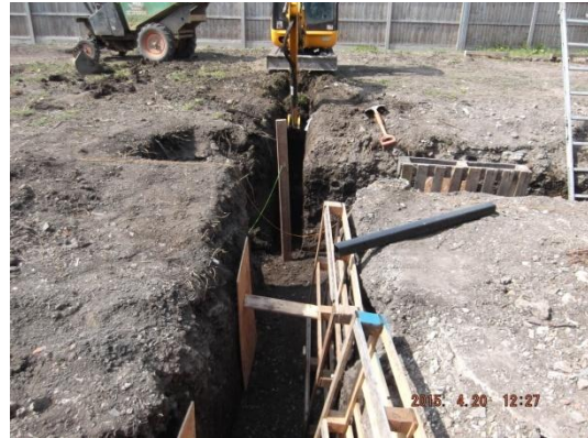
Plate 23: Excavation of the foundations, from the east
