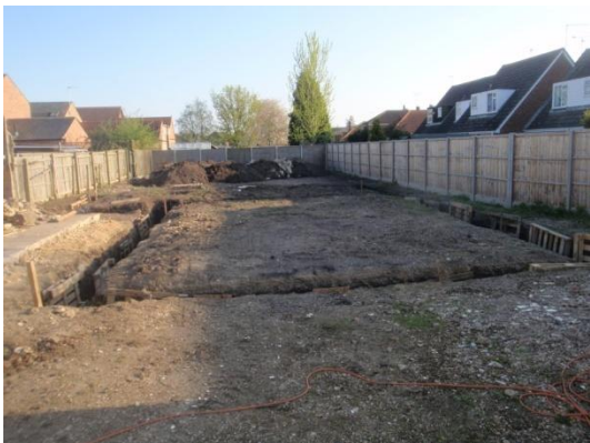
Plate 27: Excavated foundations, from the north
