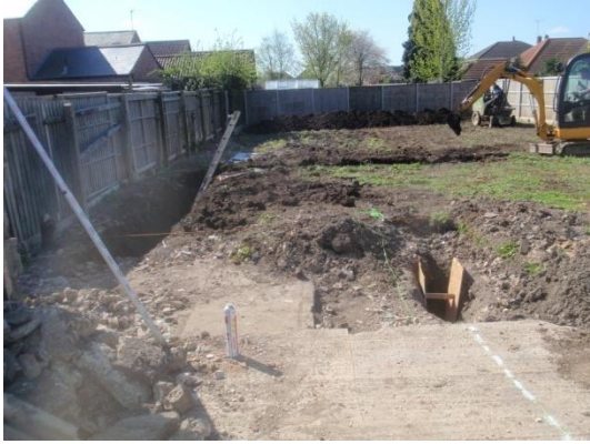
Plate 6: Excavation of the foundations, from the north
