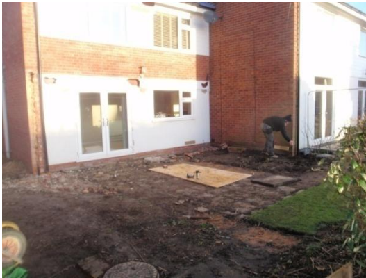
Plate 2: Pre-groundworks, Rear Extension, from the south
