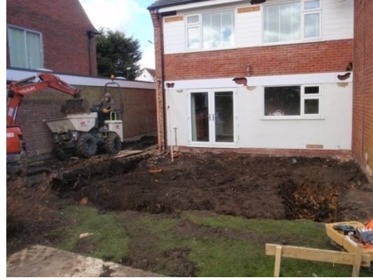
Plate 16: Excavation of the foundations, from the east
