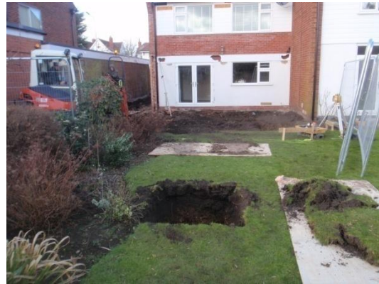
Plate 17: The groundworks, Rear Extension, from the east
