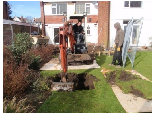
Plate 12: Excavation of the first soakaway, from the east
