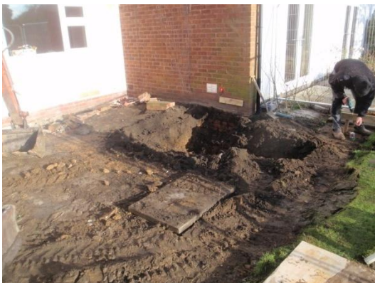
Plate 3: Excavation of the foundations, from the south
