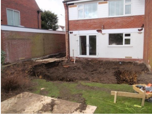
Plate 19: Excavated foundations, from the east
