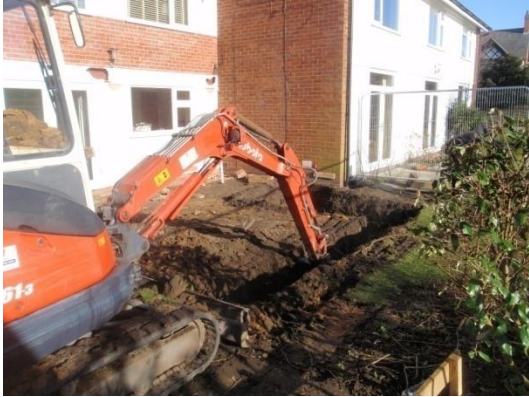
Plate 7: Excavation of the foundations, from the south
