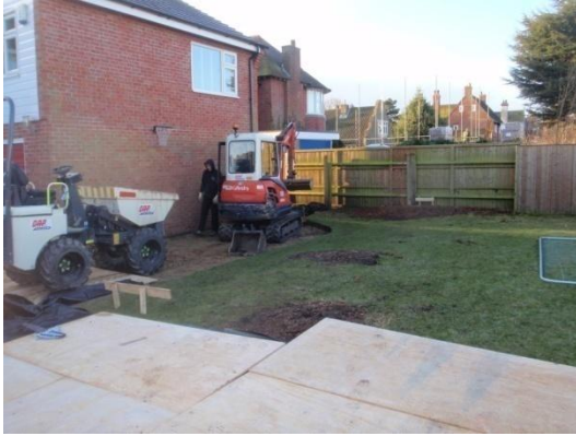
Plate 1: Pre-groundworks, Front Extension, from the north
