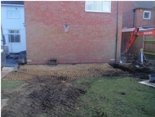
Plate 20: Excavation of the foundations, from the west
