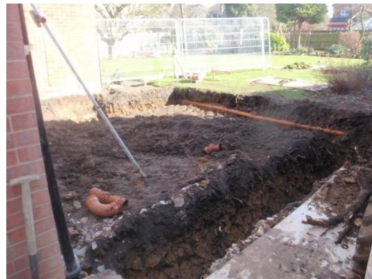
Plate 18: Excavated foundations, from the south-west
