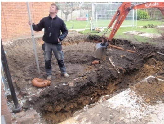
Plate 15: Excavation of the foundations, from the south-west
