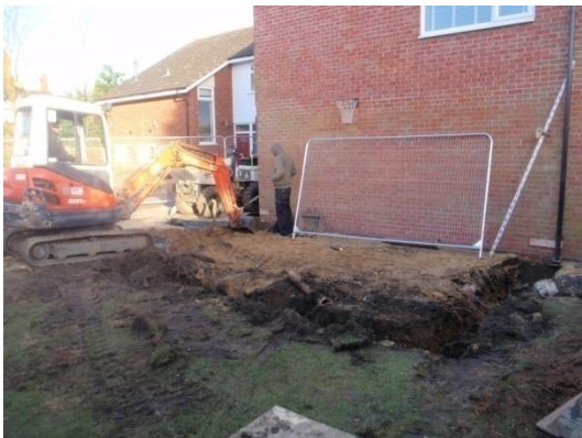
Plate 26: Excavation of the foundations, from the south-west
