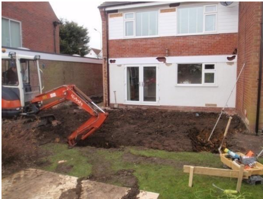
Plate 14: Excavation of the foundations, from the east
