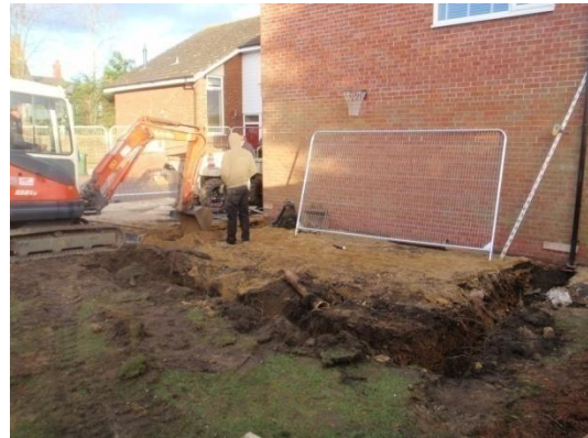
Plate 28: Excavation of the foundations, from the south-west
