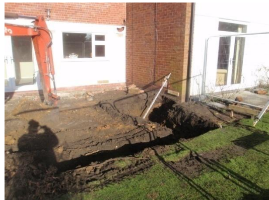
Plate 6: Excavation of the foundations, from the south-east
