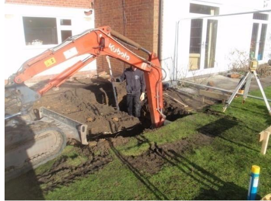
Plate 4: Excavation of the foundations, from the south-east
