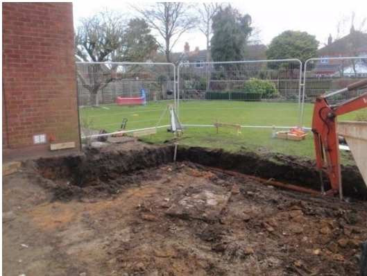
Plate 8: Excavation of the foundations, from the south-west
