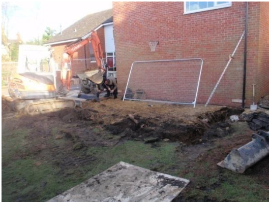
Plate 25: Excavation of the foundations, from the south-west
