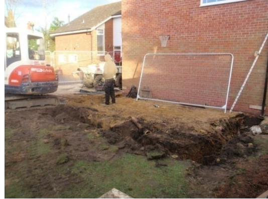
Plate 27: Excavation of the foundations, from the south-west
