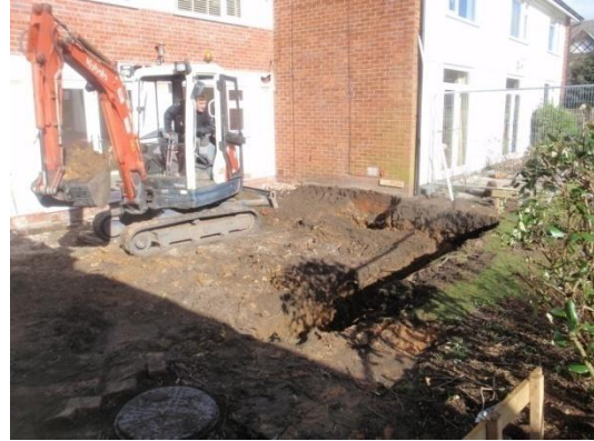
Plate 10: Excavation of the foundations, from the south
