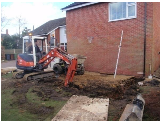
Plate 21: Excavation of the foundations, from the south-west
