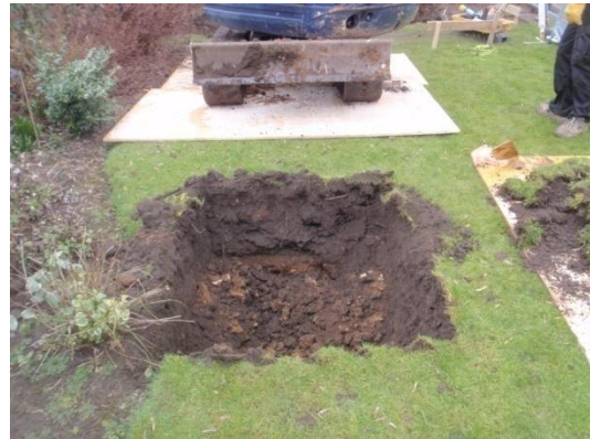
Plate 11: Excavation of the first soakaway, from the east
