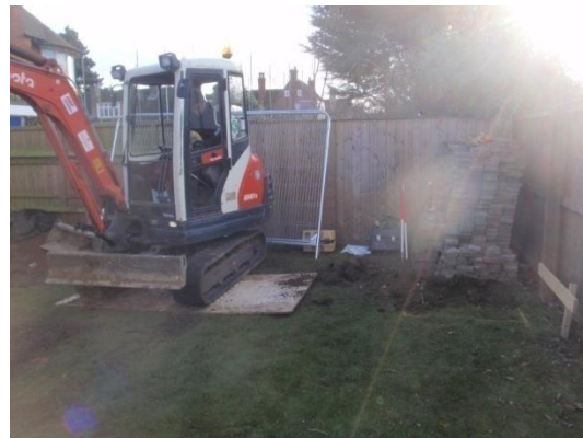
Plate 23: Excavation of the second soakaway, from the north
