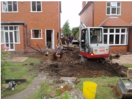
Plate 20: Ground reduction within the new build footprints, from the south
