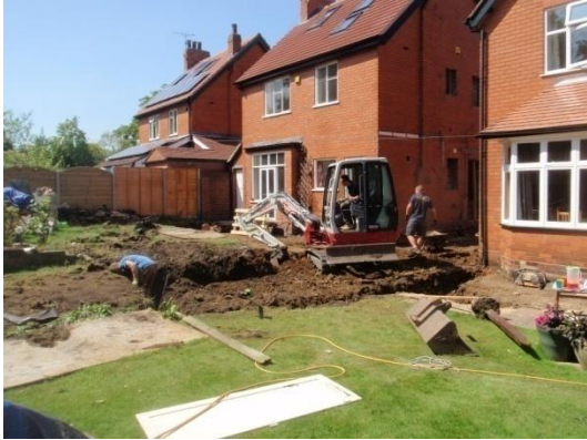
Plate 37: Excavation of the foundations, from the south-east
