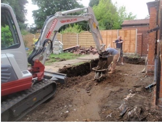
Plate 13: Excavation of the foundations, from the east
