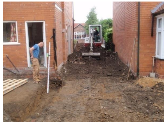
Plate 23: Ground reduction within the new build footprints, from the south
