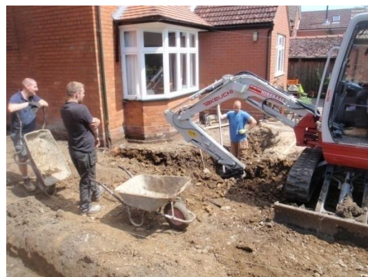
Plate 30: Excavation of the foundations, from the west
