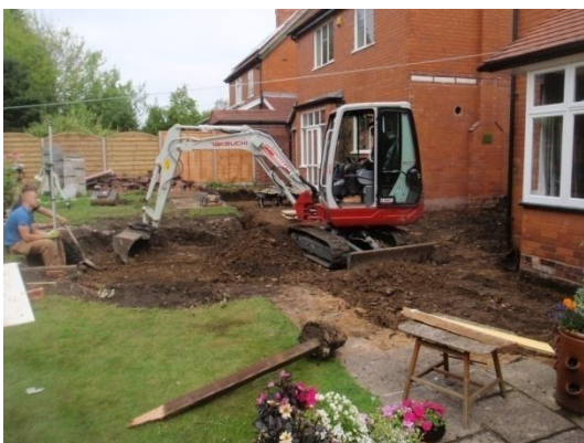
Plate 27: Ground reduction within the new build footprints, from the east
