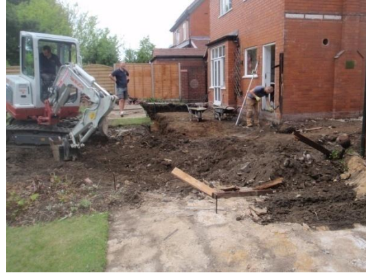
Plate 16: Excavation of the foundations, from the east
