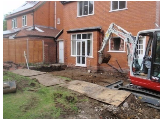
Plate 11: Excavation of the foundations, from the south-east
