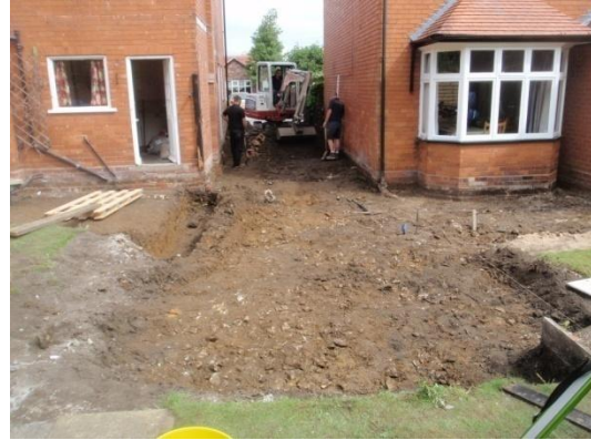
Plate 28: Ground reduction within the new build footprints, from the south
