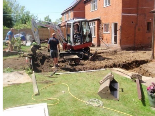
Plate 34: Excavation of the foundations, from the south-east
