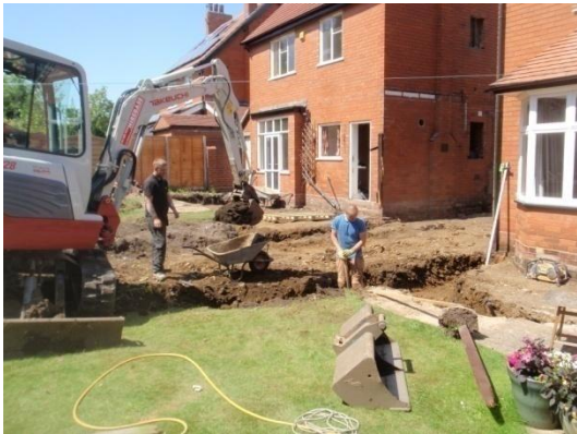
Plate 32: Excavation of the foundations, from the south-east
