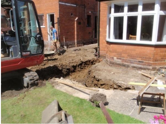
Plate 31: Excavation of the foundations, from the south-east
