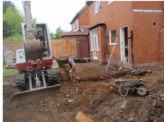
Plate 17: Excavation of the foundations, from the east
