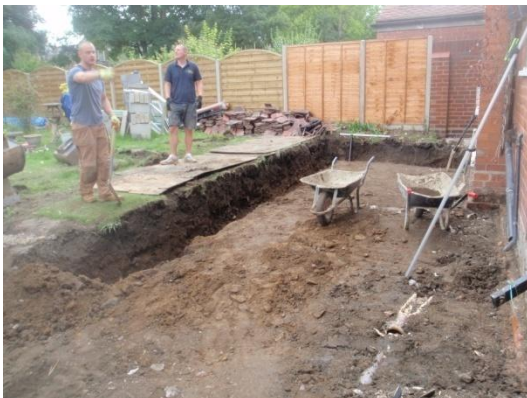
Plate 15: Excavation of the foundations, from the east
