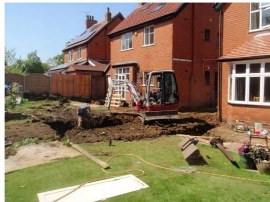
Plate 36: Excavation of the foundations, from the south-east
