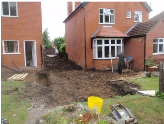
Plate 26: Ground reduction within the new build footprints, from the south
