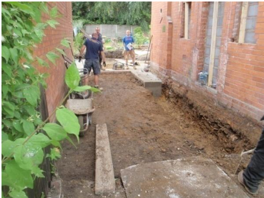
Plate 38: Excavation of the foundations, from the north
