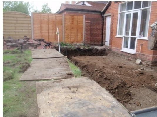
Plate 12: Excavation of the foundations, from the east
