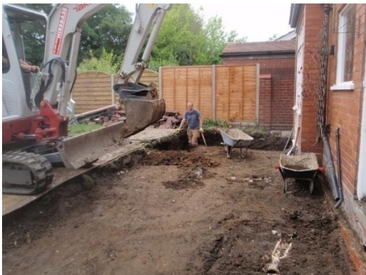
Plate 9: Excavation of the foundations, from the east
