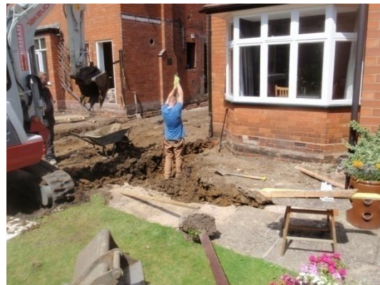
Plate 29: Excavation of the foundations, from the south-east
