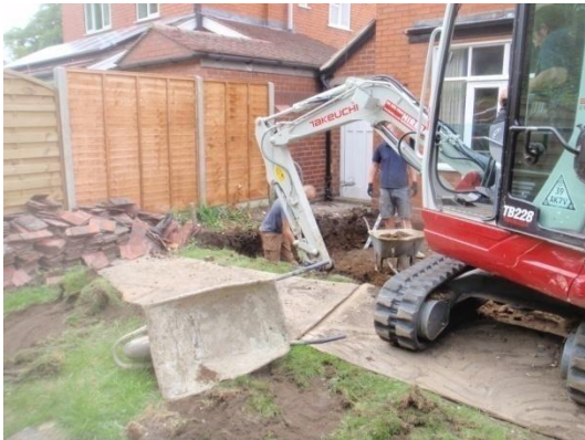
Plate 8: Excavation of the foundations, from the south-east
