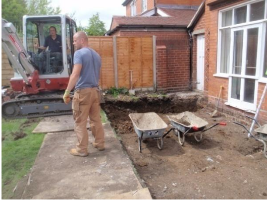
Plate 7: Excavation of the foundations, from the east
