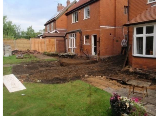
Plate 22: Ground reduction within the new build footprints, from the east
