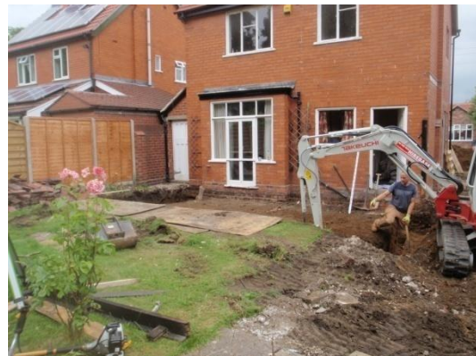
Plate 18: Excavation of the foundations, from the south-east
