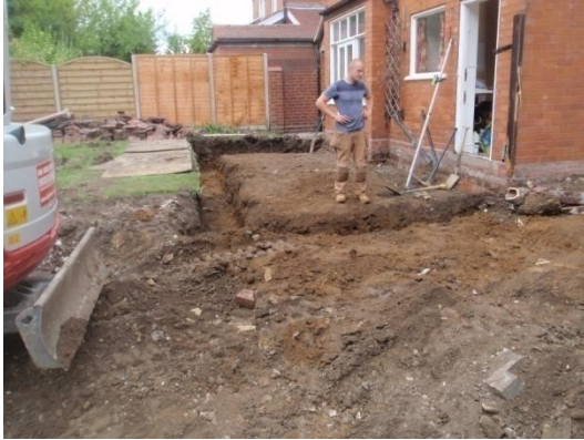
Plate 19: Excavation of the foundations, from the east
