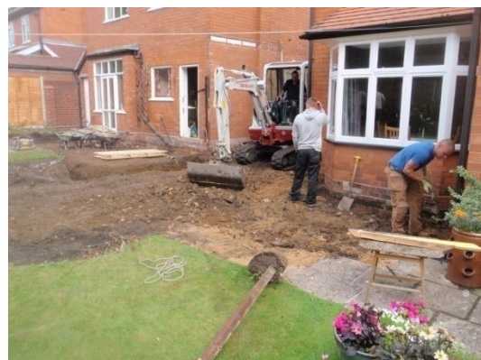
Plate 24: Ground reduction within the new build footprints, from the south-east
