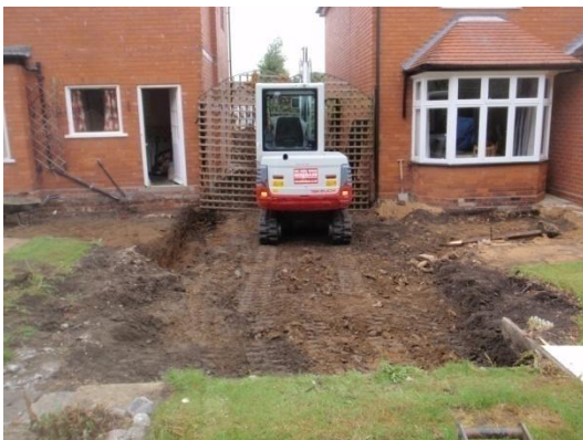
Plate 21: Ground reduction within the new build footprints, from the south
