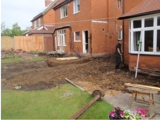
Plate 25: Ground reduction within the new build footprints, from the south-east
