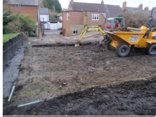
Plate 34: Excavation of the foundations, from the north
