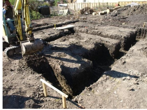
Plate 87: Excavation of the foundations, from the north-east
