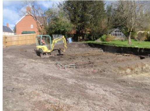
Plate 41: Excavation of the foundations, from the south-west
