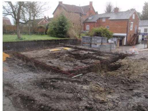
Plate 54: Completed foundation excavations, from the north-west
