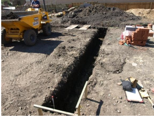
Plate 85: Excavation of the foundations, from the north
