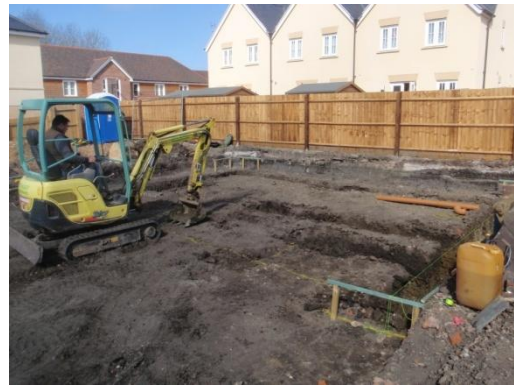
Plate 77: Excavation of the foundations, from the south
