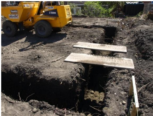
Plate 86: Excavation of the foundations, from the east
