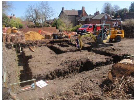
Plate 83: Excavation of the foundations, from the west
