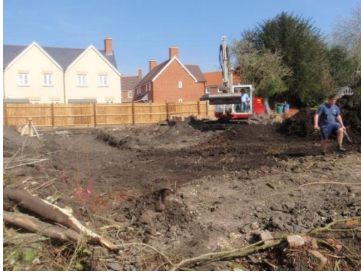
Plate 61: Ground reduction, from the south
