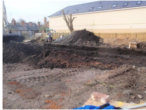
Plate 58: Ground reduction, from the north-east
