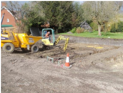
Plate 50: Excavation of the foundations, from the south-west
