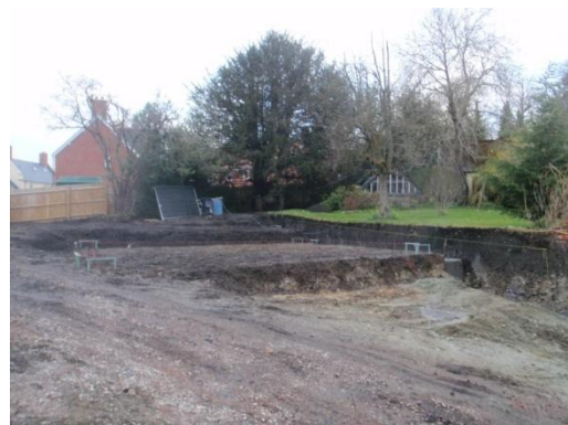
Plate 30: House Plot 1, set out, boundary wall & reduced areas, from the south-west
