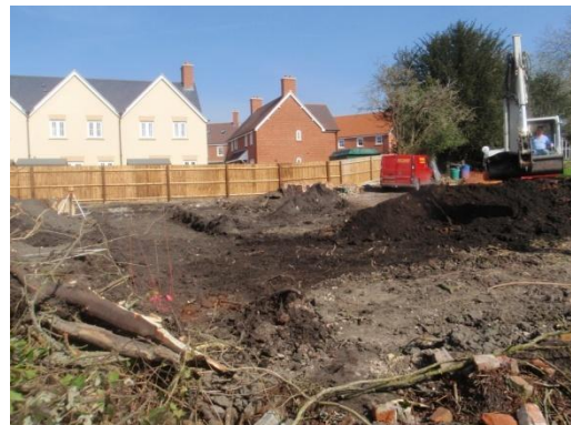
Plate 60: Ground reduction, from the south
