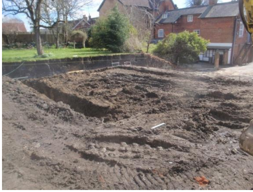
Plate 43: Excavation of the foundations, from the west
