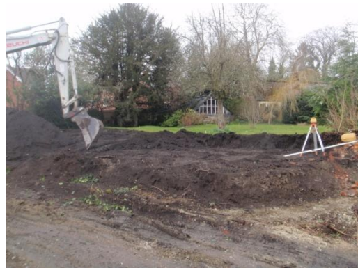
Plate 23: Ground reduction, from the west
