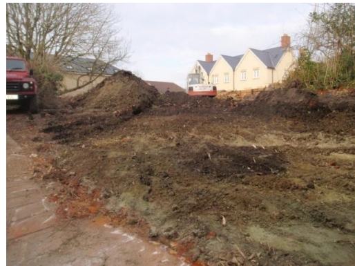
Plate 11: Ground reduction, from the south
