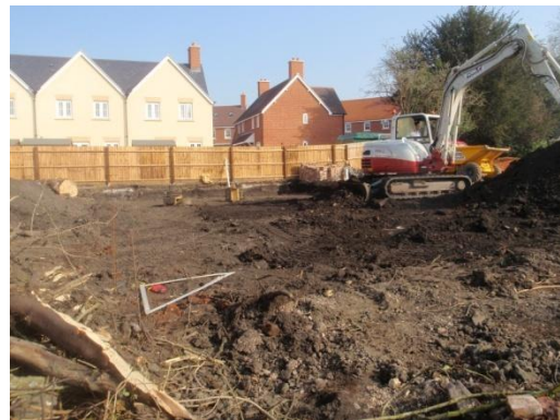
Plate 66: Ground reduction, from the south
