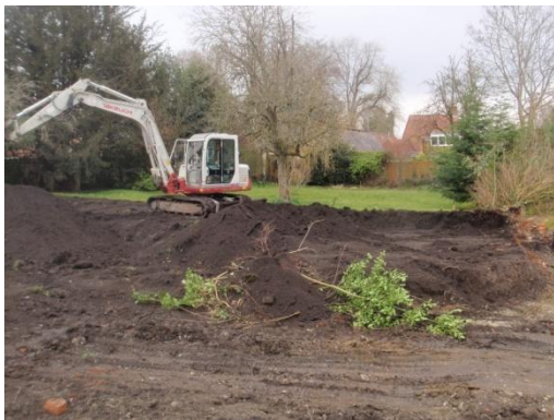
Plate 21: Ground reduction, from the west
