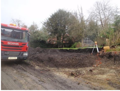
Plate 25: Ground reduction, from the south
