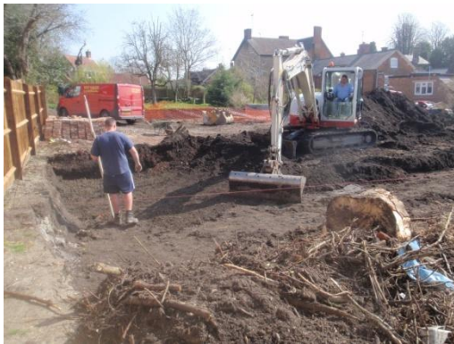
Plate 62: Ground reduction, from the west
