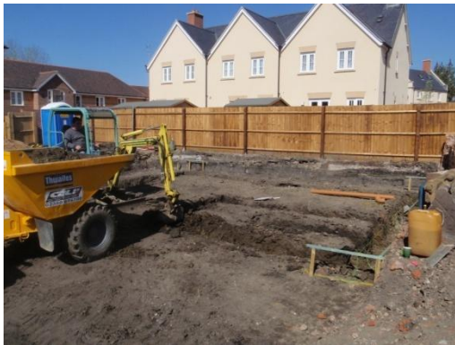
Plate 80: Excavation of the foundations, from the south
