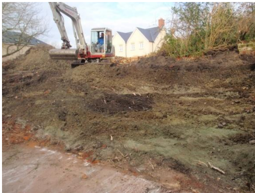
Plate 8: Ground reduction, from the south
