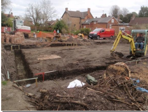
Plate 73: Excavation of the foundations, from the west
