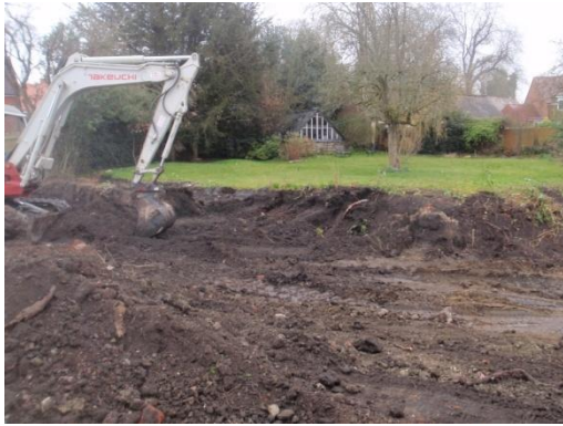
Plate 14: Ground reduction, from the south-west
