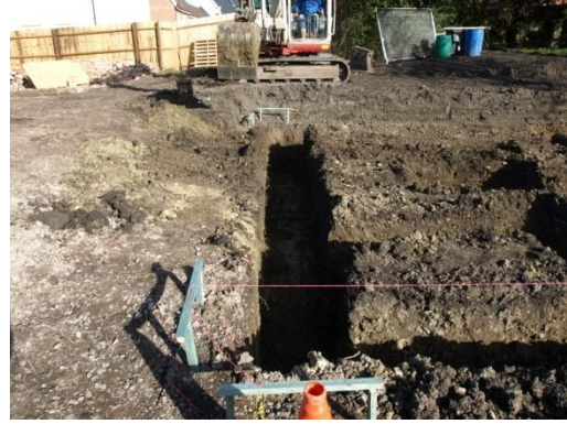
Plate 52: Excavation of the foundations, from the south
