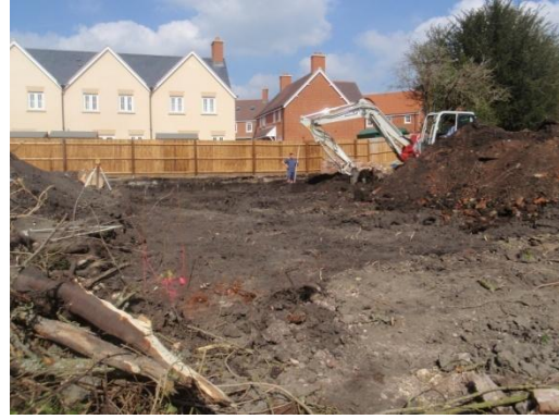
Plate 64: Ground reduction, from the south
