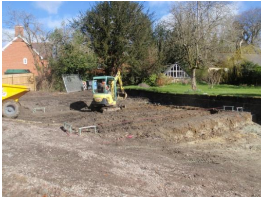
Plate 38: Excavation of the foundations, from the south-west
