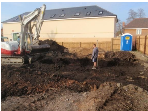
Plate 57: Ground reduction, from the east
