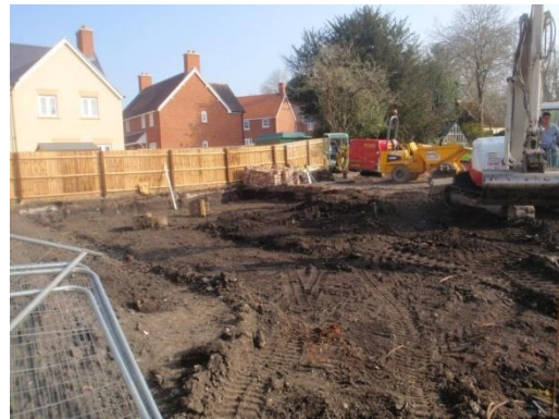
Plate 65: Ground reduction, from the south
