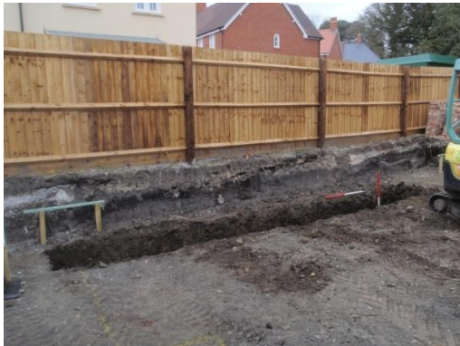
Plate 69: Excavation of the foundations, from the south
