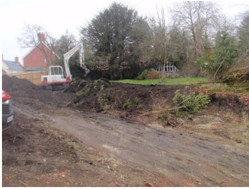
Plate 19: Ground reduction, from the south
