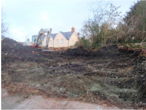
Plate 1: Ground reduction, from the south
