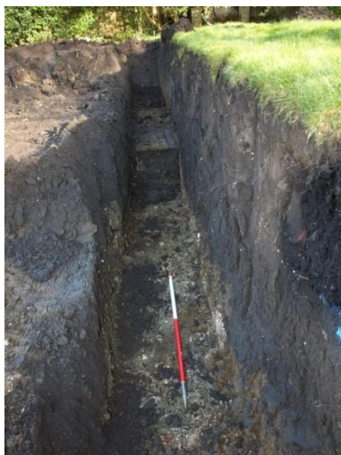
Plate 27: The boundary wall foundation trench, from the south
