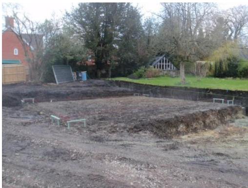
Plate 32: House Plot 1, set out, from the south-west
