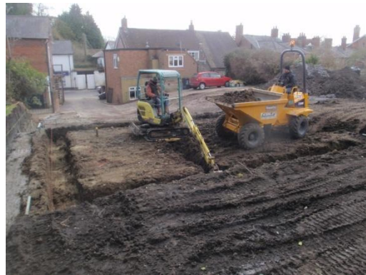
Plate 47: Excavation of the foundations, from the north
