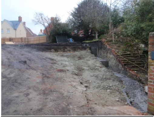
Plate 31: House Plot 1, set out, boundary wall & reduced areas, from the south
