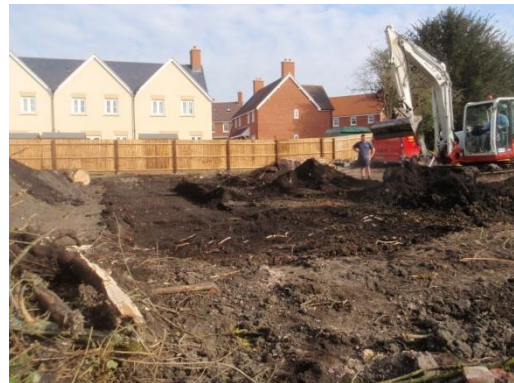
Plate 59: Ground reduction, from the south
