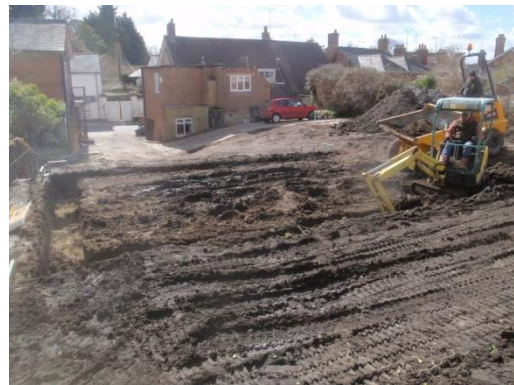
Plate 42: Excavation of the foundations, from the north
