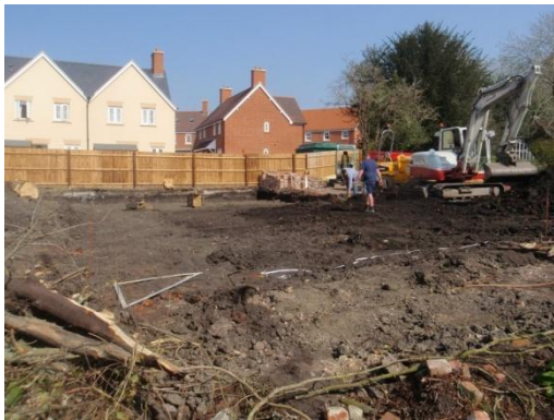
Plate 68: Ground reduction, from the south
