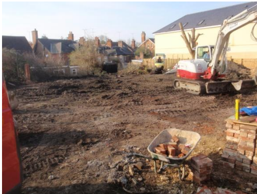
Plate 55: Ground reduction, from the east
