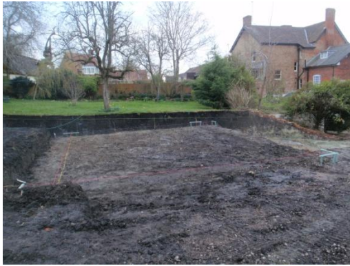
Plate 33: House Plot 1, set out, from the west
