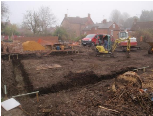
Plate 74: Excavation of the foundations, from the west
