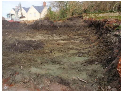
Plate 12: Ground reduction, from the south
