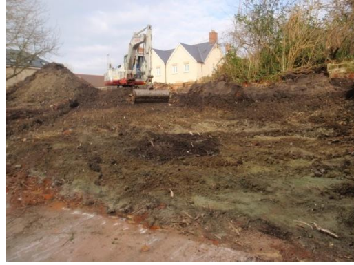
Plate 10: Ground reduction, from the south
