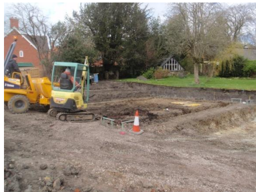
Plate 48: Excavation of the foundations, from the south-west
