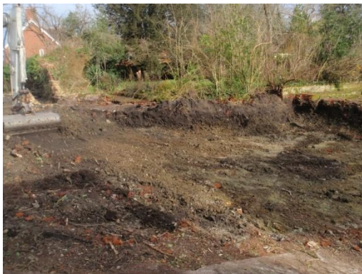
Plate 9: Ground reduction, from the south-west
