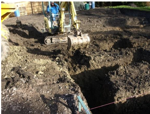
Plate 51: Excavation of the foundations, from the east
