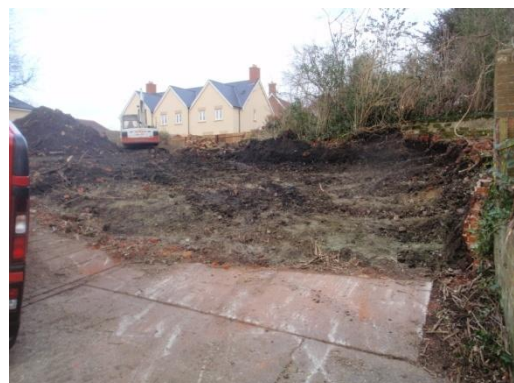
Plate 6: Ground reduction, from the south
