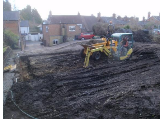
Plate 40: Excavation of the foundations, from the north
