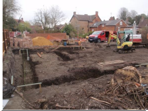
Plate 76: Excavation of the foundations, from the west
