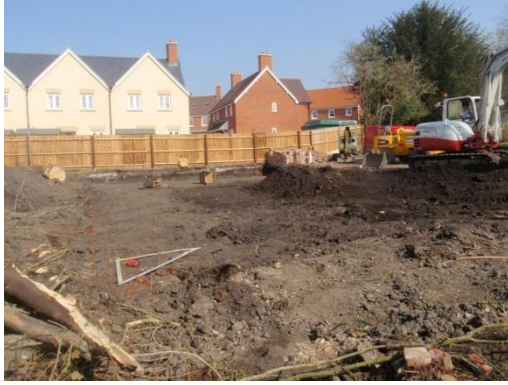
Plate 67: Ground reduction, from the south
