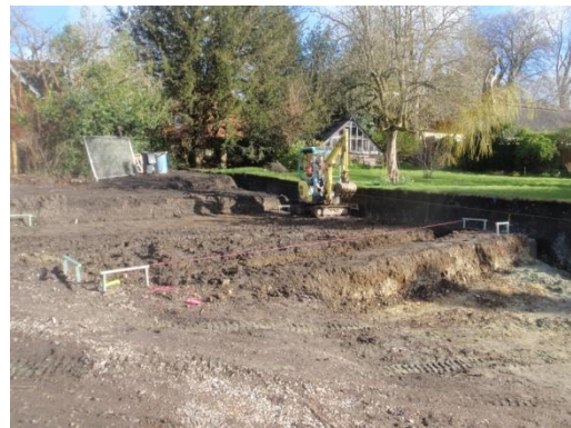
Plate 36: Excavation of the foundations, from the south-west
