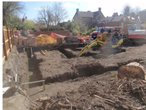
Plate 78: Excavation of the foundations, from the west
