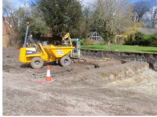
Plate 46: Excavation of the foundations, from the south-west
