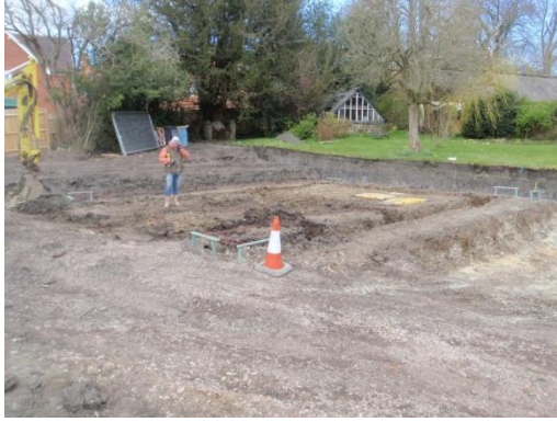
Plate 49: Excavation of the foundations, from the south-west
