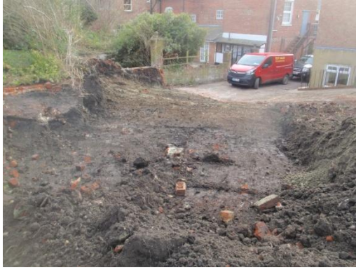
Plate 13: Ground reduction, from the north-west
