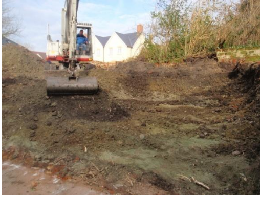
Plate 7: Ground reduction, from the south
