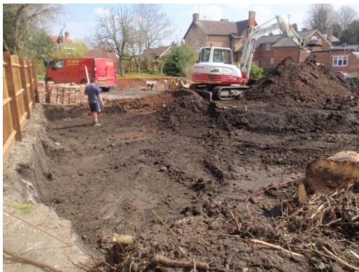
Plate 63: Ground reduction, from the west
