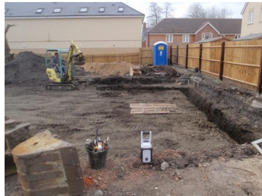
Plate 71: Excavation of the foundations, from the east
