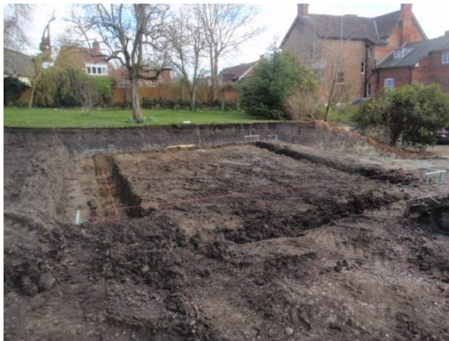
Plate 44: Excavation of the foundations, from the west
