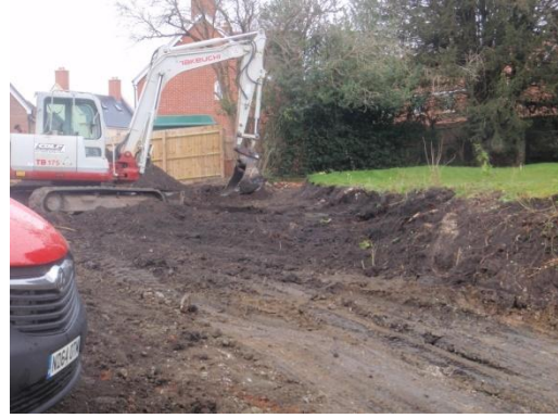
Plate 16: Ground reduction, from the south-west
