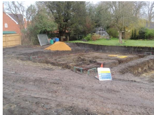
Plate 53: Completed foundation excavations, from the south-west
