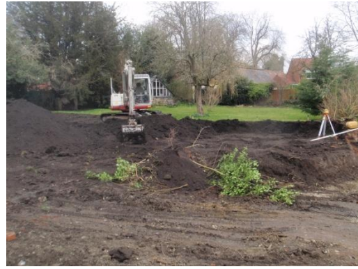
Plate 22: Ground reduction, from the west
