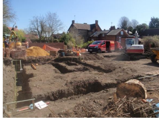
Plate 82: Excavation of the foundations, from the west
