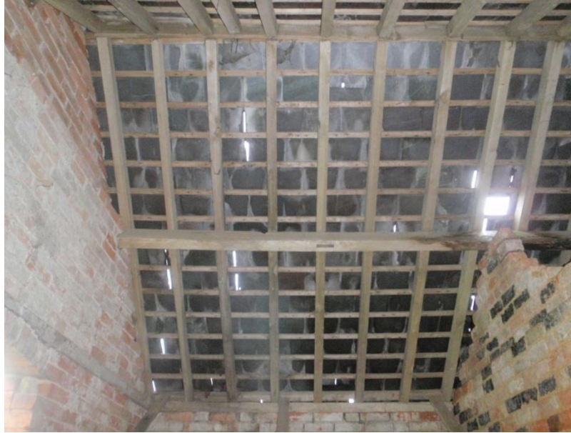
Plate 23: View of the roof of Cell 2, from the south
