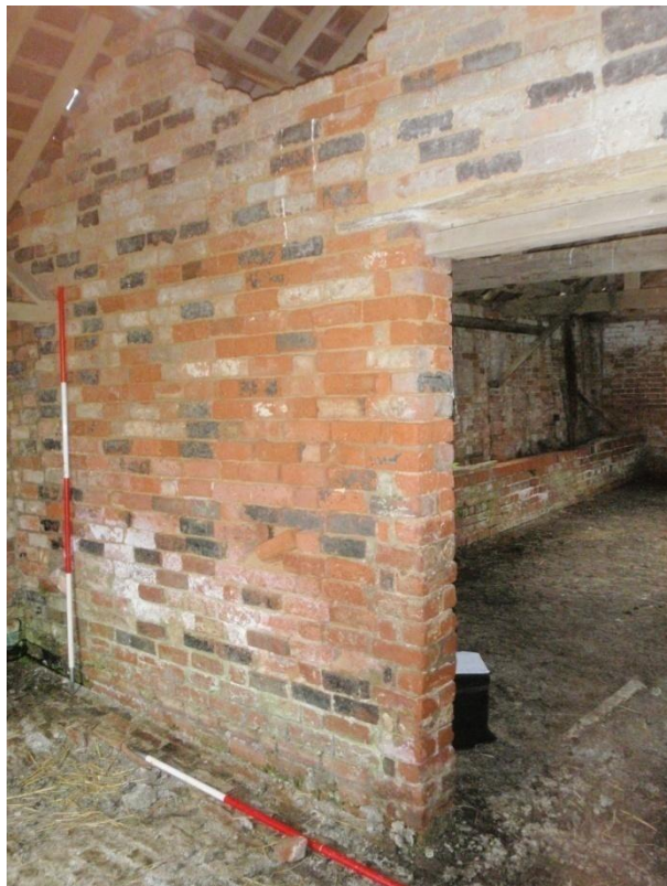
Plate 21: View of the East Wall (Internal Partition Wall), from the south-west
