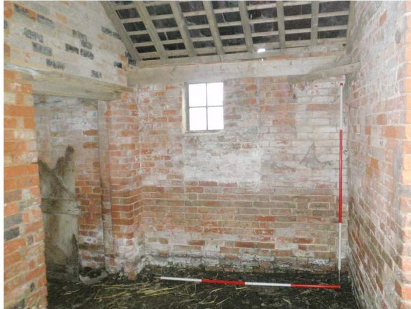
Plate 20: View of the floor and South Wall, from the north
