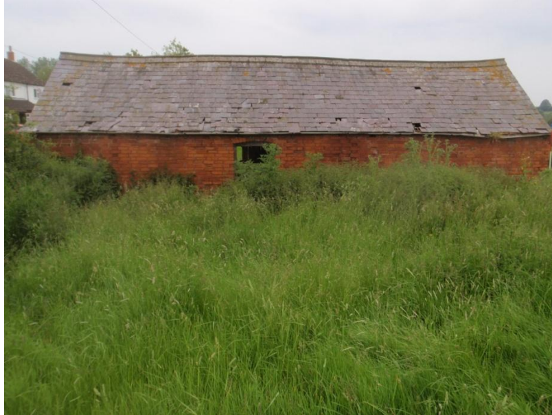
Plate 2: The North Elevation, from the north
