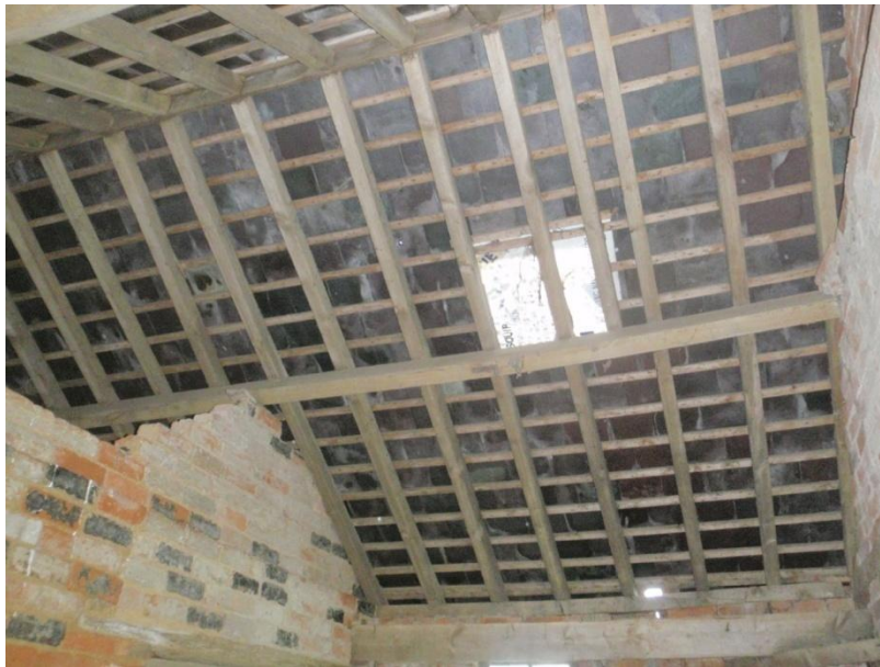
Plate 24: View of the roof of Cell 2, from the north
