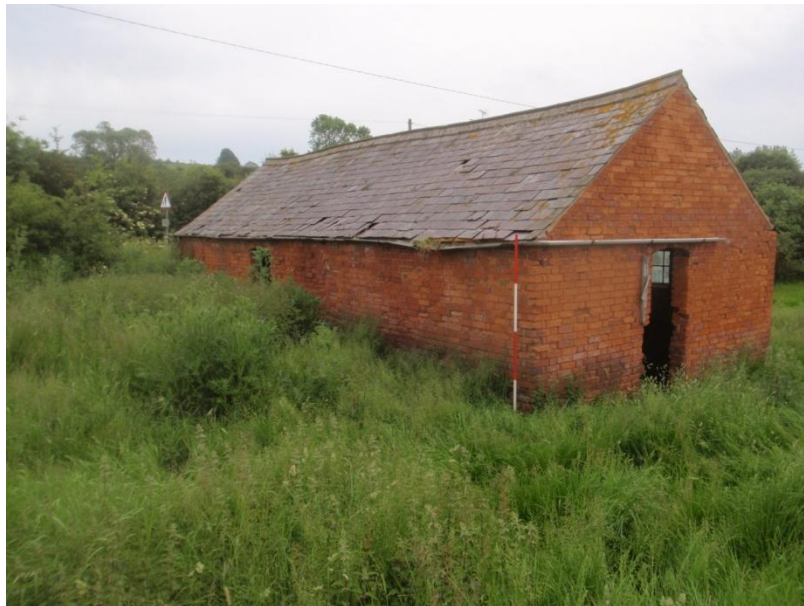
Plate 3: The North and West Elevations, from the north-west
