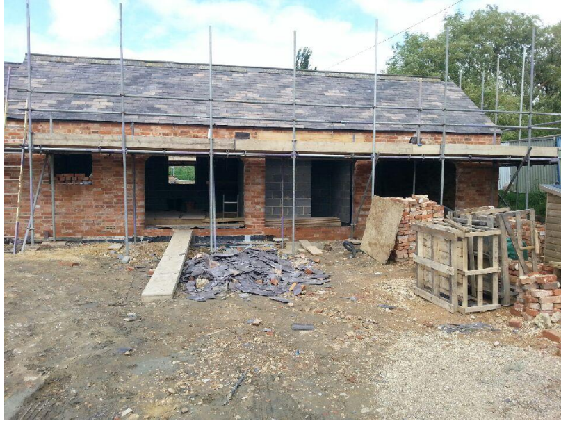
Plate 27: View of the new South Elevation, from the south
