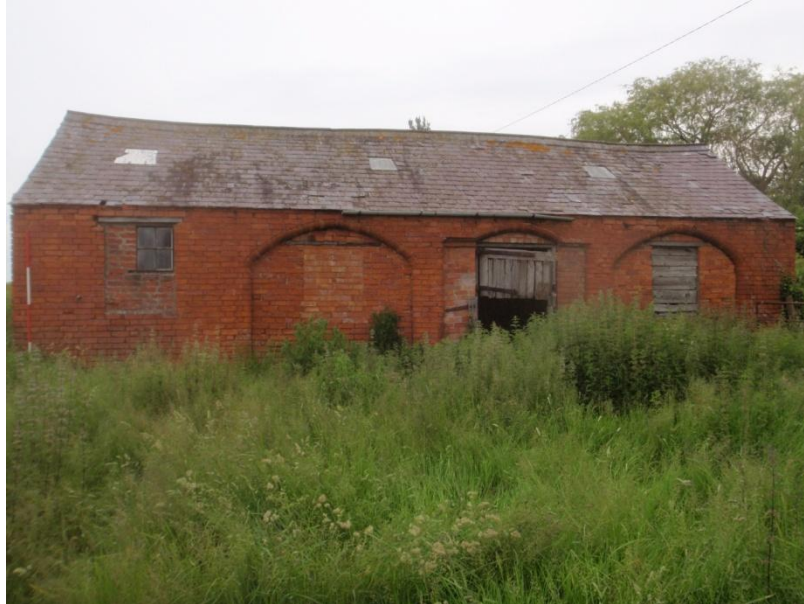
Plate 6: View of the South Elevation, from the south
