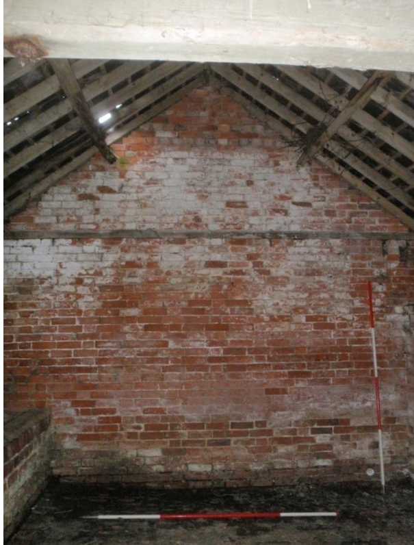
Plate 12: View of the East Wall, from the west
