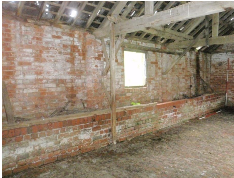
Plate 16: View of the South Wall, from the south-west
