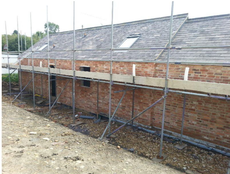
Plate 29: View of the new North Elevation, from the north-east
