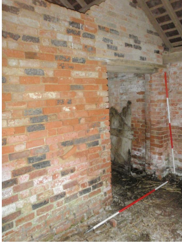
Plate 22: View of the East Wall (Internal Partition Wall), from the north-west
