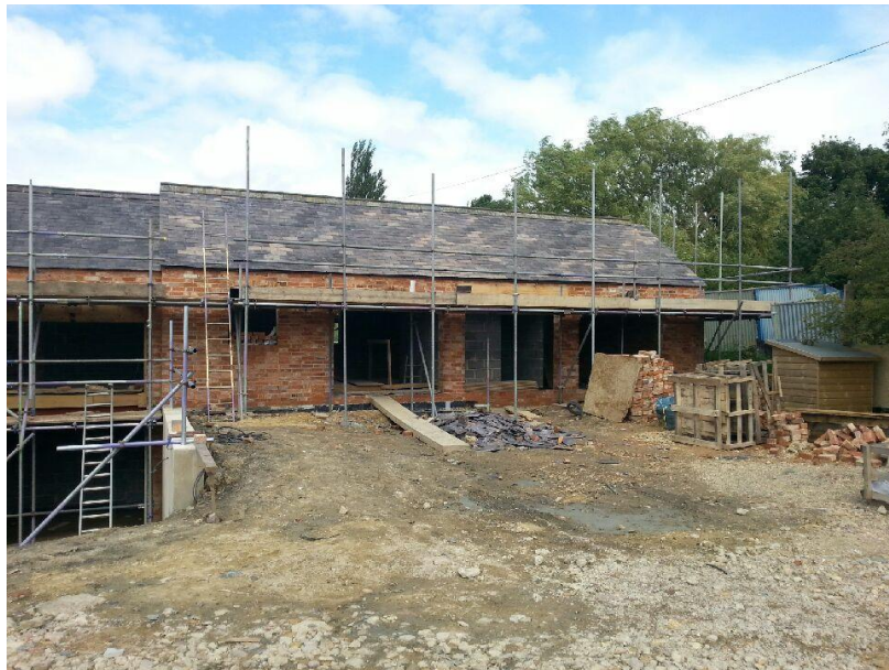
Plate 28: View of the new South Elevation and extension, from the south
