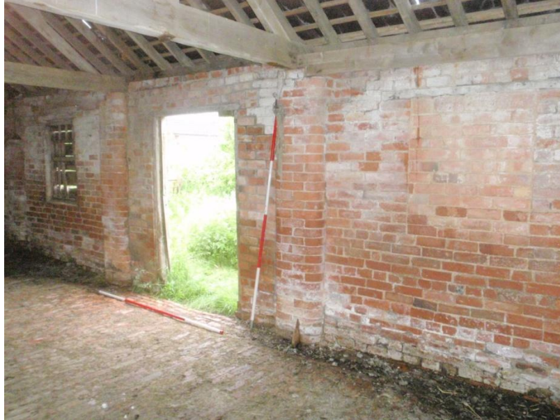
Plate 14: View of the South Wall, from the north-west
