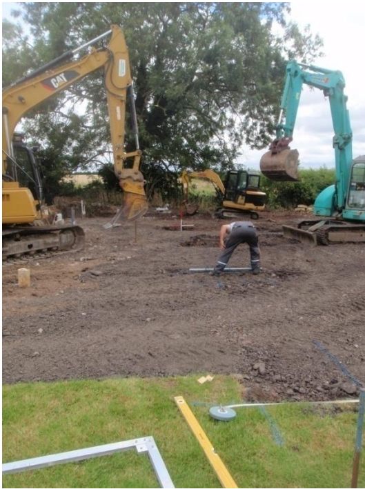
Plate 36: Excavation of the Stanchion Bases, from the west
