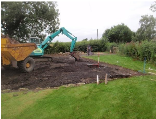
Plate 24: Excavation of the Stanchion Bases, from the west
