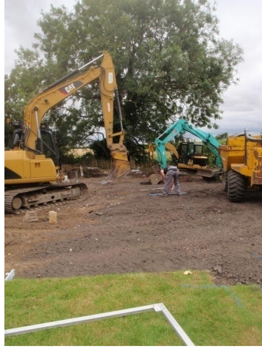
Plate 33: Excavation of the Stanchion Bases, from the west
