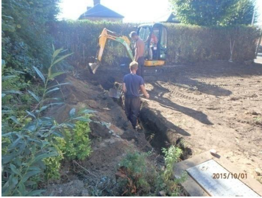
Plate 7: Excavation of the service trench, from the north
