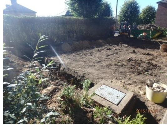
Plate 10: Excavation of the service trench, from the north-east
