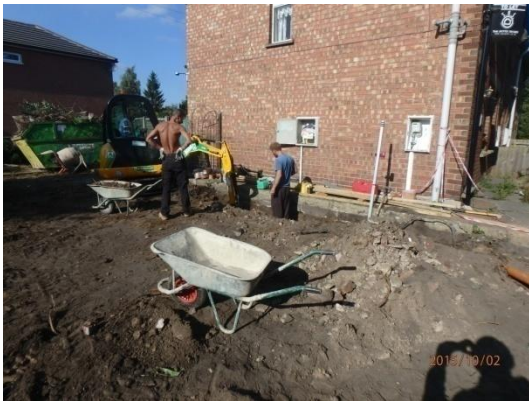
Plate 15: Excavation of the foundations, from the south
