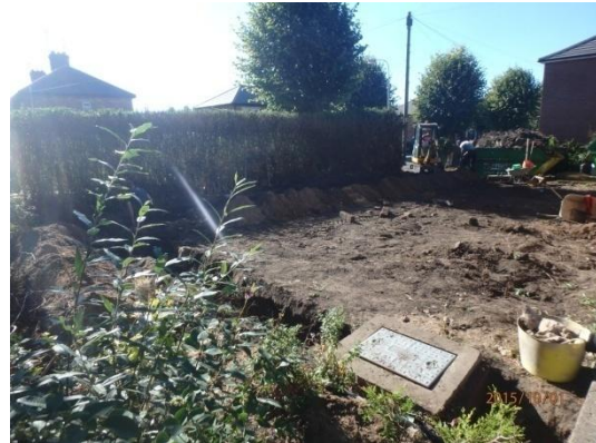
Plate 11: Excavation of the service trench, from the north-east
