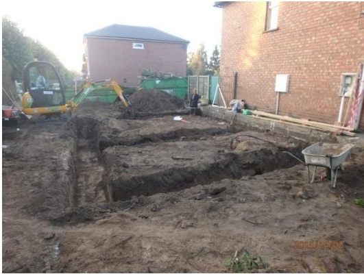
Plate 26: Excavation of the foundations, from the east
