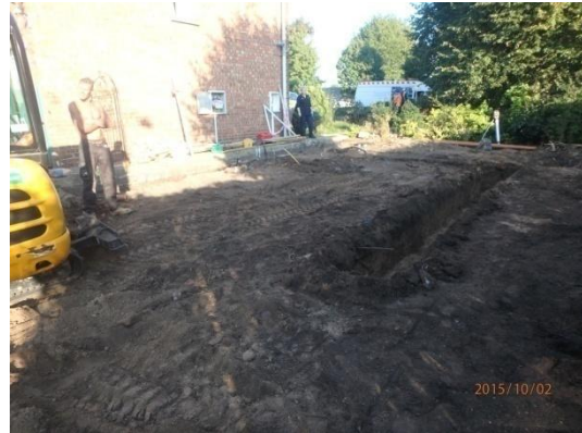
Plate 23: Excavation of the foundations, from the west
