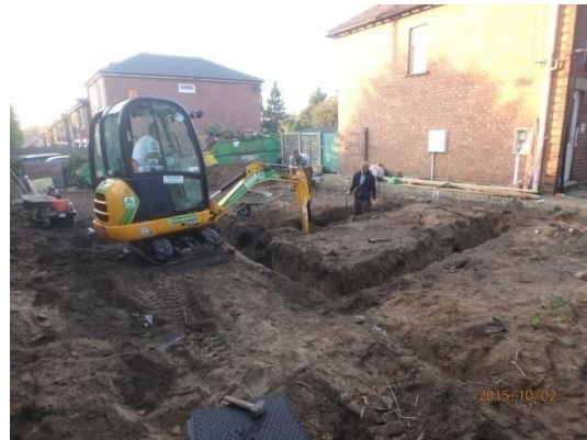
Plate 24: Excavation of the foundations, from the east
