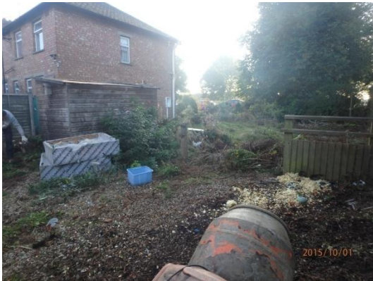
Plate 2: Pre-groundworks, from the west
