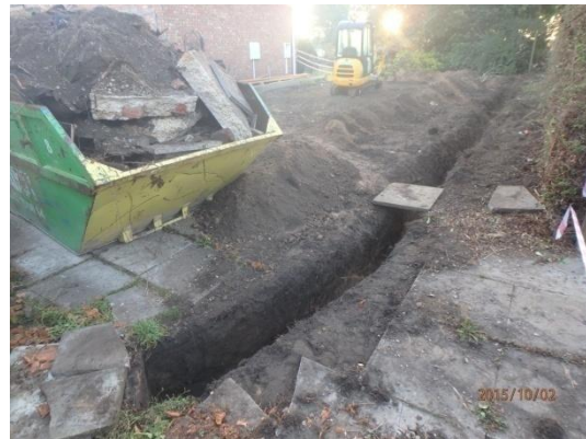
Plate 12: Excavated service trench, from the west
