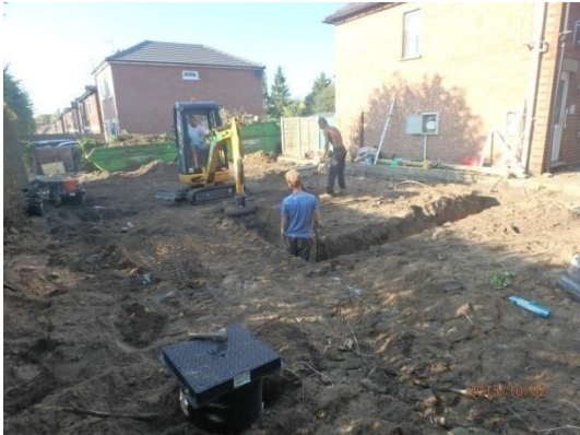
Plate 20: Excavation of the foundations, from the east
