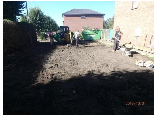
Plate 5: Initial ground reduction, from the east
