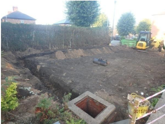
Plate 14: Excavated service trench, from the north-east
