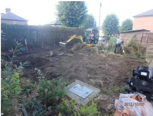
Plate 3: Initial ground reduction, from the east
