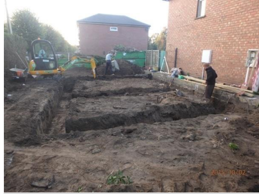
Plate 28: Excavation of the foundations, from the east
