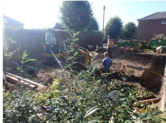
Plate 17: Excavation of the foundations, from the east
