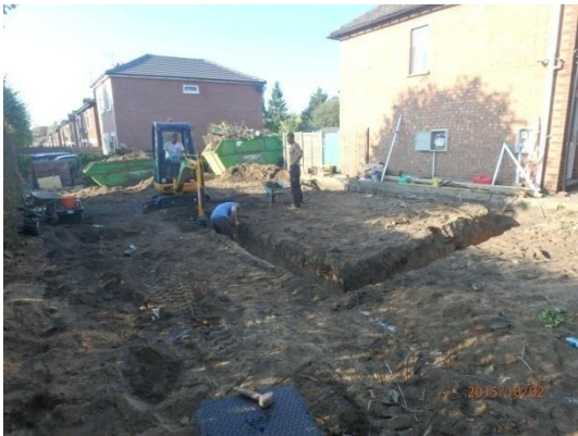
Plate 21: Excavation of the foundations, from the east
