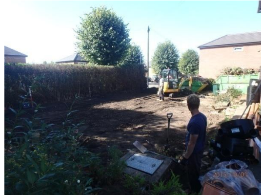
Plate 4: Initial ground reduction, from the east
