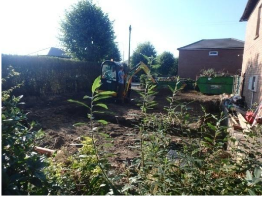
Plate 19: Excavation of the foundations, from the east
