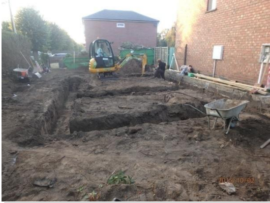
Plate 25: Excavation of the foundations, from the east
