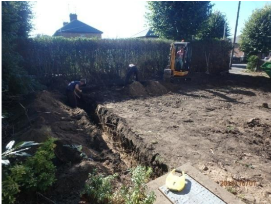
Plate 8: Excavation of the service trench, from the north
