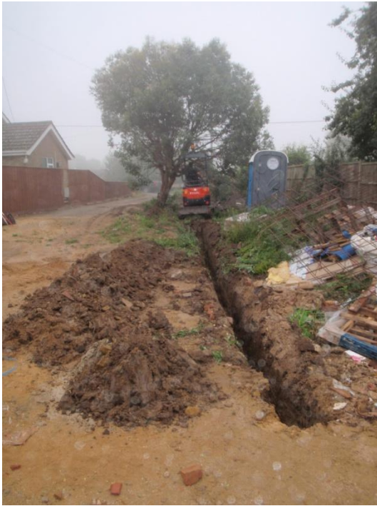
Plate 36: Service trench excavation, from the west
