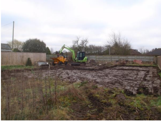
Plate 1: Initial ground reduction, from the north
