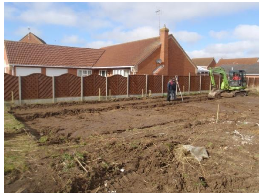
Plate 5: Excavation of the foundations, from the east
