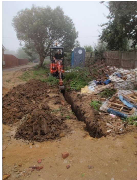
Plate 34: Service trench excavation, from the west
