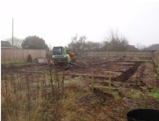
Plate 19: Excavation of the foundations, from the north
