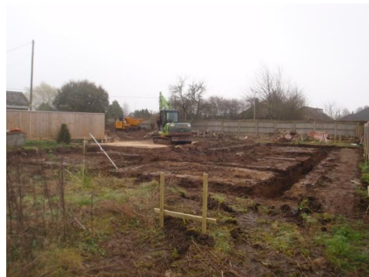
Plate 22: Excavation of the foundations, from the north
