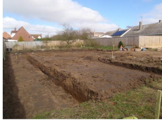
Plate 10: Excavation of the foundations, from the south
