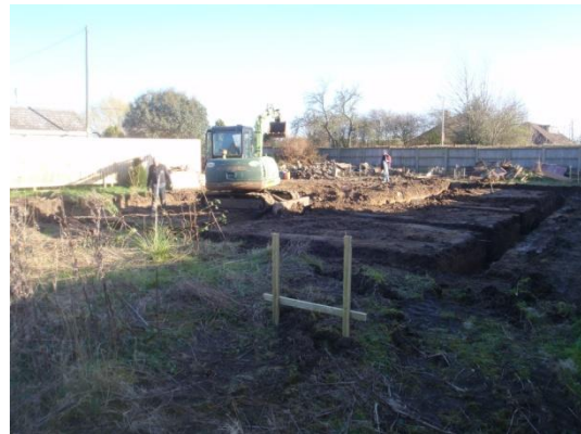
Plate 17: Excavation of the foundations, from the north
