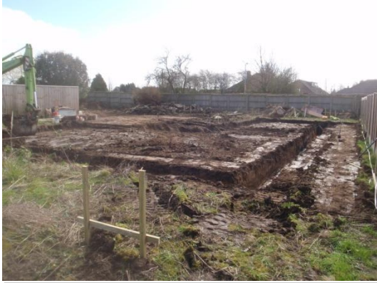
Plate 7: Excavation of the foundations, from the north
