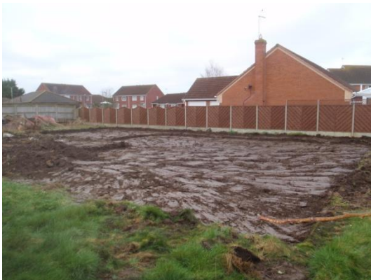
Plate 2: Initial ground reduction, from the east
