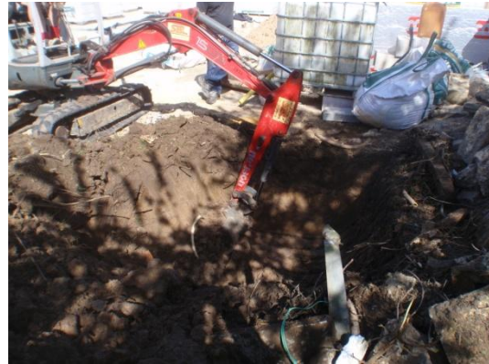
Plate 28: Excavation of the first soakaway, from the east
