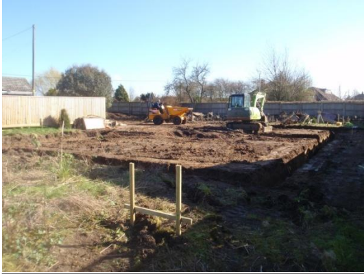
Plate 13: Excavation of the foundations, from the north
