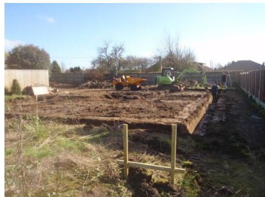
Plate 12: Excavation of the foundations, from the north
