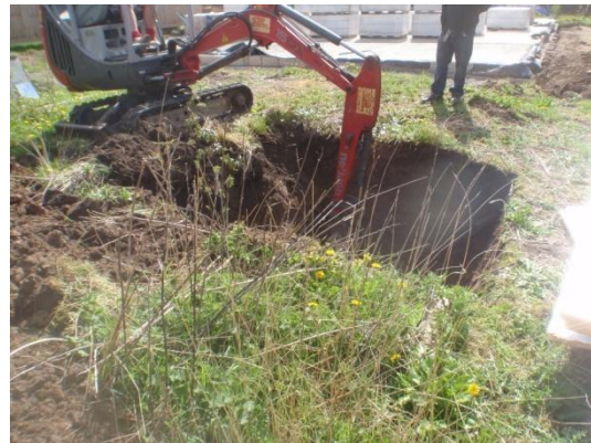
Plate 30: Excavation of the second soakaway, from the north
