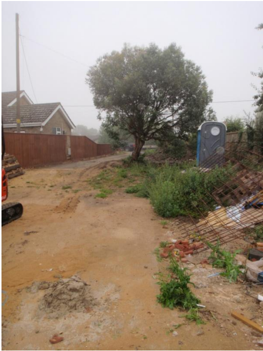
Plate 32: Service trench, pre-excitation, from the west
