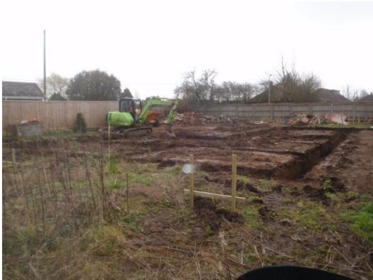
Plate 25: Excavation of the foundations, from the north
