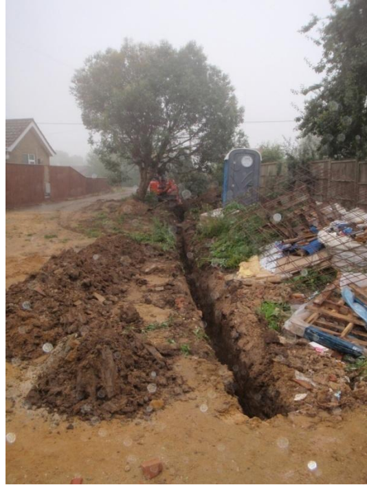
Plate 37: Service trench excavation, from the west
