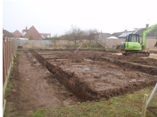
Plate 23: Excavation of the foundations, from the south
