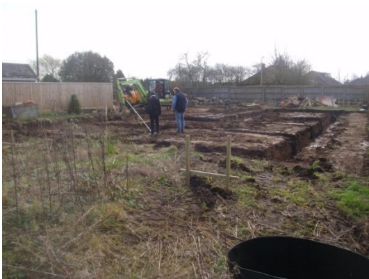
Plate 27: Excavation of the foundations, from the north
