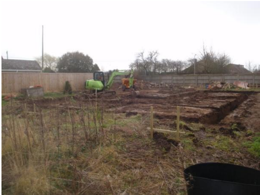
Plate 26: Excavation of the foundations, from the north
