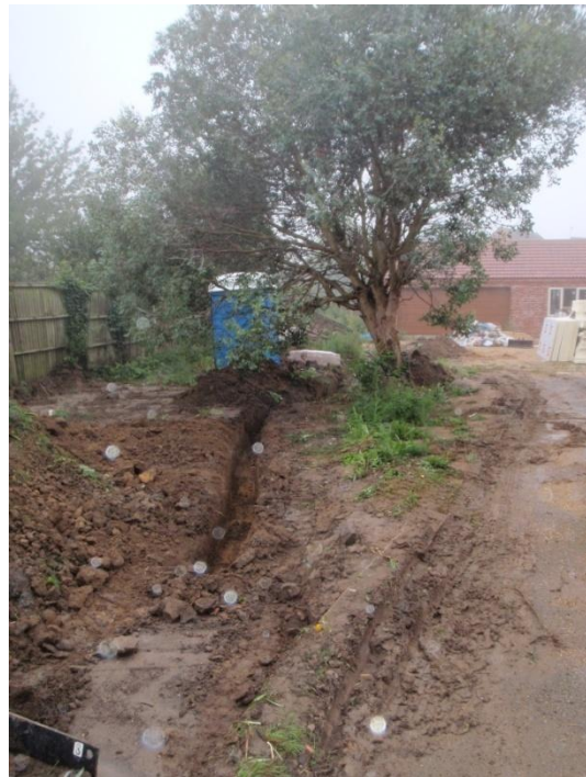
Plate 38: Service trench excavation, from the east
