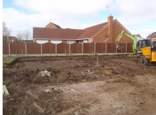
Plate 4: Excavation of the foundations, from the east
