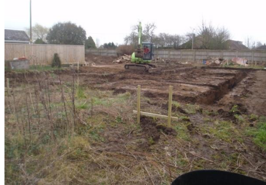
Plate 24: Excavation of the foundations, from the north
