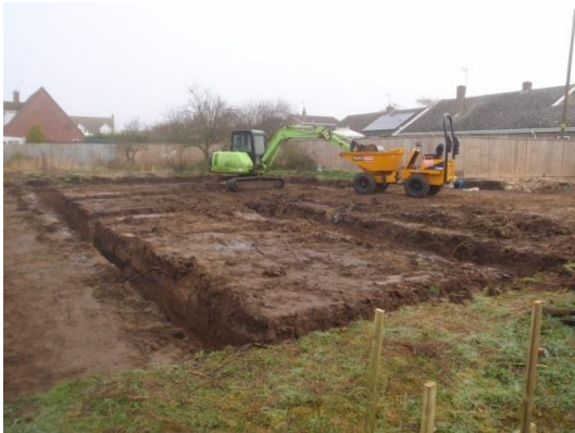
Plate 20: Excavation of the foundations, from the south
