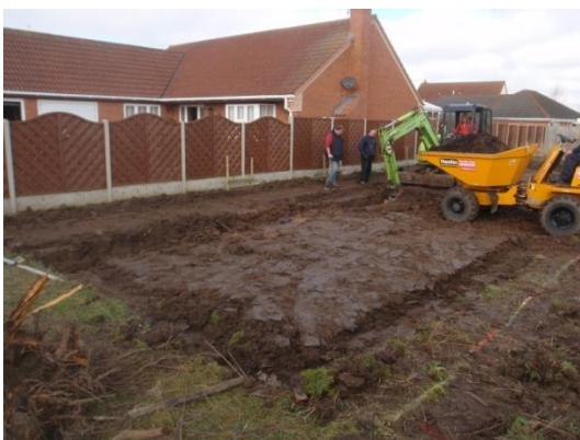
Plate 3: Excavation of the foundations, from the south-east
