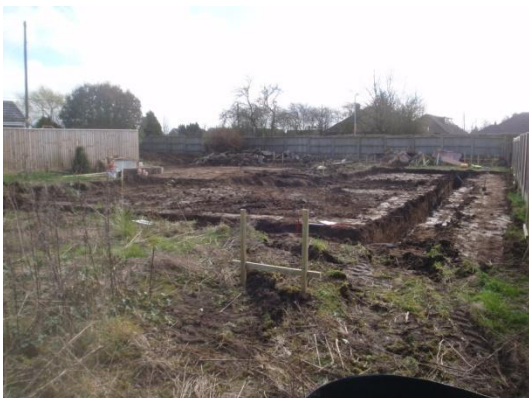
Plate 9: Excavation of the foundations, from the north
