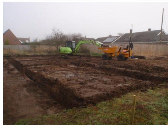
Plate 18: Excavation of the foundations, from the south
