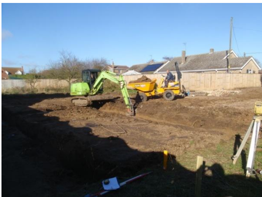
Plate 15: Excavation of the foundations, from the south-west
