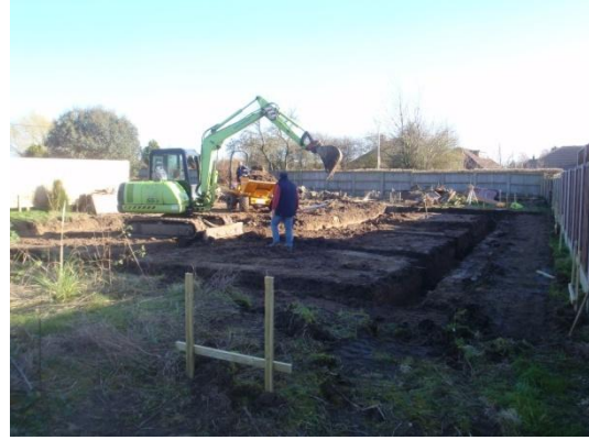
Plate 16: Excavation of the foundations, from the north
