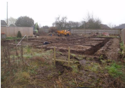
Plate 21: Excavation of the foundations, from the north
