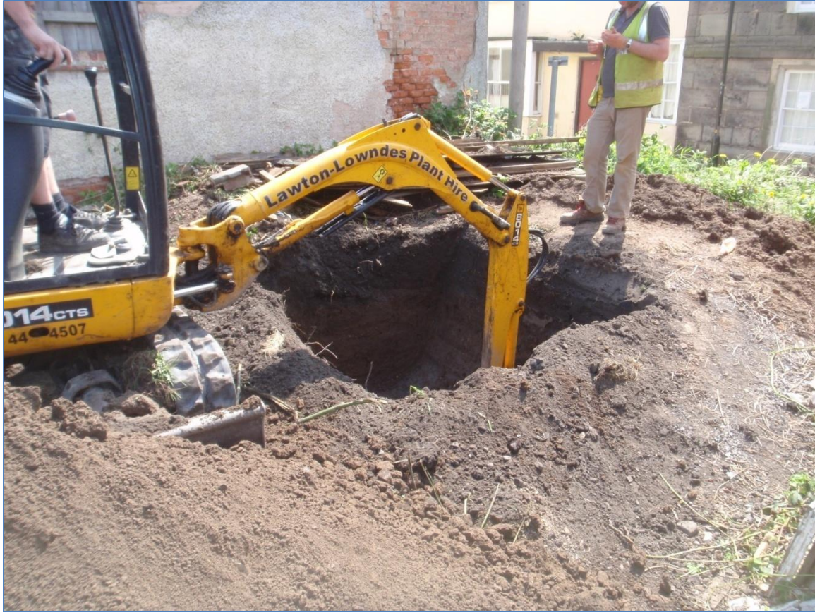
Plate 32: Work in progress, excavation of Trench 2 , from the west
