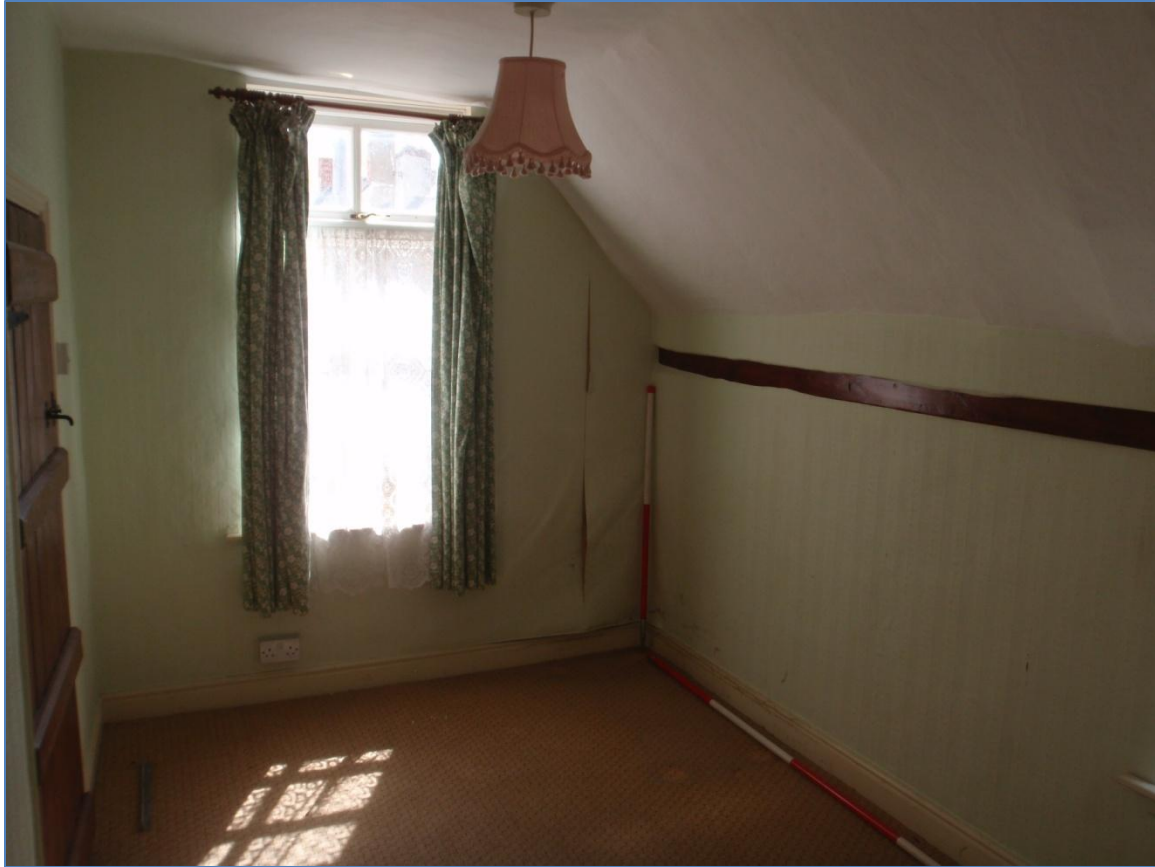
Plate 13: First floor bedroom of 9, Apiary Gate, from the west
