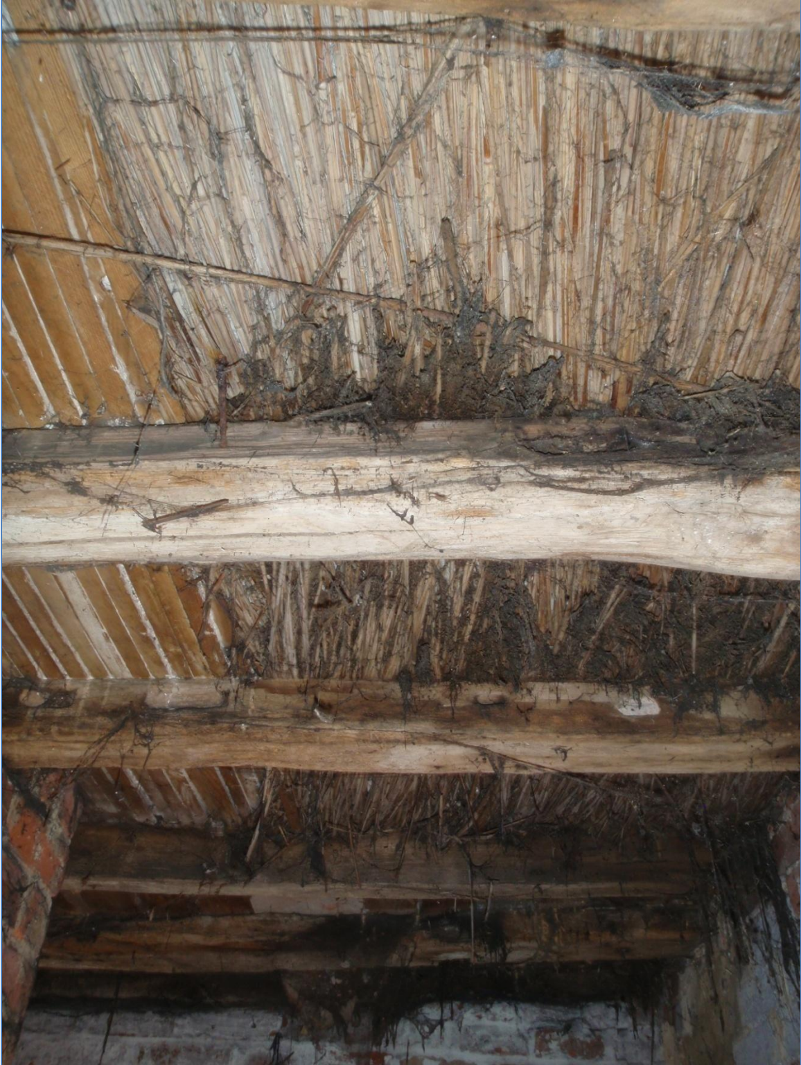
Plate 24: Ceiling of second ground floor room, Side Extension
