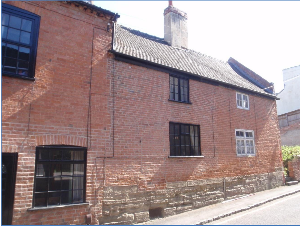
Plate 4: North Elevation of 9, Apiary Gate, from the south-west
