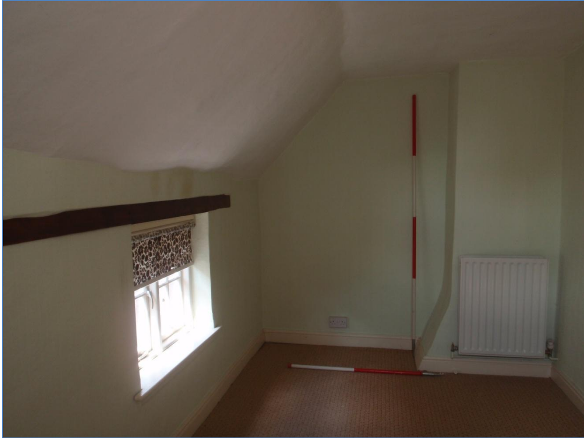
Plate 12: First floor bedroom of 9, Apiary Gate, from the east
