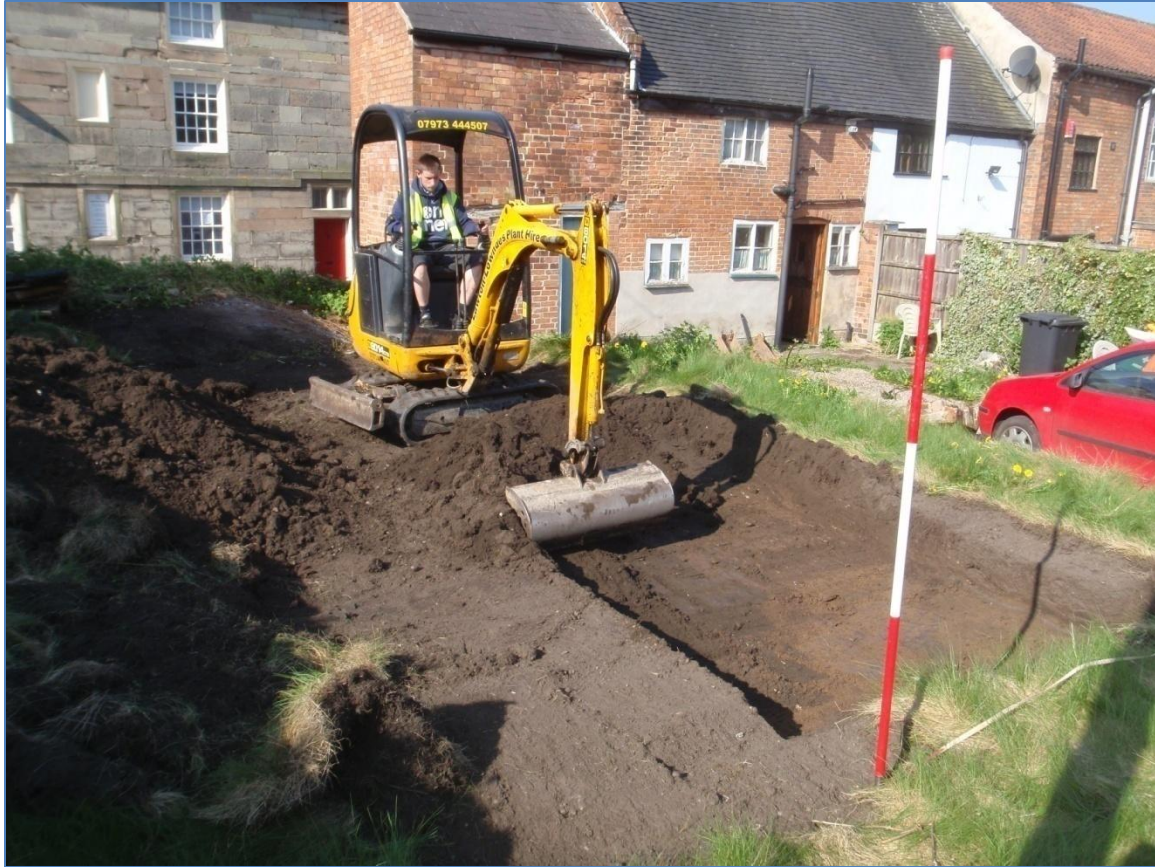
Plate 27: Work in progress, excavation of Trench 1 , from the north
