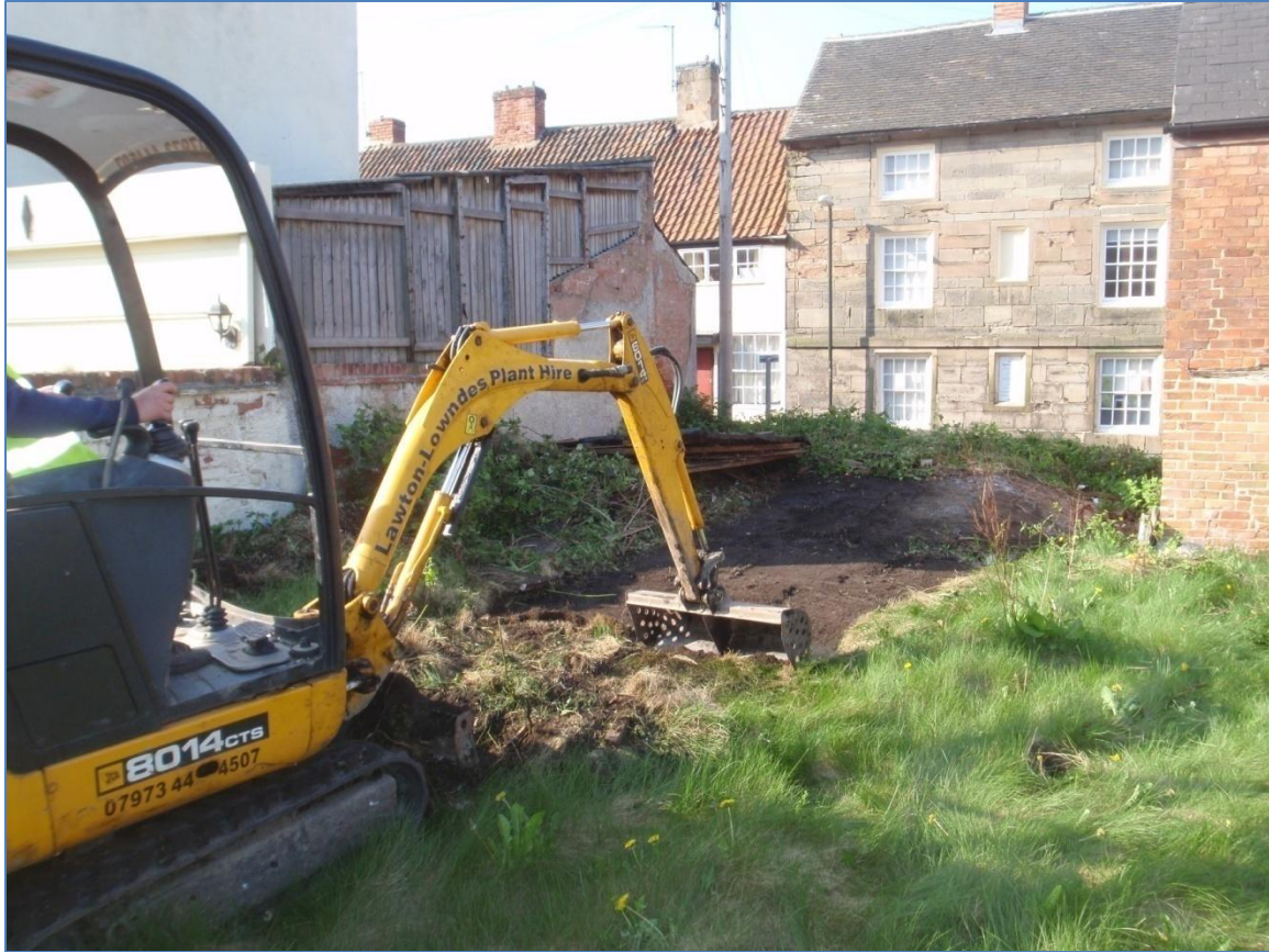
Plate 26: Work in progress, excavation of Trench 1 , from the north
