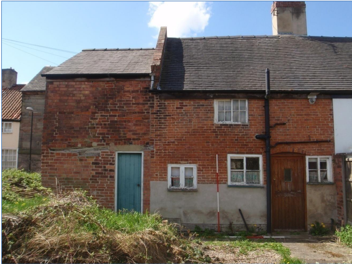
Plate 1: Rear (North) Elevation of 9, Apiary Gate & Side Extension, from the north
