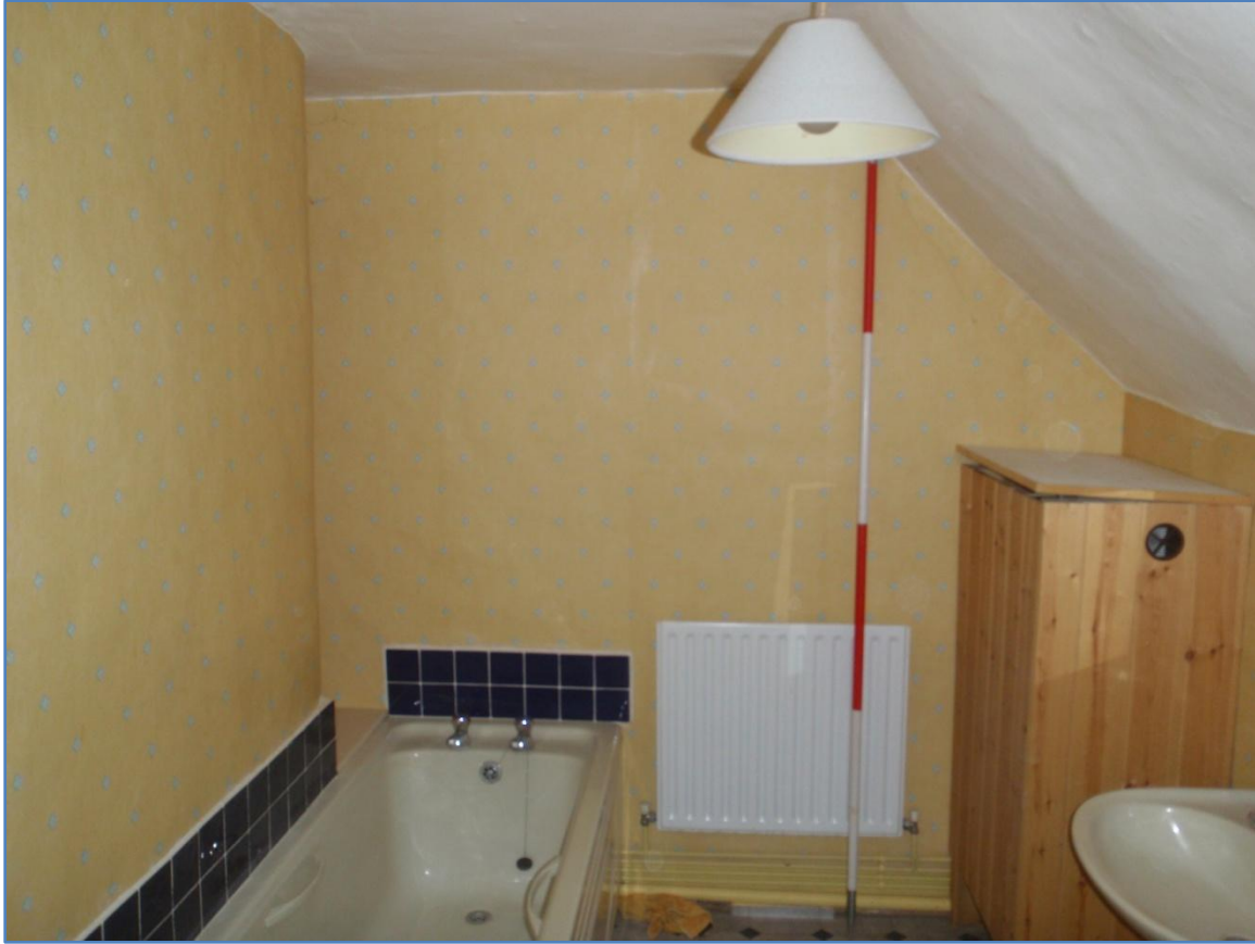
Plate 14: First floor bathroom, 9, Apiary Gate, from the east
