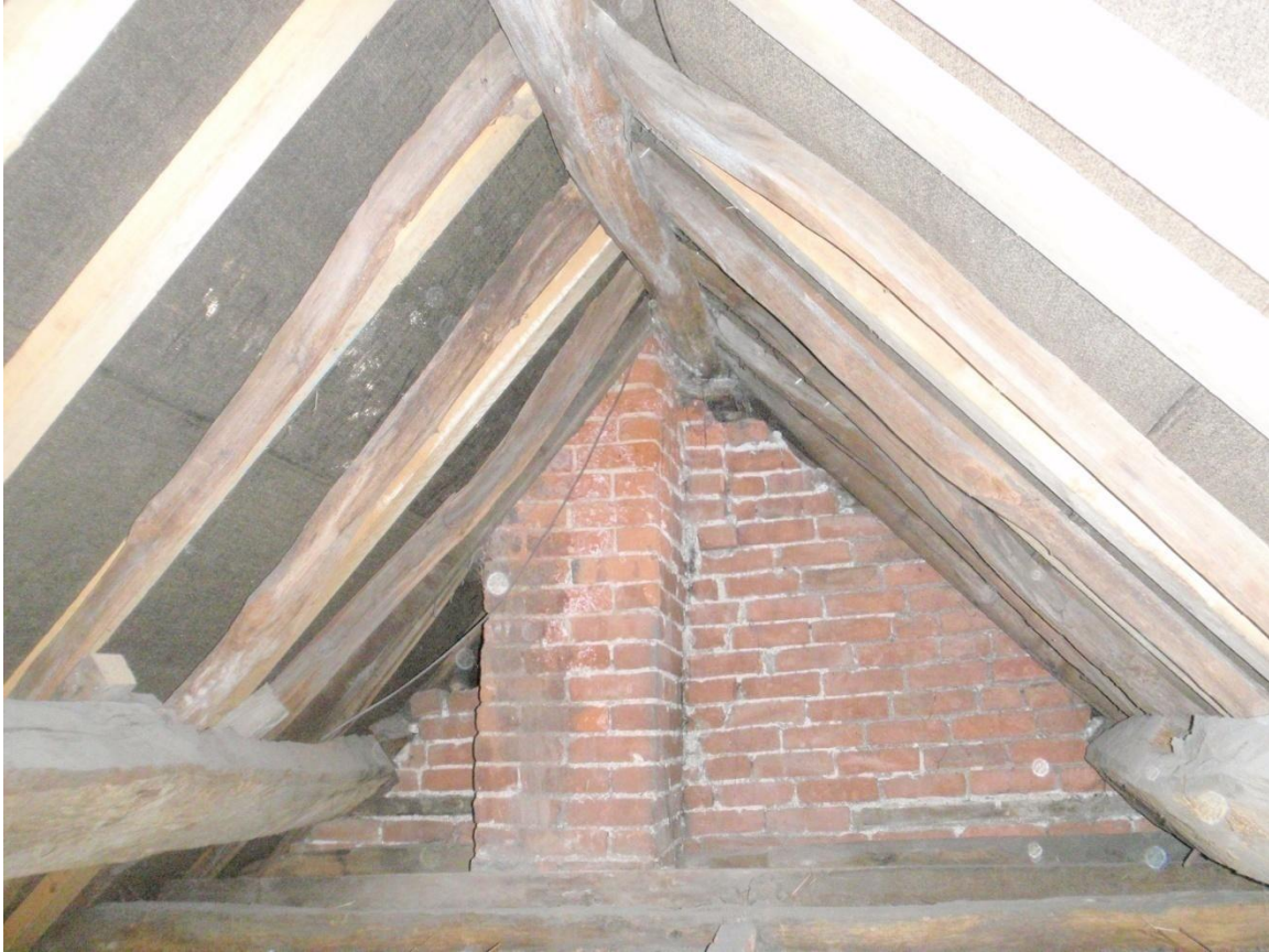
Plate 57: View of the internal roof space, from the east
