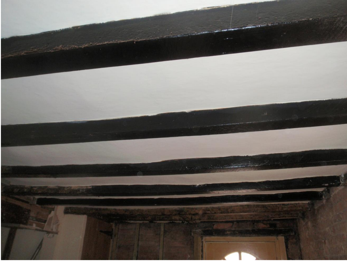
Plate 45: View of the ground floor lounge ceiling, from the west
