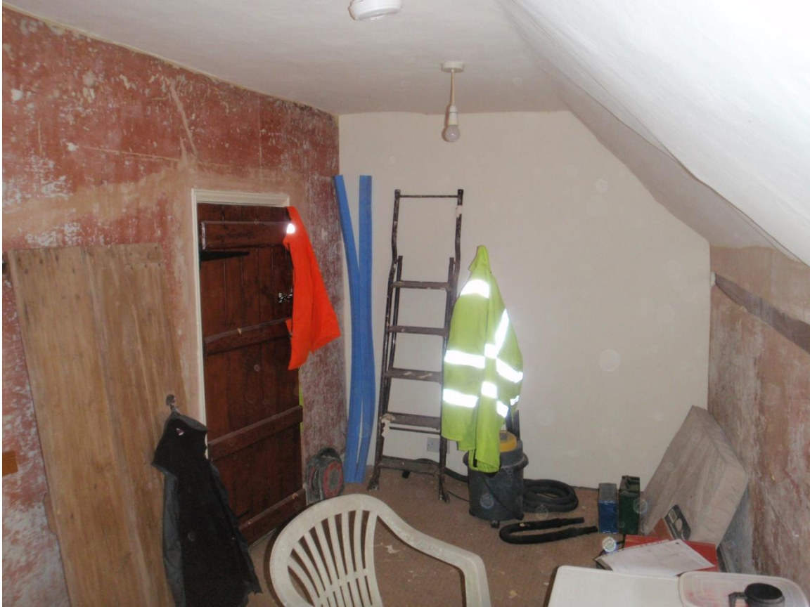
Plate 54: View of the first floor bedroom, from the west
