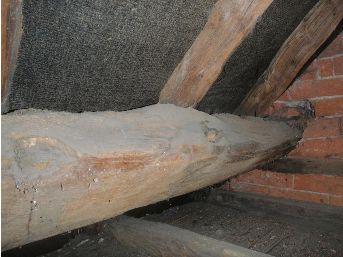
Plate 65: View of the internal roof space, from the west
