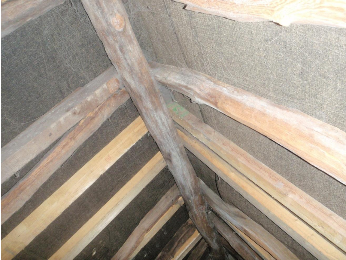
Plate 58: View of the internal roof space, from the east
