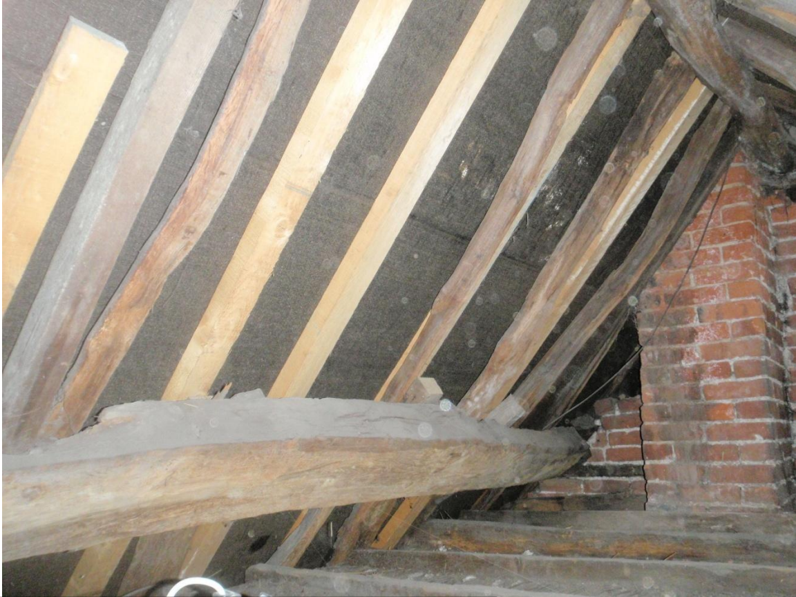
Plate 60: View of the internal roof space, from the east
