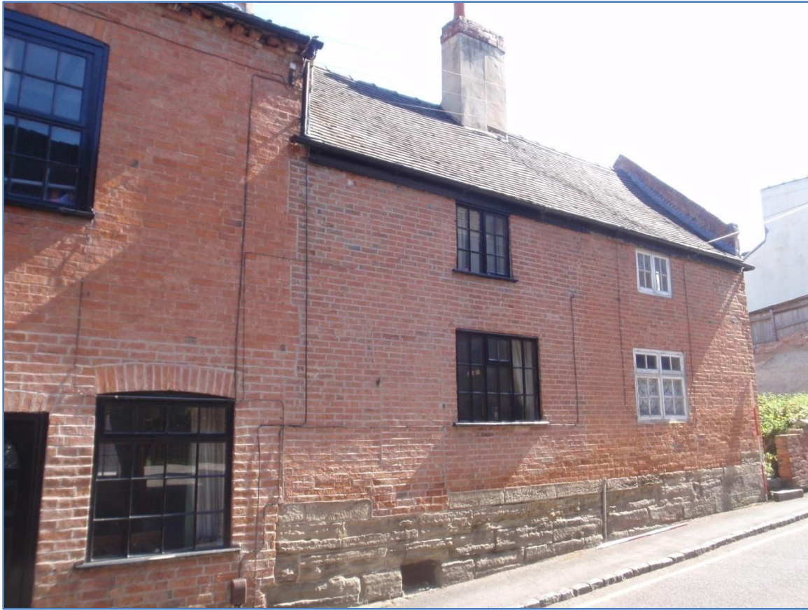
Plate 4: Front (South) Elevation of 9, Apiary Gate, from the south-west
