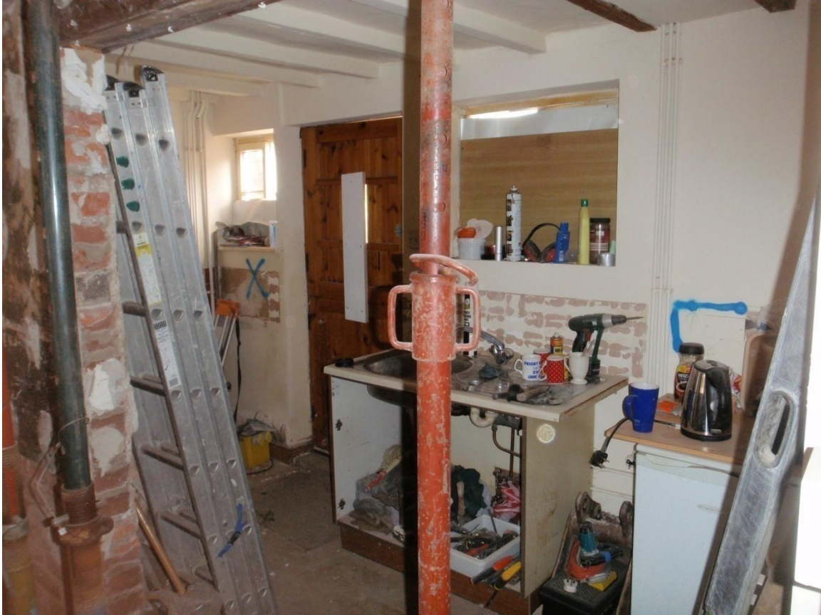
Plate 35: View of the ground floor kitchen, from the south-east
