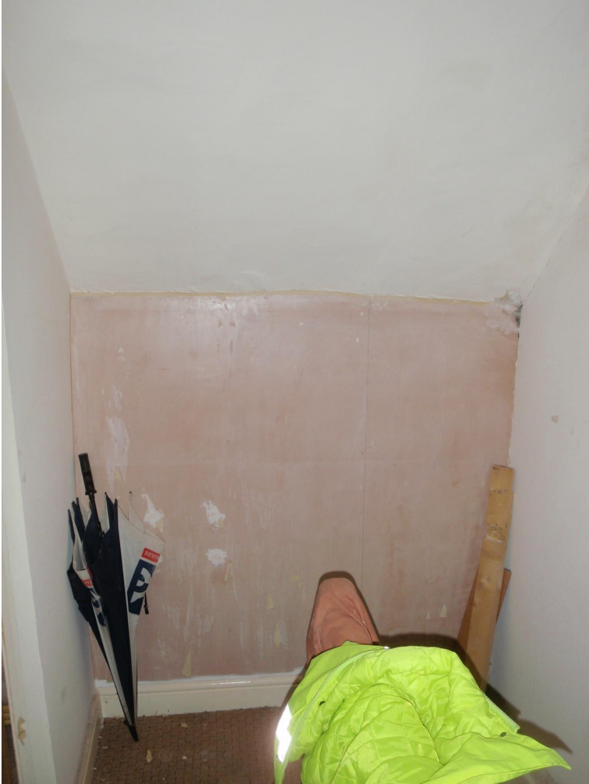
Plate 46: View of the first floor landing, from the south
