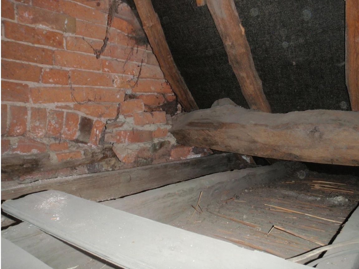
Plate 62: View of the internal roof space, from the west
