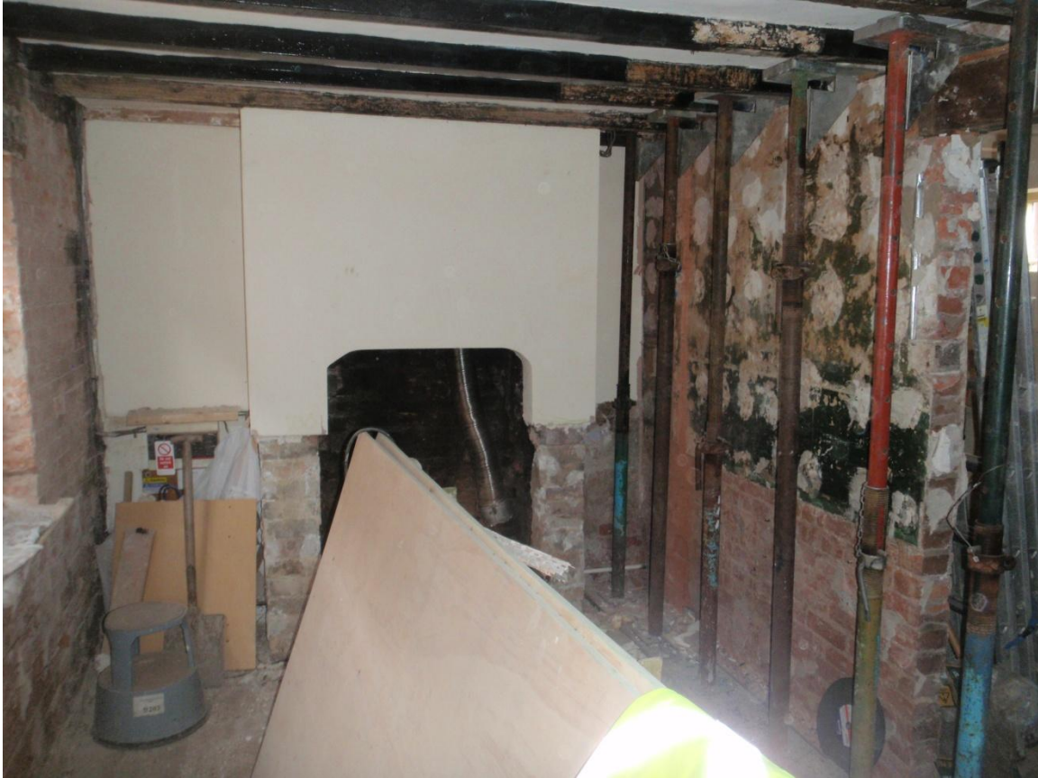
Plate 42: View of the ground floor lounge, from the east
