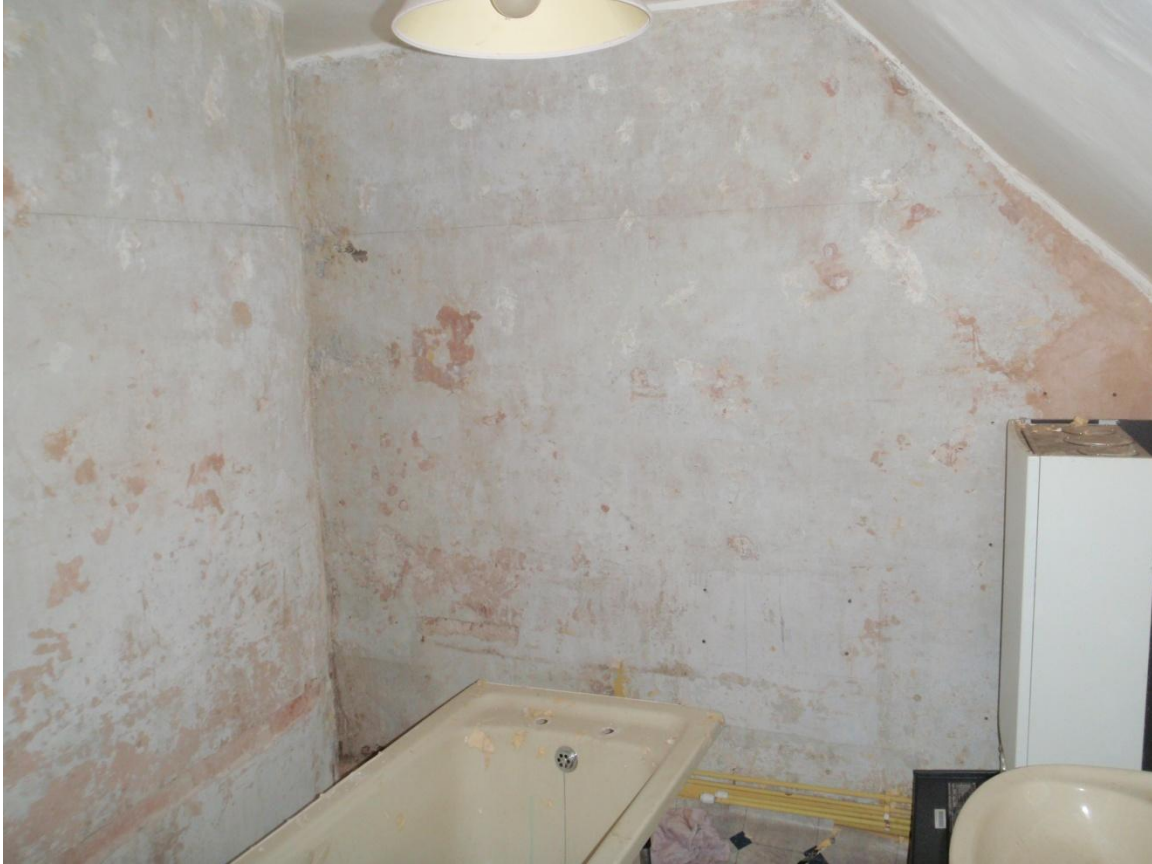
Plate 48: View of the first floor bathroom, from the east
