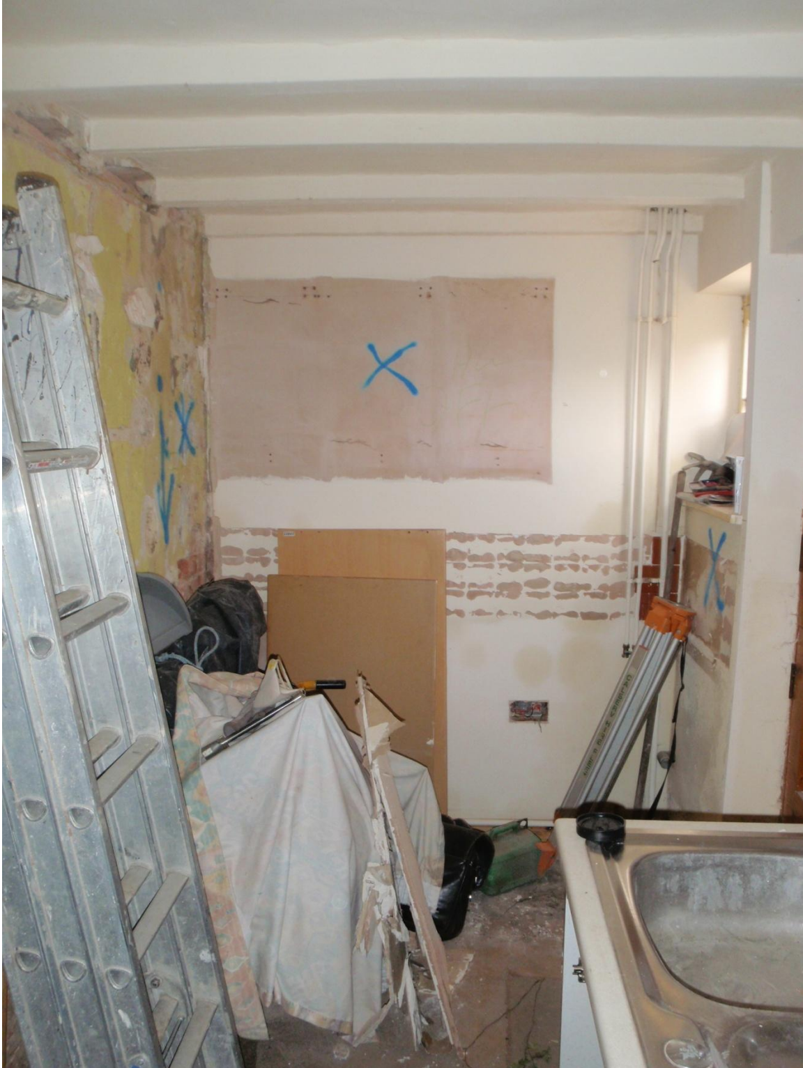
Plate 34: View of the ground floor kitchen, from the east
