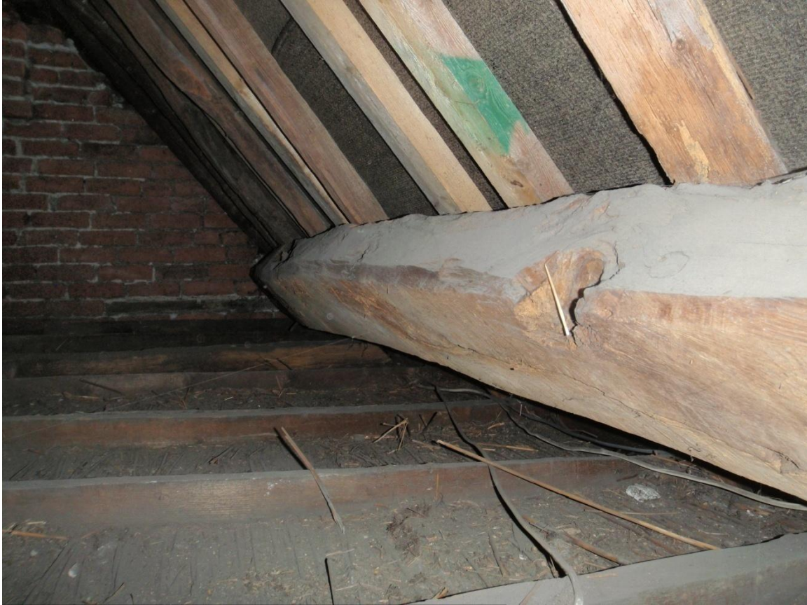
Plate 61: View of the internal roof space, from the east
