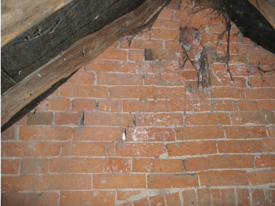
Plate 63: View of the internal roof space, from the west
