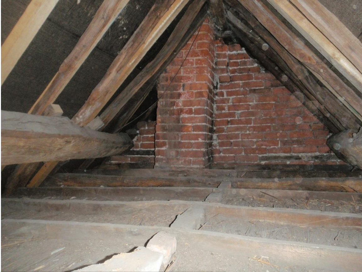
Plate 59: View of the internal roof space, from the east
