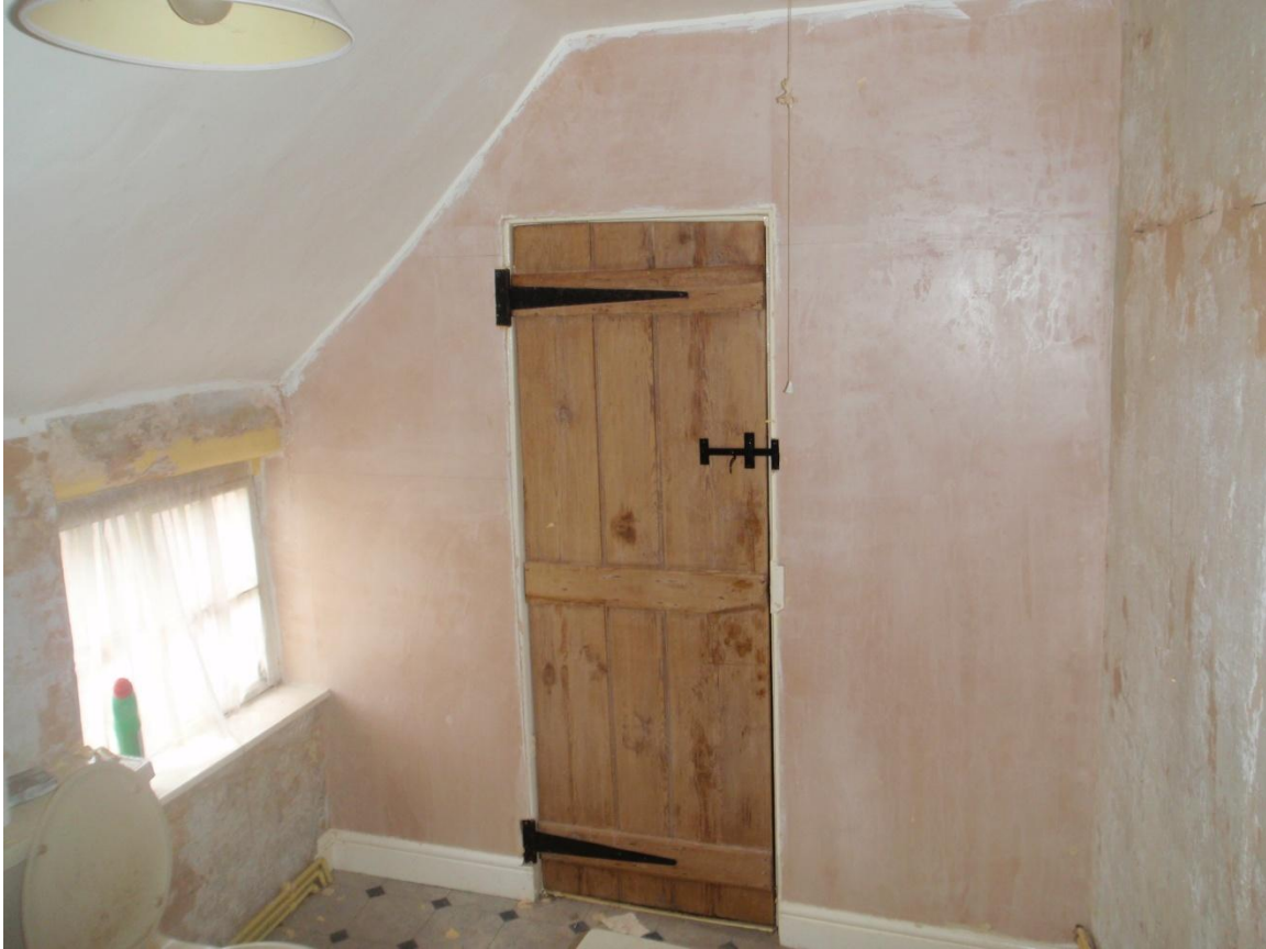
Plate 49: View of the first floor bathroom, from the west
