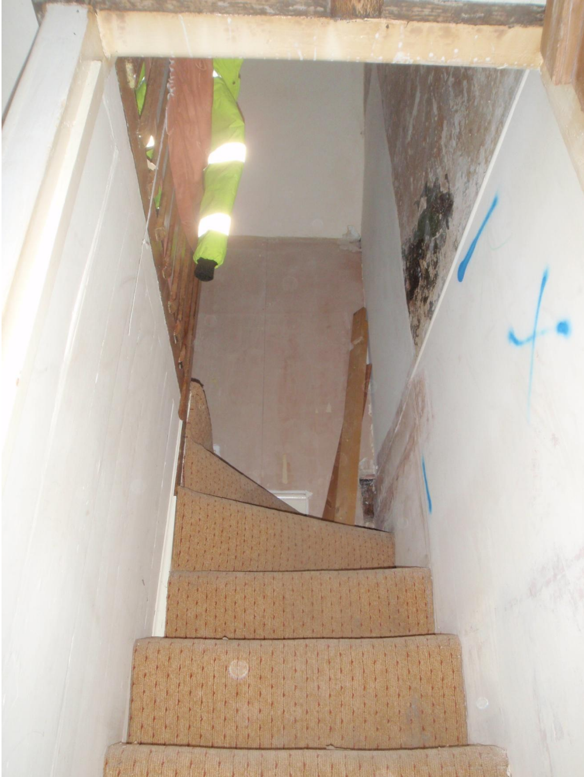
Plate 44: View of the stairwell to the first floor, from the south
