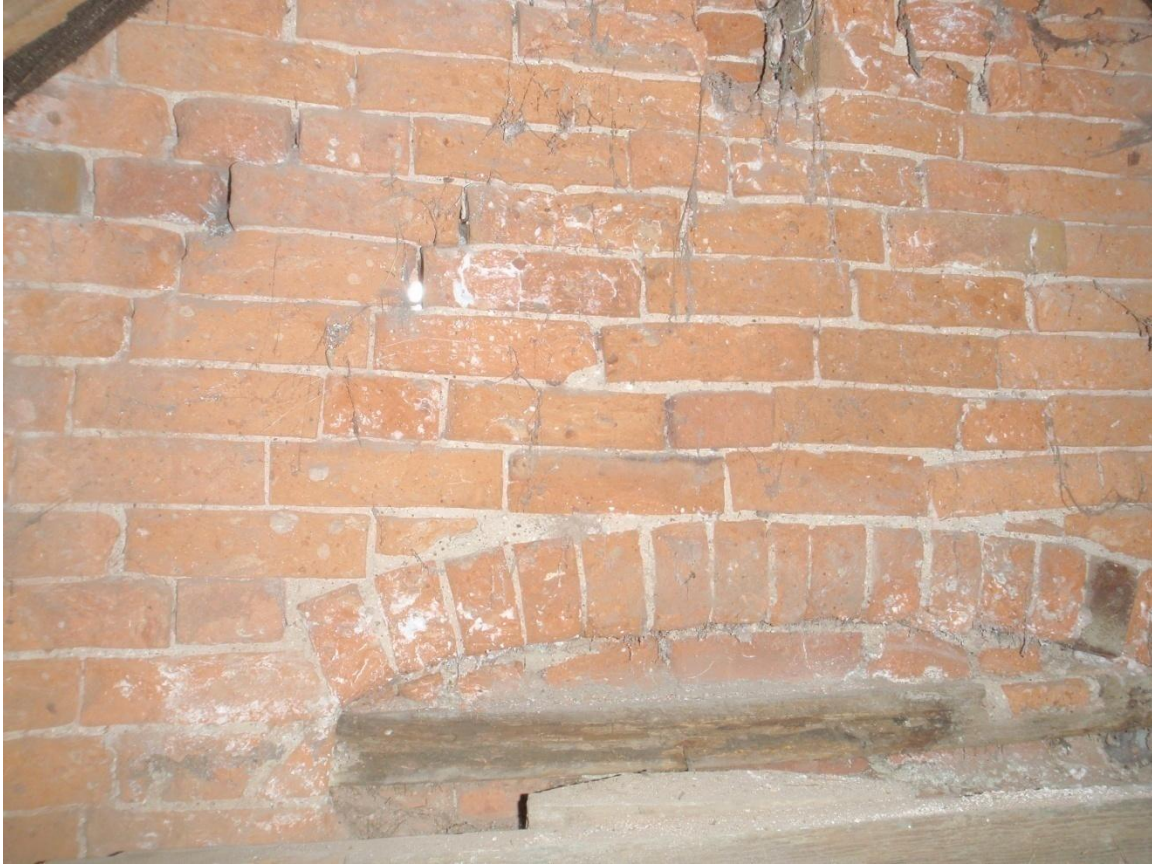
Plate 64: View of the internal roof space, from the west
