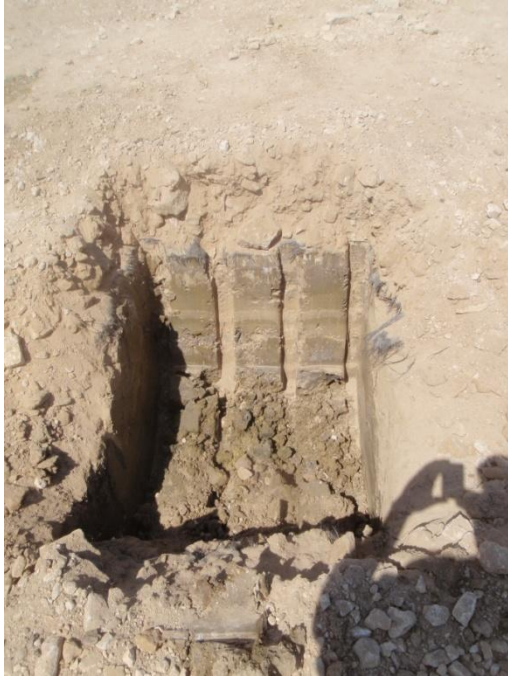
Plate 56: Stanchion Base 60, from the south
