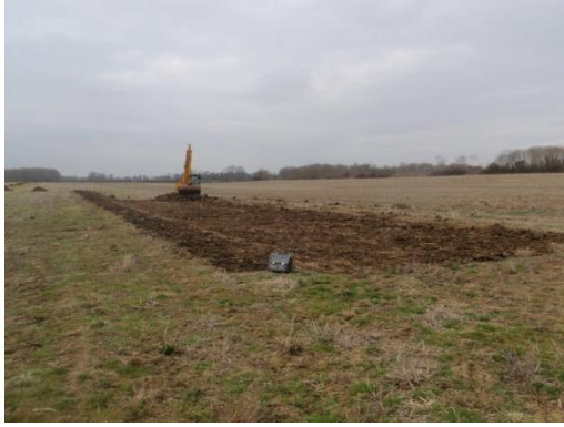
Plate 7: Ground reduction, from the east
