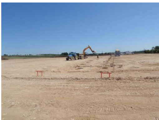
Plate 49: Excavation of the Stanchion Bases, from the east
