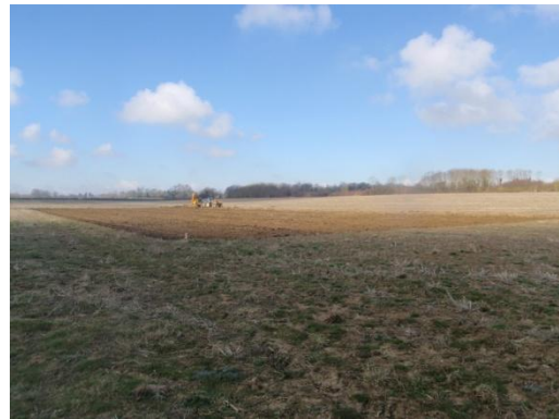
Plate 17: Ground reduction, from the east
