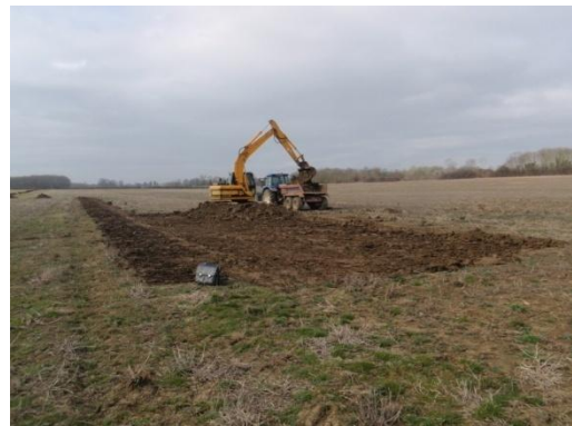
Plate 6: Ground reduction, from the east
