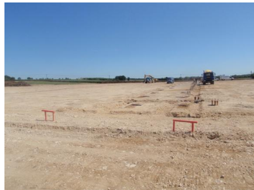
Plate 51: Excavation of the Stanchion Bases, from the east
