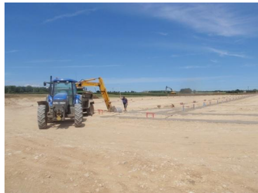
Plate 60: Excavation of the Stanchion Bases, from the west
