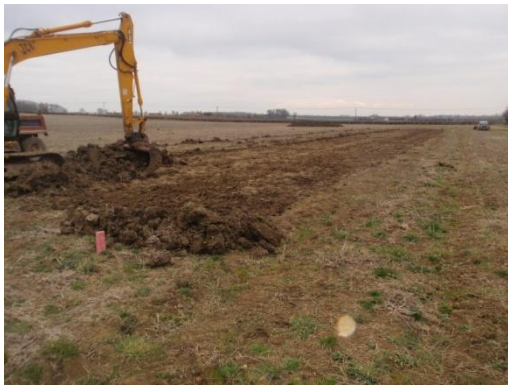
Plate 8: Ground reduction, from the west
