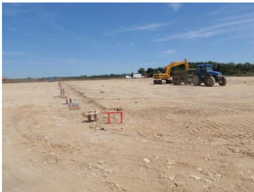
Plate 57: Excavation of the Stanchion Bases, from the west
