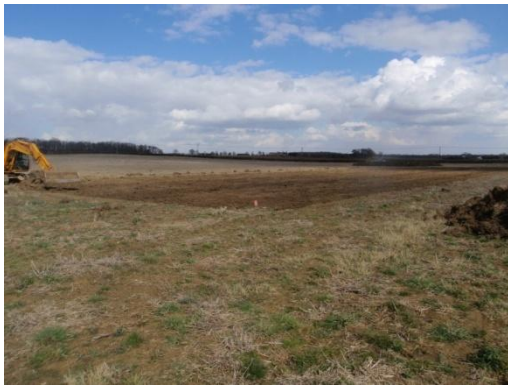
Plate 14: Ground reduction, from the west
