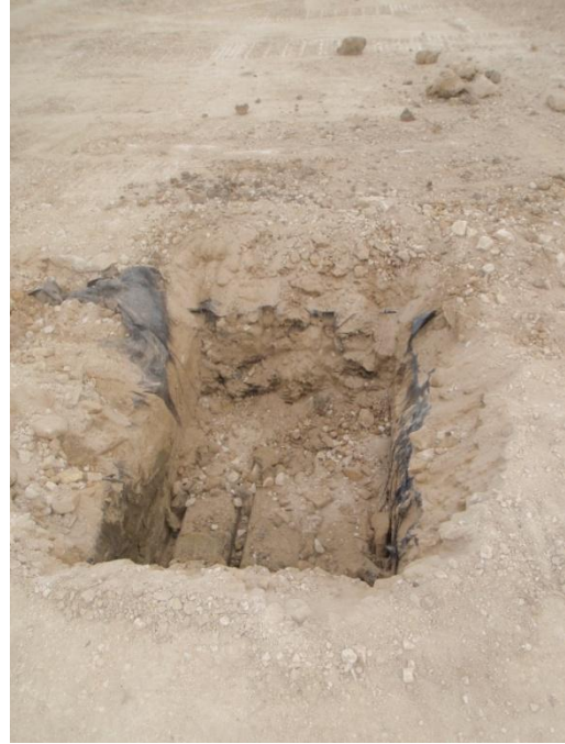
Plate 34: Stanchion Base 15, from the south
