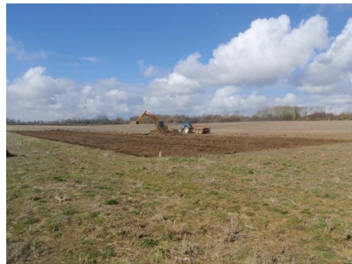
Plate 12: Ground reduction, from the east
