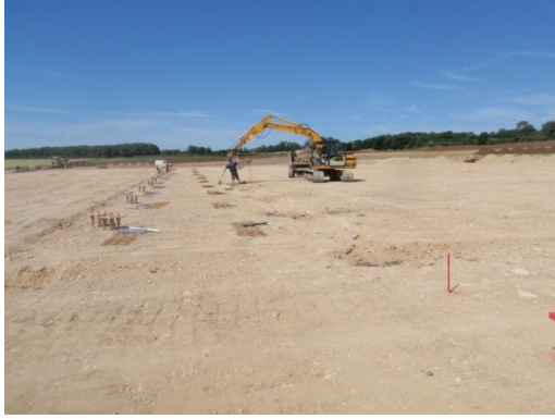
Plate 47: Excavation of the Stanchion Bases, from the east
