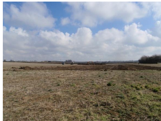
Plate 18: Ground reduction, from the west
