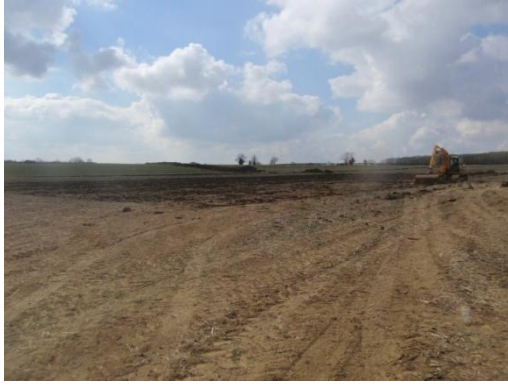
Plate 19: Ground reduction, from the east
