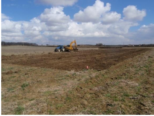
Plate 13: Ground reduction, from the west
