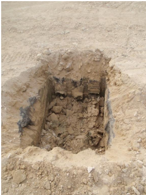
Plate 32: Stanchion Base 10, from the south
