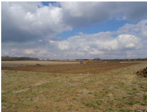
Plate 21: Ground reduction, from the west
