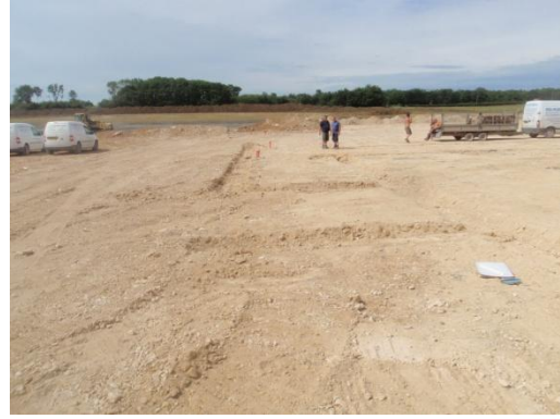
Plate 44: Excavated ring beams for the feed silos, from the south
