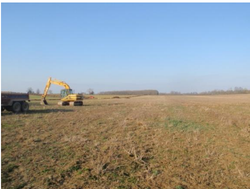
Plate 3: Pre-groundworks, from the east
