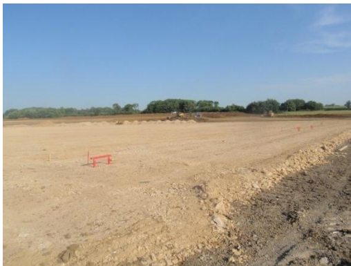
Plate 27: Pre-groundworks, from the east
