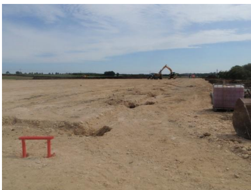
Plate 33: Excavation of the Stanchion Bases, from the west
