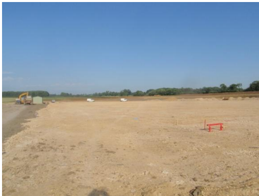
Plate 26: Pre-groundworks, from the east
