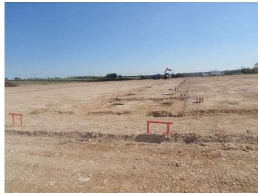
Plate 45: Excavation of the Stanchion Bases, from the west
