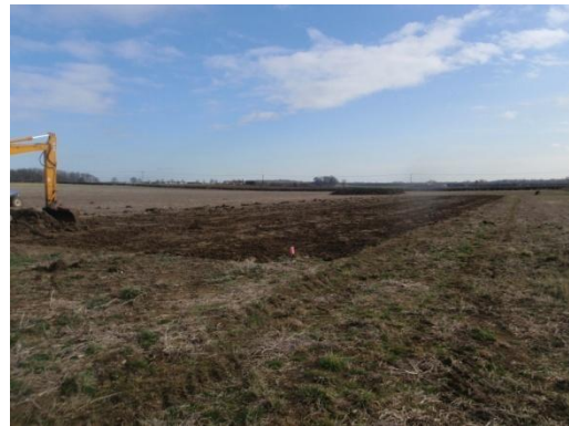
Plate 11: Ground reduction, from the west
