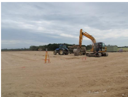
Plate 43: Excavation of the Stanchion Bases, from the west
