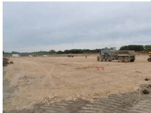
Plate 35: Excavation of the Stanchion Bases, from the east
