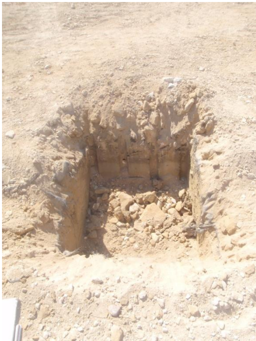
Plate 48: Stanchion Base 40, from the north
