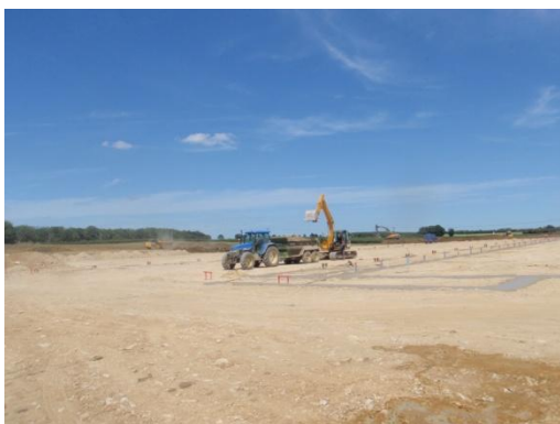
Plate 58: Excavation of the Stanchion Bases, from the west
