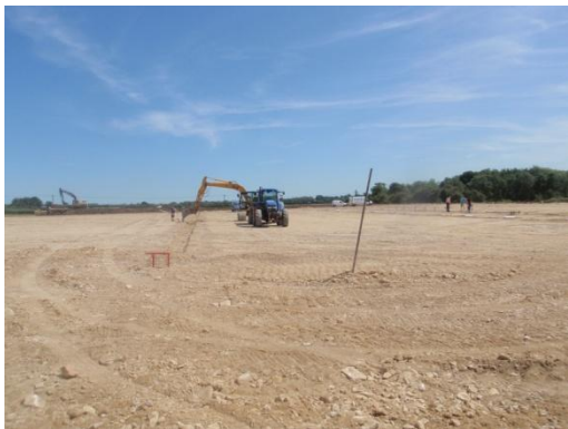
Plate 53: Excavation of the Stanchion Bases, from the west
