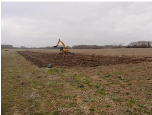
Plate 9: Ground reduction, from the east
