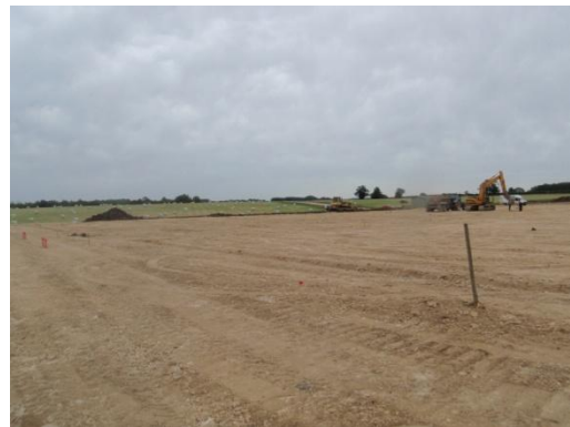
Plate 39: Excavation of the Stanchion Bases, from the east
