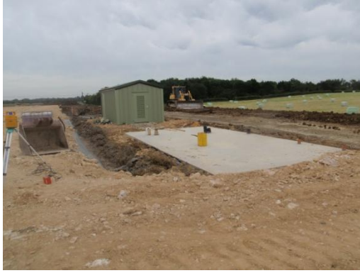
Plate 62: The General Purpose Building and Back-up Generator House, from the west
