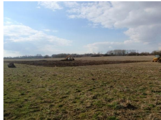
Plate 23: Ground reduction, from the east
