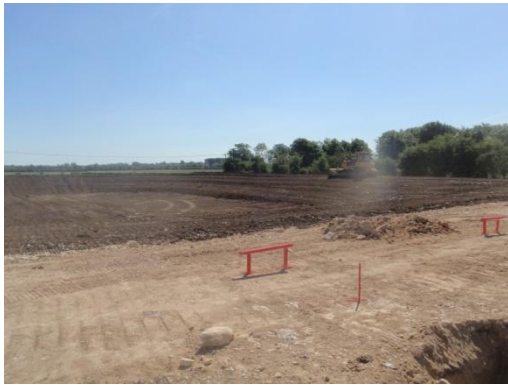
Plate 63: Construction of the pond, from the west
