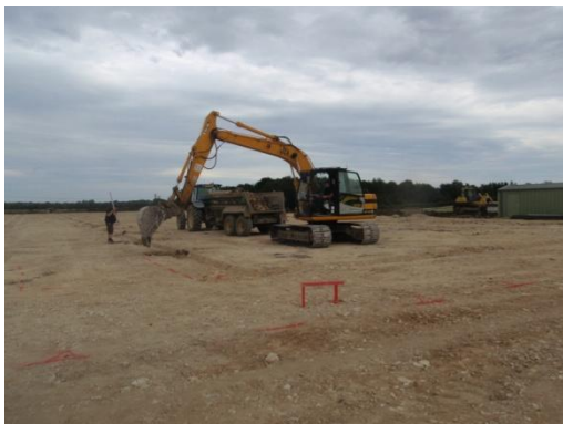
Plate 42: Excavation of the Stanchion Bases, from the west
