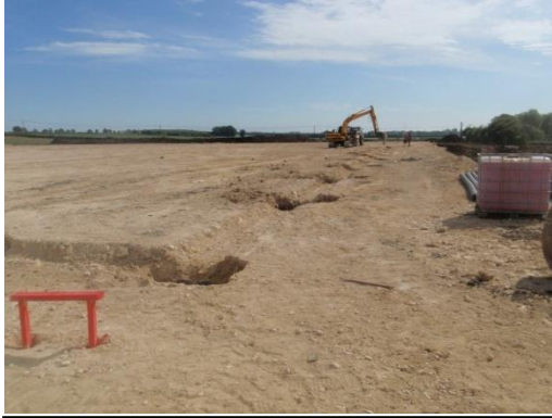
Plate 31: Excavation of the Stanchion Bases, from the west
