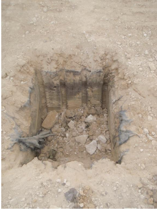
Plate 36: Stanchion Base 20, from the south
