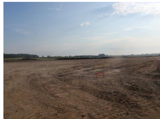
Plate 24: Pre-groundworks, from the south
