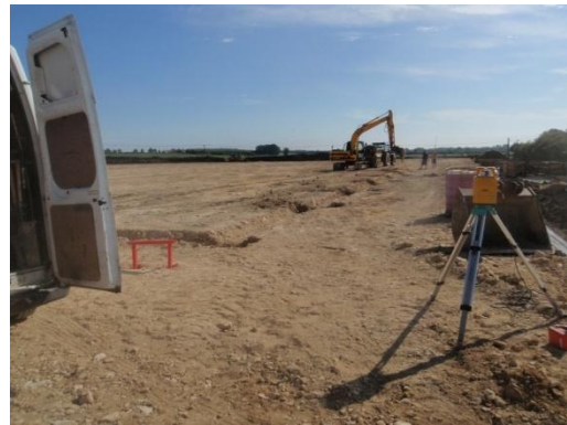
Plate 29: Excavation of the Stanchion Bases, from the west
