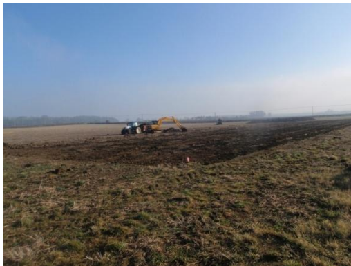
Plate 15: Ground reduction, from the west
