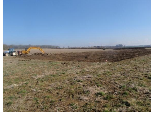
Plate 16: Ground reduction, from the west
