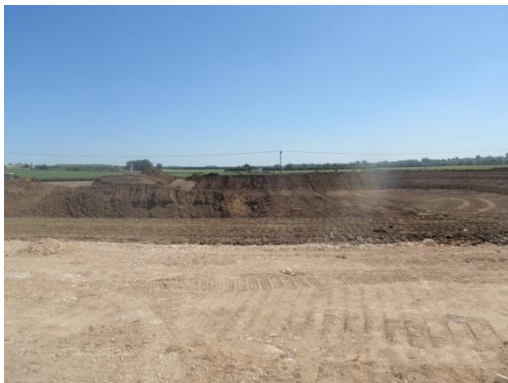
Plate 64: Construction of the pond, from the west
