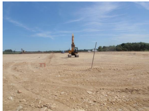
Plate 55: Excavation of the Stanchion Bases, from the west
