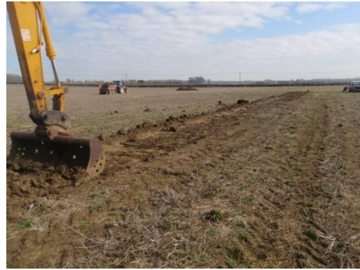
Plate 4: Ground reduction, from the west
