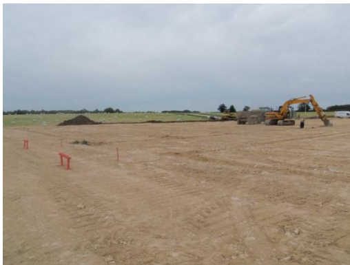
Plate 37: Excavation of the Stanchion Bases, from the east
