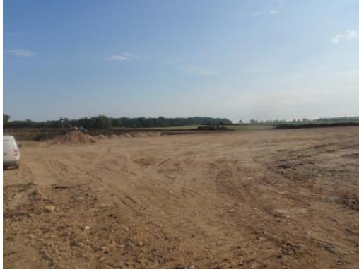
Plate 25: Pre-groundworks, from the south
