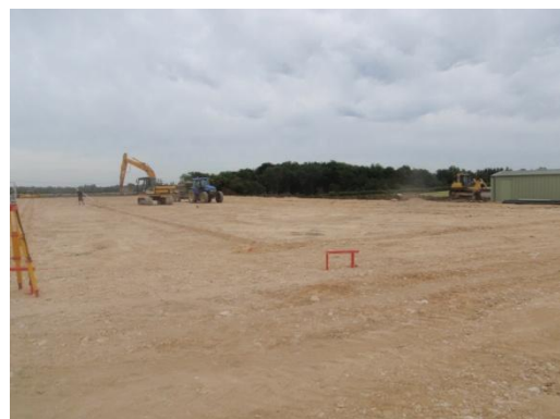
Plate 40: Excavation of the Stanchion Bases, from the east
