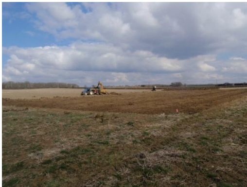
Plate 20: Ground reduction, from the west
