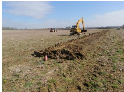
Plate 5: Ground reduction, from the west
