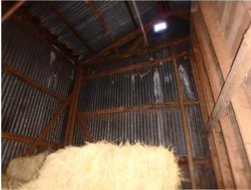
Plate 18: View of the internal timber framework for the external wall cladding of the north wall of the Hay Barn and supporting roof structure, from the south
