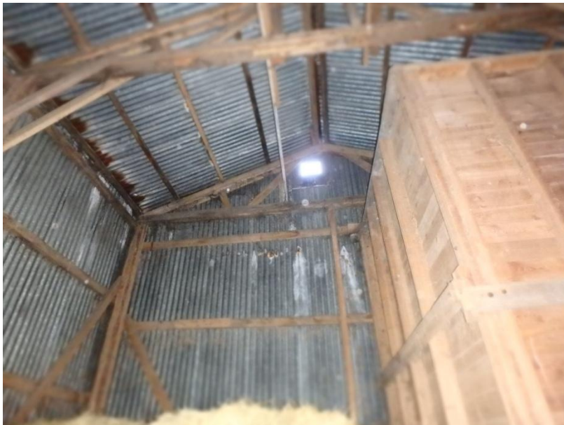
Plate 13: View of the internal timber framework for the external wall cladding of the north wall of the Hay Barn and supporting roof structure, from the south
