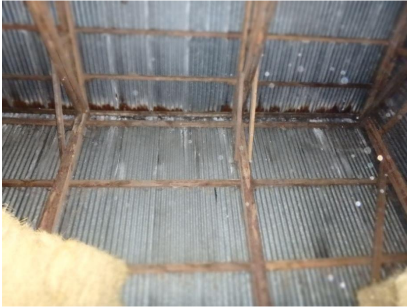
Plate 12: View of the internal timber framework for the external wall cladding of the west wall of the Hay Barn and supporting roof structure, from the east
