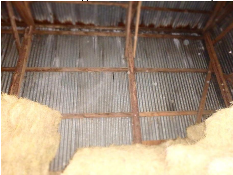
Plate 17: View of the internal timber framework for the external wall cladding of the west wall of the Hay Barn and supporting roof structure, from the east
