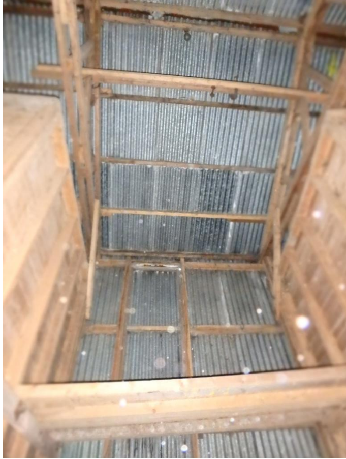
Plate 23: View of the internal timber framework for the external wall cladding of the east wall of the Hay Barn and supporting roof structure, from the west
