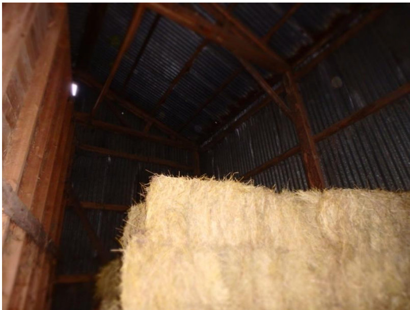
Plate 24: View of the internal timber framework for the external wall cladding of the south wall of the Hay Barn and supporting roof structure, from the north
