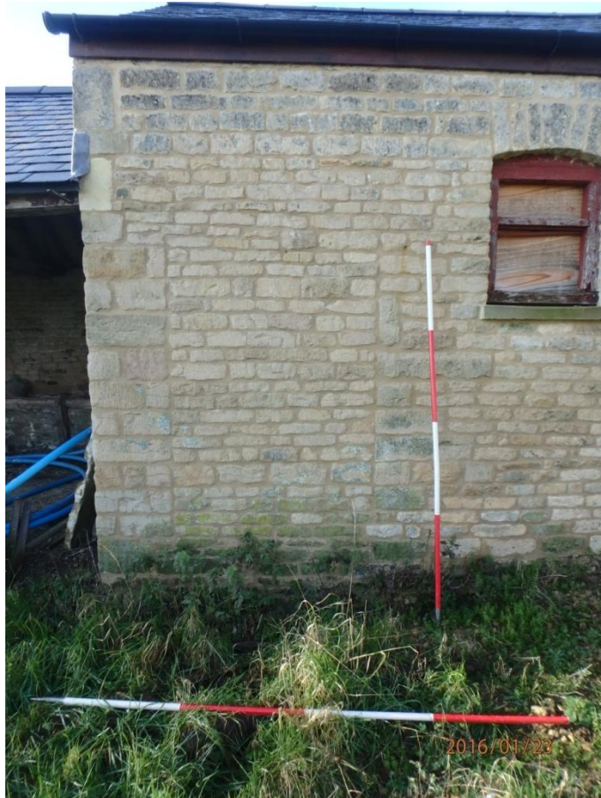
Plate 11: Detail: View of a blocked in door opening within the East Elevation of Outbuilding 2, from the east
