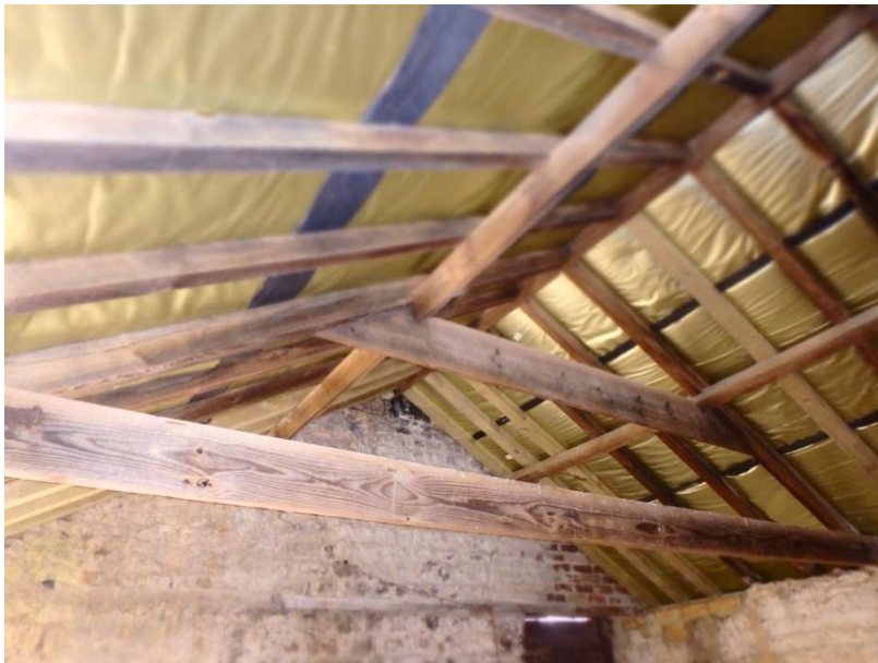
Plate 166: View of the roof supporting structure of Cell 7, from the south
