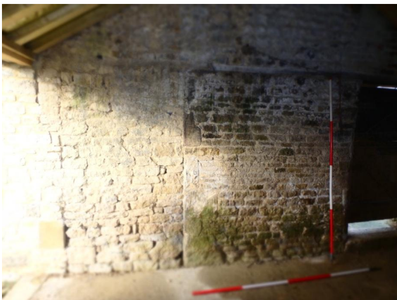
Plate 173: Detail: view of infilled door opening in the north wall of Cell 7, from the south
