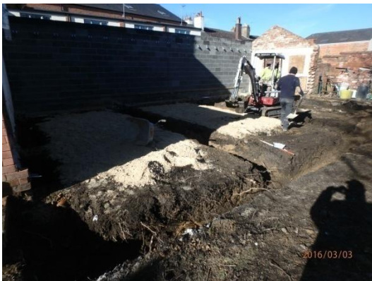
Plate 21: Excavation of the foundations, from the south-east
