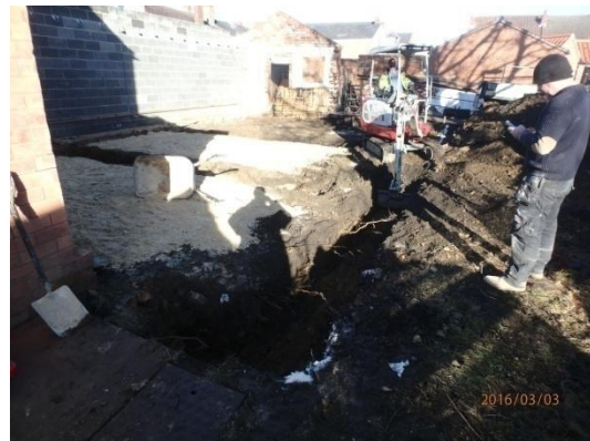
Plate 17: Excavation of the foundations, from the south-east
