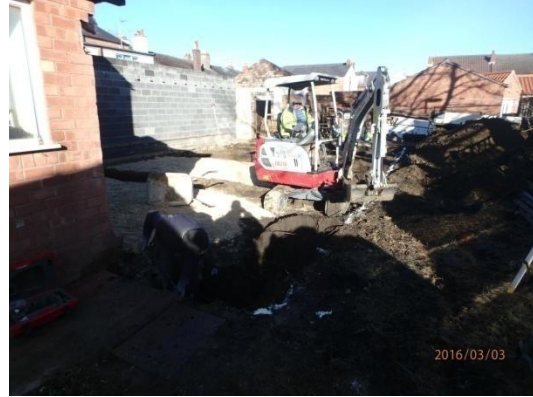
Plate 16: Excavation of the foundations, from the south-east
