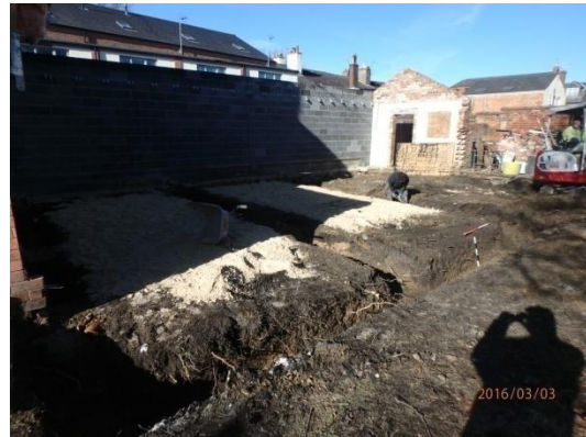
Plate 23: Excavation of the foundations, from the south-east
