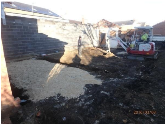
Plate 9: Excavation of the foundations, from the south-east
