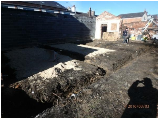
Plate 26: Excavation of the foundations, from the south-east
