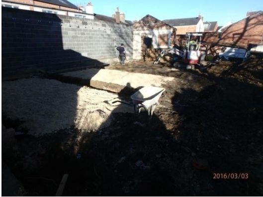
Plate 13: Excavation of the foundations, from the south-east
