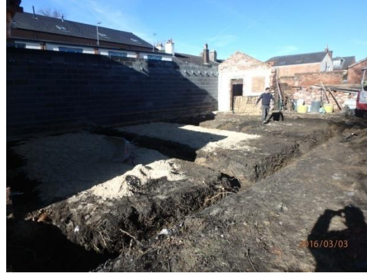
Plate 28: Completed foundation excavations, from the south-east
