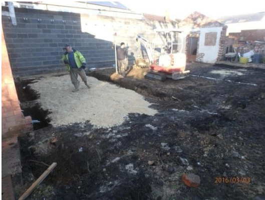
Plate 8: Excavation of the foundations, from the south-east
