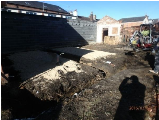
Plate 20: Excavation of the foundations, from the south-east
