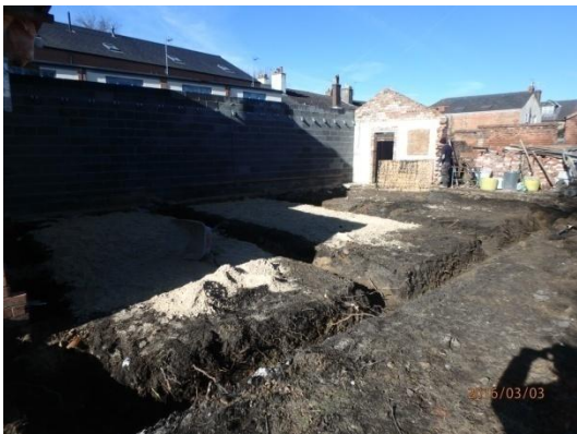
Plate 27: Excavation of the foundations, from the south-east
