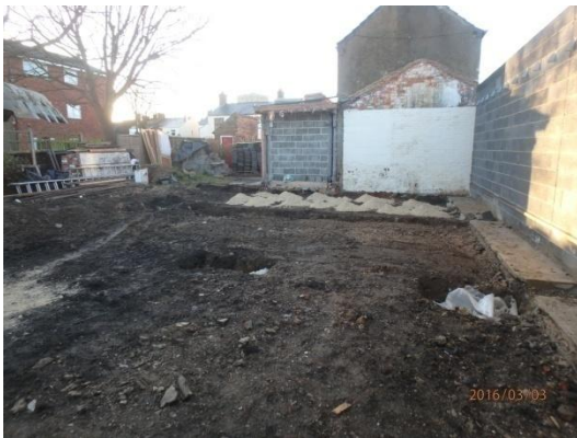
Plate 2: Excavation of the foundations, from the north
