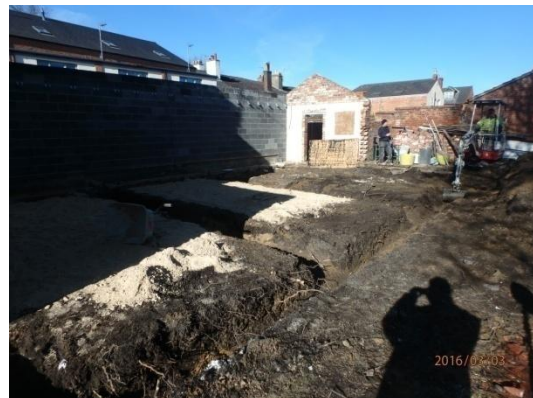
Plate 24: Excavation of the foundations, from the south-east
