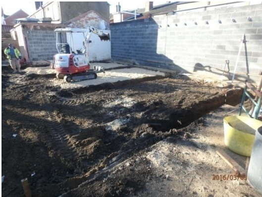
Plate 14: Excavation of the foundations, from the north
