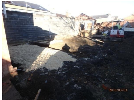
Plate 11: Excavation of the foundations, from the south-east
