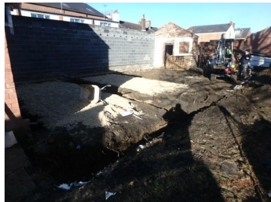
Plate 18: Excavation of the foundations, from the south-east
