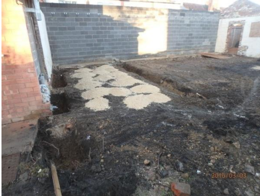
Plate 1: Excavation of the foundations, from the east
