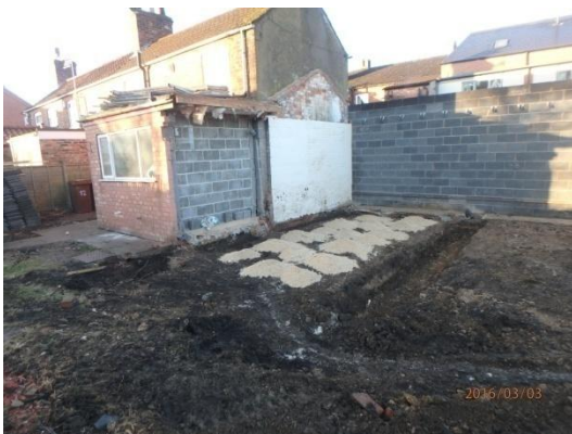
Plate 3: Excavation of the foundations, from the north-east
