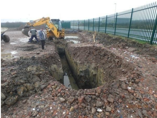
Plate 48: Excavation of the storage tank, from the north-east
