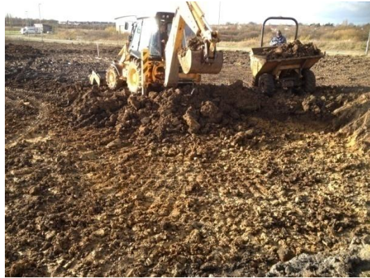
Plate 25: Initial ground reduction, from the south-east
