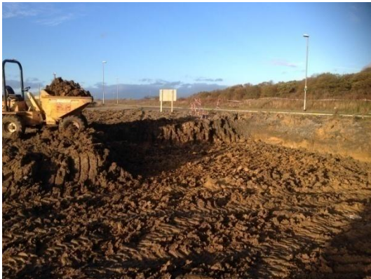
Plate 29: Initial ground reduction, from the south
