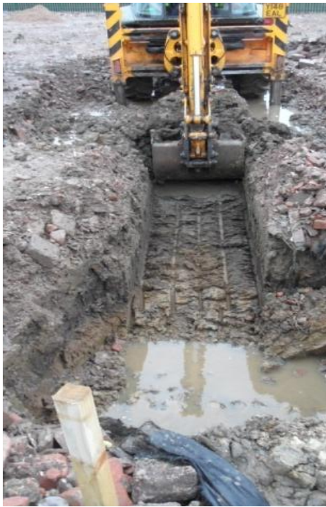
Plate 65: Excavation of the manhole, connecting trench and interceptor, from the north-west
