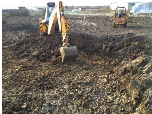
Plate 27: Initial ground reduction, from the south east
