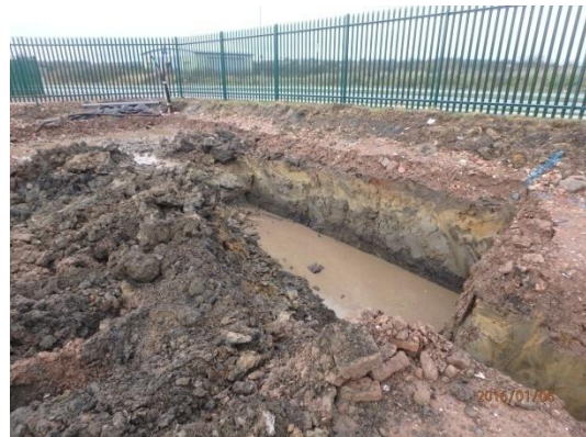
Plate 51: Excavation of the storage tank, from the south
