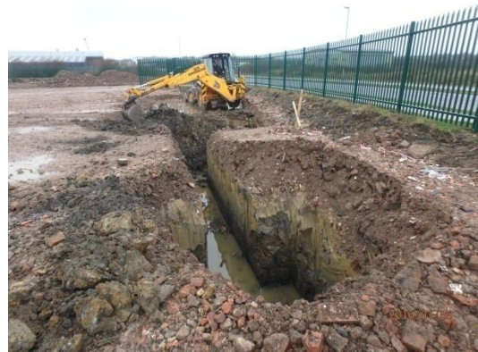
Plate 50: Excavation of the storage tank, from the north-east
