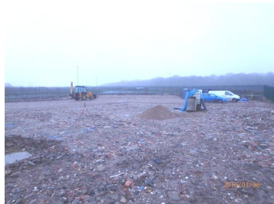
Plate 38: Compacted hardcore over the area of the development site, from the south-west
