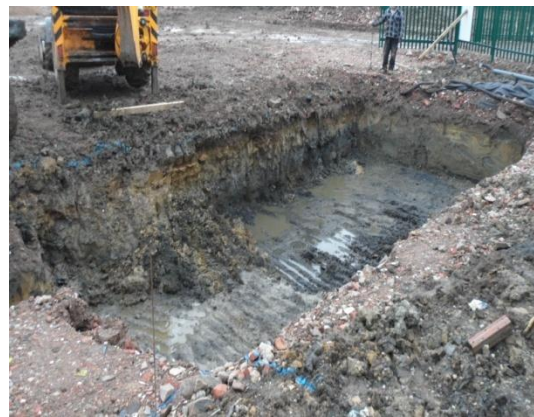
Plate 63: Excavation of the storage tank, from the north
