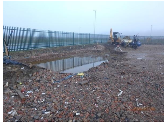
Plate 43: Excavation of the chamber and connecting trench, from the south-west
