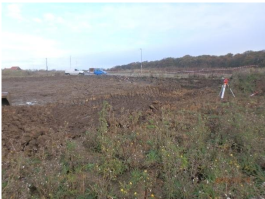
Plate 12: Initial ground reduction, from the south-east
