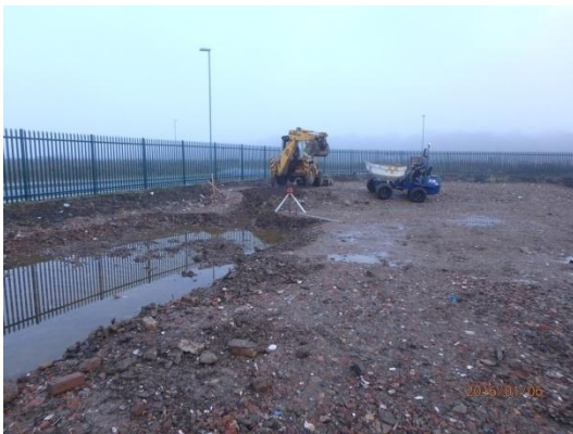
Plate 42: Excavation of the chamber and connecting trench, from the south-west
