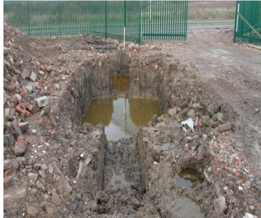
Plate 68: Excavation of the manhole, connecting trench and interceptor, from the south-east
