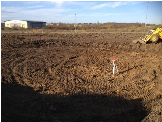
Plate 23: Initial ground reduction, from the south-east
