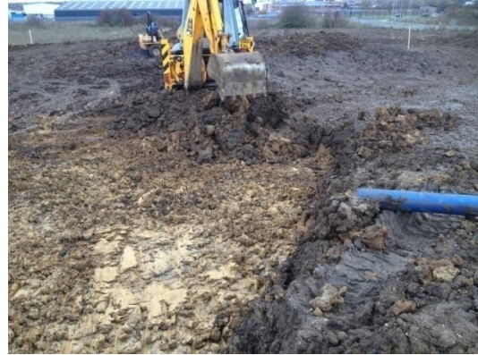
Plate 31: Initial ground reduction, from the east
