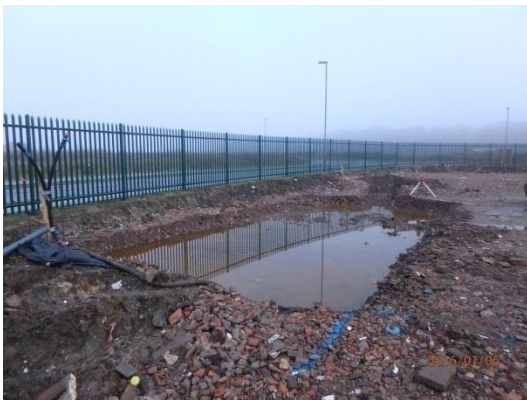
Plate 41: Set out storage tank, from the south-west
