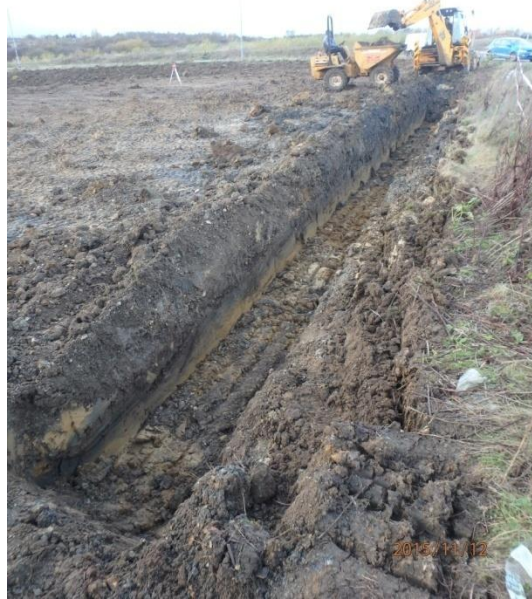
Plate 3: Initial ground reduction, from the south-east
