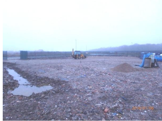
Plate 37: Compacted hardcore over the area of the development site, from the south
