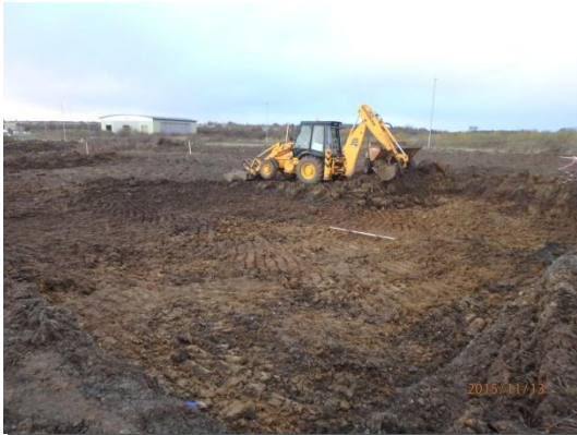
Plate 22: Initial ground reduction, from the east
