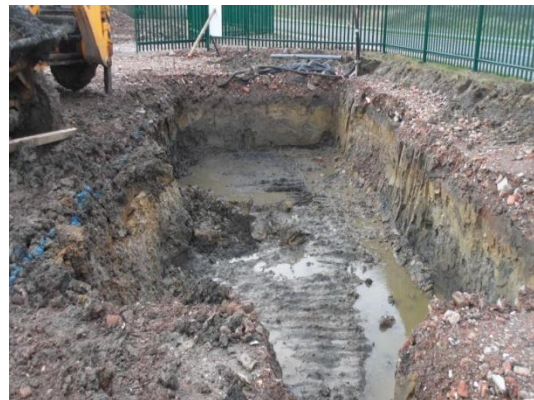
Plate 62: Excavation of the storage tank, from the north-east
