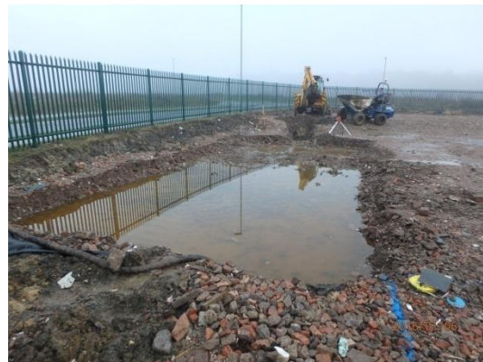
Plate 44: Excavation of the chamber and connecting trench, from the south-west
