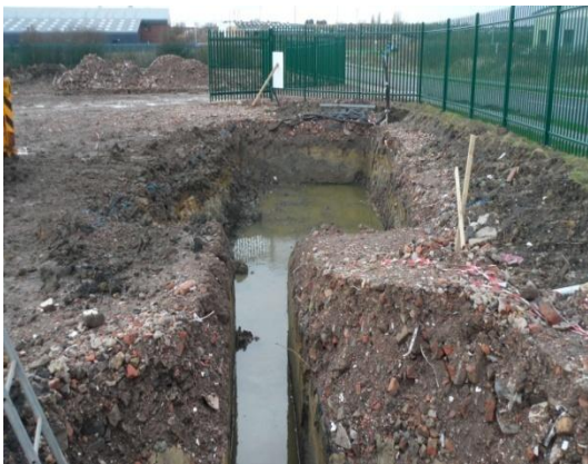
Plate 60: Excavation of the storage tank, from the north-east
