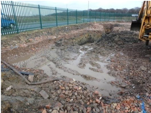
Plate 53: Excavation of the storage tank, from the south-west
