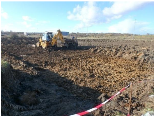
Plate 18: Initial ground reduction, from the east
