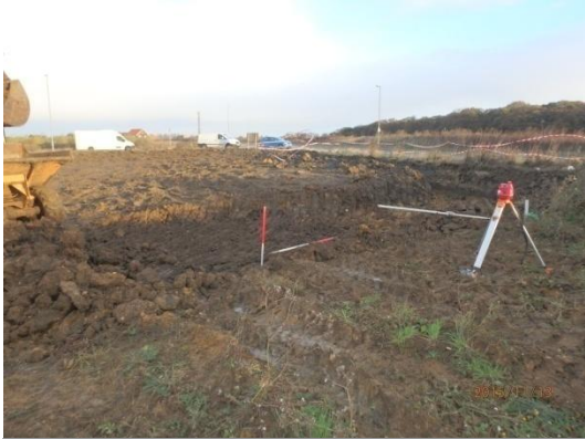
Plate 10: Initial ground reduction, from the south
