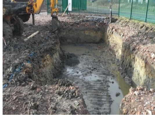
Plate 61: Excavation of the storage tank, from the north-east
