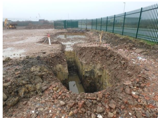
Plate 45: Completed excavation of the chamber and connecting trench, from the north-east
