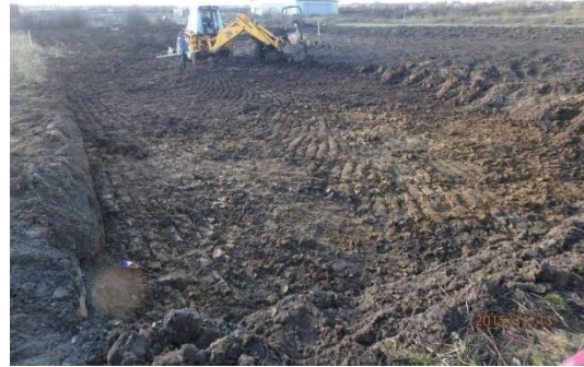
Plate 19: Initial ground reduction, from the east
