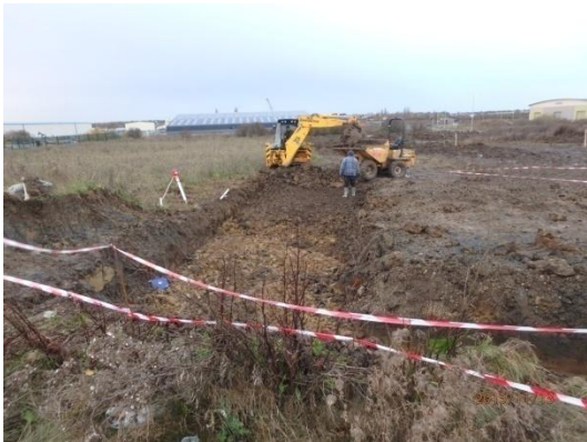
Plate 11: Initial ground reduction, from the north-east
