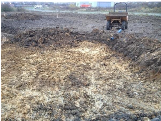
Plate 30: Initial ground reduction, from the south-east
