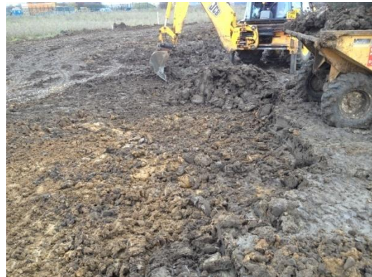
Plate 32: Initial ground reduction, from the east
