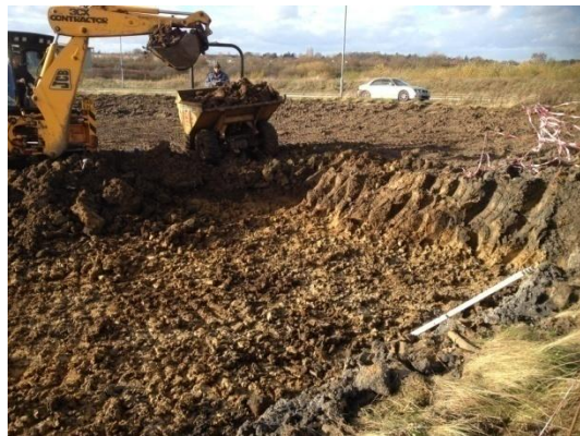
Plate 26: Initial ground reduction, from the east
