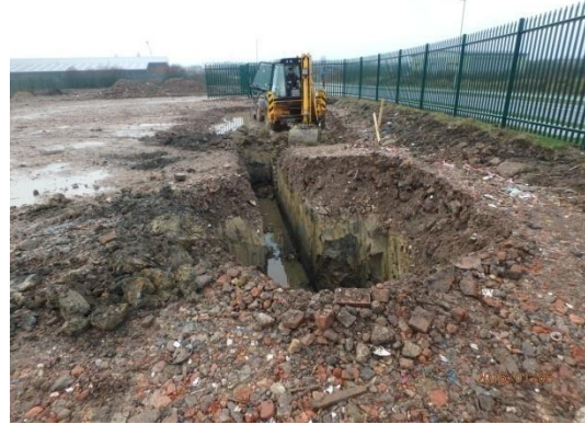
Plate 49: Excavation of the storage tank, from the north-east
