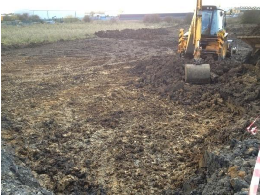
Plate 28: Initial ground reduction, from the east
