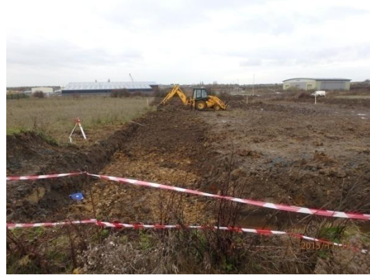
Plate 13: Initial ground reduction, from the north-east
