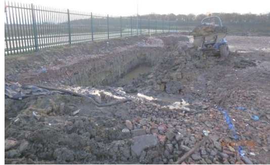
Plate 55: Excavation of the storage tank, from the south-west
