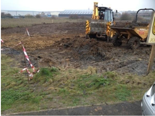
Plate 34: Initial ground reduction, from the east
