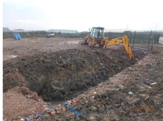
Plate 56: Excavation of the storage tank, from the north-west
