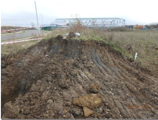
Plate 6: Section through the earthen bund around the site, from the north-east
