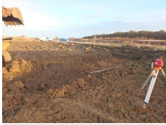
Plate 8: Initial ground reduction, from the south
