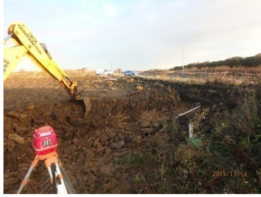
Plate 7: Initial ground reduction, from the south
