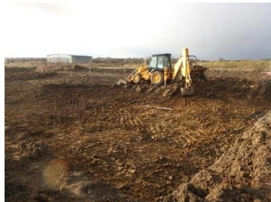
Plate 21: Initial ground reduction, from the east
