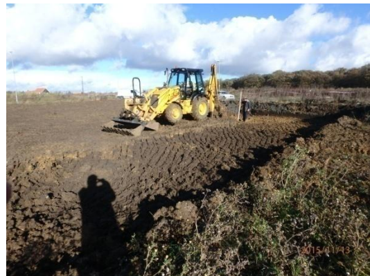
Plate 15: Initial ground reduction, from the south-east
