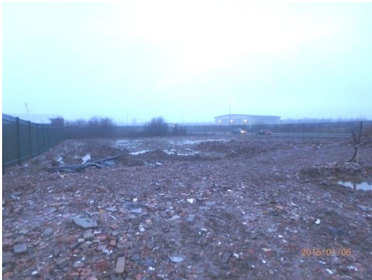
Plate 35: Compacted hardcore over the area of the development site, from the north-east
