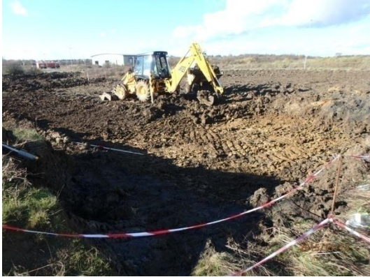
Plate 16: Initial ground reduction, from the east
