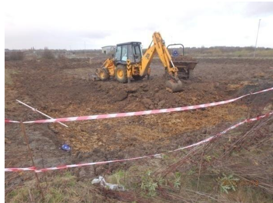
Plate 14: Initial ground reduction, from the east
