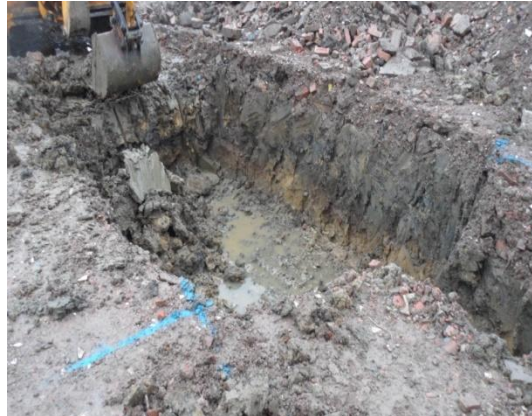
Plate 67: Excavation of the manhole, connecting trench and interceptor, from the south-east
