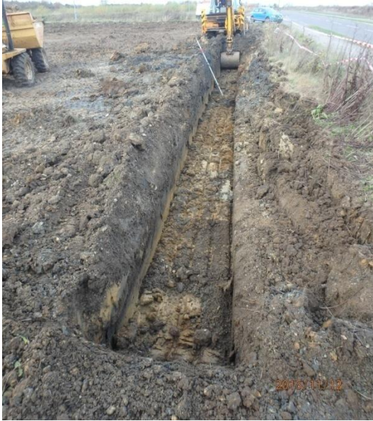
Plate 1: Initial ground reduction, from the south-east
