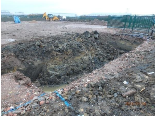
Plate 58: Excavation of the storage tank, from the north-west
