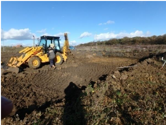
Plate 17: Initial ground reduction, from the south-east
