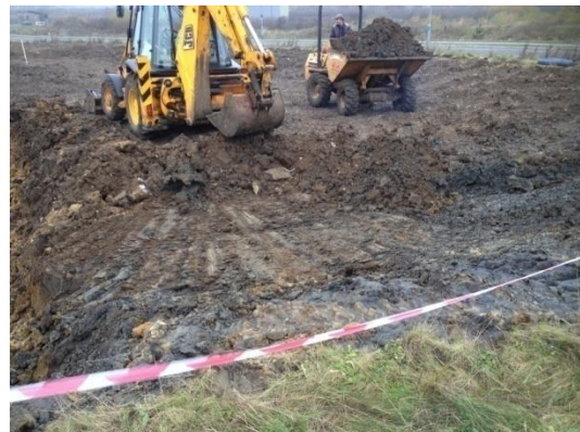
Plate 33: Initial ground reduction, from the east
