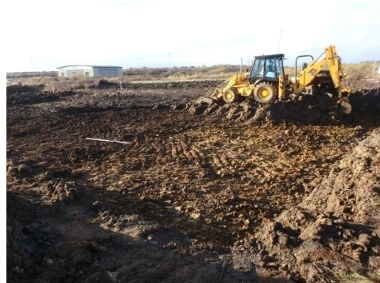
Plate 20: Initial ground reduction, from the east
