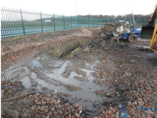
Plate 54: Excavation of the storage tank, from the south-west
