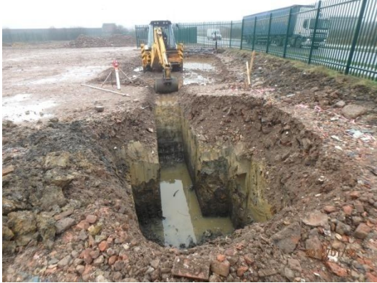
Plate 46: Completed excavation of the chamber and connecting trench, from the north-east
