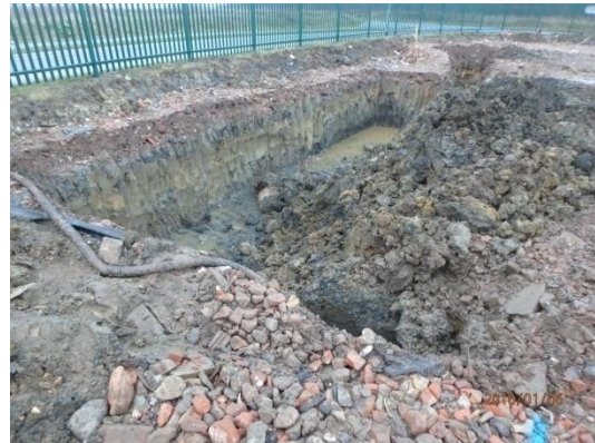
Plate 57: Excavation of the storage tank, from the south-west
