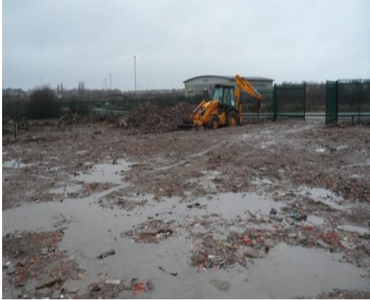
Plate 64: Excavation of the manhole, connecting trench and interceptor, from the south-east
