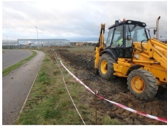
Plate 4: Initial ground reduction, from the north-east
