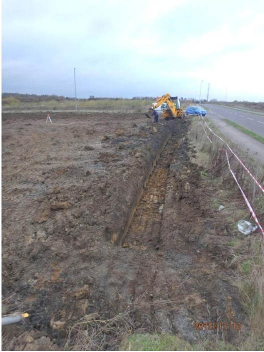
Plate 5: Initial ground reduction, from the south-east
