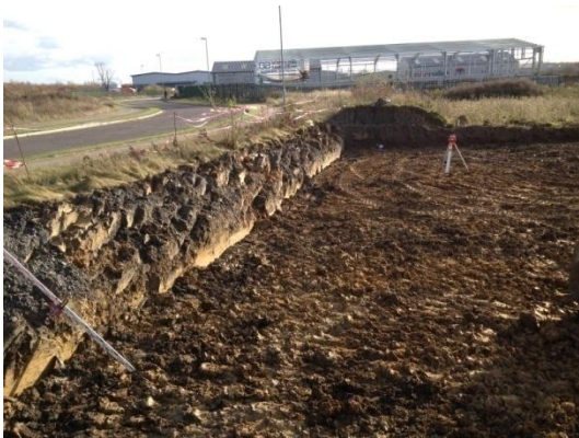
Plate 24: Initial ground reduction, from the north-west
