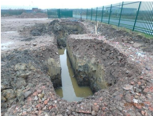
Plate 59: Excavation of the storage tank, from the north-east
