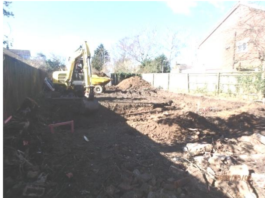
Plate 11: Excavation of the foundations, from the east
