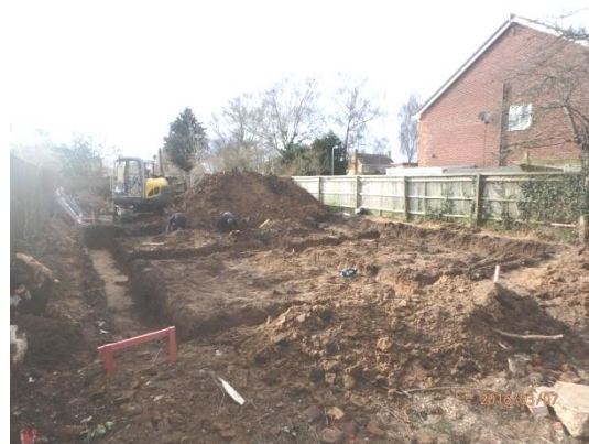
Plate 24: Excavation of the foundations, from the east
