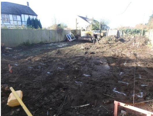
Plate 3: Set out foundations, from the east
