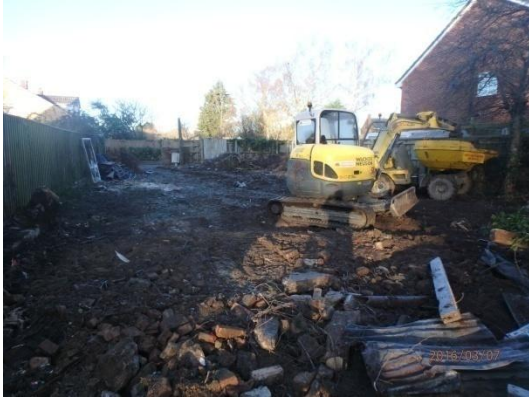
Plate 1: Pre-groundworks, from the east
