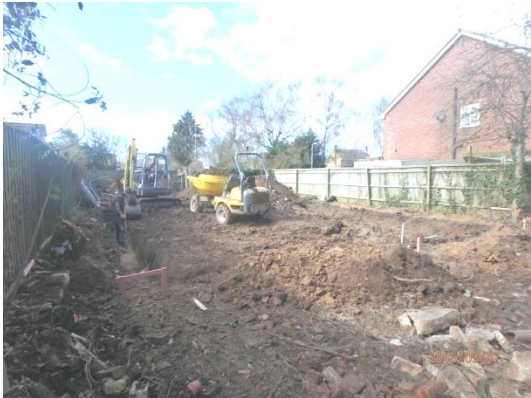
Plate 14: Excavation of the foundations, from the east
