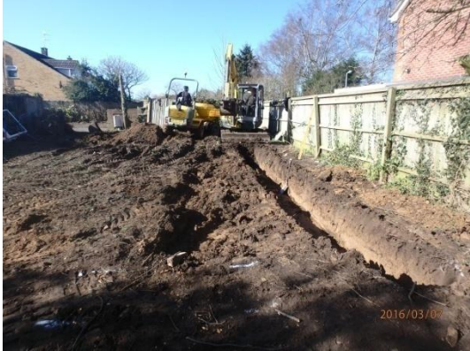
Plate 7: Excavation of the foundations, from the east
