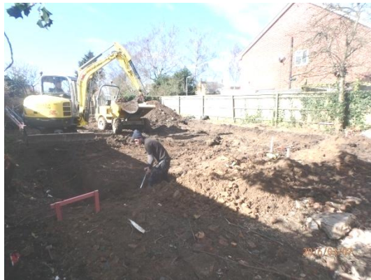
Plate 12: Excavation of the foundations, from the east
