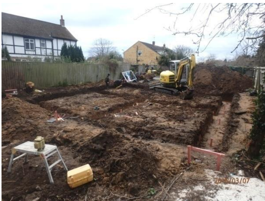
Plate 21: Excavation of the foundations, from the east
