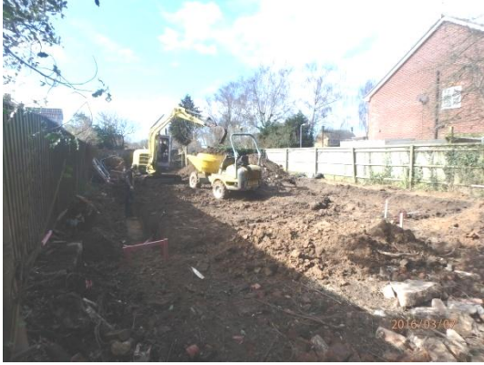
Plate 13: Excavation of the foundations, from the east
