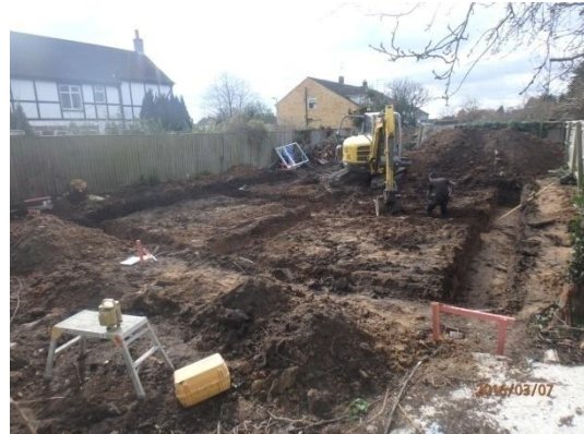
Plate 17: Excavation of the foundations, from the east
