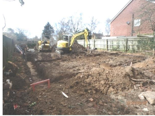
Plate 16: Excavation of the foundations, from the east
