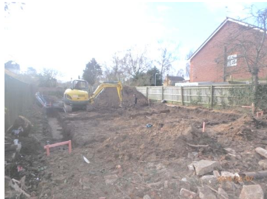
Plate 23: Excavation of the foundations, from the east
