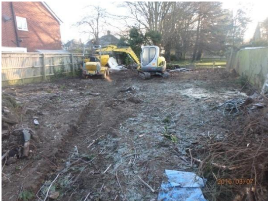
Plate 2: Pre-groundworks, from the west
