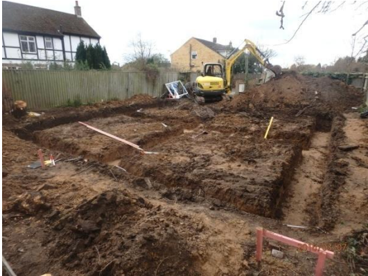
Plate 19: Excavation of the foundations, from the east
