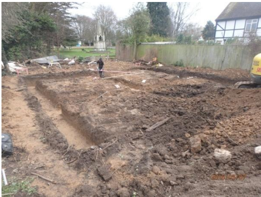
Plate 20: Excavation of the foundations, from the west
