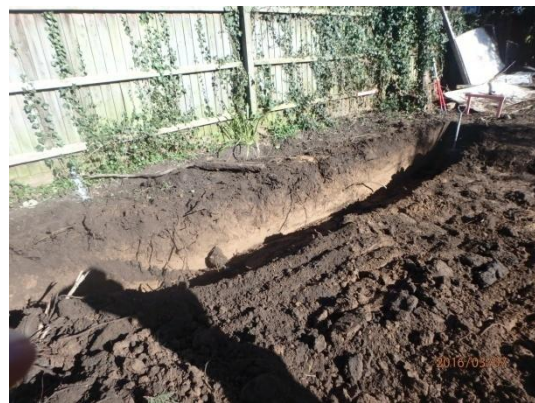
Plate 6: Excavation of the foundations, from the west
