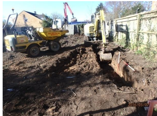
Plate 5: Excavation of the foundations, from the east
