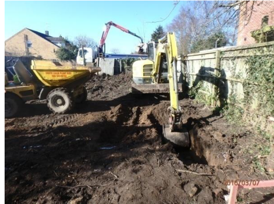
Plate 4: Excavation of the foundations, from the east
