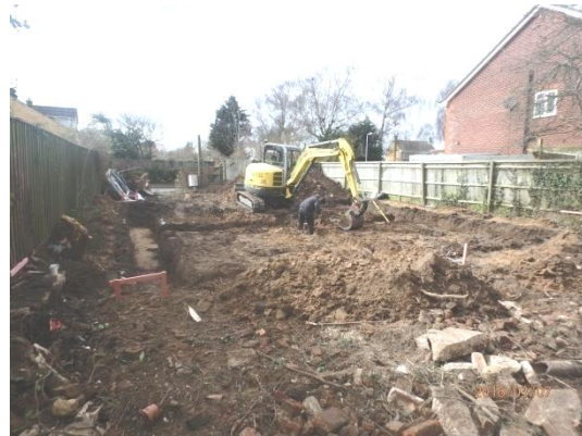
Plate 18: Excavation of the foundations, from the east
