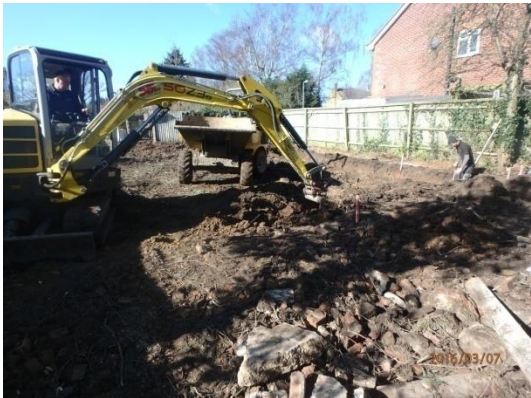
Plate 9: Excavation of the foundations, from the east
