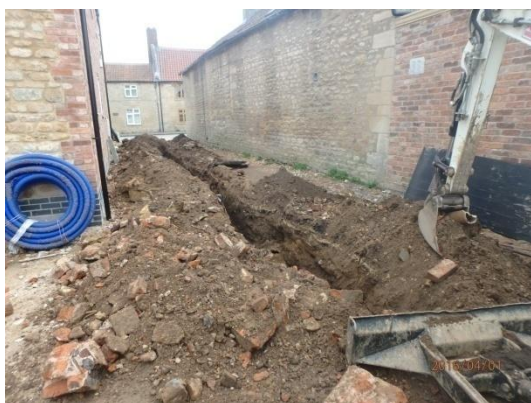
Plate 45: Excavation of the service trench, from the west
