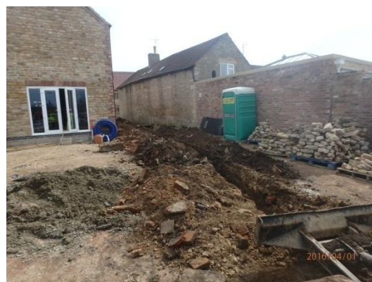
Plate 47: Excavation of the service trench, from the west
