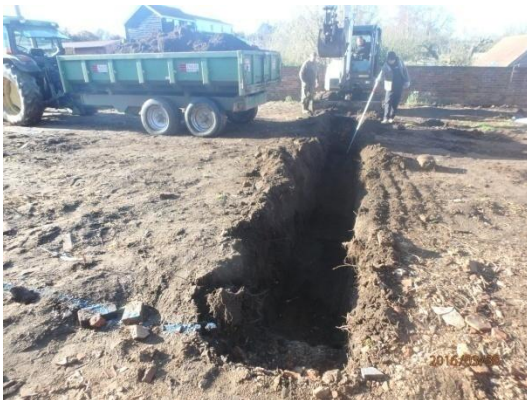
Plate 3: Excavation of the foundations, from the north
