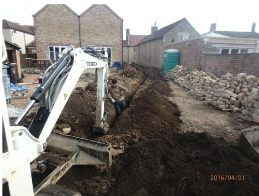
Plate 51: Excavation of the service trench, from the west
