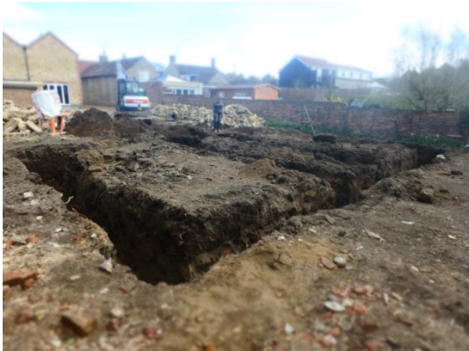
Plate 26: Excavation of the foundations, from the west
