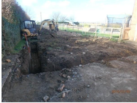
Plate 14: Excavation of the foundations, from the east
