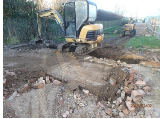
Plate 4: Excavation of the foundations, from the east
