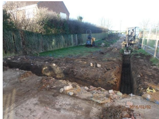
Plate 6: Excavation of the foundations, from the east
