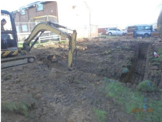
Plate 18: Excavation of the foundations, from the west
