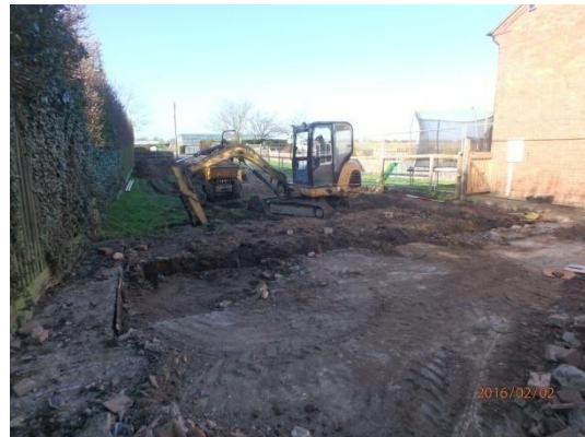
Plate 10: Excavation of the foundations, from the east
