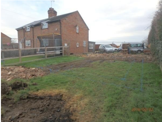
Plate 2: Pre-groundworks, from the west
