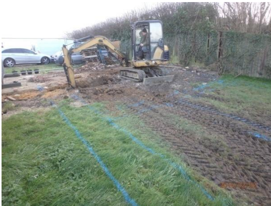
Plate 3: Excavation of the foundations, from the west
