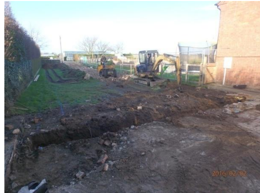
Plate 5: Excavation of the foundations, from the east
