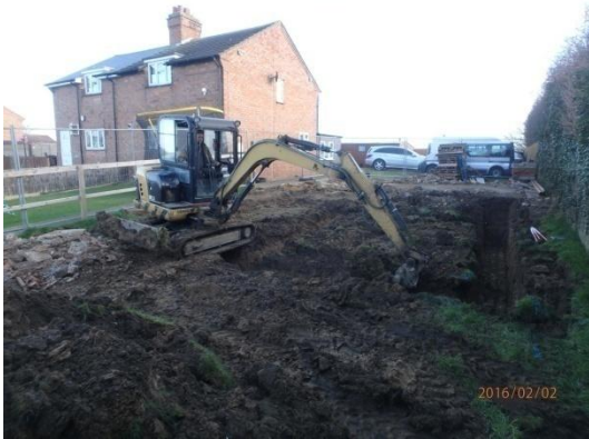
Plate 17: Excavation of the foundations, from the west
