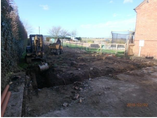
Plate 12: Excavation of the foundations, from the east
