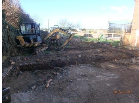
Plate 9: Excavation of the foundations, from the east
