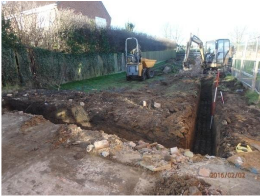
Plate 8: Excavation of the foundations, from the east
