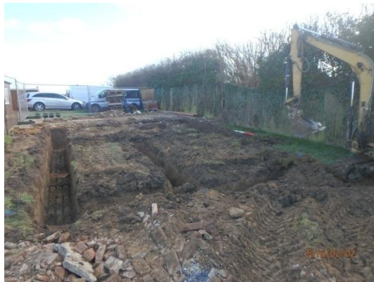
Plate 16: Excavation of the foundations, from the west
