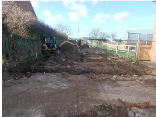
Plate 15: Excavation of the foundations, from the east
