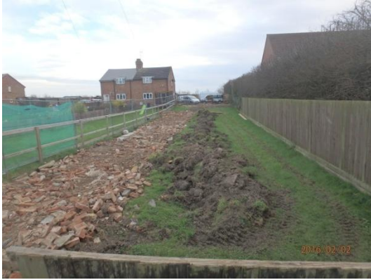
Plate 1: Pre-groundworks, from the west
