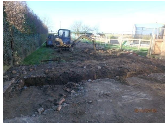
Plate 11: Excavation of the foundations, from the east
