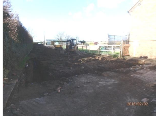
Plate 19: Excavation of the foundations, from the east
