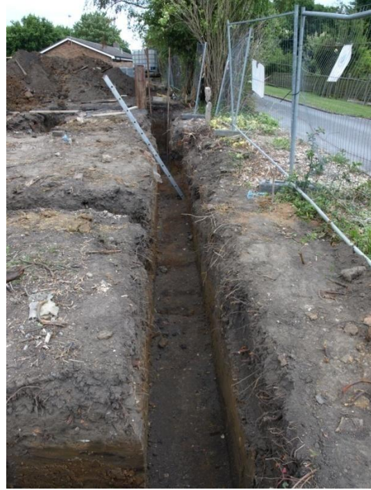
Plate 27: Excavation of the foundations, from the west
