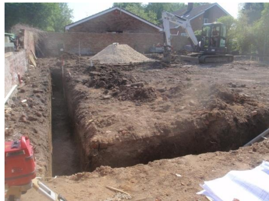
Plate 6: Excavation of the foundations, from the west
