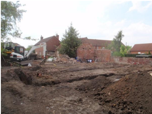
Plate 14: Excavation of the foundations, from the east
