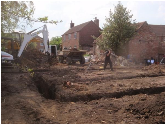
Plate 20: Excavation of the foundations, from the east
