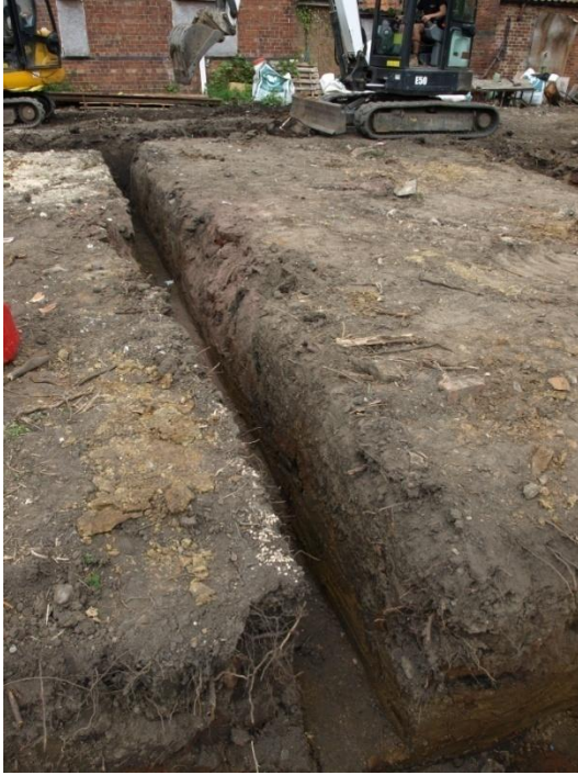
Plate 29: Excavation of the foundations, from the south
