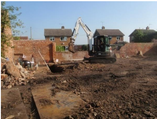
Plate 2: Excavation of the foundations, from the south
