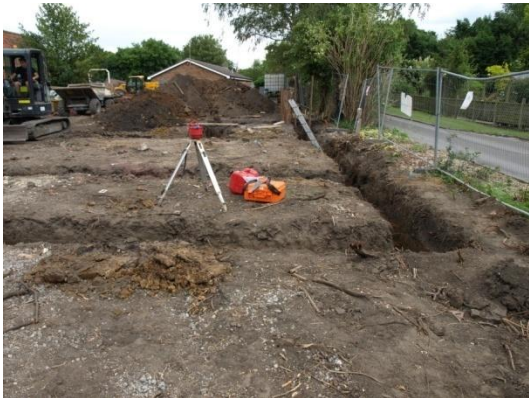
Plate 25: Excavation of the foundations, from the west
