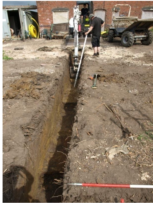
Plate 23: Excavation of the foundations, from the south
