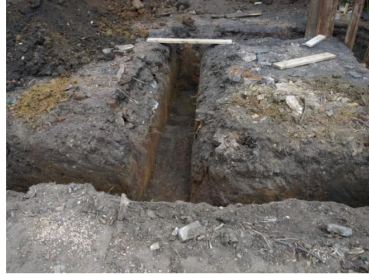
Plate 31: Excavation of the foundations, from the west
