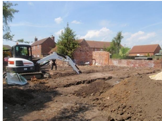
Plate 11: Excavation of the foundations, from the east
