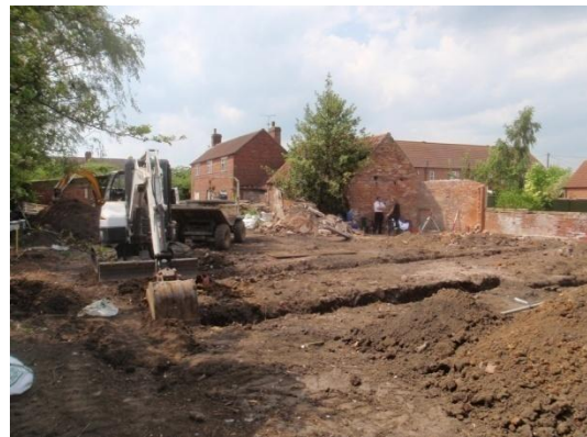
Plate 12: Excavation of the foundations, from the east
