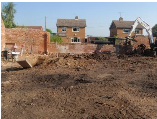
Plate 3: Excavation of the foundations, from the south
