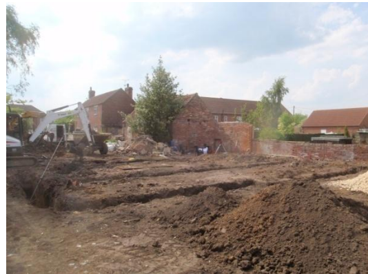
Plate 17: Excavation of the foundations, from the east
