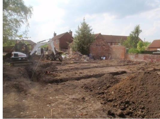
Plate 16: Excavation of the foundations, from the east
