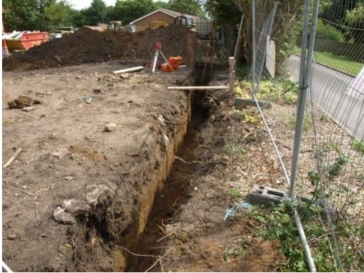
Plate 24: Excavation of the foundations, from the west
