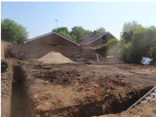
Plate 9: Excavation of the foundations, from the west
