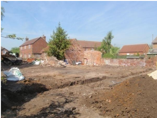
Plate 8: Excavation of the foundations, from the east
