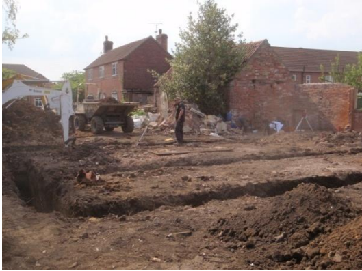
Plate 19: Excavation of the foundations, from the east
