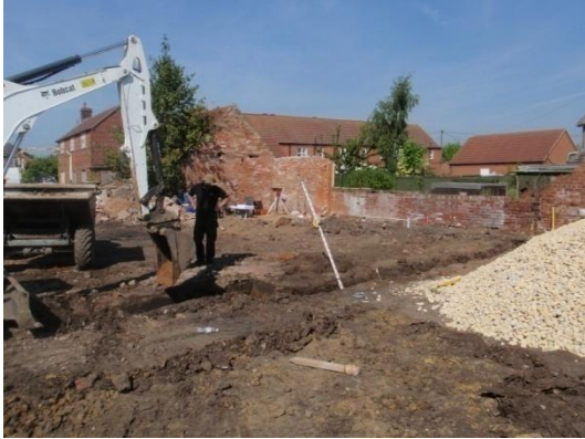
Plate 7: Excavation of the foundations, from the east
