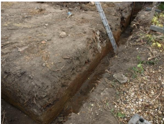
Plate 30: Excavation of the foundations, from the west
