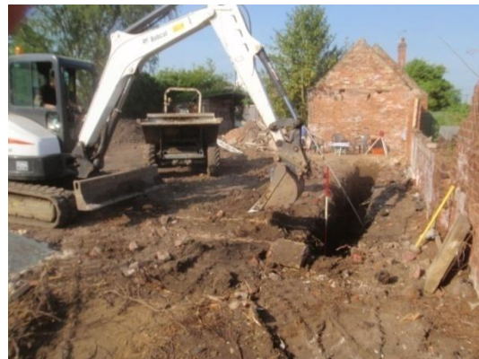
Plate 5: Excavation of the foundations, from the east
