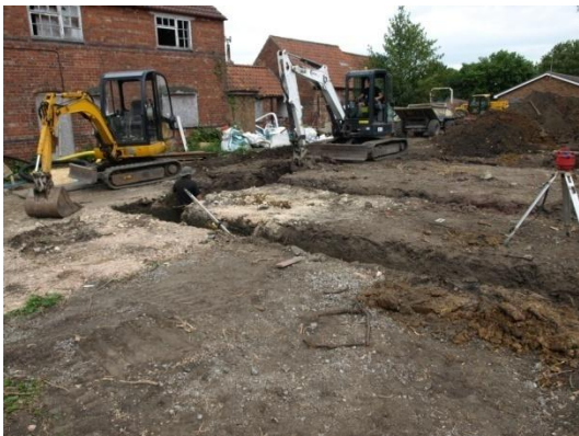
Plate 26: Excavation of the foundations, from the west
