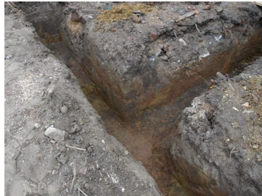
Plate 32: Excavation of the foundations, from the south
