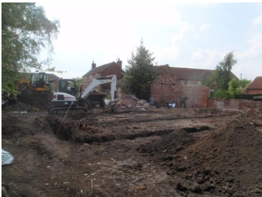
Plate 15: Excavation of the foundations, from the east
