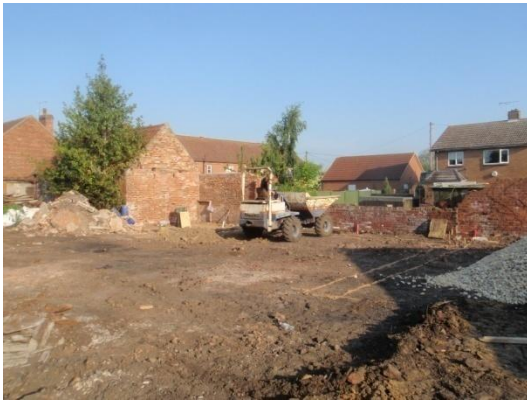
Plate 1: Set out foundations, from the south-east
