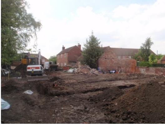
Plate 13: Excavation of the foundations, from the east
