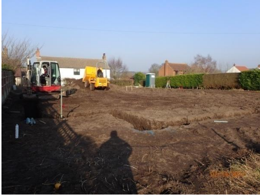
Plate 13: Excavation of the foundations, from the south
