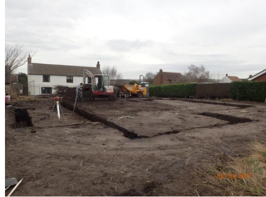
Plate 34: Excavation of the foundations, from the south
