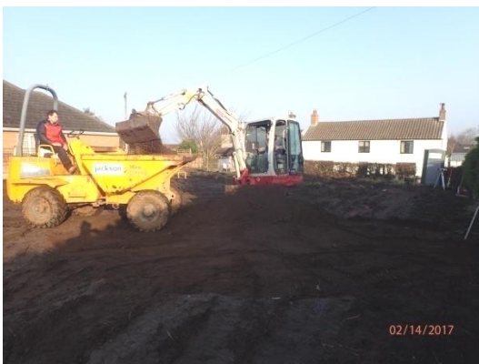
Plate 3: Initial ground reduction, from the south
