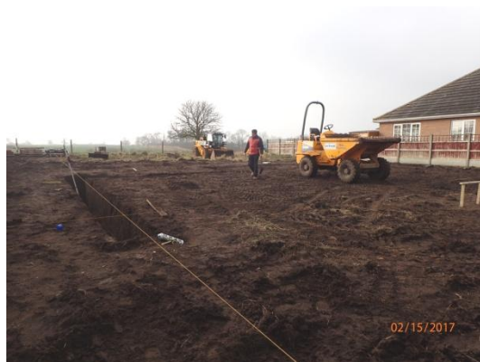
Plate 22: Excavation of the foundations, from the north
