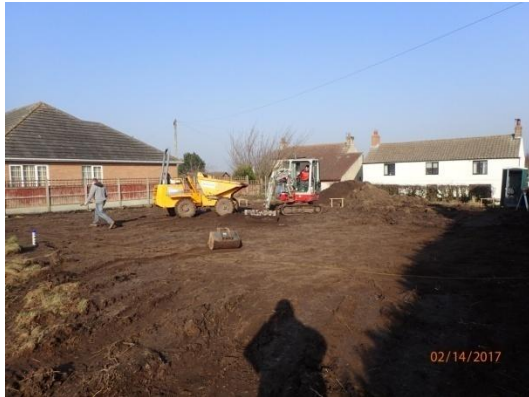
Plate 7: Initial ground reduction, from the south-east
