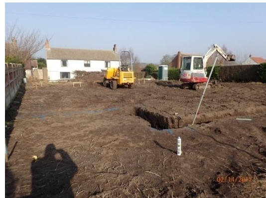
Plate 11: Excavation of the foundations, from the south
