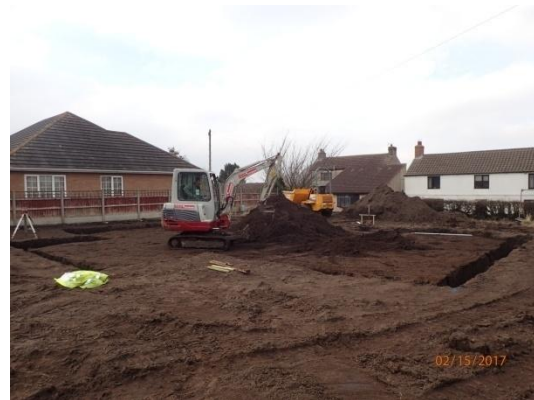
Plate 29: Further ground reduction, from the south-east
