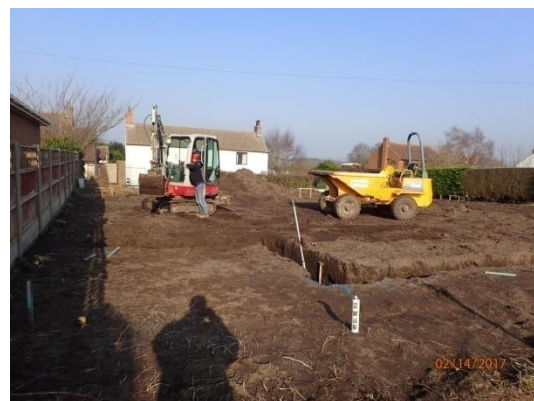
Plate 12: Excavation of the foundations, from the south
