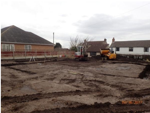
Plate 32: Excavation of the foundations, from the south
