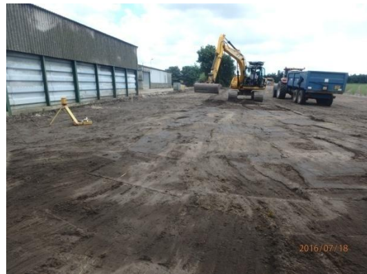
Plate 11: Initial ground reduction, from the north
