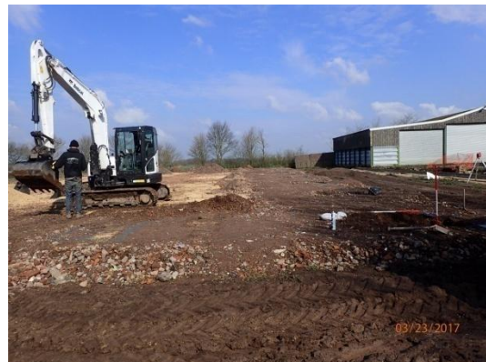
Plate 54: Excavation of the stanchion bases, from the south
