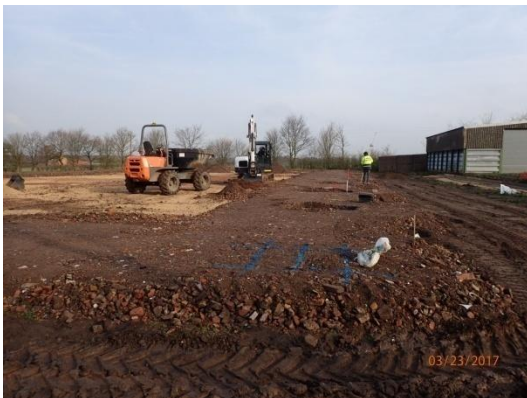
Plate 33: Excavation of the stanchion bases, from the south
