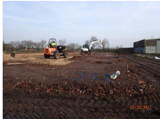
Plate 35: Excavation of the stanchion bases, from the south
