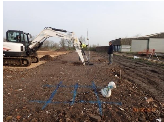
Plate 29: Excavation of the stanchion bases, from the south
