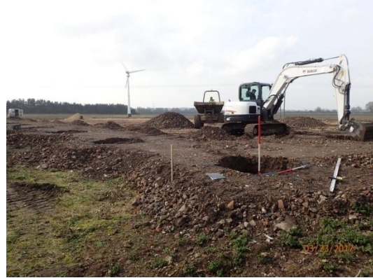
Plate 46: Excavation of the stanchion bases, from the north
