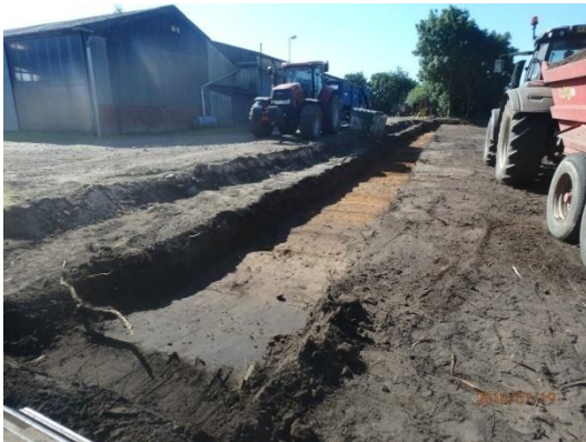
Plate 26: Excavation of the service trench, from the north
