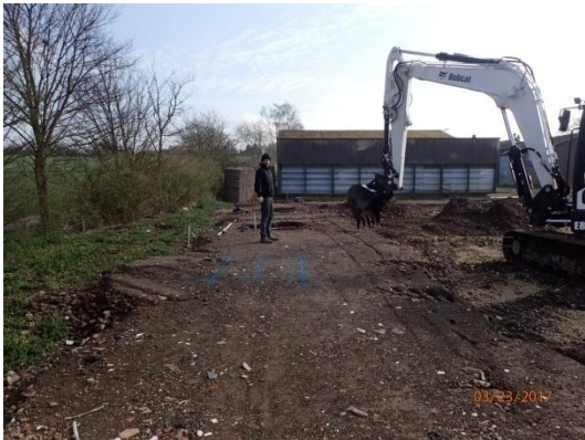
Plate 50: Excavation of the stanchion bases, from the west
