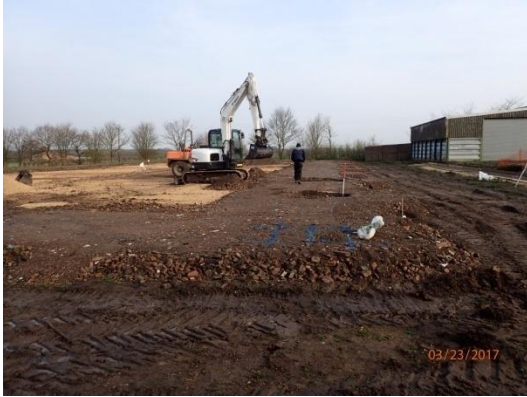
Plate 31: Excavation of the stanchion bases, from the south
