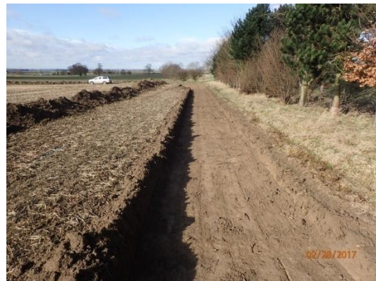
Plate 24: Ground reduction, from the east
