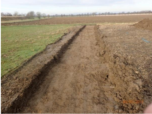
Plate 43: Ground reduction, from the west
