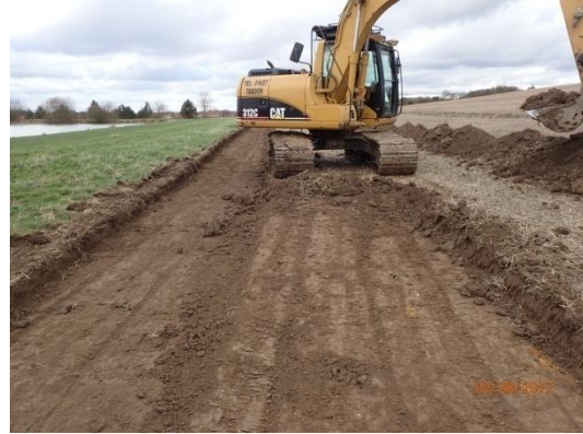
Plate 34: Ground reduction, from the south
