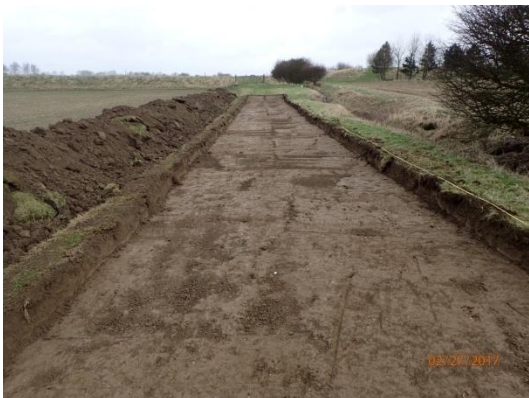
Plate 9: Ground reduction, from the south
