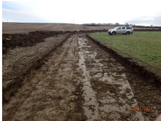
Plate 47: Ground reduction, from the west
