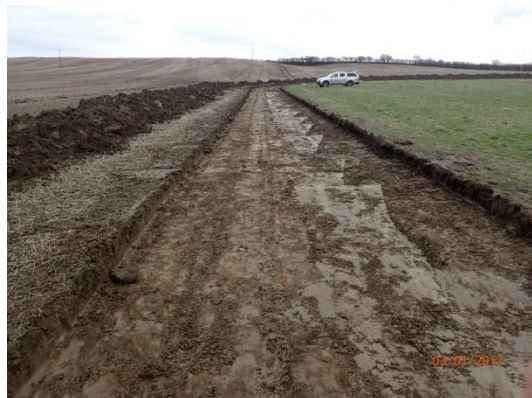
Plate 48: Ground reduction, from the west
