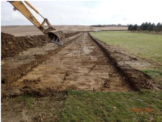
Plate 50: Ground reduction, from the west
