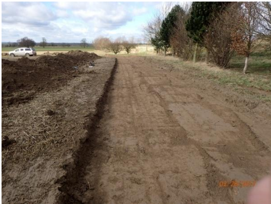
Plate 26: Ground reduction, from the east
