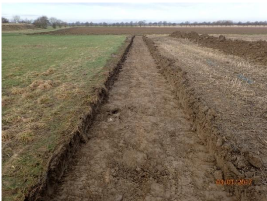
Plate 45: Ground reduction, from the west
