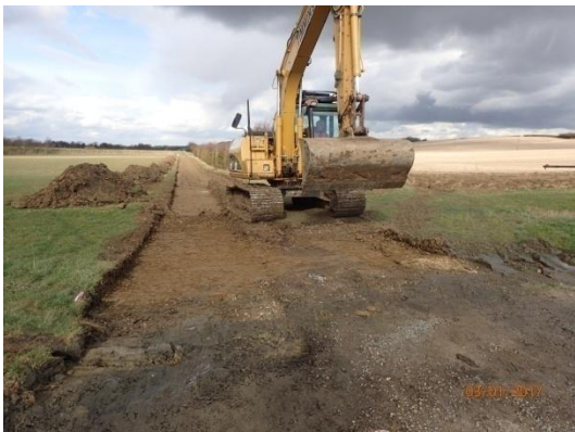
Plate 51: Ground reduction, from the south
