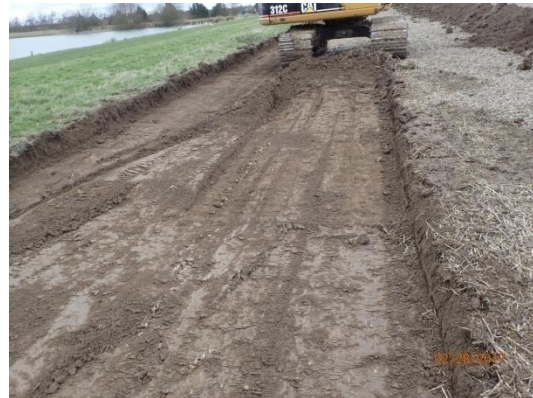
Plate 35: Ground reduction, from the south
