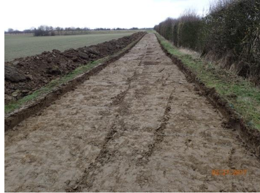
Plate 16: Ground reduction, from the south
