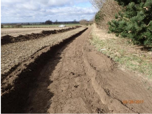
Plate 25: Ground reduction, from the east
