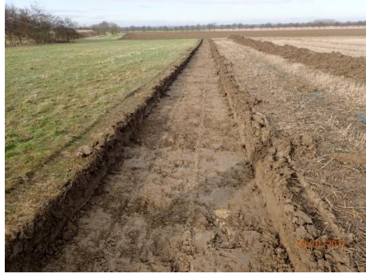
Plate 46: Ground reduction, from the west
