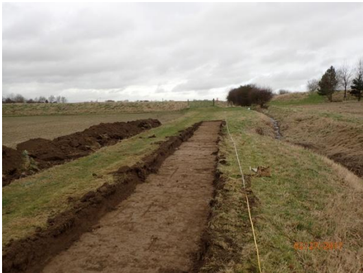
Plate 3: Ground reduction, from the south
