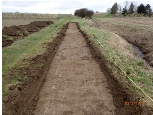
Plate 4: Ground reduction, from the south
