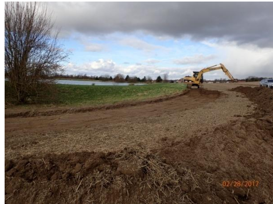
Plate 29: Ground reduction, from the south
