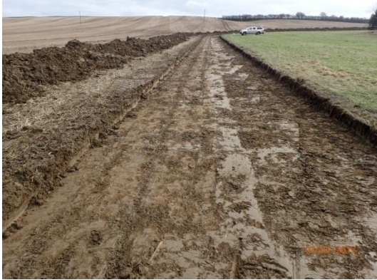
Plate 49: Ground reduction, from the west
