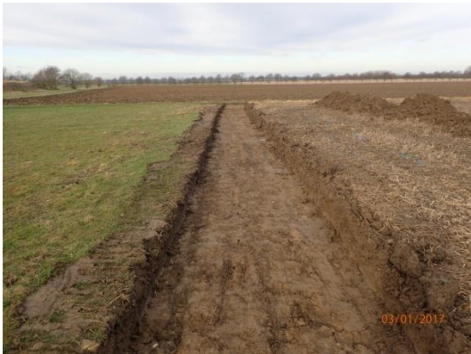
Plate 44: Ground reduction, from the west
