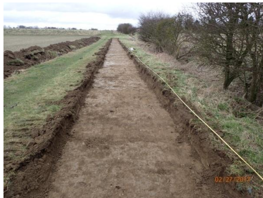
Plate 6: Ground reduction, from the south
