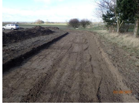
Plate 22: Ground reduction, from the east
