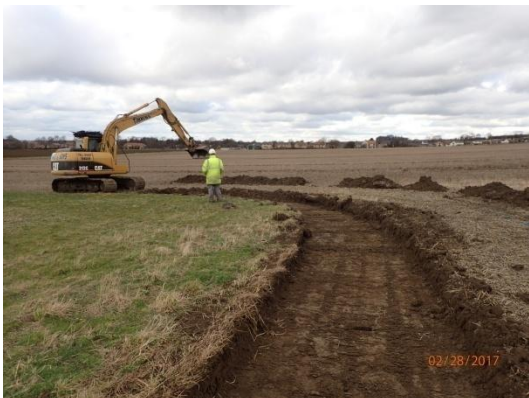
Plate 33: Ground reduction, from the south
