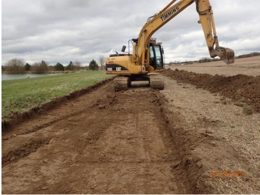
Plate 37: Ground reduction, from the south
