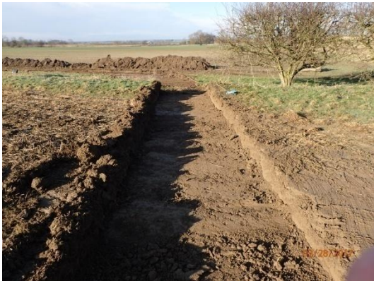
Plate 21: Ground reduction, from the east
