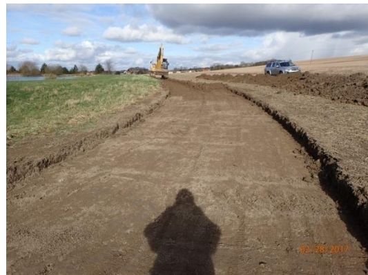
Plate 30: Ground reduction, from the south
