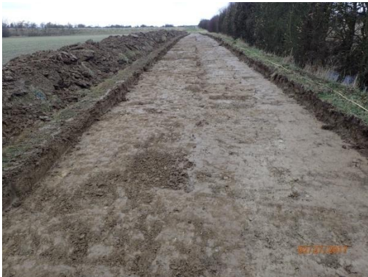
Plate 14: Ground reduction, from the south
