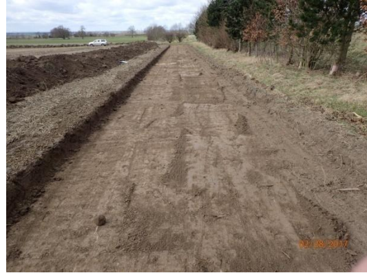
Plate 28: Ground reduction, from the east
