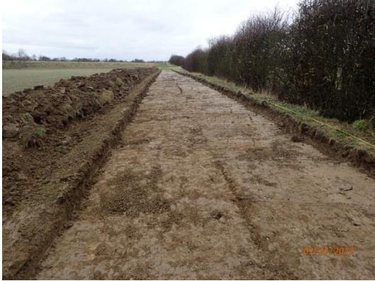
Plate 13: Ground reduction, from the south
