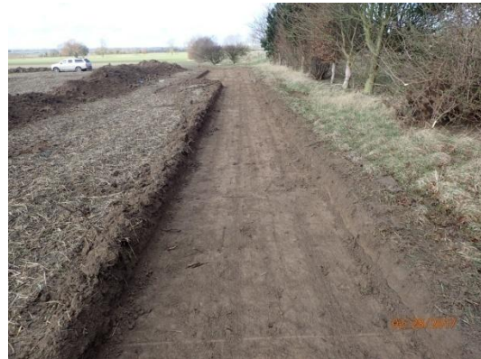
Plate 23: Ground reduction, from the east
