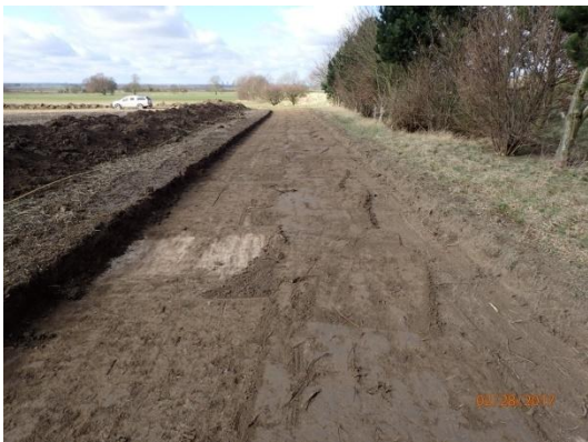
Plate 27: Ground reduction, from the east
