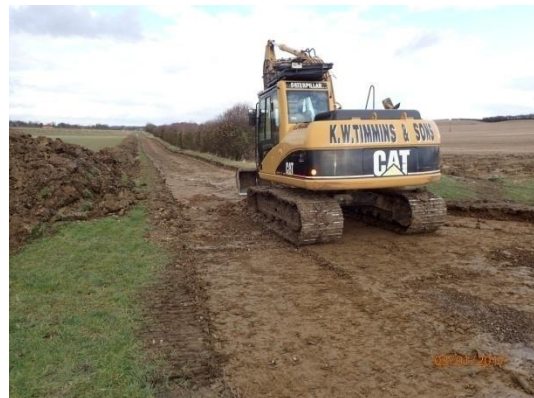
Plate 54: Ground reduction, from the south
