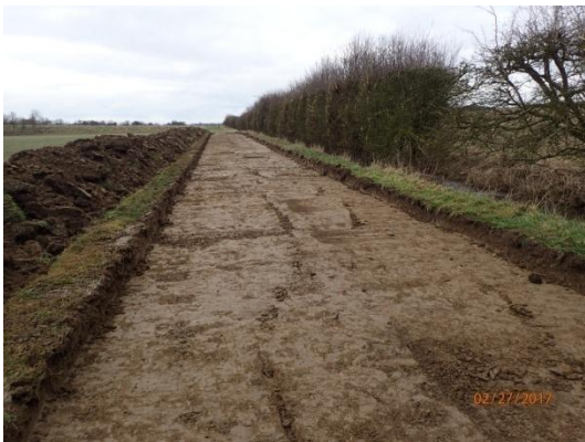
Plate 15: Ground reduction, from the south
