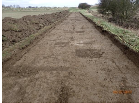
Plate 10: Ground reduction, from the south
