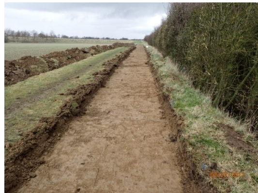
Plate 12: Ground reduction, from the south
