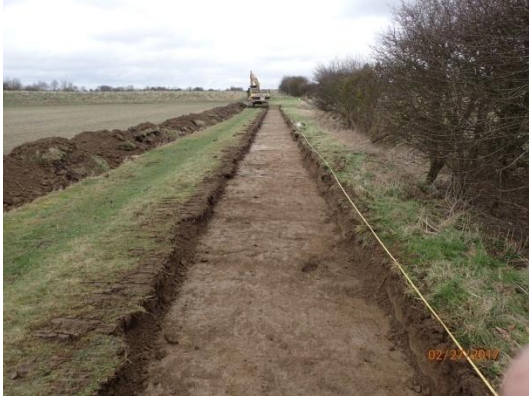
Plate 7: Ground reduction, from the south
