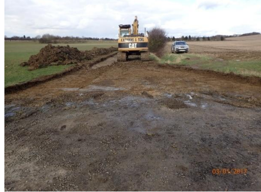
Plate 52: Ground reduction, from the south
