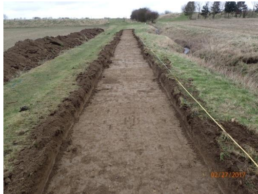
Plate 5: Ground reduction, from the south
