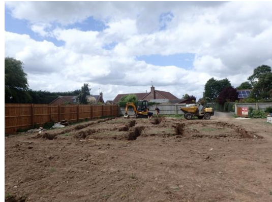
Plate 58: Excavation of the foundations, from the south
