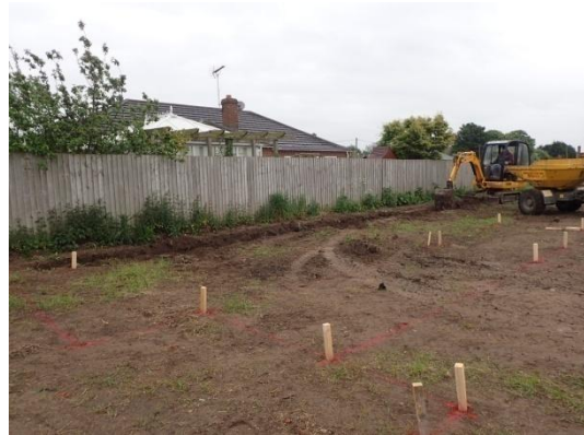
Plate 4: Excavation of the foundations, from the north-west
