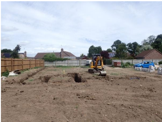
Plate 44: Excavation of the foundations, from the south
