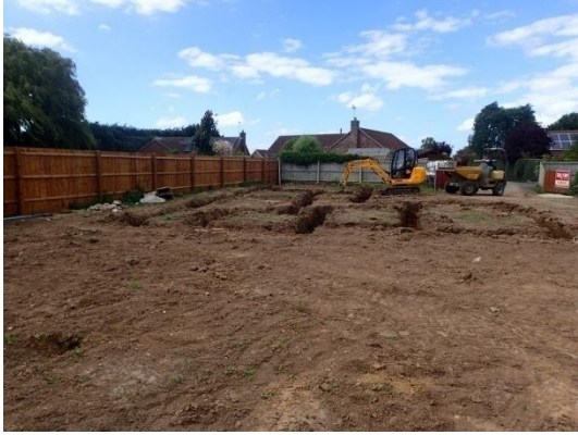
Plate 60: Completed excavation of the foundations, from the south
