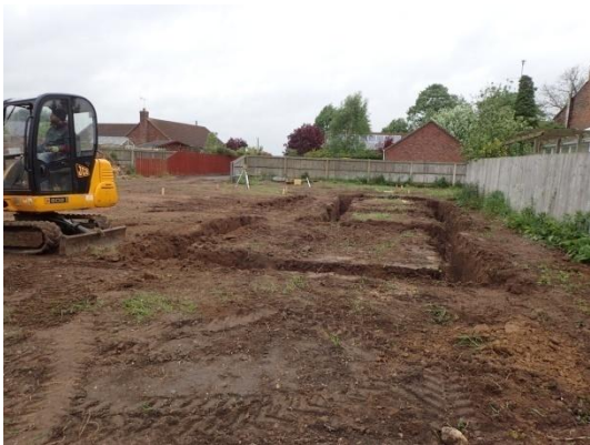
Plate 14: Excavation of the foundations, from the south
