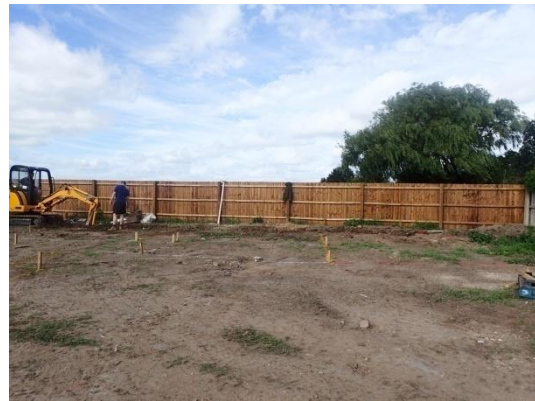
Plate 35: Excavation of the foundations, from the east
