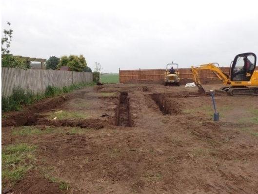
Plate 18: Excavation of the foundations, from the north
