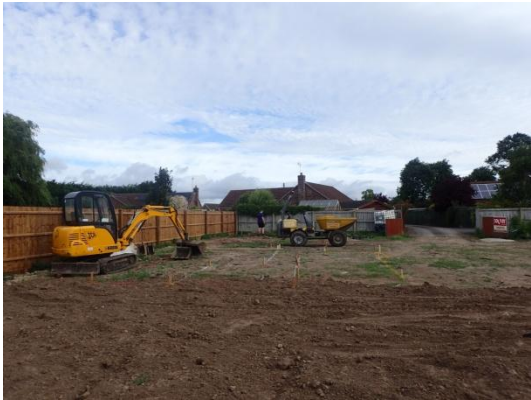
Plate 31: Pre-groundworks, from the south
