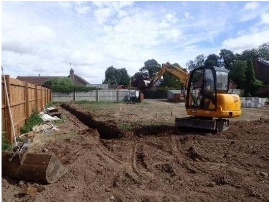
Plate 37: Excavation of the foundations, from the south
