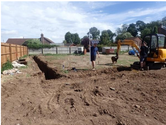
Plate 38: Excavation of the foundations, from the south
