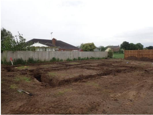
Plate 25: Completed foundations, from the west
