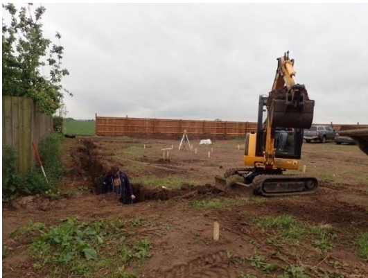
Plate 8: Excavation of the foundations, from the north
