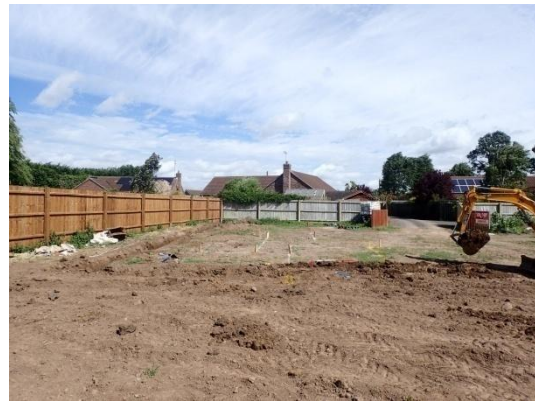
Plate 41: Excavation of the foundations, from the south
