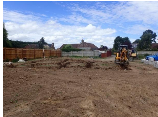
Plate 53: Excavation of the foundations, from the south
