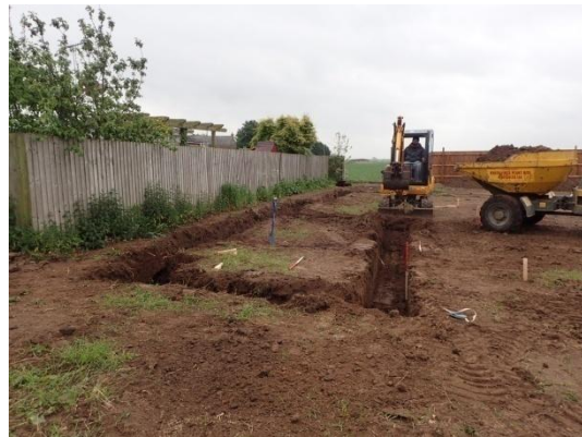
Plate 11: Excavation of the foundations, from the north
