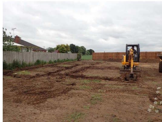
Plate 17: Excavation of the foundations, from the north
