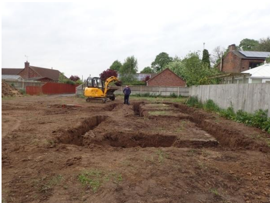
Plate 20: Excavation of the foundations, from the south
