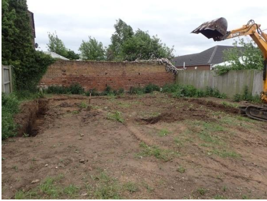
Plate 30: Completed foundations, from the west
