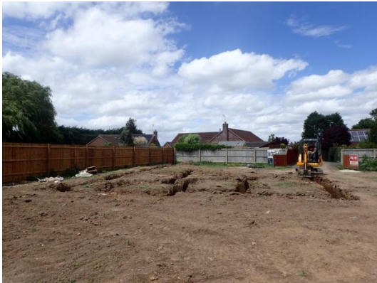
Plate 55: Excavation of the foundations, from the south
