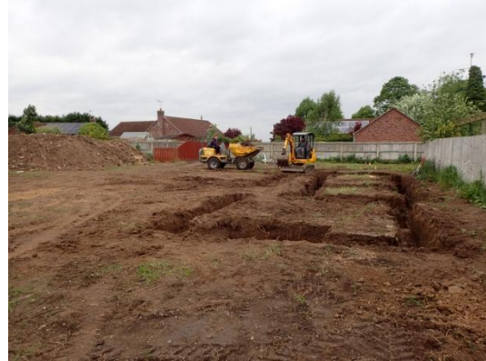
Plate 21: Excavation of the foundations, from the south
