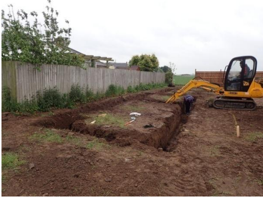
Plate 12: Excavation of the foundations, from the north
