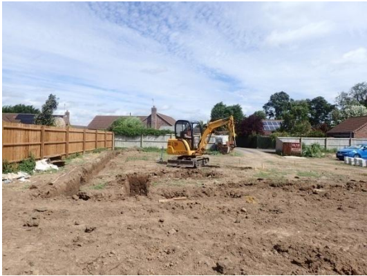
Plate 43: Excavation of the foundations, from the south
