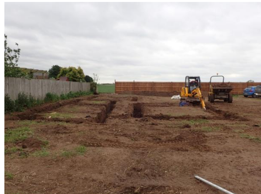
Plate 23: Excavation of the foundations, from the north
