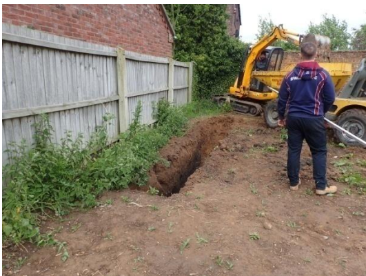
Plate 26: Excavation of the foundations, from the west
