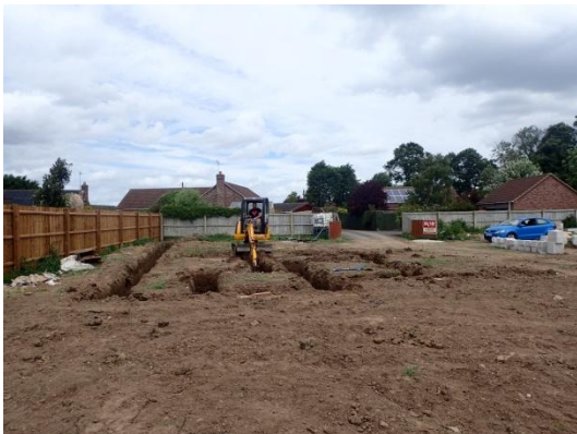
Plate 50: Excavation of the foundations, from the south
