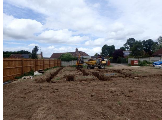
Plate 51: Excavation of the foundations, from the south
