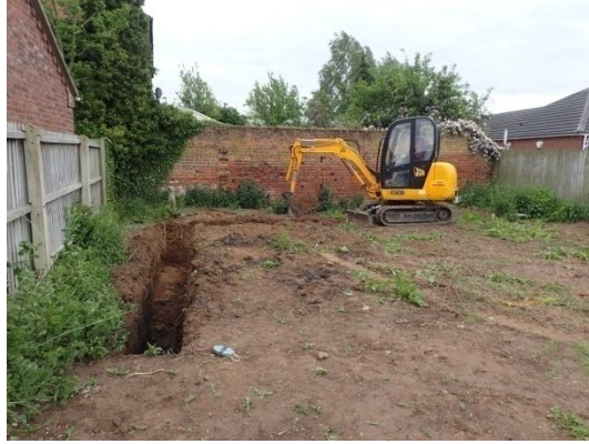
Plate 27: Excavation of the foundations, from the west
