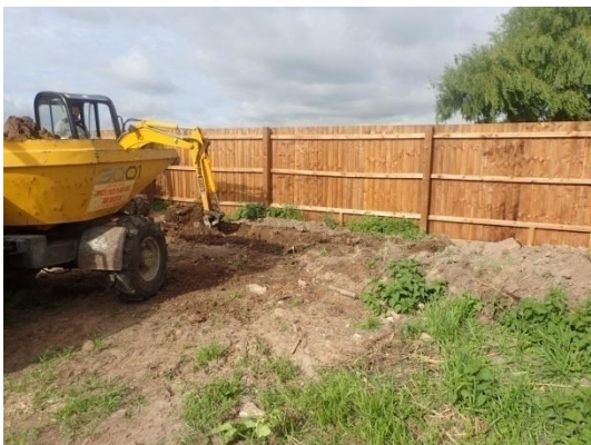
Plate 32: Excavation of the foundations, from the east
