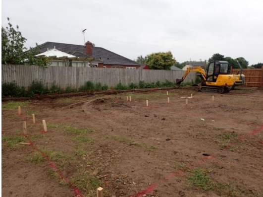
Plate 6: Excavation of the foundations, from the north-west
