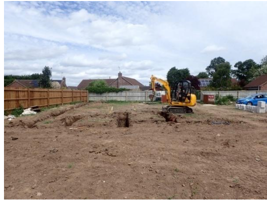
Plate 46: Excavation of the foundations, from the south
