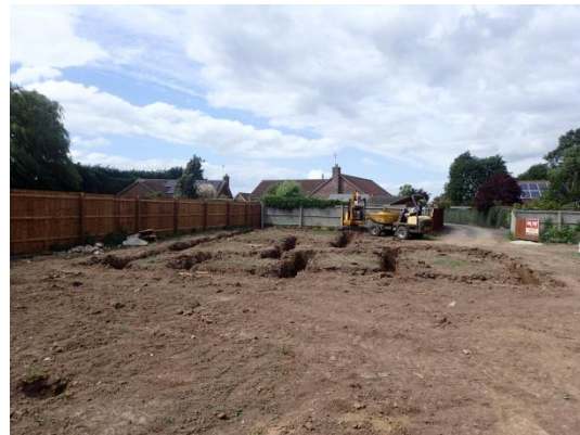
Plate 59: Excavation of the foundations, from the south
