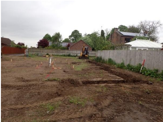
Plate 7: Excavation of the foundations, from the south
