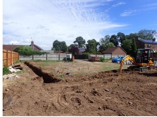
Plate 39: Excavation of the foundations, from the south
