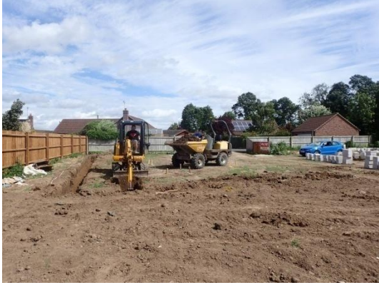
Plate 42: Excavation of the foundations, from the south
