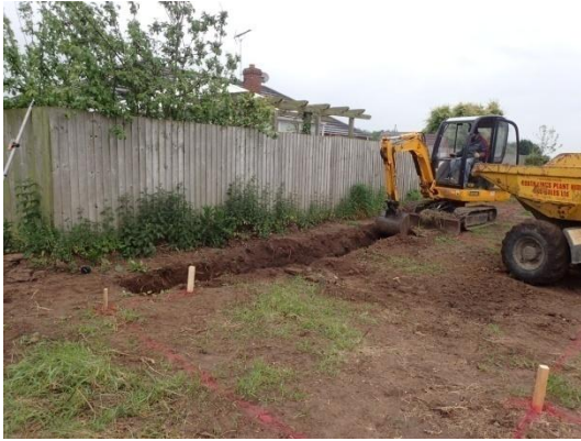
Plate 1: Excavation of the foundations, from the north-west
