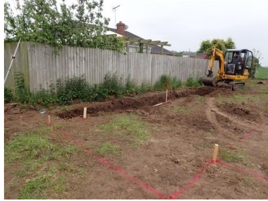
Plate 3: Excavation of the foundations, from the north-west
