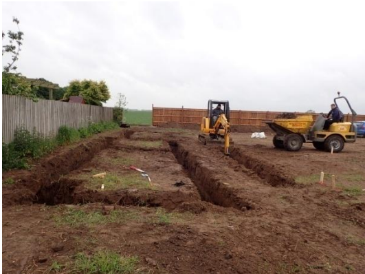
Plate 13: Excavation of the foundations, from the north
