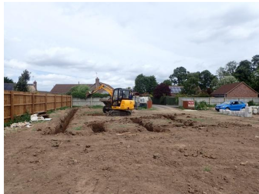
Plate 47: Excavation of the foundations, from the south
