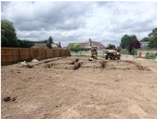
Plate 56: Excavation of the foundations, from the south
