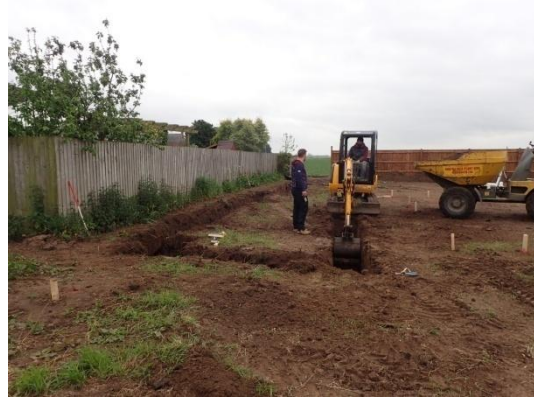
Plate 9: Excavation of the foundations, from the north
