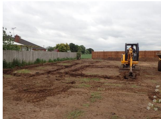
Plate 22: Excavation of the foundations, from the north
