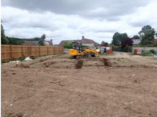
Plate 48: Excavation of the foundations, from the south
