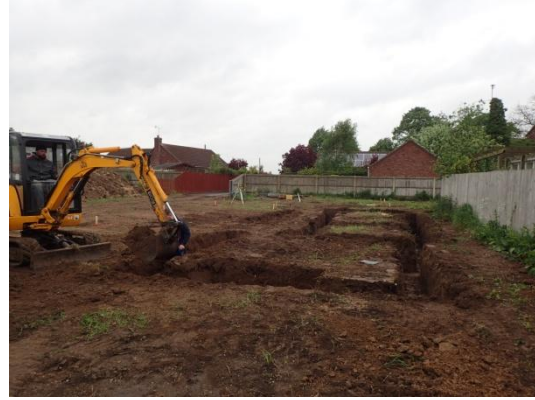
Plate 15: Excavation of the foundations, from the south
