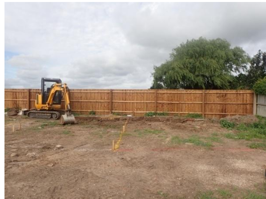
Plate 34: Excavation of the foundations, from the east
