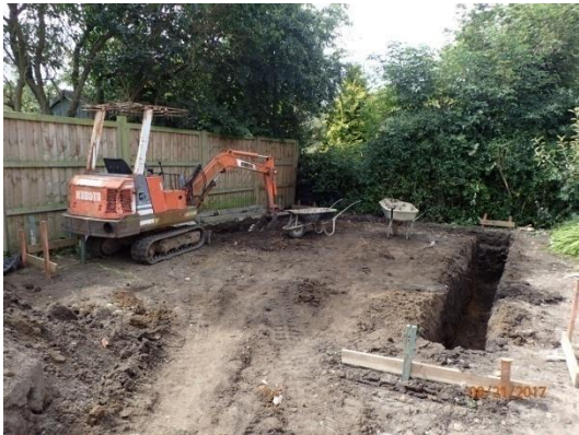
Plate 38: Excavation of the foundations, from the east
