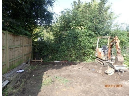
Plate 29: Excavation of the foundations, from the east
