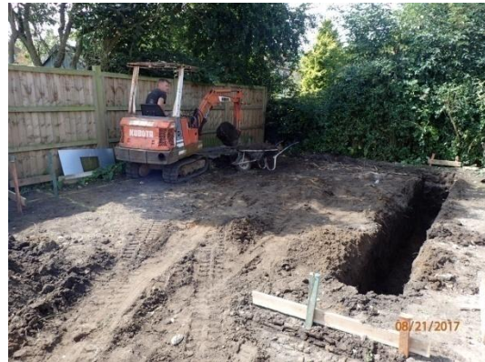
Plate 35: Excavation of the foundations, from the east
