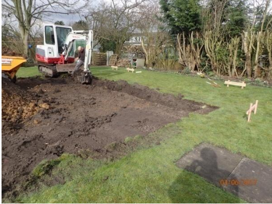
Plate 7: Excavation of the foundations, from the south-east
