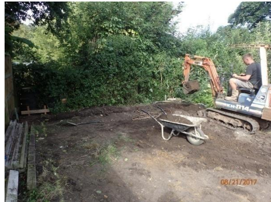
Plate 30: Excavation of the foundations, from the east
