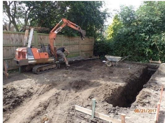
Plate 36: Excavation of the foundations, from the east
