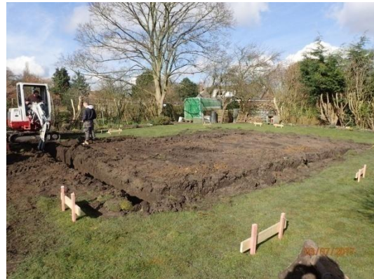
Plate 24: Excavation of the foundations, from the south-east
