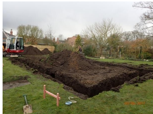
Plate 18: Excavation of the foundations, from the north-east
