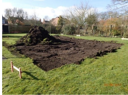
Plate 4: Initial ground reduction, from the north-east
