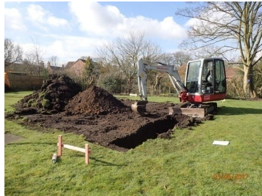
Plate 5: Excavation of the foundations, from the north-east
