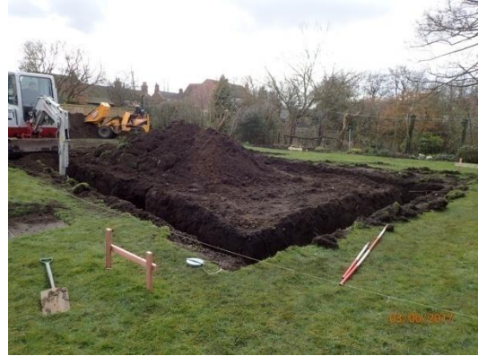
Plate 16: Excavation of the foundations, from the north-east
