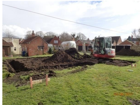
Plate 11: Excavation of the foundations, from the north-west
