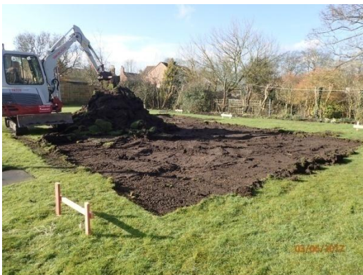
Plate 3: Initial ground reduction, from the north-east
