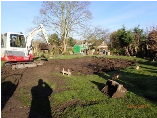
Plate 20: Internal ground reduction, from the south-east
