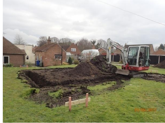
Plate 10: Excavation of the foundations, from the north-west
