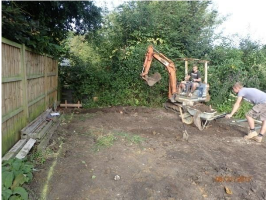
Plate 26: Excavation of the foundations, from the east
