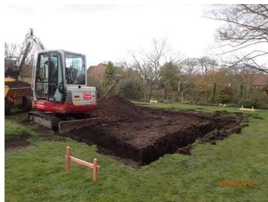
Plate 12: Excavation of the foundations, from the north-east
