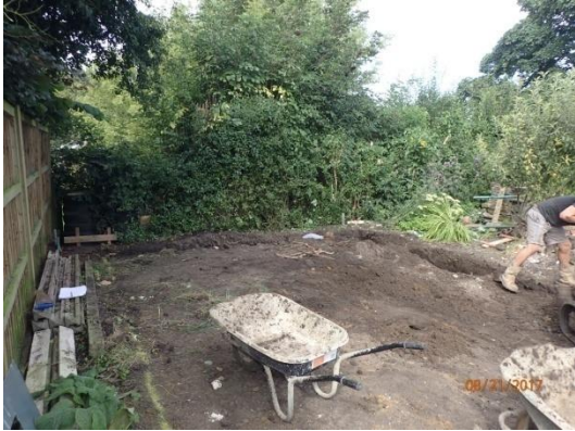
Plate 31: Excavation of the foundations, from the east
