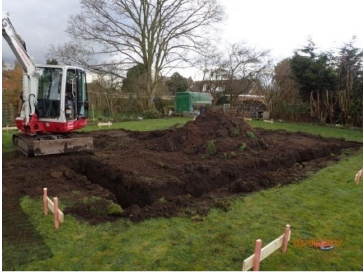
Plate 19: Excavation of the foundations, from the south-east
