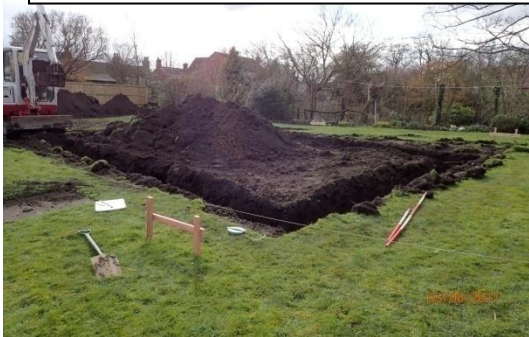
Plate 15: Excavation of the foundations, from the north-east
