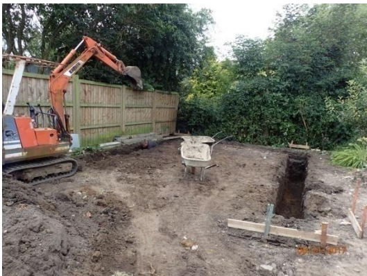
Plate 39: Excavation of the foundations, from the east
