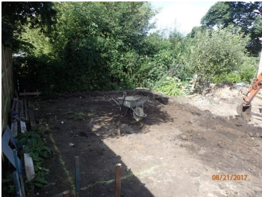
Plate 33: Excavation of the foundations, from the east
