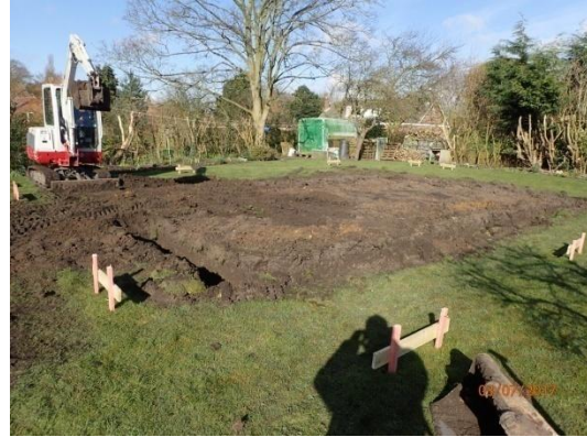
Plate 22: Excavation of the foundations, from the south-east
