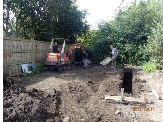
Plate 34: Excavation of the foundations, from the east
