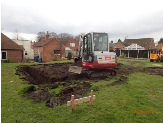
Plate 9: Excavation of the foundations, from the north-west
