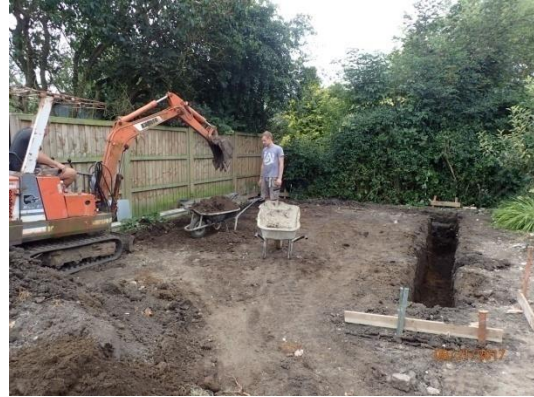
Plate 40: Excavation of the foundations, from the east
