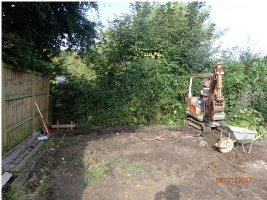
Plate 27: Excavation of the foundations, from the east
