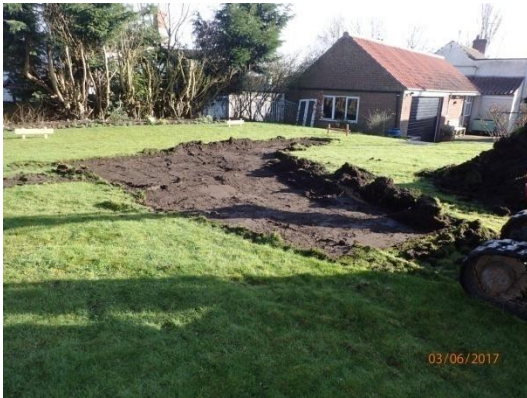
Plate 2: Initial ground reduction, from the north-east
