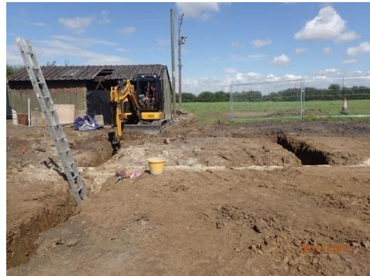
Plate 107: Excavation of the foundations, from the south
