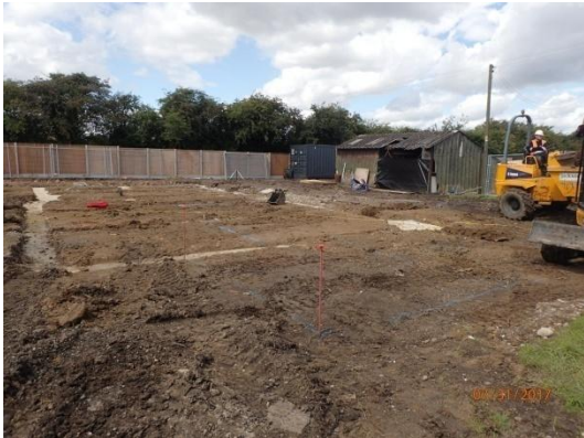
Plate 92: Excavation of the foundations, from the east
