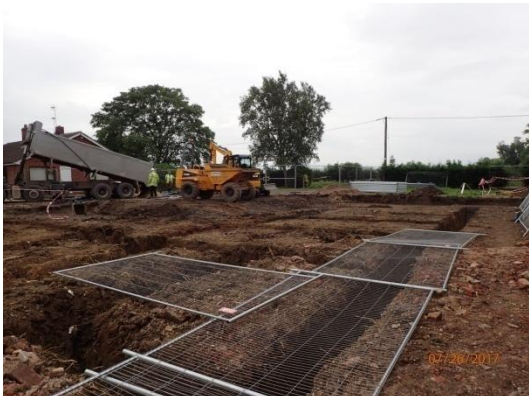
Plate 81: Excavation of the foundations, from the north
