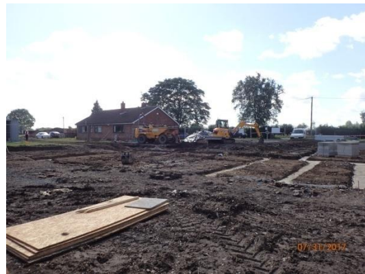
Plate 90: Excavation of the foundations, from the north
