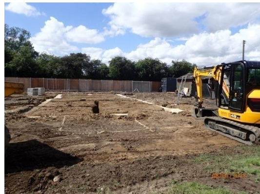
Plate 108: Excavation of the foundations, from the east
