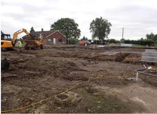
Plate 61: Excavation of the foundations, from the north
