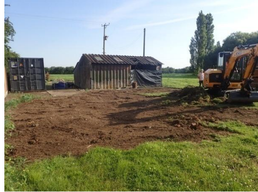
Plate 4: Initial ground reduction, from the south
