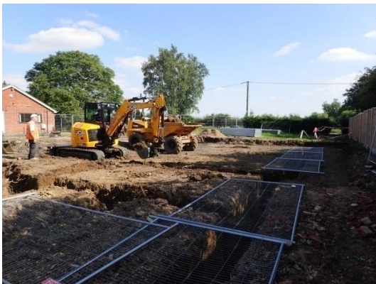
Plate 75: Excavation of the foundations, from the north
