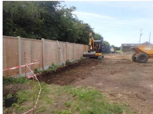
Plate 29: Further ground reduction, from the south
