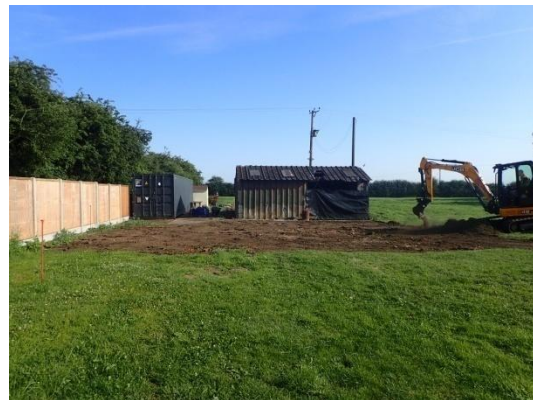
Plate 5: Initial ground reduction, from the south
