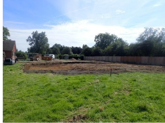
Plate 28: Further ground reduction, from the north
