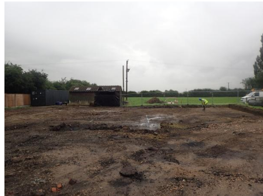
Plate 35: Set out foundations of the new house plot, from the south
