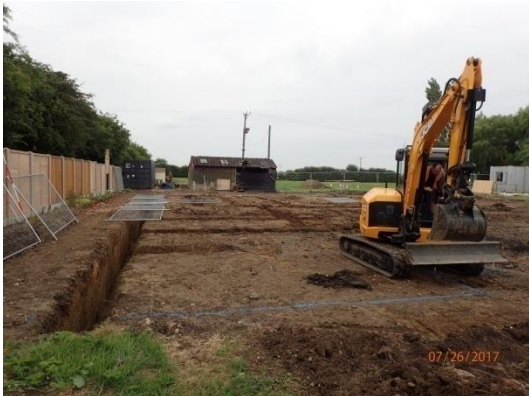
Plate 80: Excavation of the foundations, from the south
