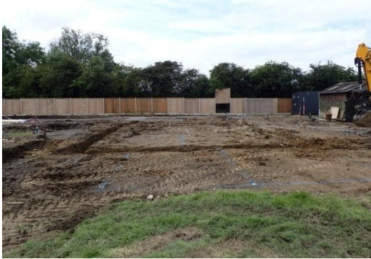
Plate 73: Excavation of the foundations, from the east
