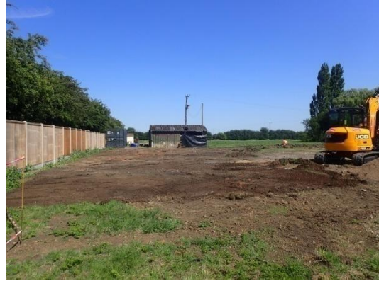
Plate 10: Initial ground reduction, from the south
