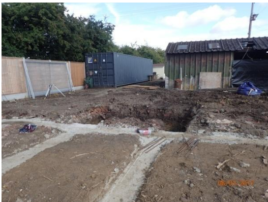
Plate 105: Excavation of the foundations, from the south
