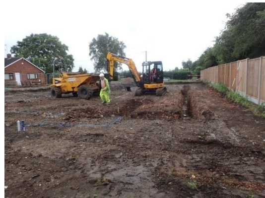
Plate 48: Excavation of the foundations, from the north
