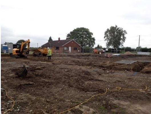
Plate 62: Excavation of the foundations, from the north
