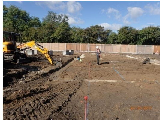
Plate 89: Excavation of the foundations, from the east
