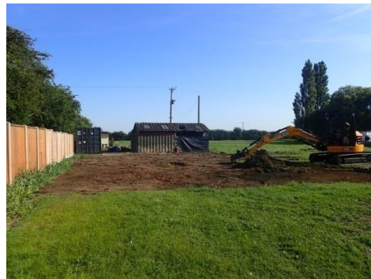
Plate 6: Initial ground reduction, from the south
