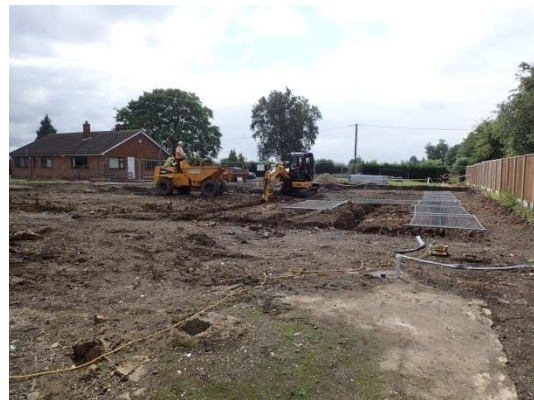
Plate 66: Excavation of the foundations, from the north
