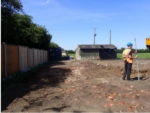
Plate 13: Further ground reduction, from the south
