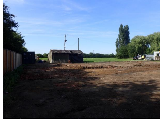
Plate 16: Further ground reduction, from the south
