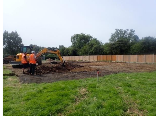
Plate 22: Further ground reduction, from the north
