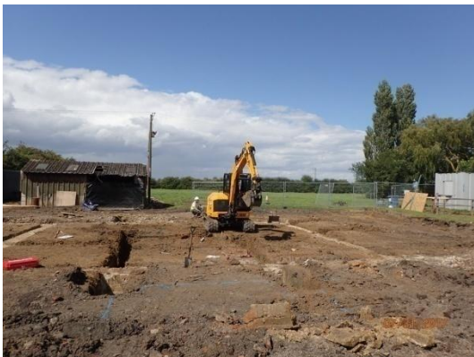
Plate 99: Excavation of the foundations, from the south
