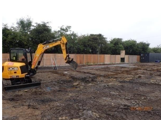
Plate 84: Excavation of the foundations, from the south-east
