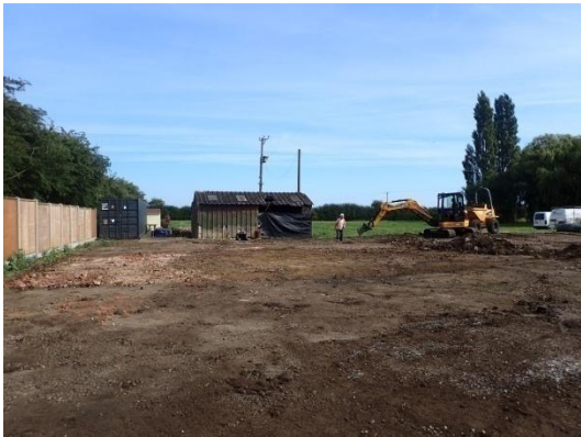
Plate 20: Further ground reduction, from the south
