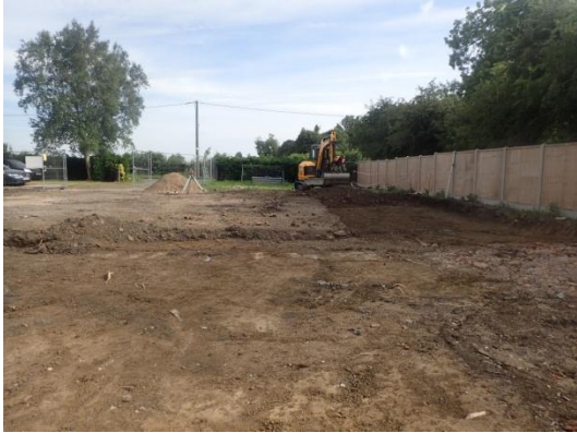
Plate 31: Further ground reduction, from the north
