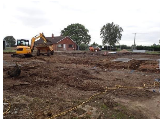
Plate 59: Excavation of the foundations, from the north
