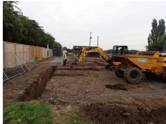
Plate 77: Excavation of the foundations, from the south
