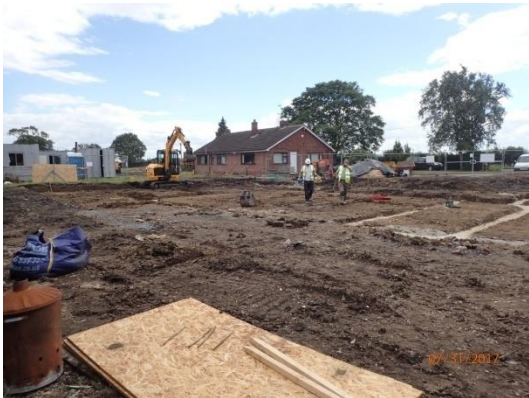
Plate 93: Excavation of the foundations, from the north-west
