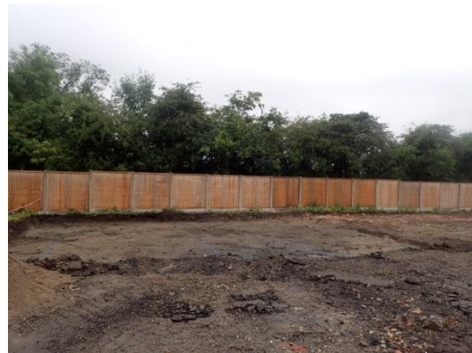
Plate 36: Set out foundations, of the new integral garage, from the east
