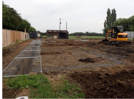
Plate 76: Excavated foundation trenches, from the south
