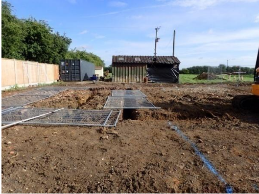
Plate 55: Excavated foundations, from the south
