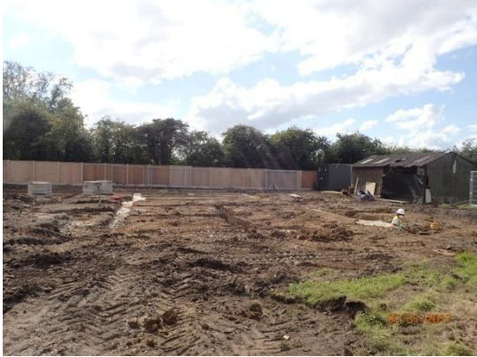
Plate 103: Excavation of the foundations, from the east
