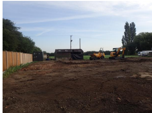
Plate 17: Further ground reduction, from the south
