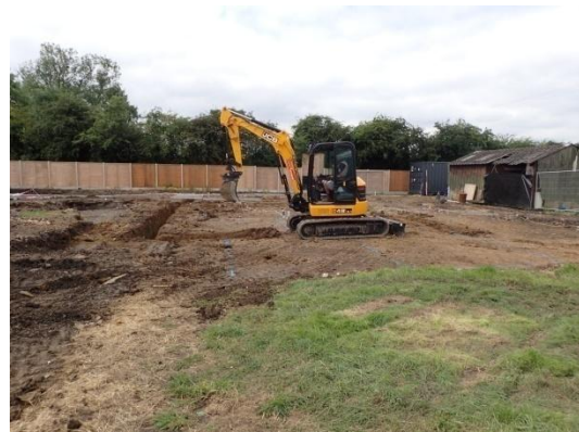
Plate 72: Excavation of the foundations, from the east
