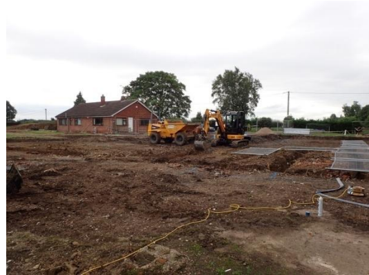
Plate 65: Excavation of the foundations, from the north
