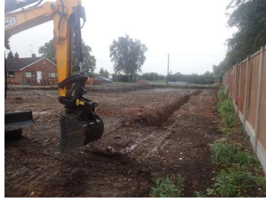
Plate 46: Excavation of the foundations, from the north
