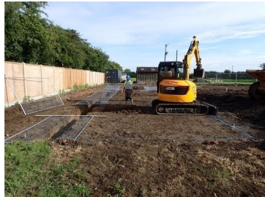
Plate 54: Excavated foundations, from the south
