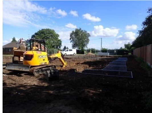
Plate 53: Excavation of the foundations, from the north
