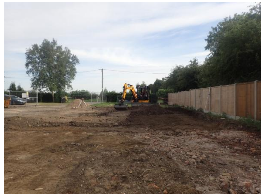
Plate 30: Further ground reduction, from the north
