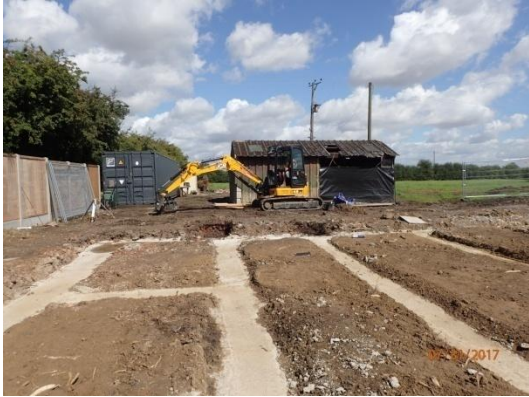
Plate 91: Excavation of the foundations, from the south
