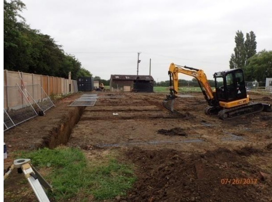
Plate 82: Excavation of the foundations, from the south
