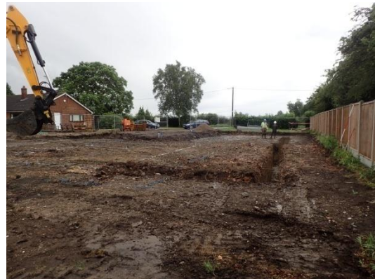
Plate 47: Excavation of the foundations, from the north
