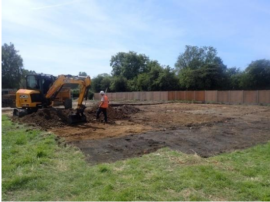
Plate 25: Further ground reduction, from the north
