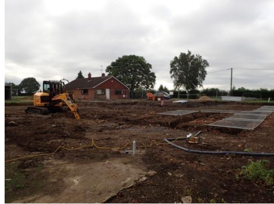
Plate 58: Excavation of the foundations, from the north
