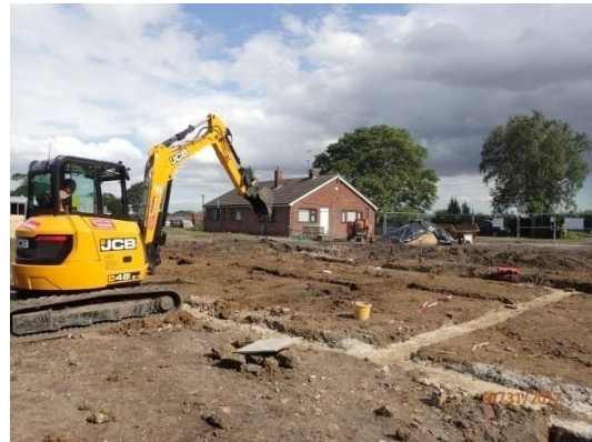
Plate 101: Excavation of the foundations, from the north-west
