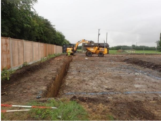
Plate 43: Excavation of the foundations, from the south
