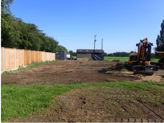
Plate 7: Initial ground reduction, from the south
