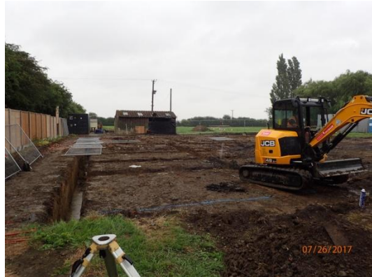
Plate 83: Excavation of the foundations, from the north
