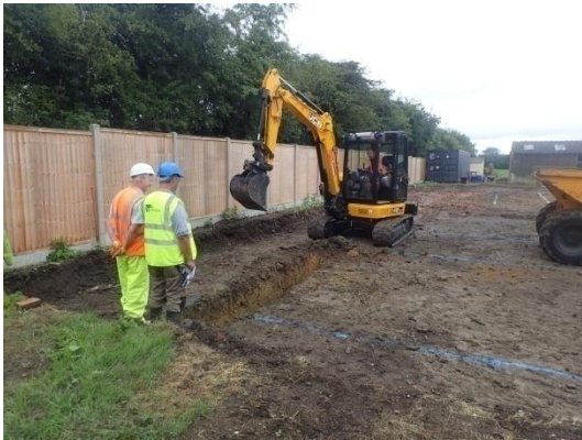
Plate 38: Excavation of the foundations, from the south
