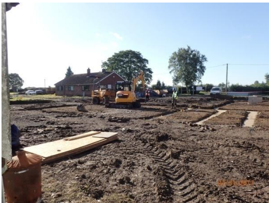
Plate 87: Excavation of the foundations, from the north
