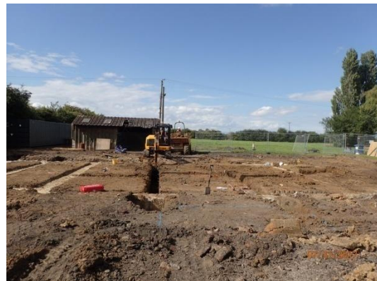
Plate 102: Excavation of the foundations, from the south
