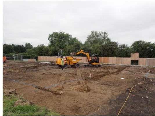
Plate 64: Excavation of the foundations, from the east
