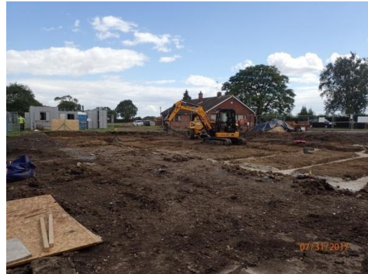
Plate 95: Excavation of the foundations, from the north-west
