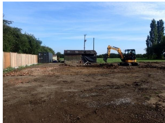
Plate 18: Further ground reduction, from the south
