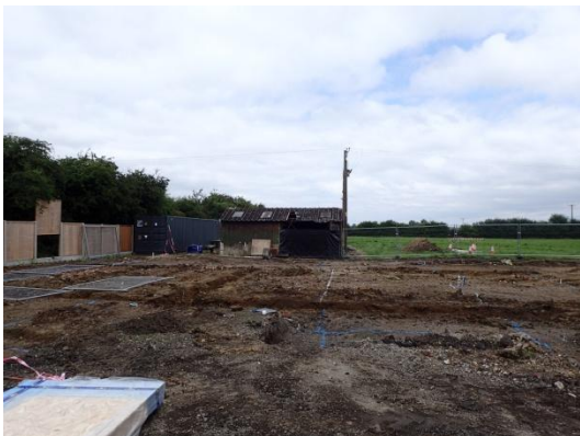
Plate 69: Excavation of the foundations, from the south
