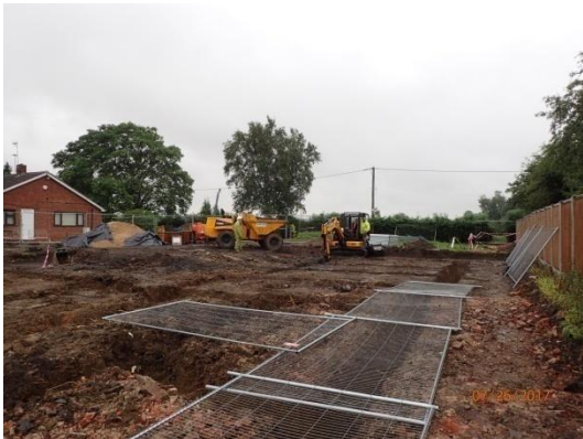
Plate 86: Excavation of the foundations, from the north
