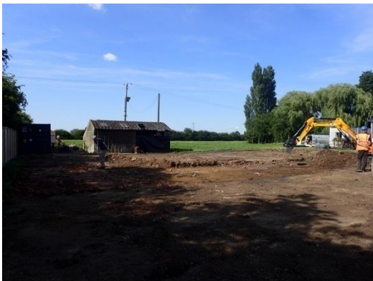
Plate 15: Further ground reduction, from the south
