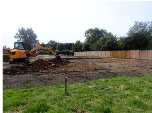
Plate 23: Further ground reduction, from the north
