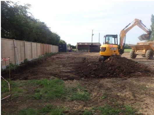
Plate 32: Further ground reduction, from the south
