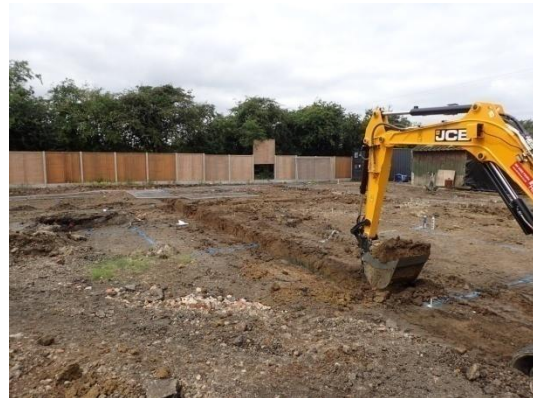
Plate 71: Excavation of the foundations, from the south-east
