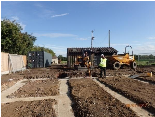
Plate 104: Excavation of the foundations, from the south
