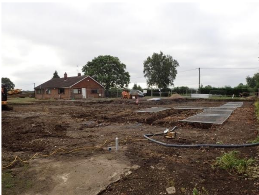
Plate 57: Excavation of the foundations, from the north
