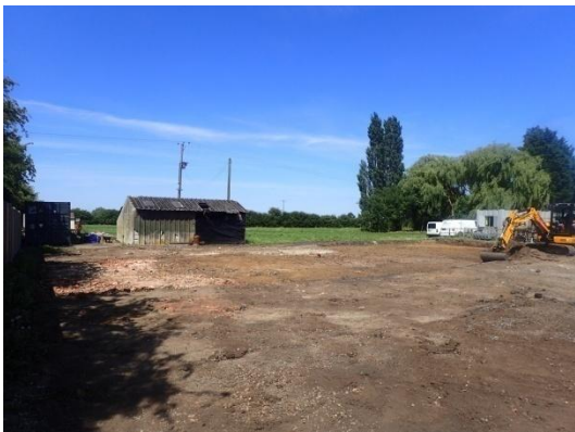
Plate 27: Further ground reduction, from the south
