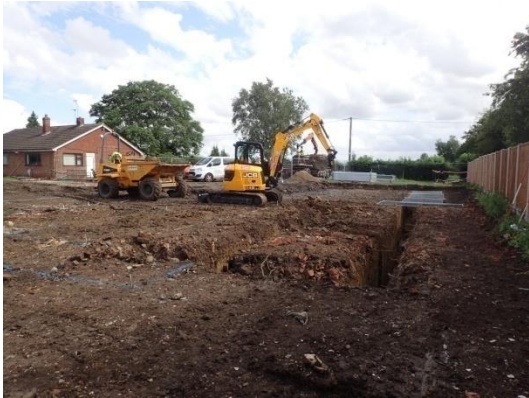
Plate 50: Excavation of the foundations, from the north
