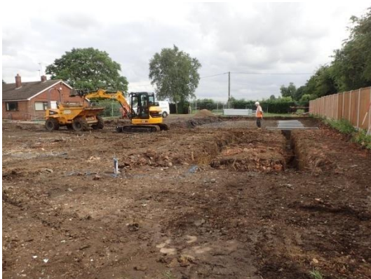
Plate 51: Excavation of the foundations, from the north
