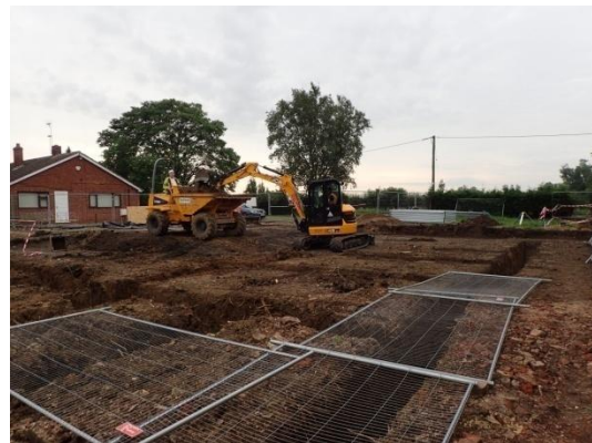
Plate 78: Excavation of the foundations, from the north
