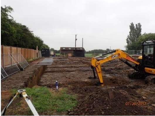
Plate 85: Excavation of the foundations, from the south
