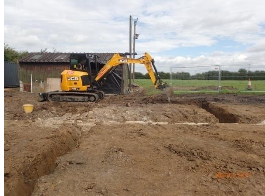
Plate 106: Excavation of the foundations, from the south
