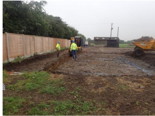
Plate 40: Excavation of the foundations, from the south
