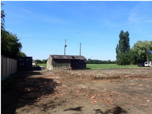
Plate 14: Further ground reduction, from the south
