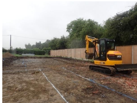
Plate 42: Excavation of the foundations, from the north
