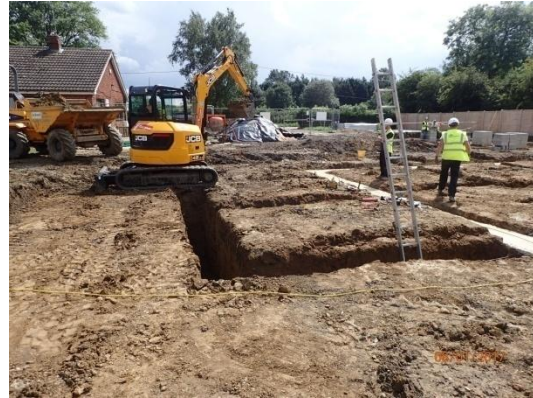
Plate 113: Excavation of the foundations, from the north
