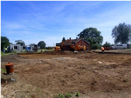
Plate 26: Further ground reduction, from the south
