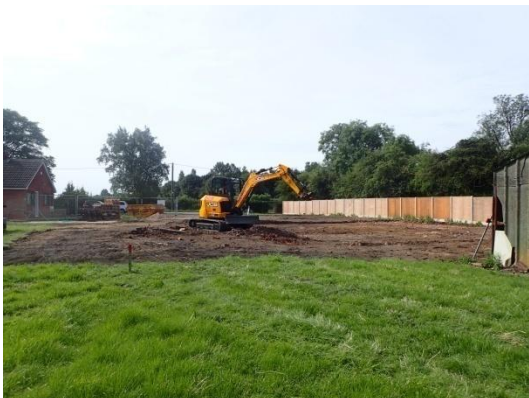
Plate 21: Further ground reduction, from the north
