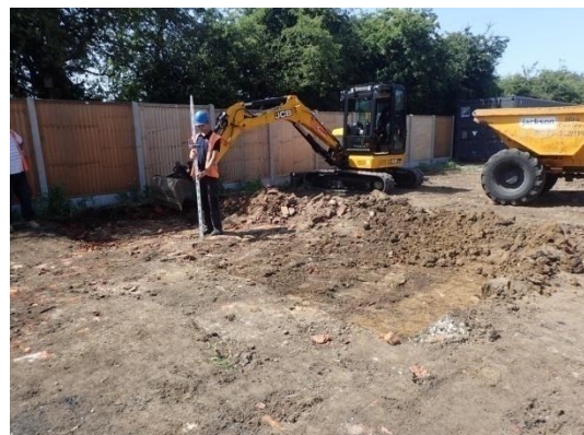
Plate 12: Further ground reduction, from the south
