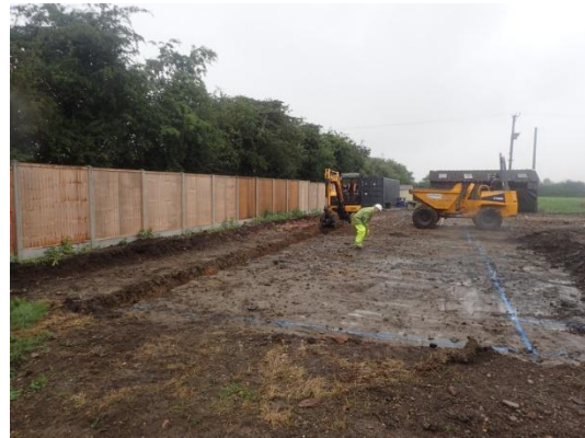
Plate 41: Excavation of the foundations, from the south
