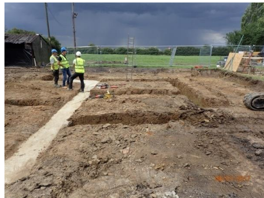
Plate 114: Excavation of the foundations, from the south
