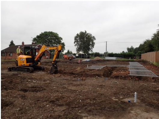
Plate 56: Excavation of the foundations, from the north
