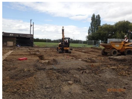
Plate 96: Excavation of the foundations, from the south
