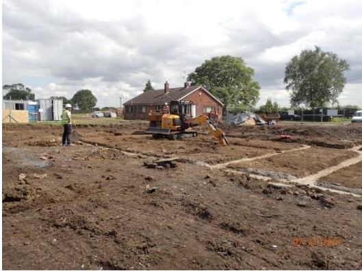
Plate 97: Excavation of the foundations, from the north-west
