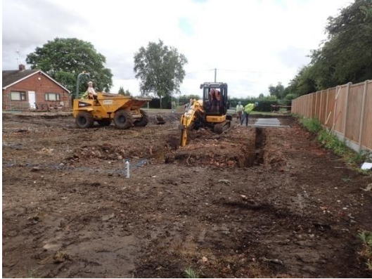
Plate 49: Excavation of the foundations, from the north
