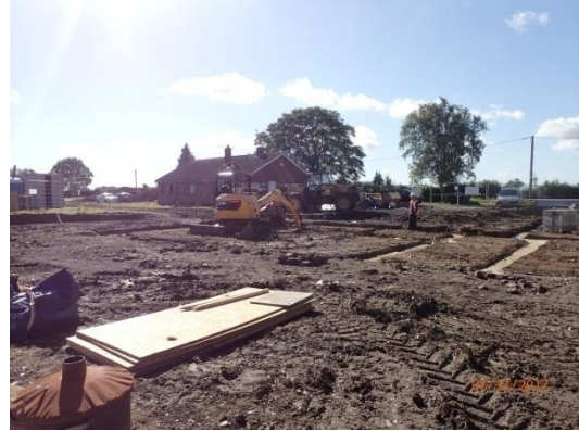
Plate 88: Excavation of the foundations, from the north
