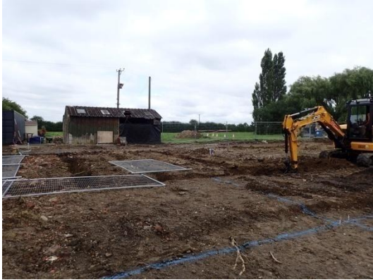
Plate 67: Excavation of the foundations, from the south
