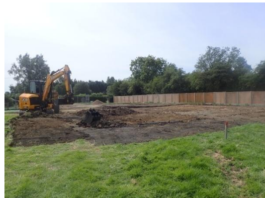
Plate 24: Further ground reduction, from the north
