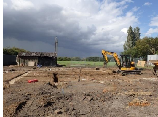
Plate 100: Excavation of the foundations, from the south
