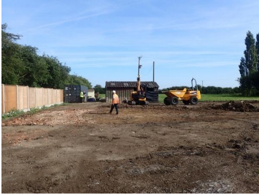
Plate 19: Further ground reduction, from the south
