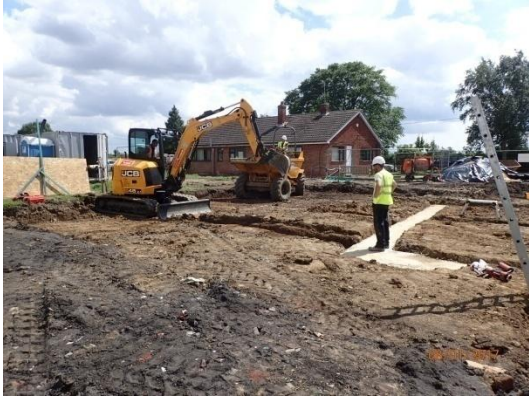
Plate 109: Excavation of the foundations, from the north-west
