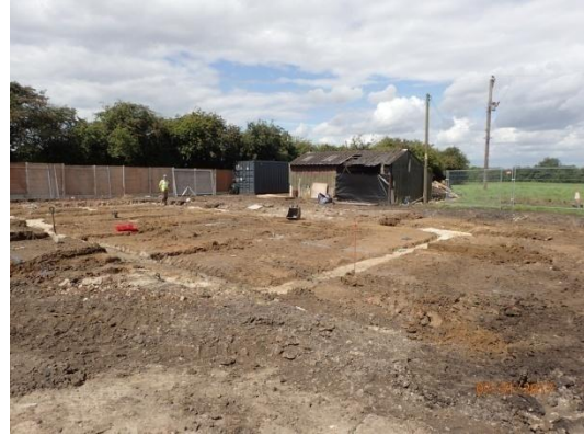
Plate 94: Excavation of the foundations, from the south-east
