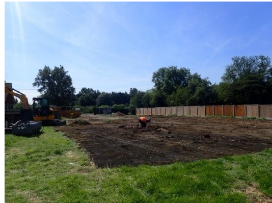
Plate 11: Initial ground reduction, from the north
