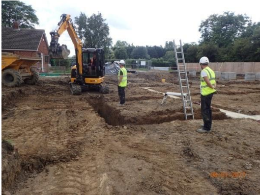
Plate 110: Excavation of the foundations, from the north
