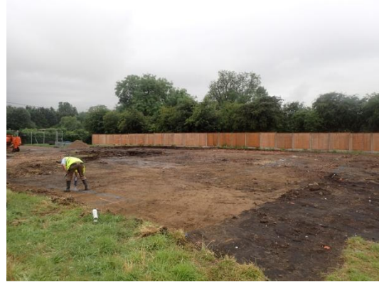
Plate 34: Set out foundations, of the new house plot, from the north-east
