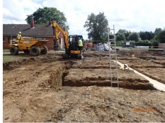
Plate 112: Excavation of the foundations, from the north
