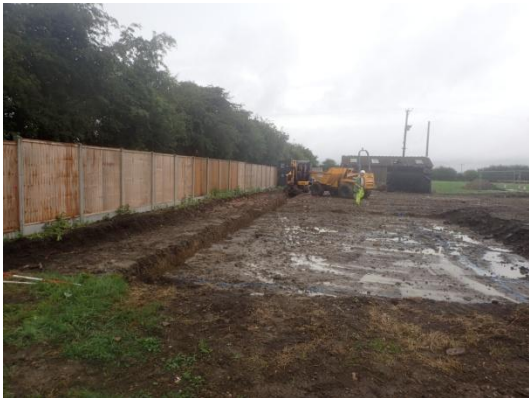
Plate 44: Excavation of the foundations, from the south
