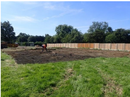
Plate 9: Initial ground reduction, from the north
