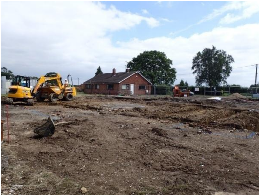
Plate 74: Excavation of the foundations, from the north
