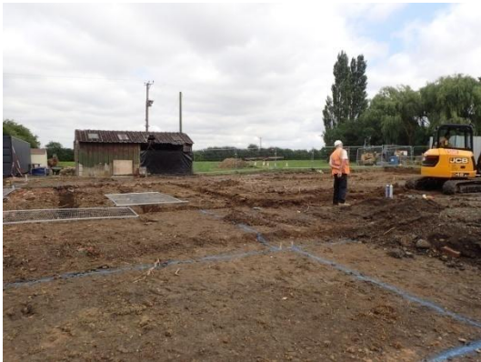
Plate 68: Excavation of the foundations, from the south
