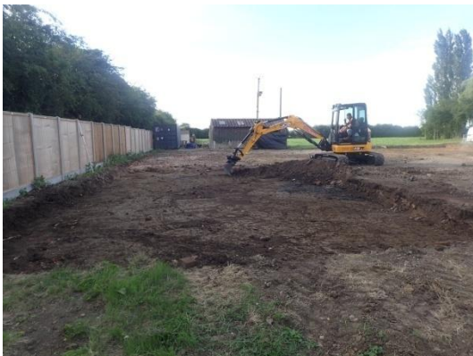
Plate 33: Further ground reduction, from the south
