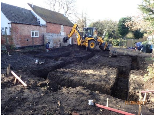
Plate 25: Excavation of the foundations, from the east
