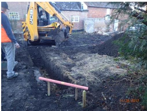
Plate 3: Excavation of the foundations, from the north
