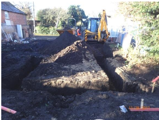
Plate 9: Excavation of the foundations, from the east
