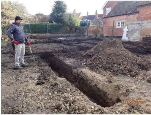
Plate 31: Excavation of the foundations, from the west
