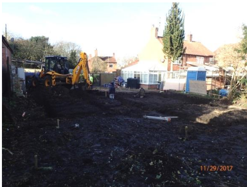
Plate 27: Excavation of the foundations, from the east
