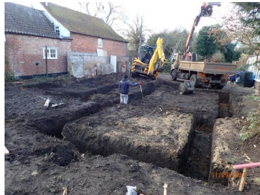
Plate 23: Excavation of the foundations, from the east
