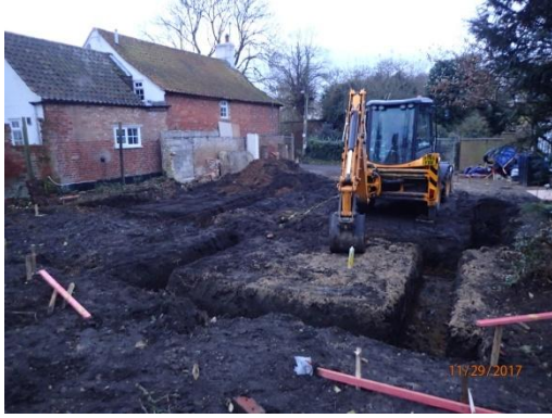
Plate 19: Excavation of the foundations, from the east
