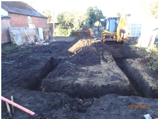
Plate 8: Excavation of the foundations, from the east
