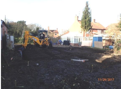
Plate 26: Excavation of the foundations, from the east
