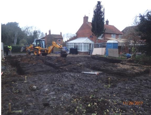
Plate 20: Excavation of the foundations, from the east
