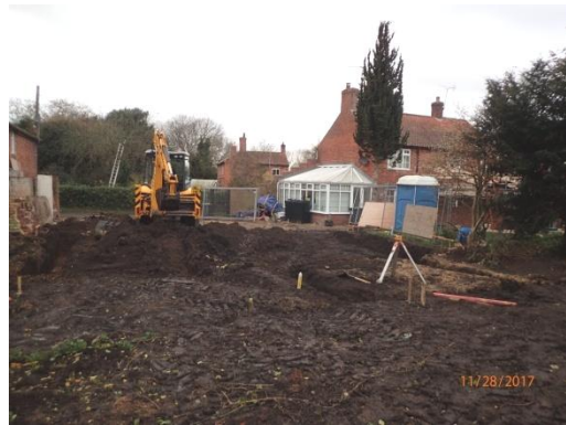
Plate 17: Excavation of the foundations, from the east
