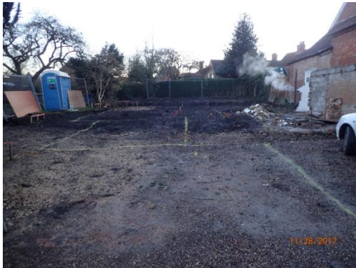
Plate 1: Pre-groundworks, from the west
