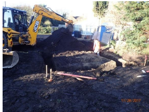
Plate 11: Excavation of the foundations, from the east
