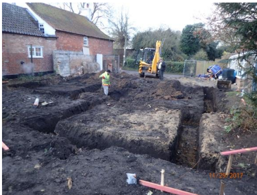
Plate 21: Excavation of the foundations, from the east
