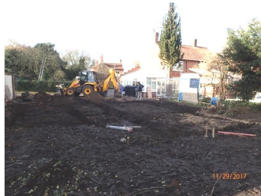
Plate 30: Excavation of the foundations, from the east
