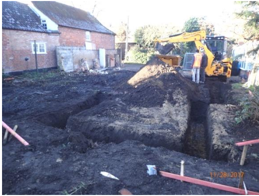
Plate 7: Excavation of the foundations, from the east
