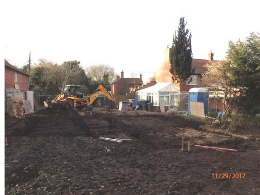
Plate 35: Excavation of the foundations, from the east
