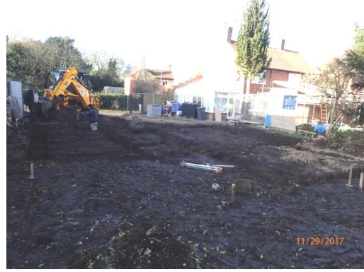
Plate 28: Excavation of the foundations, from the east
