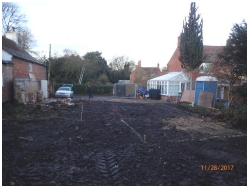
Plate 2: Pre-groundworks, from the east
