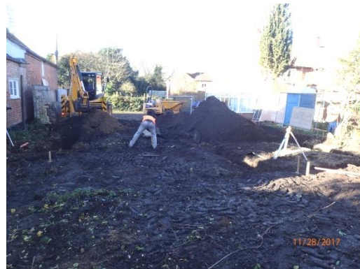
Plate 12: Excavation of the foundations, from the east
