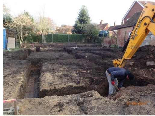
Plate 34: Excavation of the foundations, from the west
