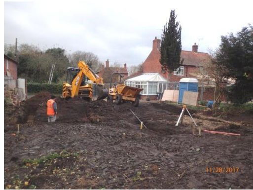
Plate 18: Excavation of the foundations, from the east
