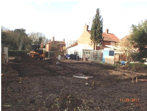
Plate 32: Excavation of the foundations, from the east
