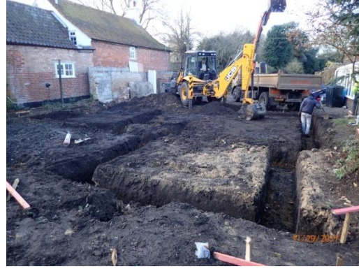
Plate 22: Excavation of the foundations, from the east
