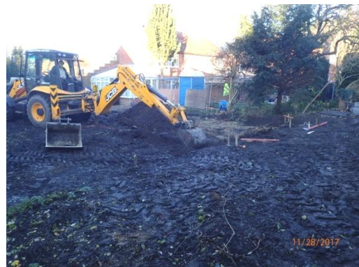
Plate 5: Excavation of the foundations, from the east
