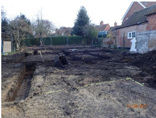
Plate 33: Excavation of the foundations, from the west
