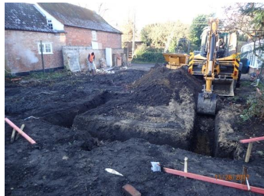
Plate 6: Excavation of the foundations, from the east
