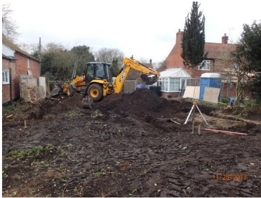
Plate 15: Excavation of the foundations, from the east
