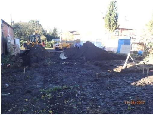
Plate 13: Excavation of the foundations, from the east
