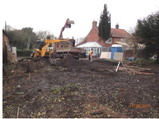
Plate 16: Excavation of the foundations, from the east
