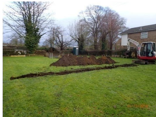
Plate 6: Excavation of the house foundations, from the south
