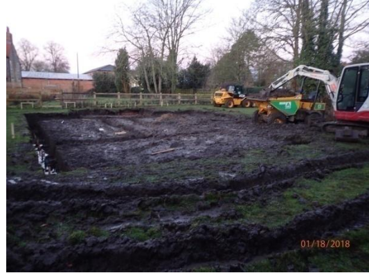
Plate 40: Excavation of the house foundations, from the east
