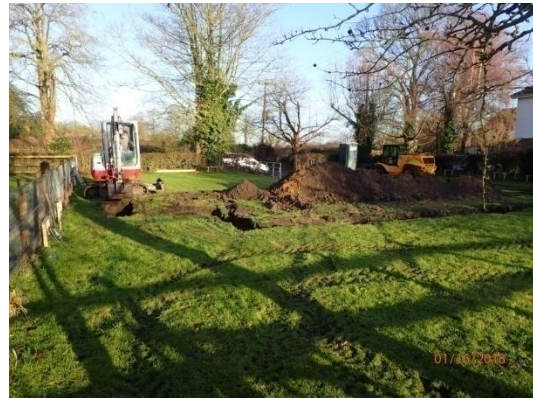
Plate 11: Excavation of the house foundations, from the south
