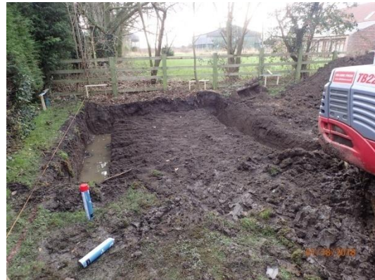
Plate 47: Excavation of the garage foundations, from the north
