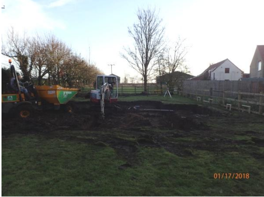
Plate 37: Excavation of the house foundations, from the north
