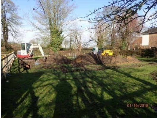
Plate 13: Excavation of the house foundations, from the south
