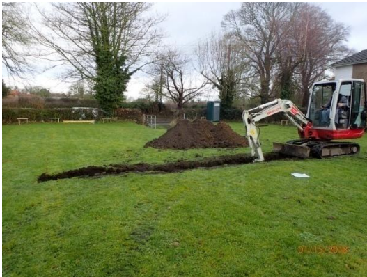
Plate 3: Excavation of the house foundations, from the south
