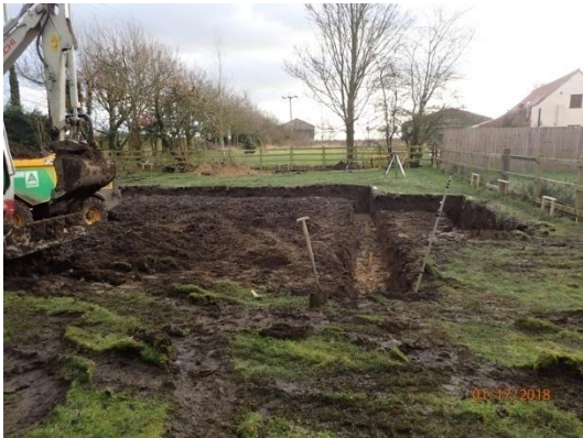
Plate 32: Excavation of the house foundations, from the north
