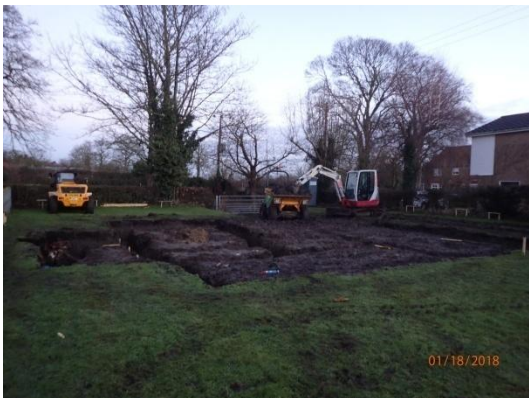
Plate 39: Excavation of the house foundations, from the south
