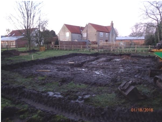
Plate 38: Excavation of the house foundations, from the south
