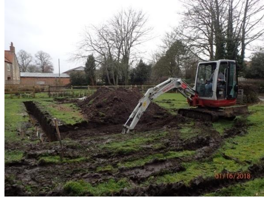
Plate 16: Excavation of the house foundations, from the east
