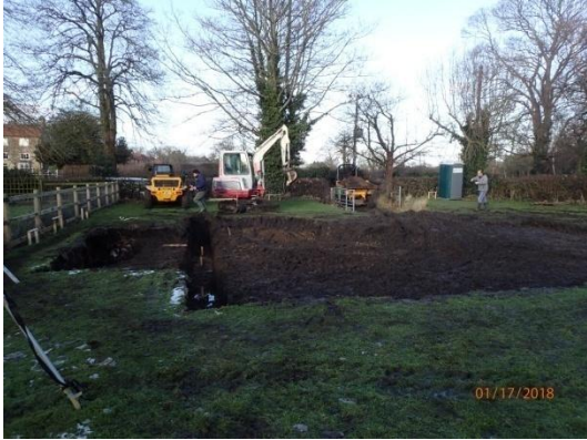
Plate 31: Excavation of the house foundations, from the south
