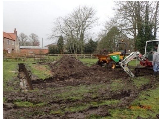
Plate 17: Excavation of the house foundations, from the east
