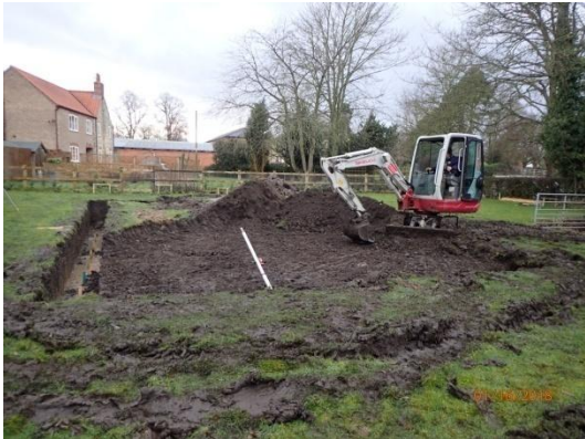
Plate 20: Excavation of the house foundations & internal ground reduction, from the east
