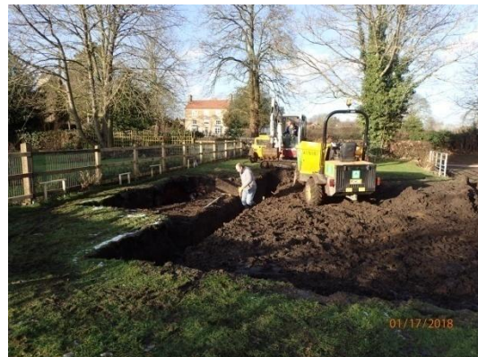
Plate 30: Excavation of the house foundations, from the south
