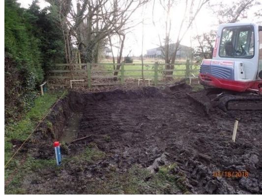
Plate 46: Internal ground reduction, garage, from the north
