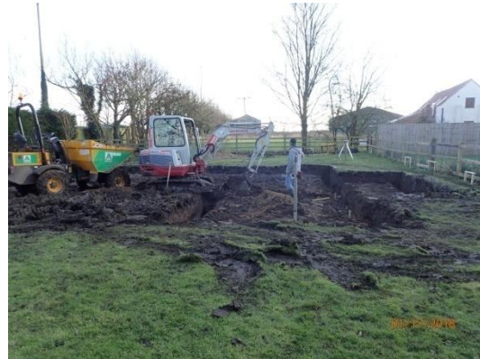
Plate 35: Excavation of the house foundations, from the north
