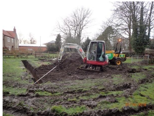
Plate 18: Excavation of the house foundations & internal ground reduction, from the east
