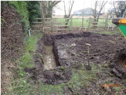
Plate 44: Internal ground reduction, garage, from the north
