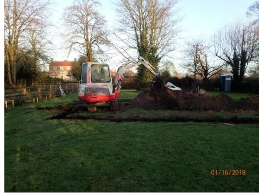
Plate 10: Excavation of the house foundations, from the south
