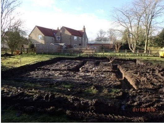
Plate 43: Excavation of the house foundations, from the south
