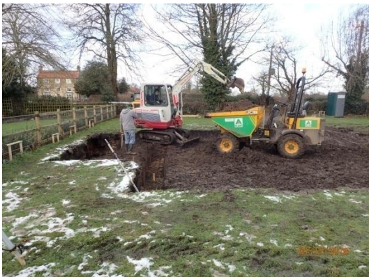
Plate 27: Excavation of the house foundations, from the south
