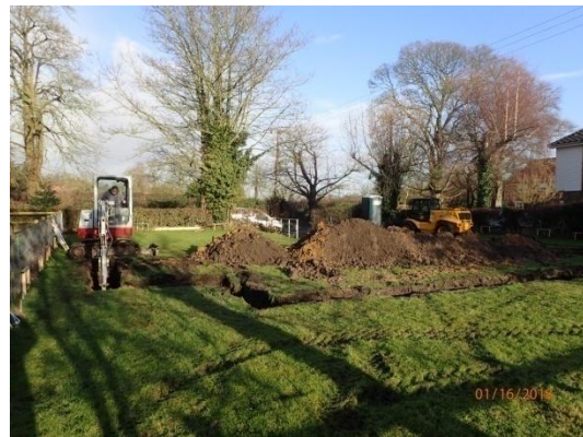
Plate 12: Excavation of the house foundations, from the south
