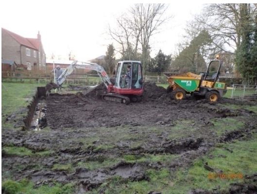
Plate 21: Excavation of the house foundations & internal ground reduction, from the east
