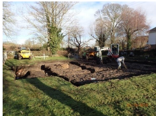
Plate 42: Excavation of the house foundations, from the south
