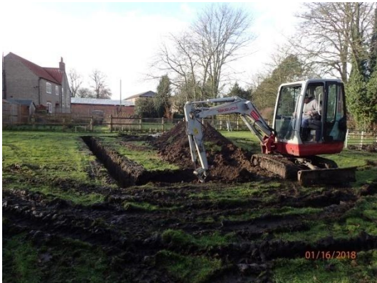
Plate 14: Excavation of the house foundations, from the east
