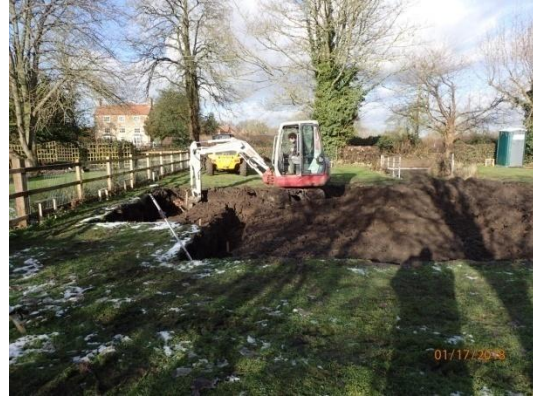
Plate 28: Excavation of the house foundations, from the south
