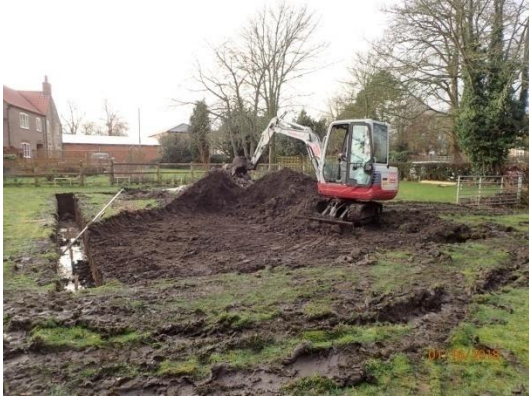
Plate 19: Excavation of the house foundations & internal ground reduction, from the east
