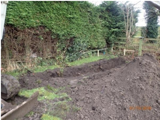
Plate 8: Excavation of the garage foundations, from the north-east
