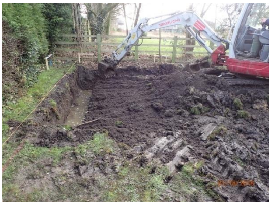
Plate 45: Internal ground reduction, garage, from the north
