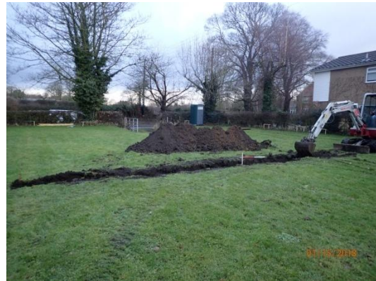
Plate 5: Excavation of the house foundations, from the south
