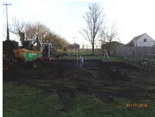
Plate 36: Excavation of the house foundations, from the north
