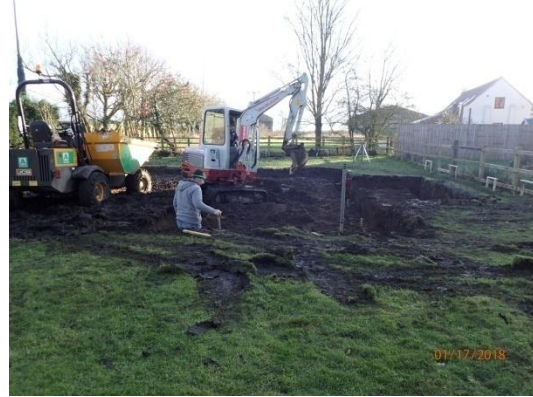
Plate 34: Excavation of the house foundations, from the north
