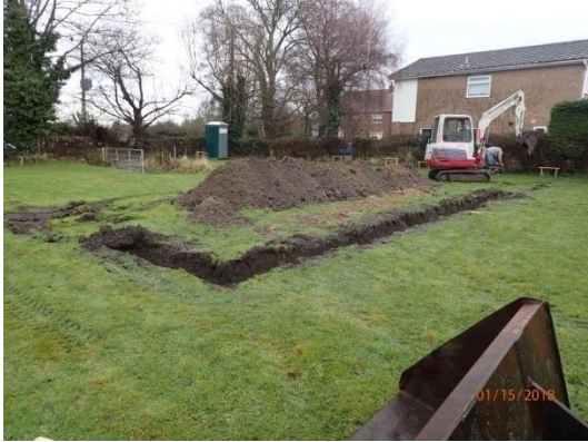
Plate 7: Excavation of the house foundations, from the south-west
