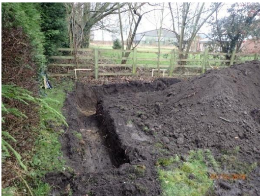
Plate 9: Excavation of the garage foundations, from the north
