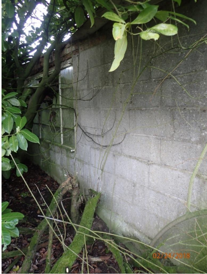
Plate 63: View of the East Elevation of Outbuilding 2, from the north
