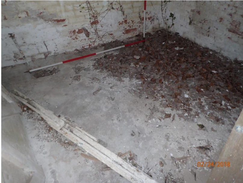
Plate 80: View of the floor of Cell 4, from the south-west
