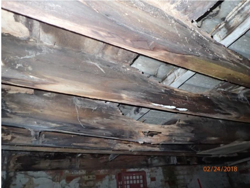
Plate 42: View of the ceiling of Cell 1, from the east
