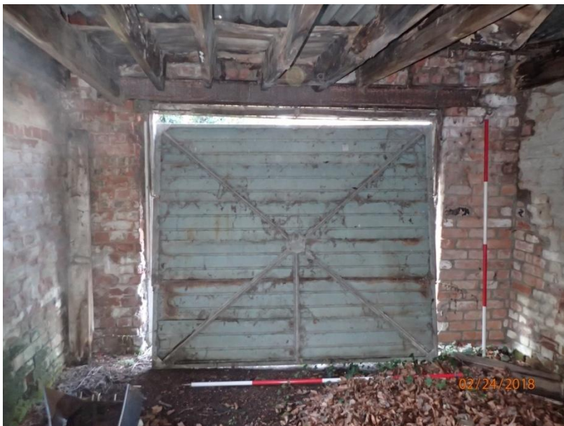
Plate 47: View of the south wall of Cell 1, from the north
