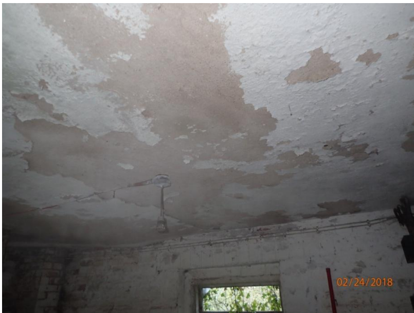
Plate 83: View of the ceiling of Cell 4, from the south
