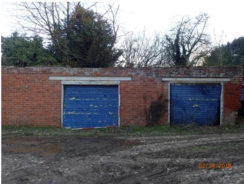
Plate 31: View of the South Elevation of Outbuilding 1, from the south
