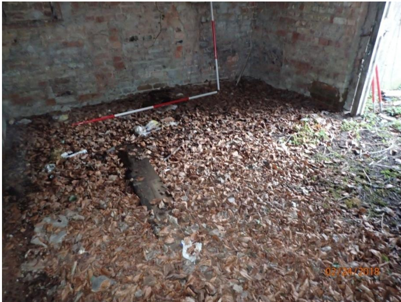
Plate 38: View of the floor of Cell 1, from the south
