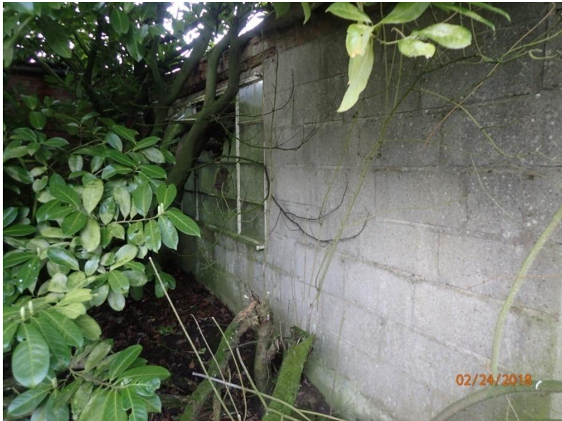
Plate 64: View of the East Elevation of Outbuilding 2, from the north
