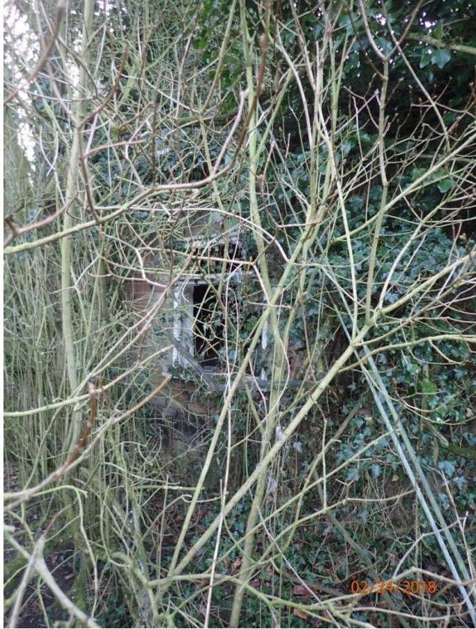
Plate 73: View of part of the North Elevation of Outbuilding 3, from the north
