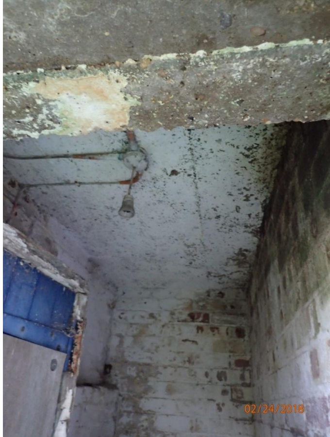
Plate 92: View of the interior of Cell 5, from the south
