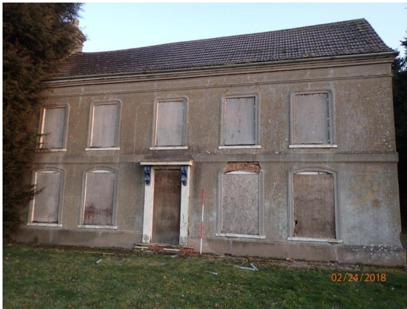
Plate 5: View of the South Elevation of the Farmhouse, from the south
