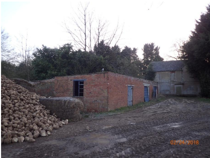
Plate 4: General view of the farmstead, from the west
