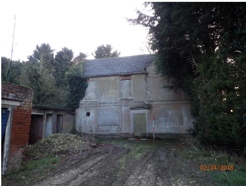
Plate 25: View of the West Elevation of the Farmhouse, from the west
