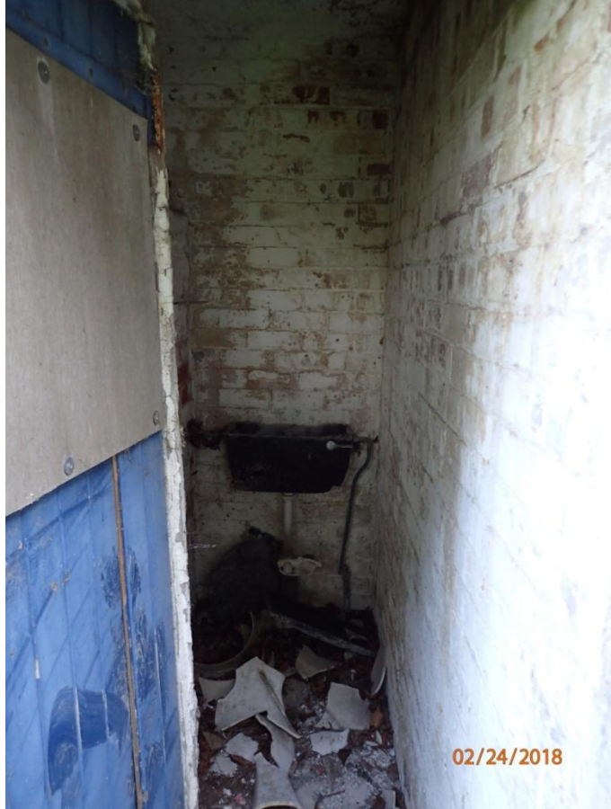
Plate 90: View of the interior of Cell 5, from the south
