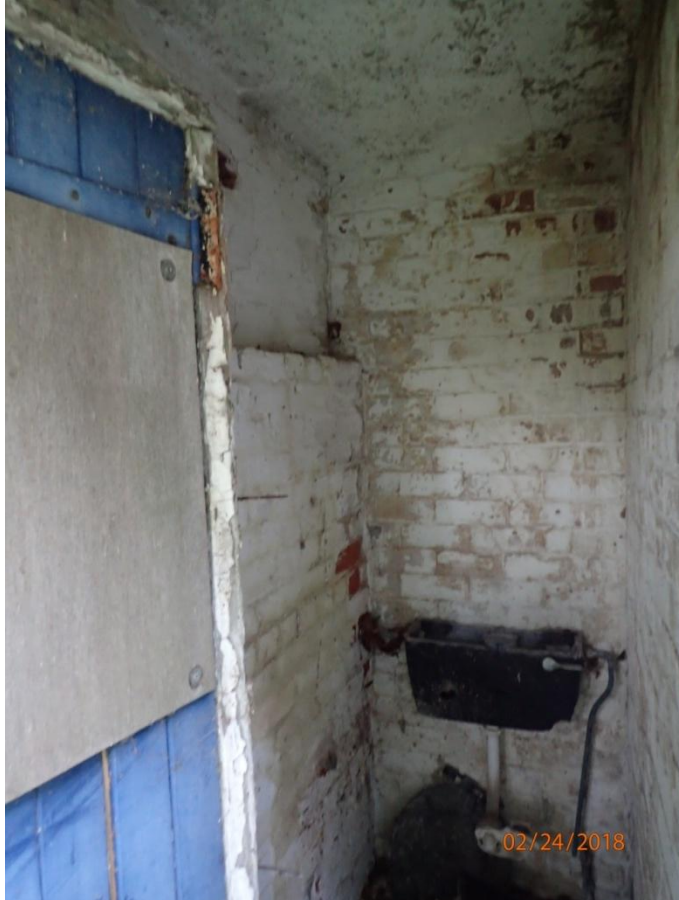
Plate 91: View of the interior of Cell 5, from the south
