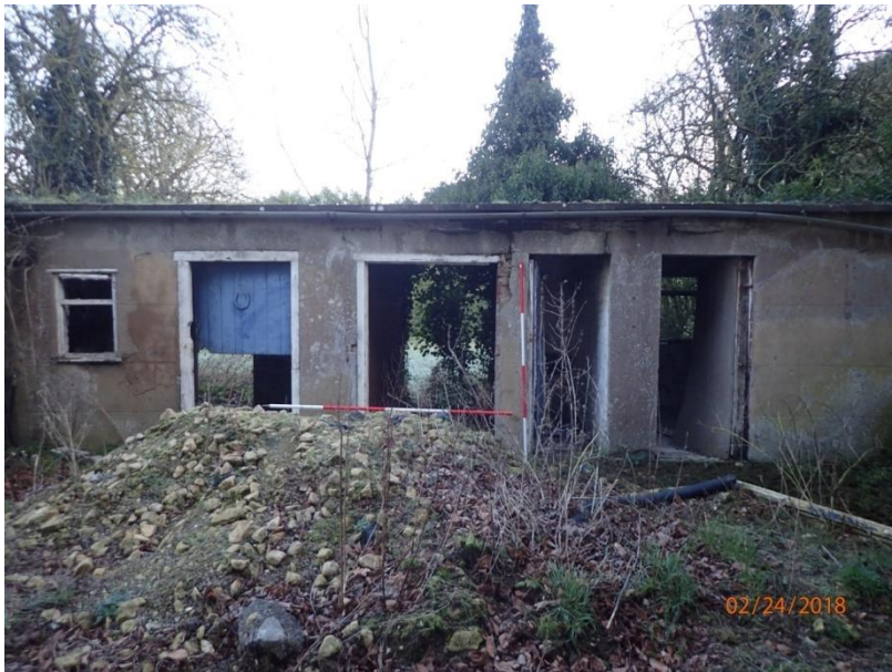
Plate 76: View of the South Elevation of Outbuilding 3, from the south
