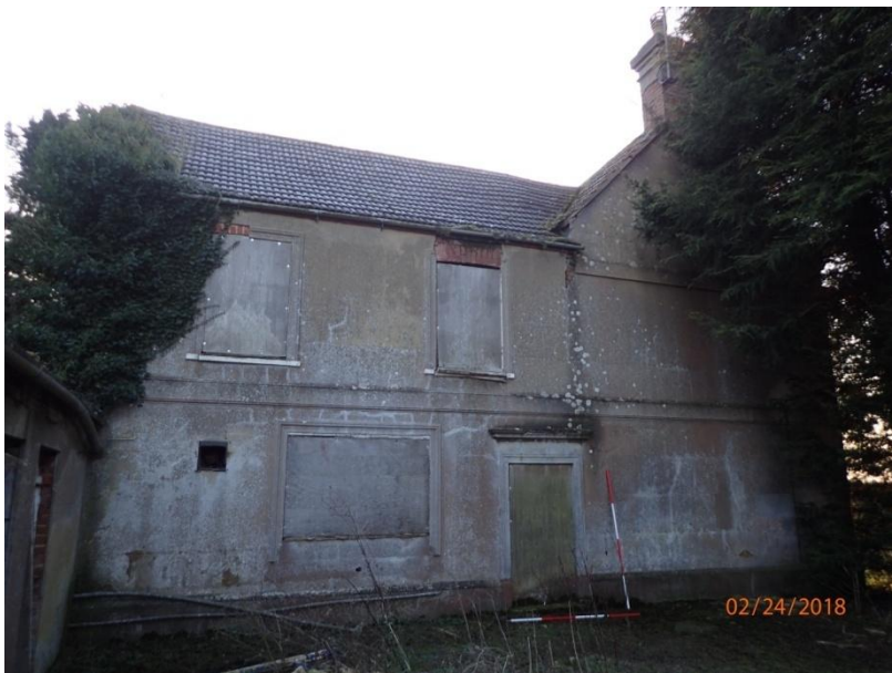
Plate 27: View of the West Elevation of the Farmhouse, from the west
