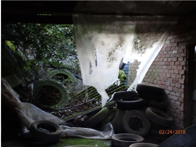
Plate 58: View of the interior of Cell 2, from the west
