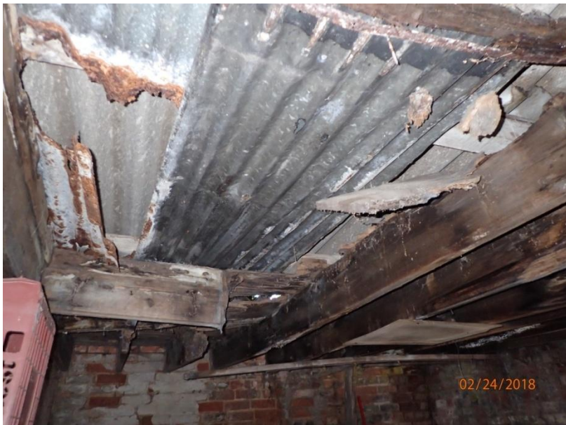
Plate 39: View of the ceiling of Cell 1, from the south
