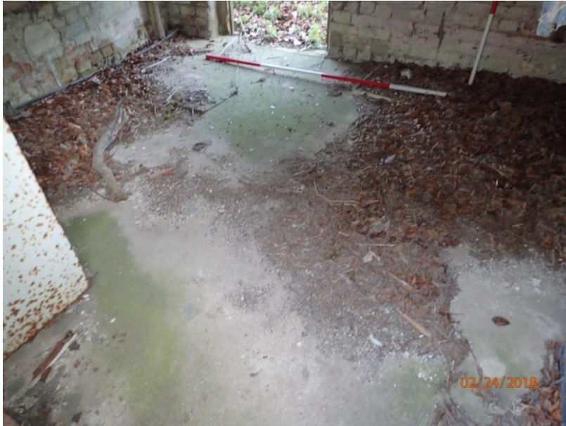
Plate 100: View of the floor of Cell 7, from the south
