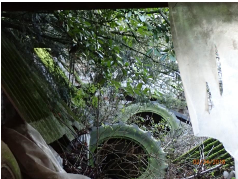
Plate 60: View of the interior of Cell 2, from the west
