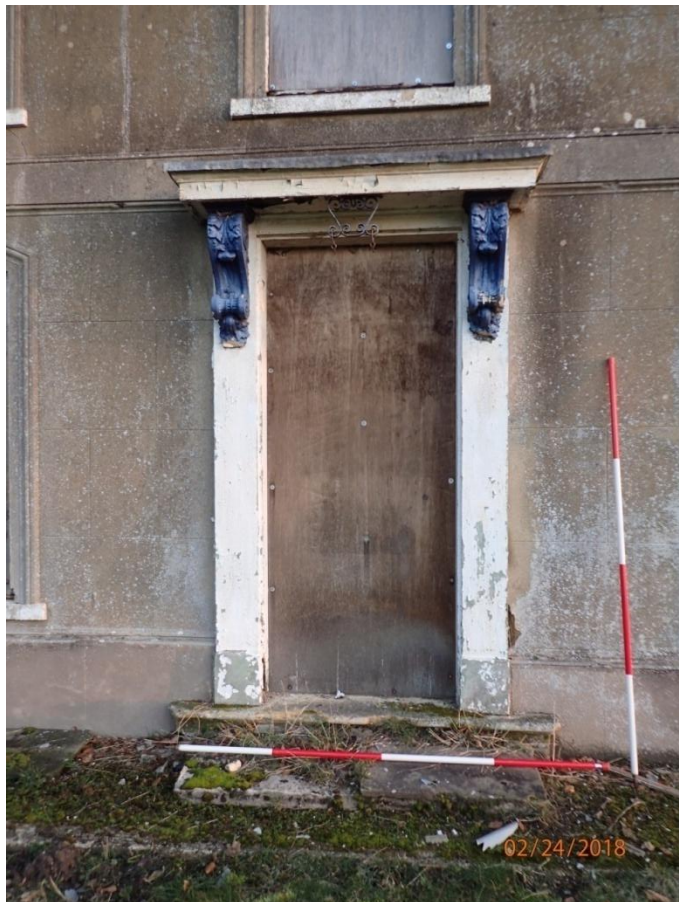
Plate 6: Detail: View of the south facing entrance to the Farmhouse, from the south
