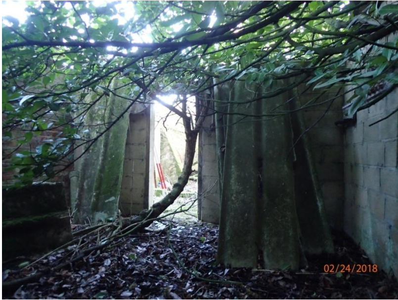
Plate 69: View of the north wall of Cell 2, from the south
