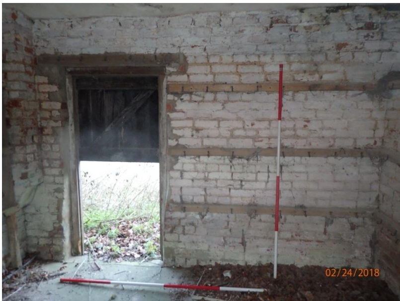
Plate 99: View of the north wall of Cell 7, from the south
