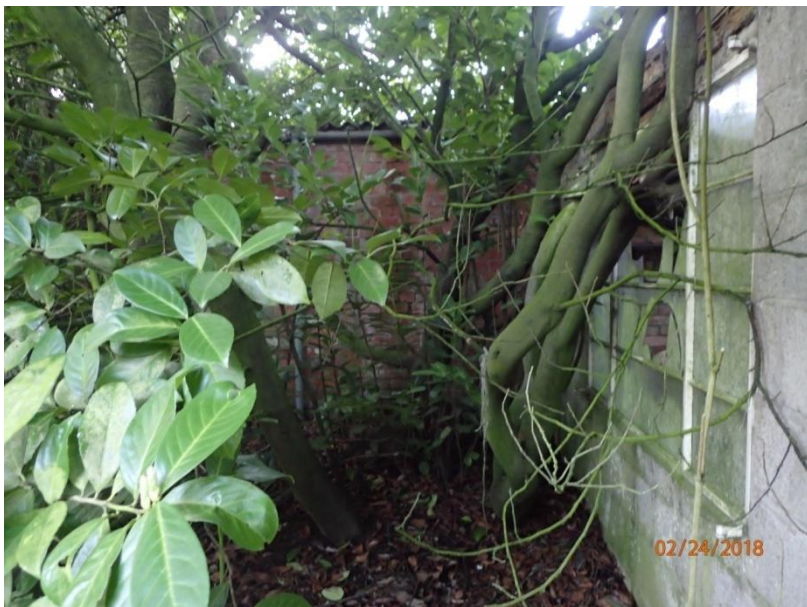
Plate 37: View of the North Elevation of Outbuilding 1, from the north
