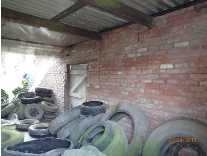
Plate 50: View of the south wall of Cell 2, from the west
