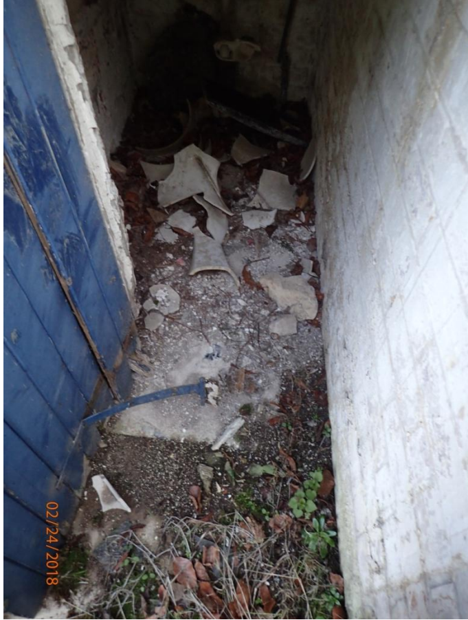
Plate 93: View of the floor of Cell 5, from the south
