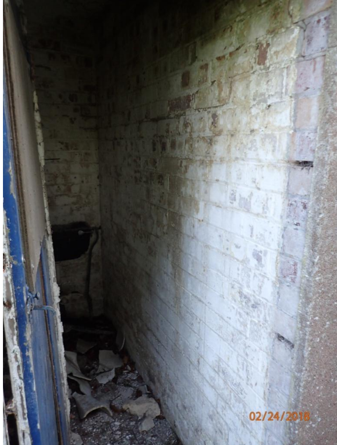
Plate 89: View of the east wall of Cell 5, from the south
