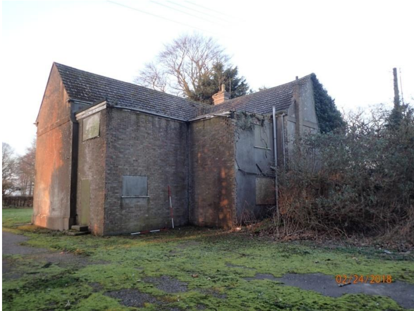
Plate 13: General View of the rear of the Farmhouse, from the north
