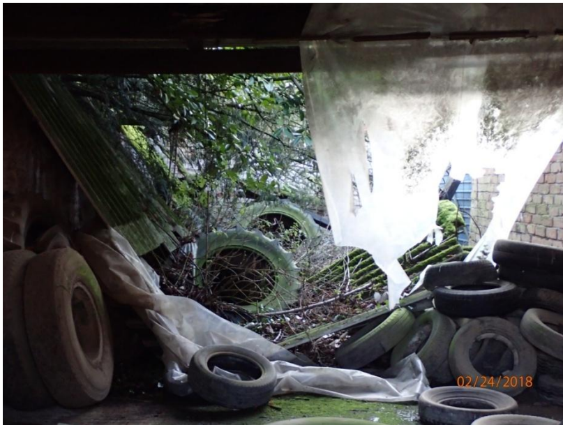
Plate 56: View of the interior of Cell 2, from the west
