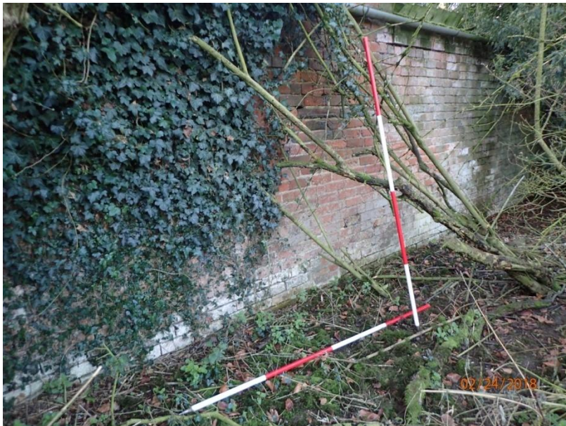
Plate 35: View of the North Elevation of Outbuilding 1, from the north-east
