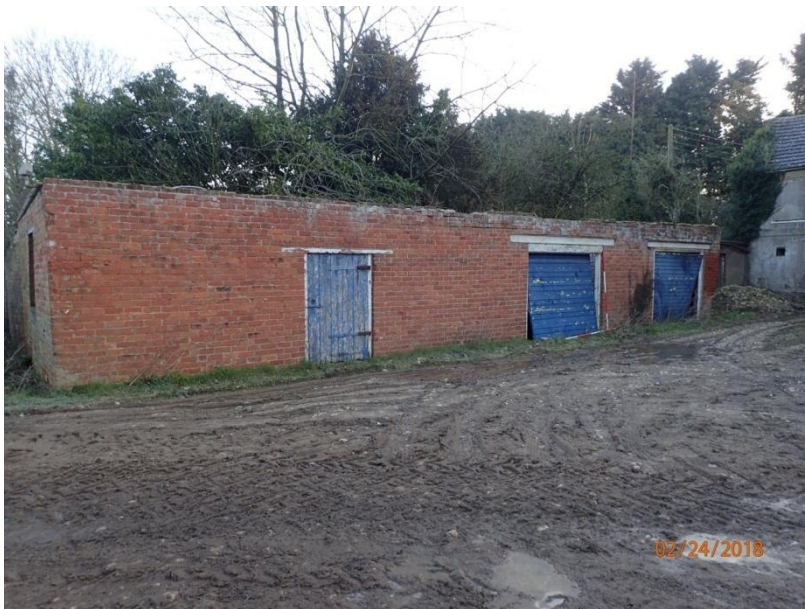
Plate 29: View of the South Elevation of Outbuilding 1, from the south
