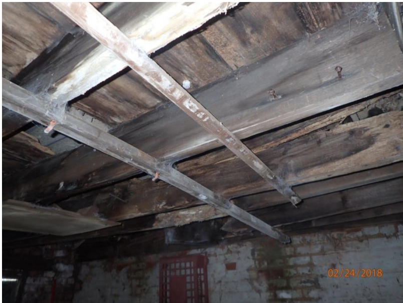
Plate 46: View of the ceiling of Cell 1, from the north-east
