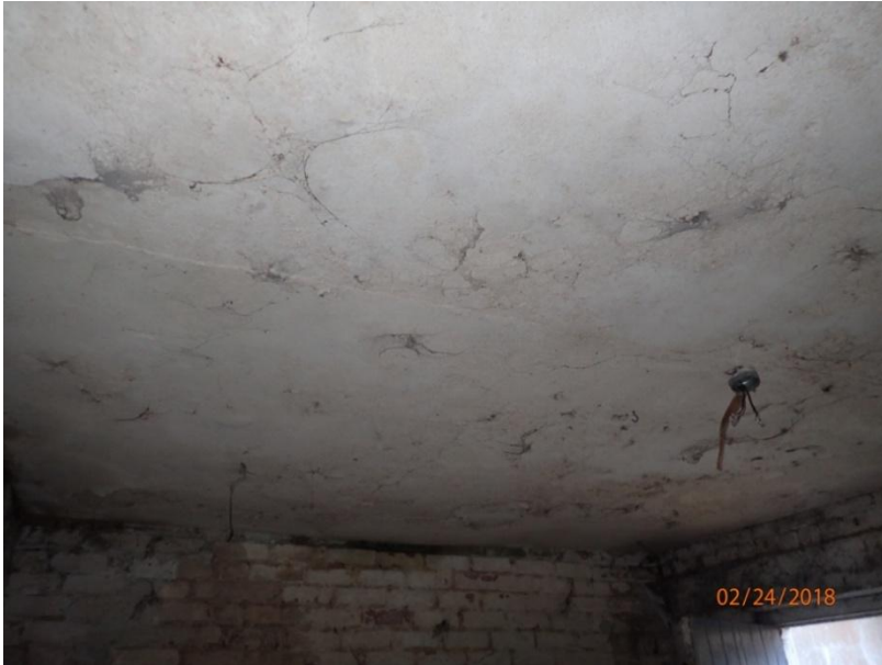
Plate 102: View of the ceiling of Cell 7, from the east
