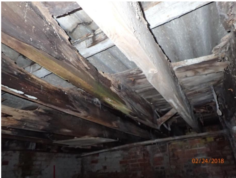
Plate 43: View of the ceiling of Cell 1, from the south
