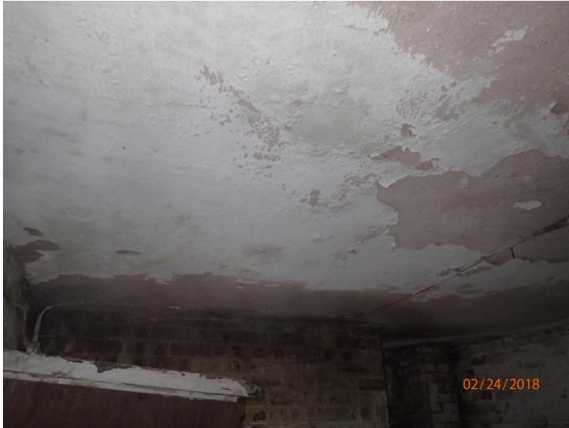
Plate 82: View of the ceiling of Cell 4, from the east
