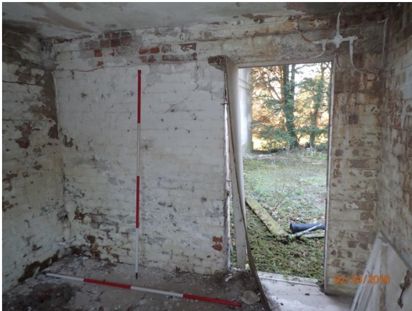
Plate 86: View of the south wall of Cell 4, from the north
