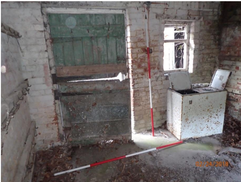
Plate 105: View of the south wall of Cell 7, from the north
