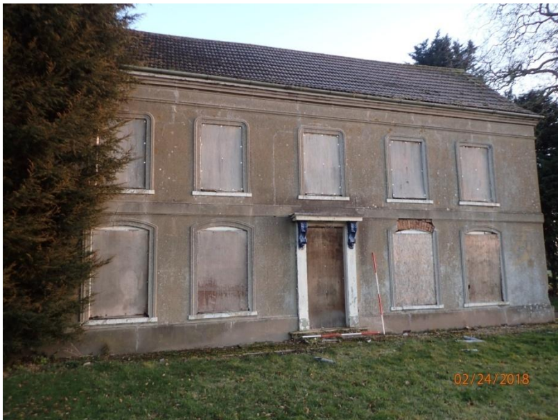
Plate 8: View of the South Elevation of the Farmhouse, from the south
