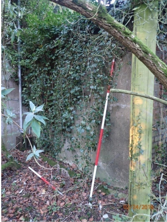
Plate 71: View of the East Elevation of Outbuilding 3, from the north
