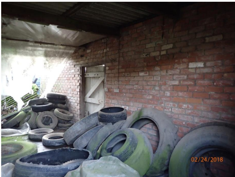
Plate 51: View of the south wall of Cell 2, from the west
