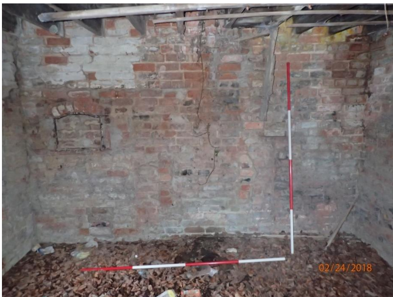
Plate 41: View of the north wall of Cell 1, from the south
