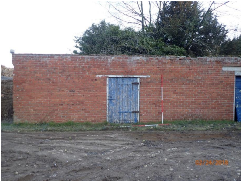
Plate 32: View of the South Elevation of Outbuilding 1, from the south
