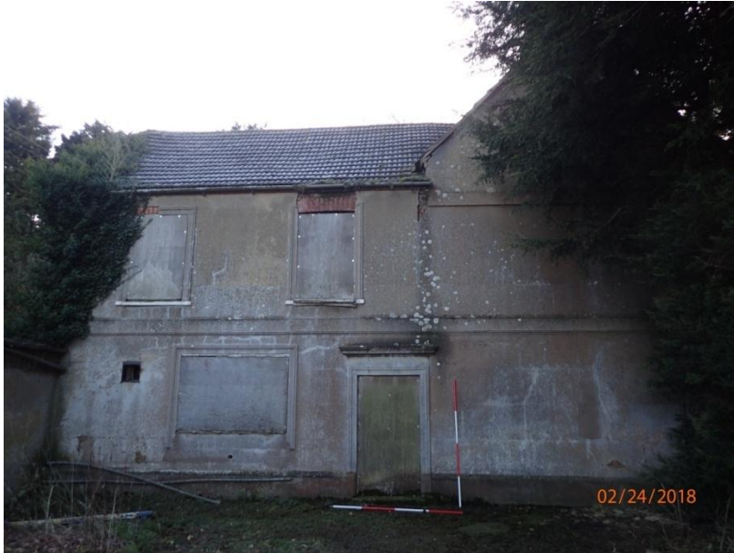
Plate 26: View of the West Elevation of the Farmhouse, from the west
