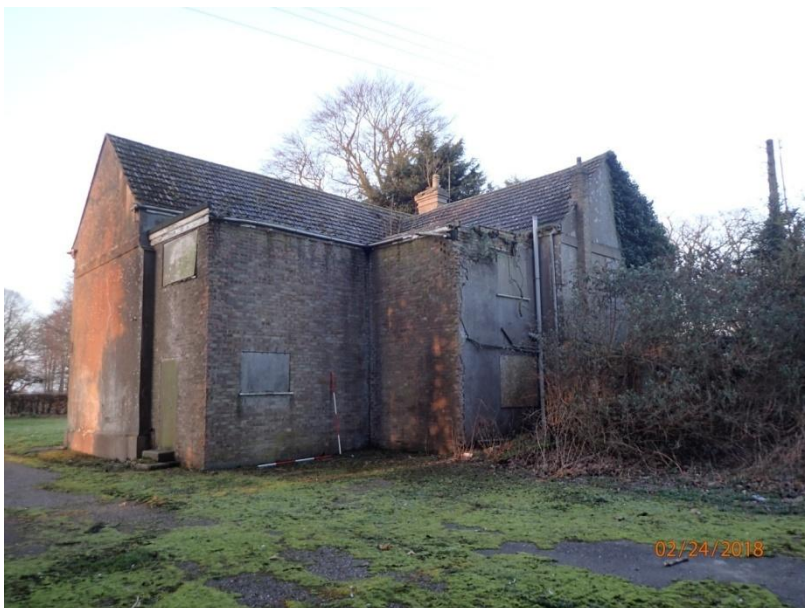
Plate 12: General View of the rear of the Farmhouse, from the north
