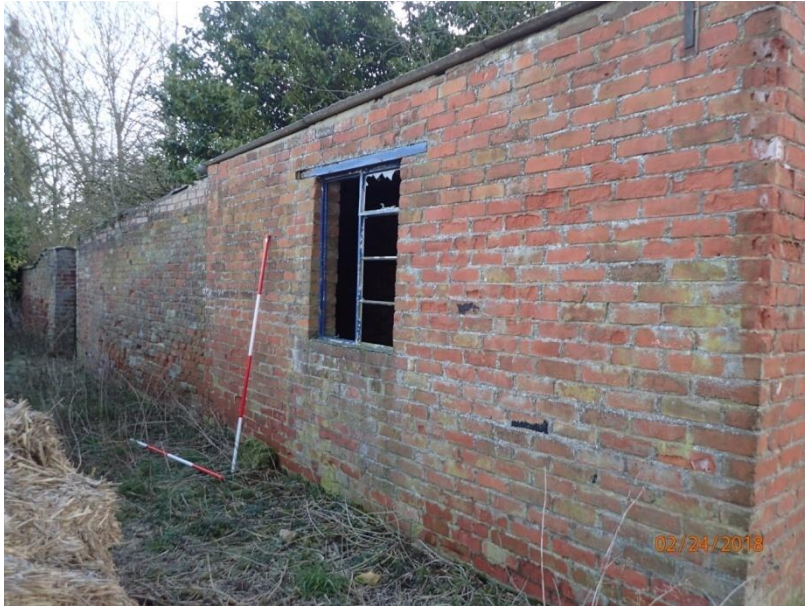
Plate 34: View of the West Elevation of Outbuilding 1, from the south
