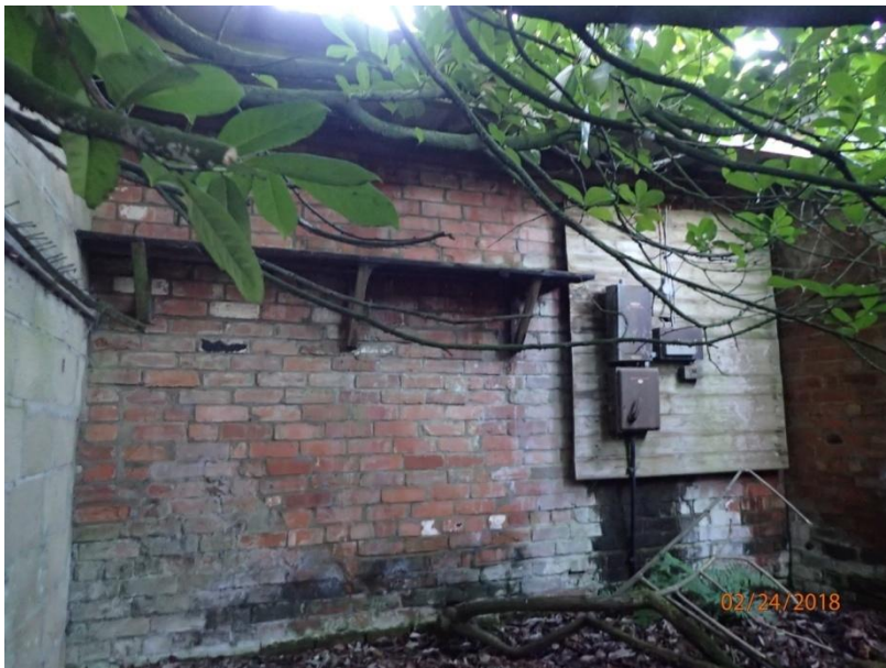
Plate 66: View of the north wall of Cell 3, from the north
