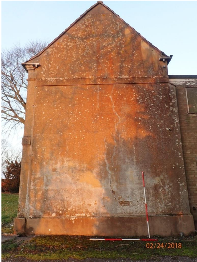
Plate 10: View of the East Elevation of the Farmhouse, from the east
