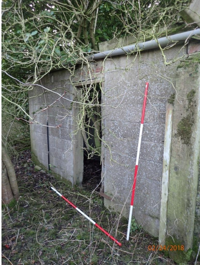
Plate 62: View of the North Elevation of Outbuilding 2, from the west
