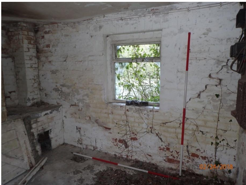
Plate 81: View of the north wall of Cell 4, from the south
