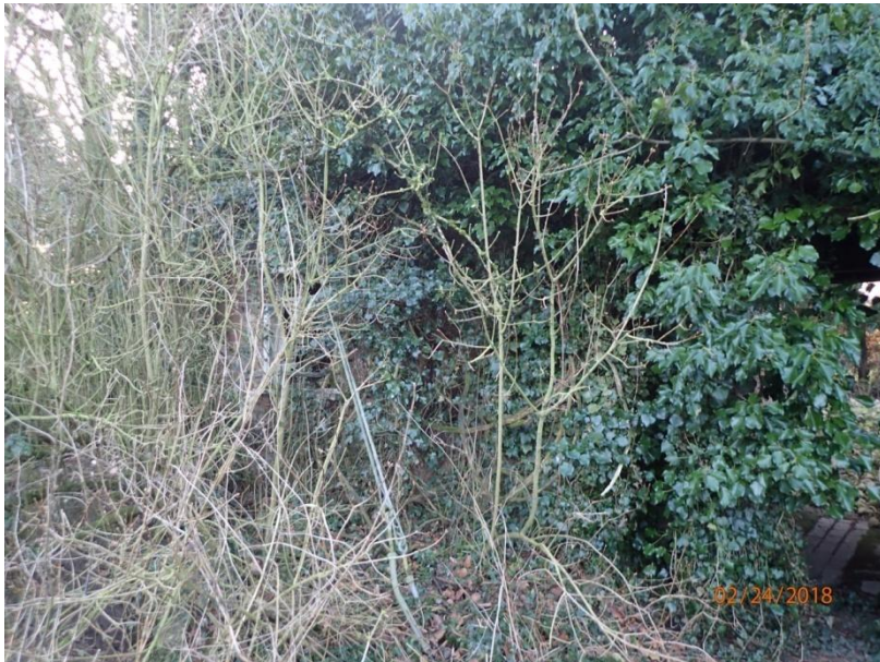
Plate 74: View of part of the North Elevation of Outbuilding 3, from the north
