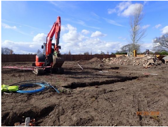
Plate 43: Excavation of the foundations, from the east
