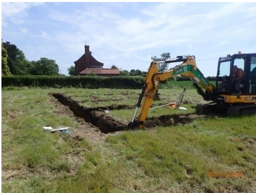
Plate 20: Excavation of the foundations, from the west
