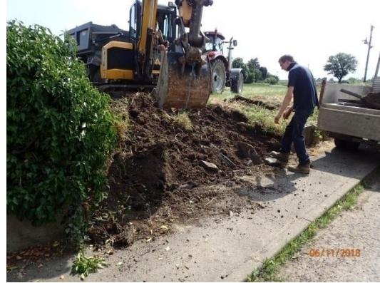
Plate 27: Ground reduction, from the east
