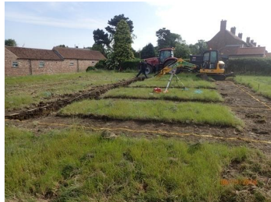
Plate 10: Excavation of the foundations, from the west
