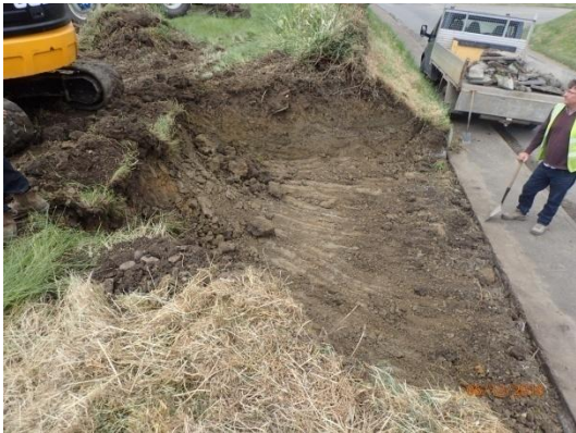
Plate 43: Ground reduction, from the east
