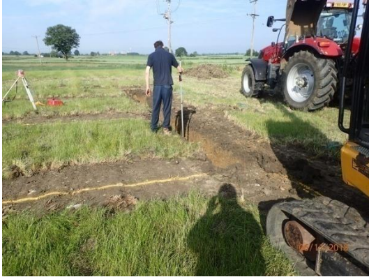
Plate 6: Excavation of the foundations, from the east
