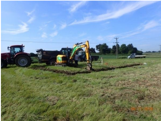
Plate 13: Excavation of the foundations, from the north-east
