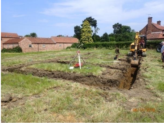
Plate 24: Excavation of the foundations, from the west
