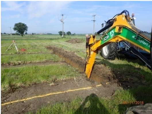
Plate 7: Excavation of the foundations, from the east
