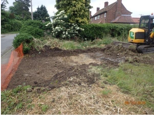
Plate 30: Ground reduction, from the west
