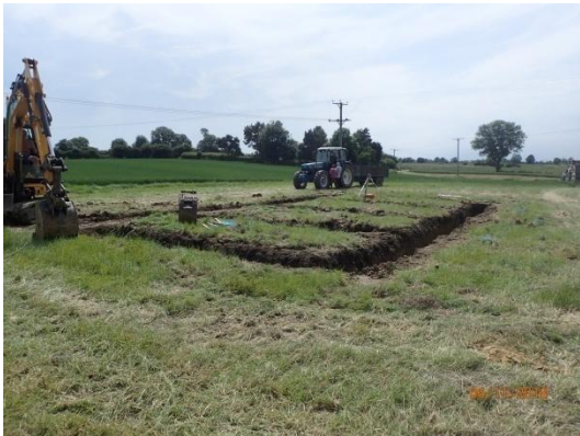
Plate 25: Excavation of the foundations, from the east
