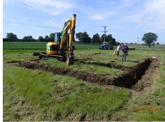
Plate 15: Excavation of the foundations, from the east
