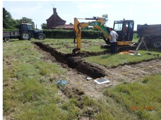
Plate 16: Excavation of the foundations, from the west
