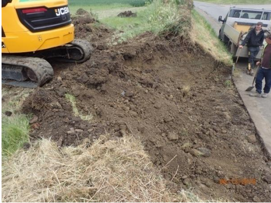
Plate 42: Ground reduction, from the east
