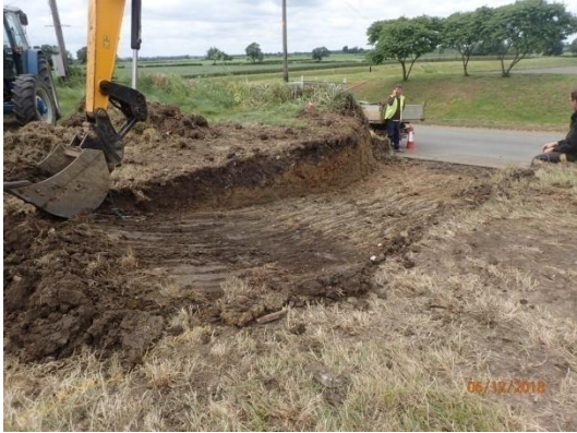
Plate 48: Ground reduction, from the south
