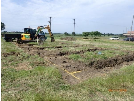
Plate 18: Excavation of the foundations, from the east
