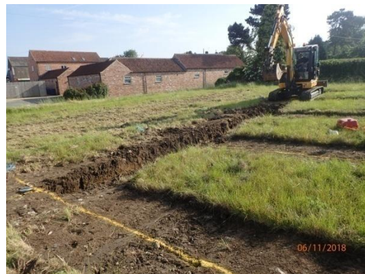
Plate 5: Excavation of the foundations, from the west
