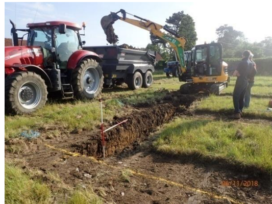
Plate 4: Excavation of the foundations, from the west
