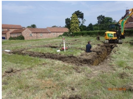
Plate 23: Excavation of the foundations, from the west
