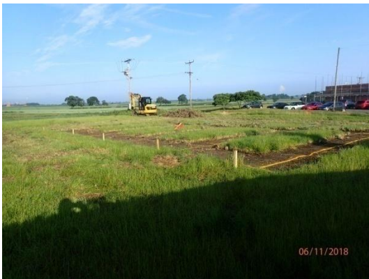
Plate 2: Pre-groundworks, from the west
