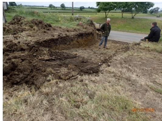
Plate 47: Ground reduction, from the south
