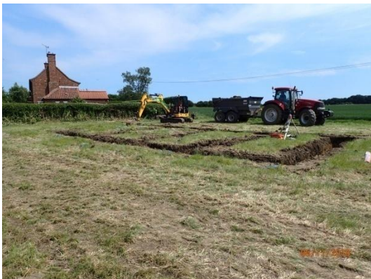
Plate 26: Excavation of the foundations, from the north-west
