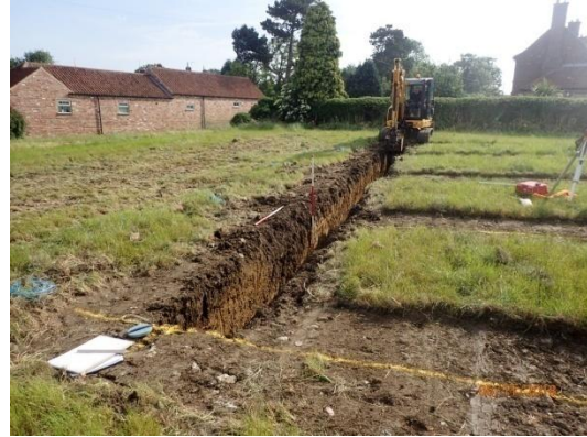
Plate 9: Excavation of the foundations, from the west
