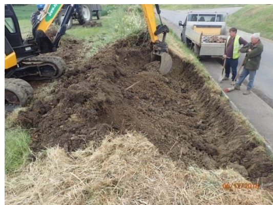
Plate 41: Ground reduction, from the east
