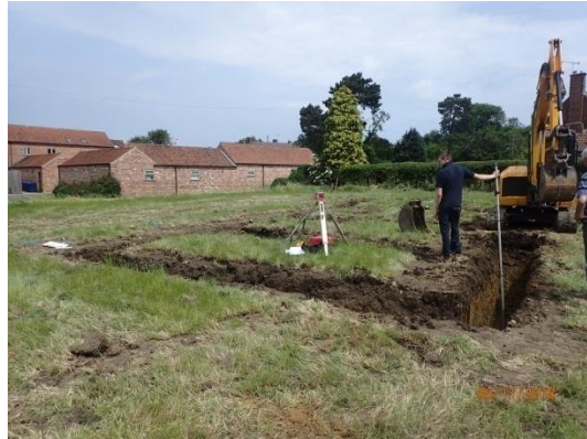
Plate 22: Excavation of the foundations, from the west
