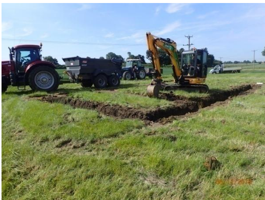
Plate 14: Excavation of the foundations, from the north-east
