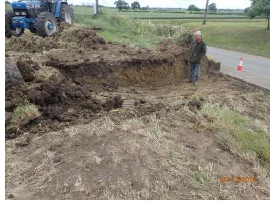
Plate 45: Ground reduction, from the east
