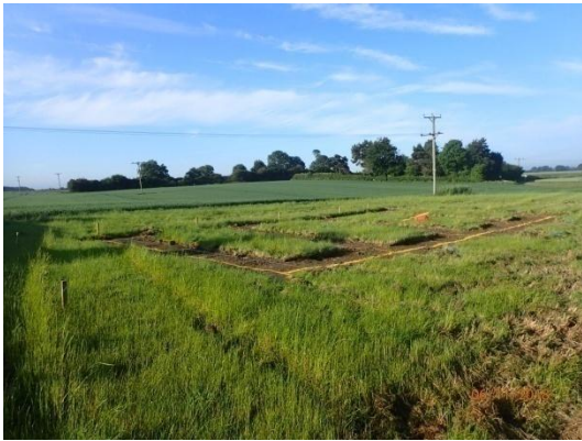
Plate 1: Pre-groundworks, from the south
