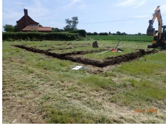
Plate 21: Excavation of the foundations, from the north-west
