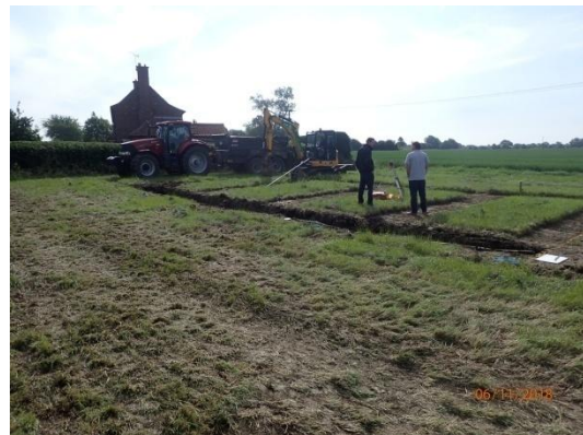
Plate 11: Excavation of the foundations, from the north-west
