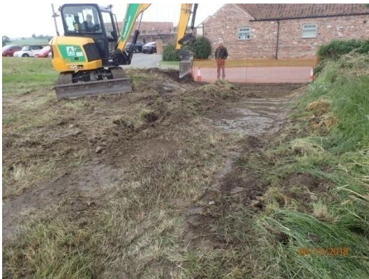
Plate 32: Ground reduction, from the south
