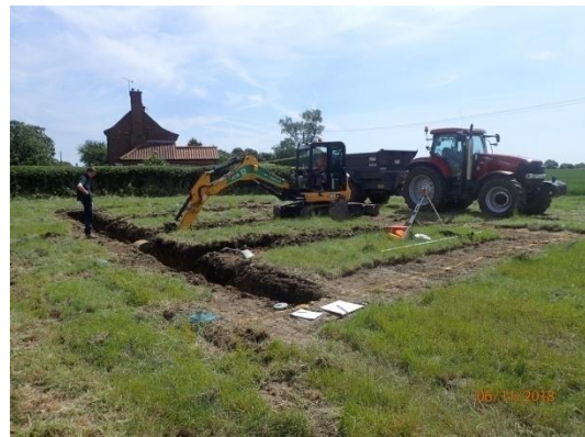
Plate 17: Excavation of the foundations, from the north-west
