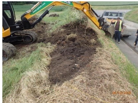
Plate 40: Ground reduction, from the east
