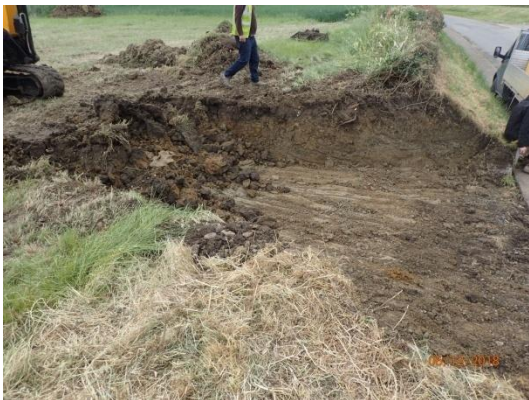
Plate 44: Ground reduction, from the east
