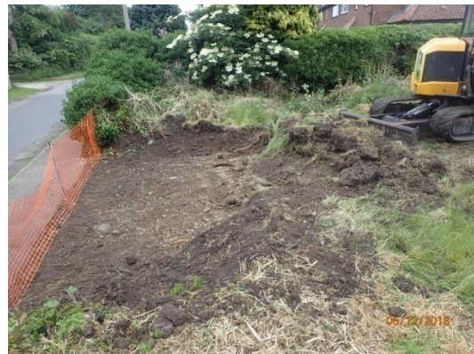
Plate 29: Ground reduction, from the west
