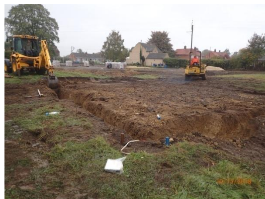
Plate 64: House Plot 4, excavation of the foundations, from the north-east
