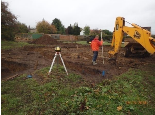
Plate 71: House Plot 4, excavation of the foundations, from the north-west
