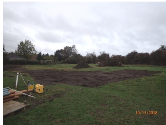
Plate 45: Initial groundworks, from the north-east
