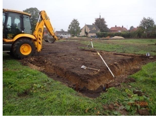
Plate 50: House Plot 4, excavation of the garage foundations, from the north-east
