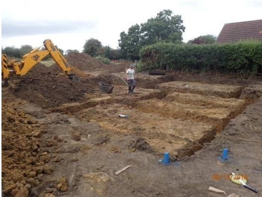
Plate 17: Excavation of the foundations, House Plot 2, from the south-west
