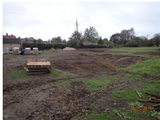
Plate 81: Backfilled relict pond & site of House Plot 3, from the north-east
