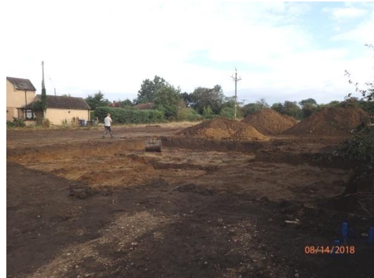
Plate 20: House Plot 2, completed groundworks, from the south-east
