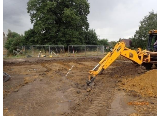
Plate 14: Excavation of the foundations, House Plot 2, from the north
