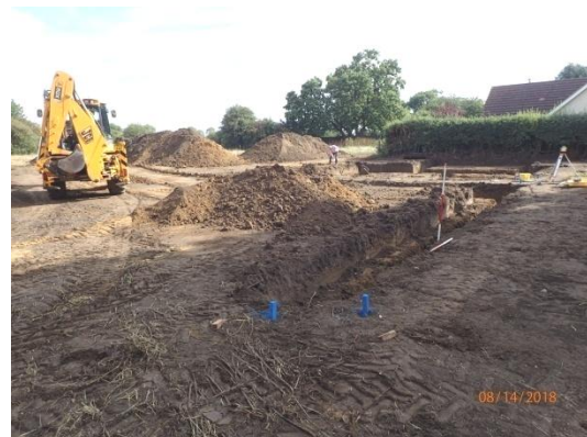
Plate 28: Excavation of the foundations, House Plot 1, from the south-west
