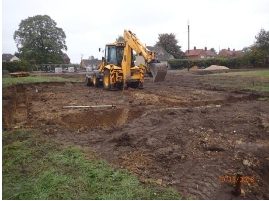
Plate 65: House Plot 4, excavation of the foundations, from the north-east
