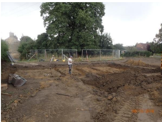
Plate 13: Excavation of the foundations, House Plot 2, from the north
