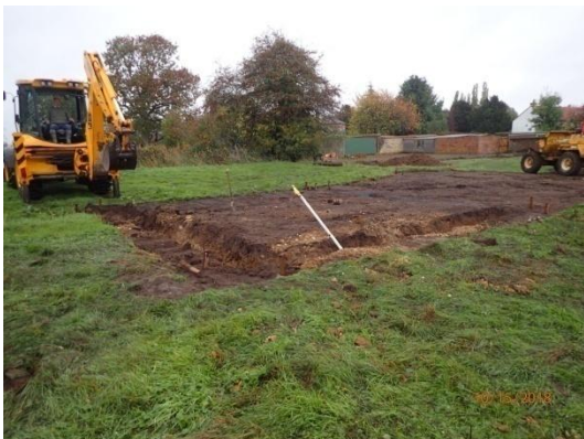
Plate 49: House Plot 4, excavation of the garage foundations, from the west
