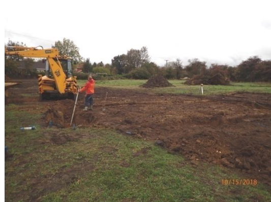
Plate 70: House Plot 4, excavation of the foundations, from the east
