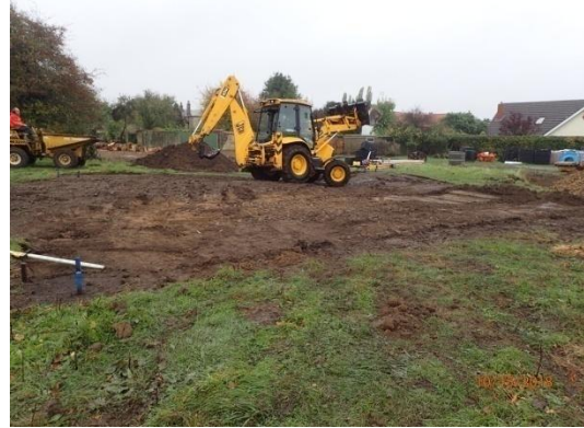
Plate 56: House Plot 4, ground reduction, from the north
