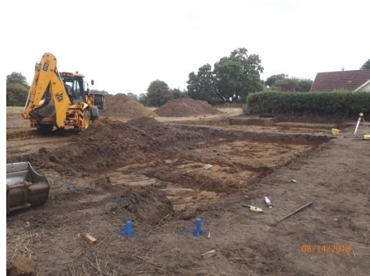
Plate 33: Excavation of the foundations, House Plot 1, from the south-west
