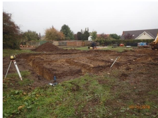
Plate 76: House Plot 4, excavation of the foundations, from the north-west
