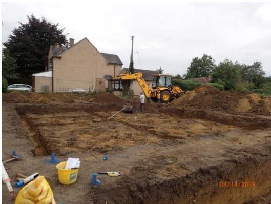
Plate 43: Completed groundworks, House Plot 1, from the east
