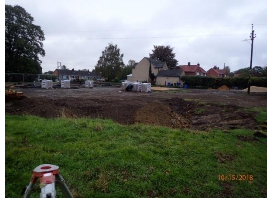
Plate 80: Backfilled relict pond & site of House Plot 3, from the east
