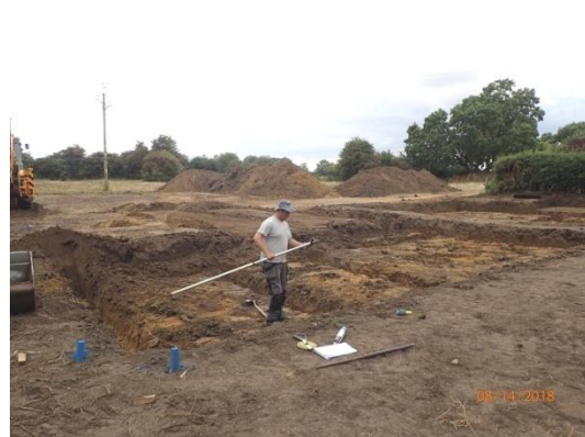
Plate 34: Excavation of the foundations, House Plot 1, from the south-west
