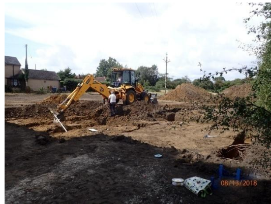
Plate 5: Excavation of the foundations, House Plot 2, from the south-east
