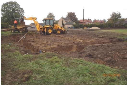
Plate 66: House Plot 4, excavation of the foundations, from the north-east
