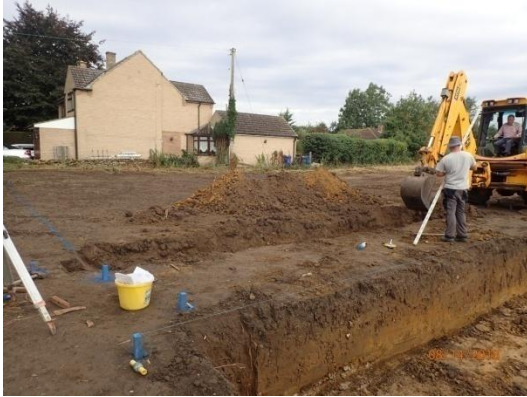
Plate 23: Excavation of the foundations, House Plot 1, from the south-east
