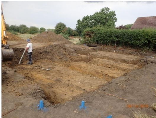
Plate 8: Excavation of the foundations, House Plot 2, from the south-west
