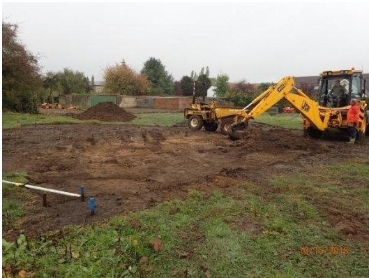
Plate 55: House Plot 4, ground reduction, from the north-west
