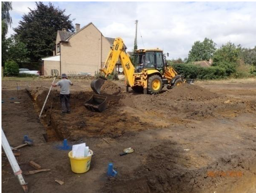
Plate 30: Excavation of the foundations, House Plot 1, from the south-east
