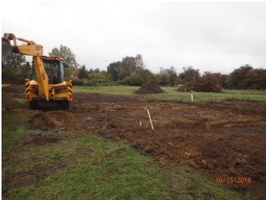
Plate 67: House Plot 4, excavation of the foundations, from the east
