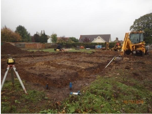
Plate 77: House Plot 4, excavation of the foundations, from the north-west
