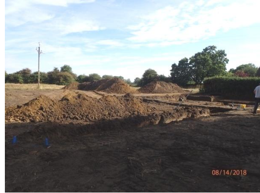
Plate 26: Excavation of the foundations, House Plot 1, from the south-west
