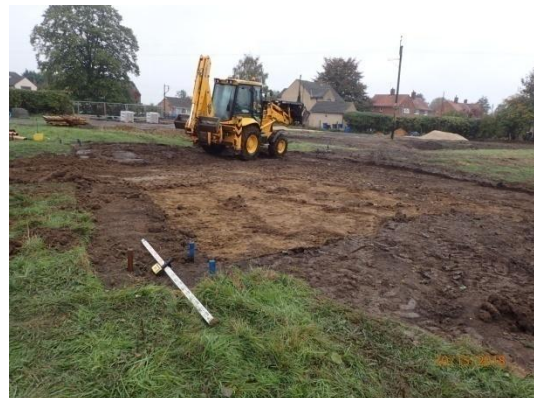
Plate 58: House Plot 4, ground reduction, from the north
