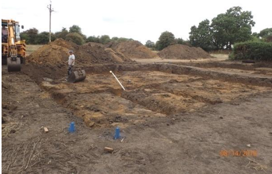
Plate 42: Completed groundworks, House Plot 1, from the south
