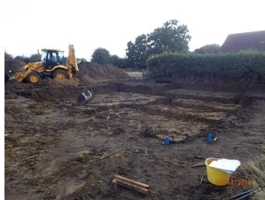
Plate 22: House Plot 2, completed groundworks, from the south-west
