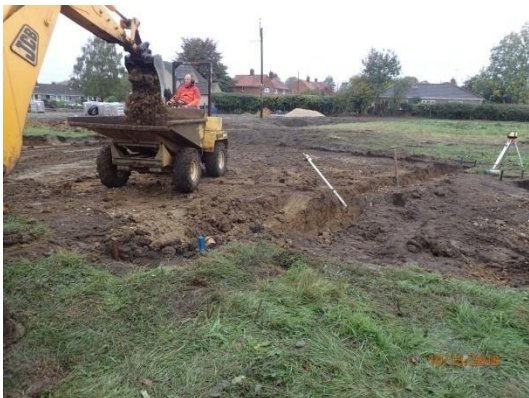
Plate 60: House Plot 4, excavation of the foundations, from the north-east
