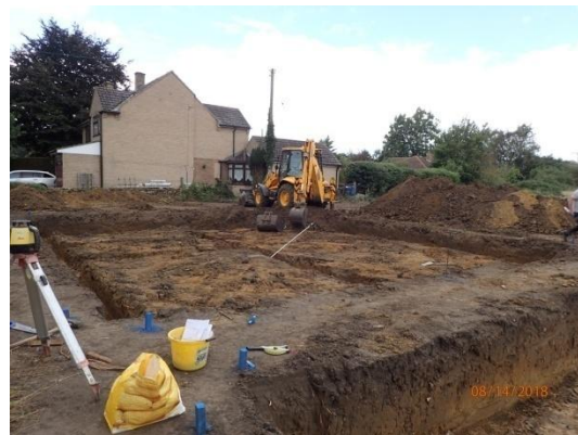
Plate 39: Excavation of the foundations, House Plot 1, from the east
