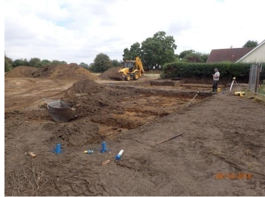
Plate 32: Excavation of the foundations, House Plot 1, from the south-west
