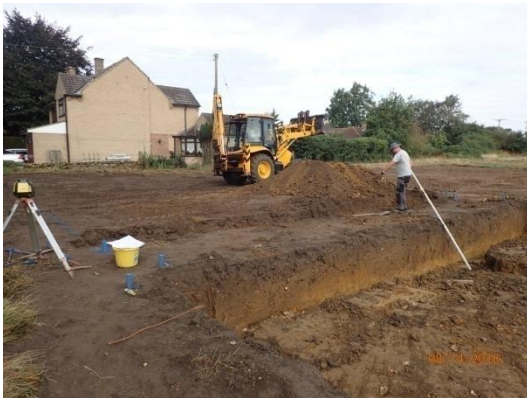
Plate 24: Excavation of the foundations, House Plot 1, from the south-east
