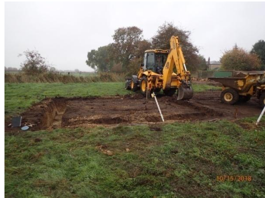
Plate 51: House Plot 4, excavation of the garage foundations, from the west
