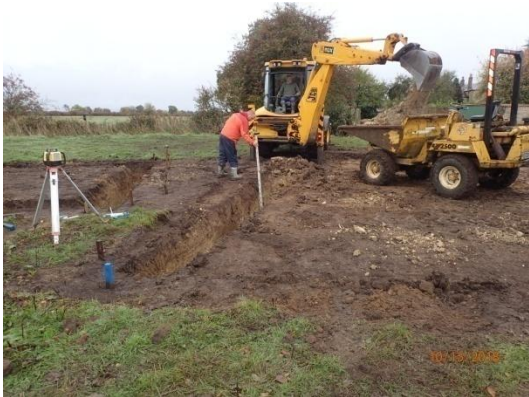
Plate 59: House Plot 4, excavation of the foundations, from the west
