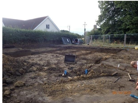
Plate 21: House Plot 2, completed groundworks, from the north-west
