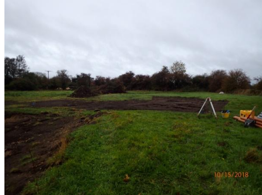
Plate 44: Initial groundworks, from the south
