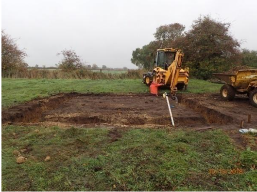
Plate 53: House Plot 4, excavation of the garage foundations, from the south
