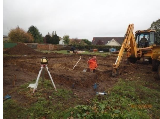
Plate 74: House Plot 4, excavation of the foundations, from the north-west
