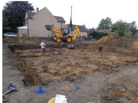
Plate 40: Excavation of the foundations, House Plot 1, from the east
