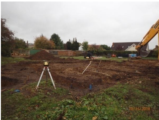
Plate 73: House Plot 4, excavation of the foundations, from the north-west
