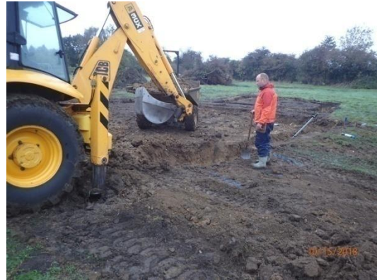
Plate 62: House Plot 4, excavation of the foundations, from the south-east
