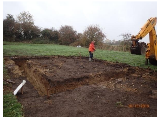
Plate 52: House Plot 4, excavation of the garage foundations, from the south
