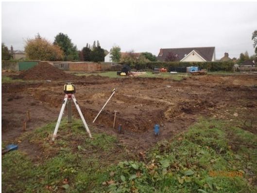
Plate 72: House Plot 4, excavation of the foundations, from the north-west
