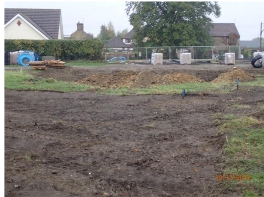
Plate 82: Backfilled relict pond & site of House Plot 3, from the north
