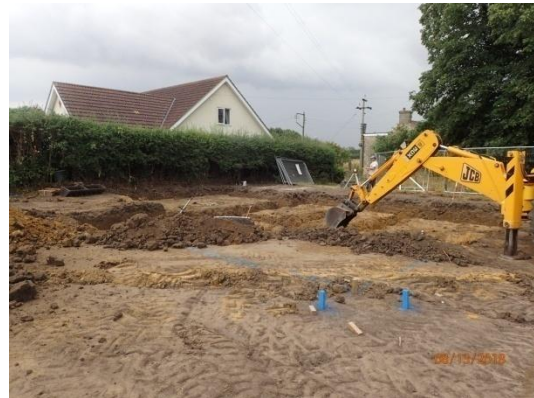
Plate 15: Excavation of the foundations, House Plot 2, from the north-west
