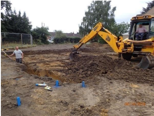
Plate 36: Excavation of the foundations, House Plot 1, from the north
