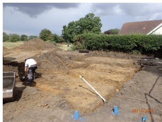
Plate 6: Excavation of the foundations, House Plot 2, from the south-west
