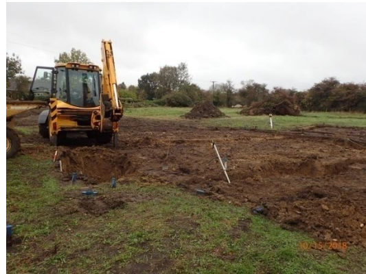
Plate 69: House Plot 4, excavation of the foundations, from the east
