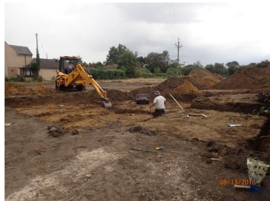
Plate 16: Excavation of the foundations, House Plot 2, from the south-east
