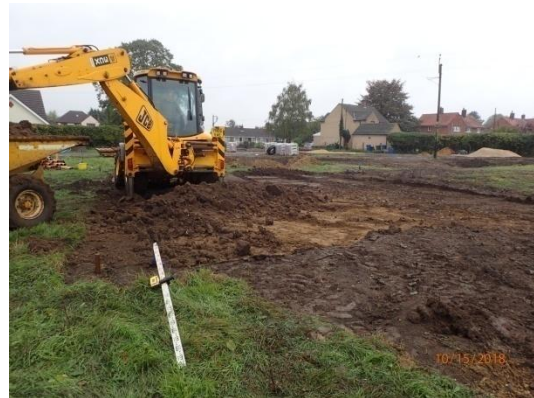
Plate 57: House Plot 4, ground reduction, from the north
