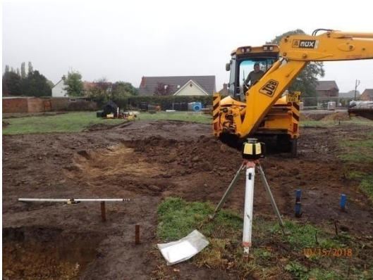
Plate 54: House Plot 4, ground reduction, from the north
