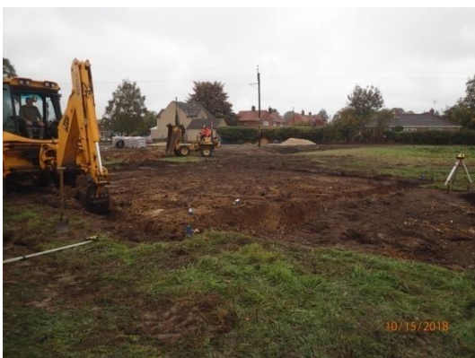
Plate 61: House Plot 4, excavation of the foundations, from the north-east
