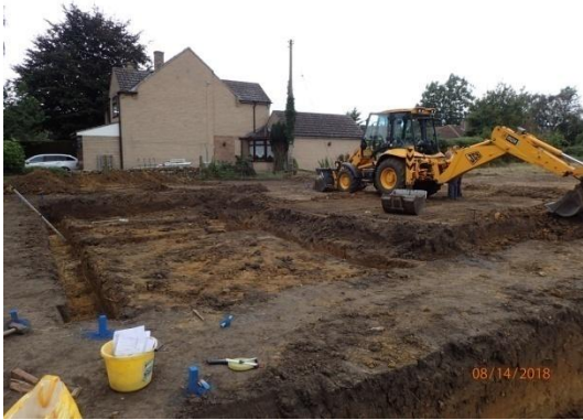
Plate 35: Excavation of the foundations, House Plot 1, from the south-east
