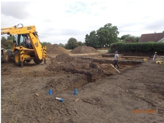
Plate 31: Excavation of the foundations, House Plot 1, from the south-west
