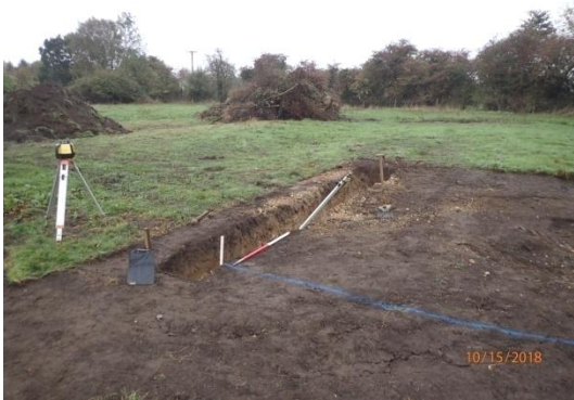
Plate 48: House Plot 4, excavation of the garage foundations, from the south
