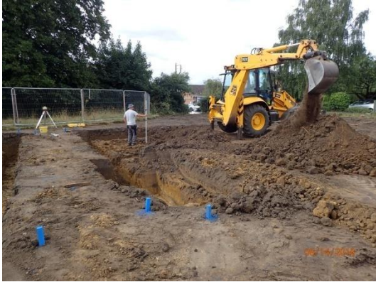
Plate 29: Excavation of the foundations, House Plot 1, from the north
