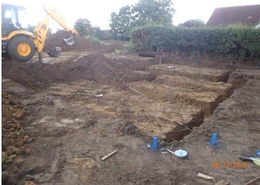
Plate 12: Excavation of the foundations, House Plot 2, from the south-west
