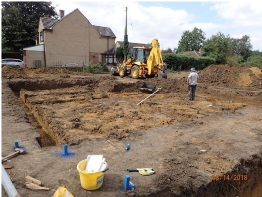
Plate 37: Excavation of the foundations, House Plot 1, from the west
