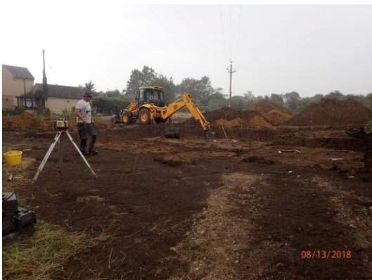
Plate 19: Excavation of the foundations, House Plot 2, from the south-west
