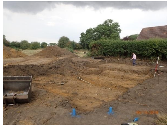
Plate 10: Excavation of the foundations, House Plot 2, from the south-west
