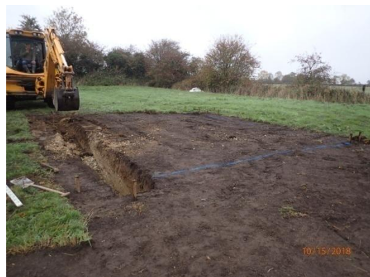
Plate 46: House Plot 4, excavation of the garage foundations, from the south
