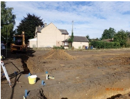
Plate 25: Excavation of the foundations, House Plot 1, from the east
