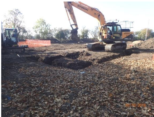
Plate 45: Excavation of the foundations, from the north-east
