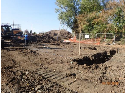
Plate 49: Excavation of the foundations, from the south-east
