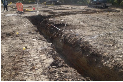
Plate 61: House Plot 13, excavated foundation trenches, from the west
