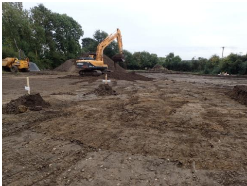
Plate 32: Further ground reduction of site access road, from the north-west
