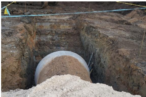
Plate 69: Excavation of the main foul sewer trench, from the west
