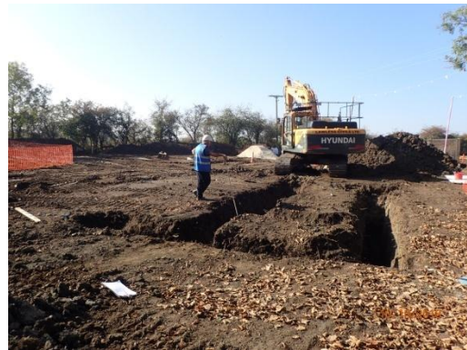
Plate 47: Excavation of the foundations, from the east
