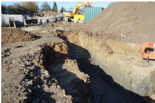
Plate 78: Excavation of the main foul sewer trench, from the east
