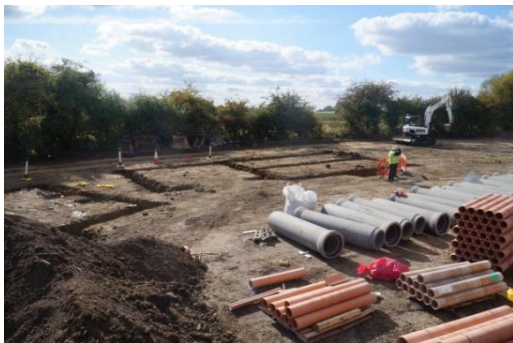
Plate 57: House Plot 11, excavated foundation trenches, from the north
