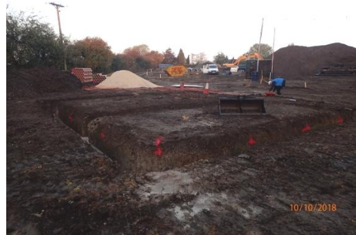
Plate 66: House Plots 8 and 9, excavated foundation trenches, from the south
