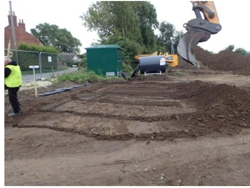
Plate 34: Further ground reduction within site compound area, from the west
