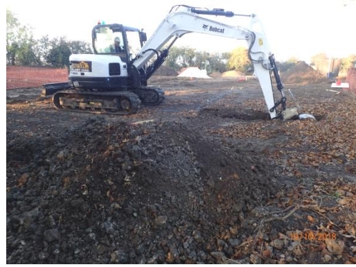
Plate 40: Excavation of the foundations, from the east
