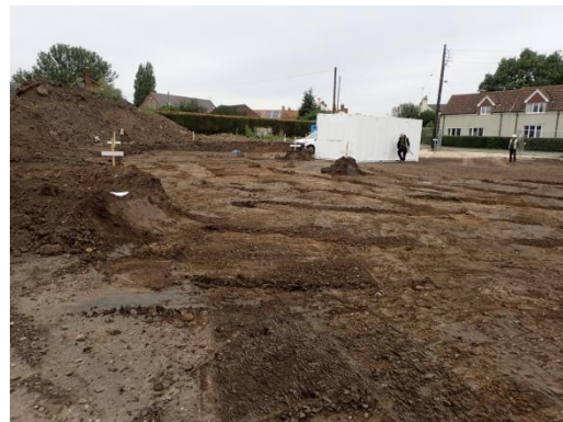
Plate 30: Further ground reduction of site access road, from the south-east
