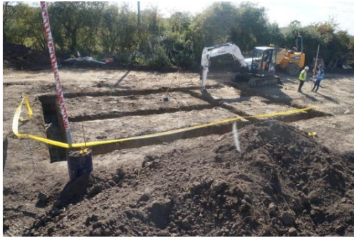
Plate 55: House Plot 10, excavated foundation trenches, from the north
