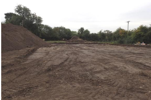
Plate 14: Initial ground reduction, from the west
