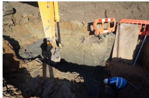
Plate 73: Excavation of the main foul sewer trench, from the south
