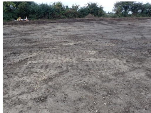
Plate 24: Initial ground reduction, from the north
