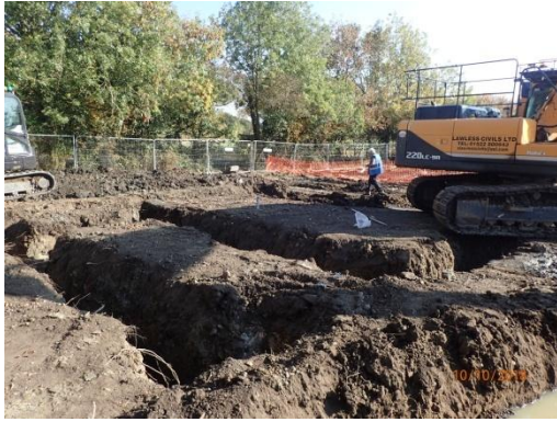
Plate 50: Excavation of the foundations, from the west
