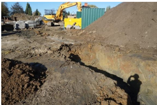
Plate 79: Excavation of the main foul sewer trench, from the east
