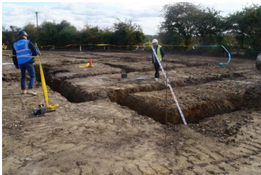
Plate 64: House Plot 13, excavated foundation trenches, from the west
