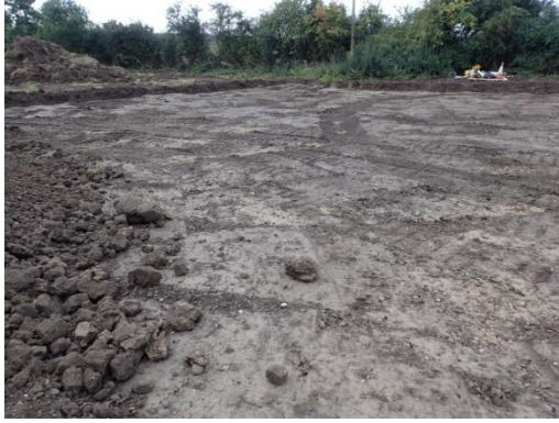
Plate 25: Initial ground reduction, from the west
