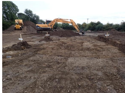
Plate 29: Further ground reduction of site access road, from the north-west
