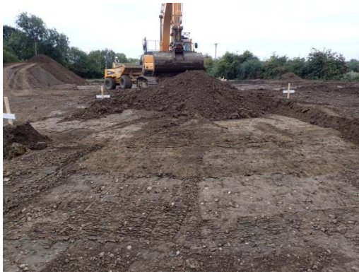
Plate 26: Further ground reduction of site access road, from the north-west
