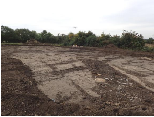
Plate 13: Initial ground reduction, from the west
