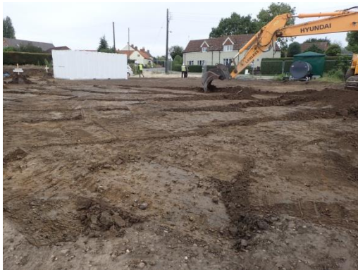
Plate 33: Further ground reduction of site access road, from the south-east
