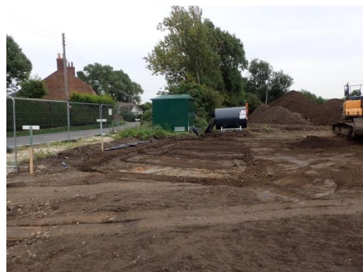
Plate 35: Further ground reduction within site compound area, from the west
