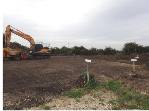
Plate 4: Initial ground reduction, from the north
