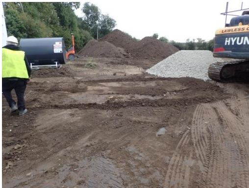
Plate 38: Further ground reduction within the site compound area, from the west
