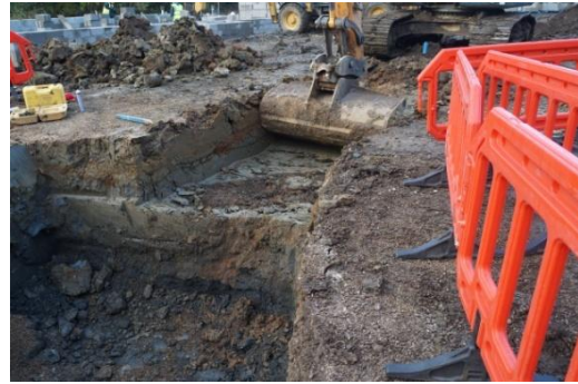
Plate 72: Excavation of the main foul sewer trench, from the east
