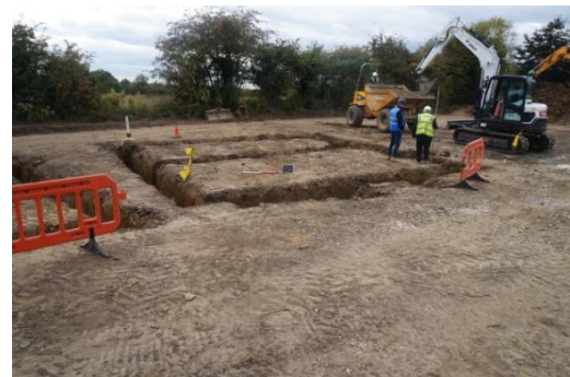
Plate 60: House Plot 12, excavated foundation trenches, from the north
