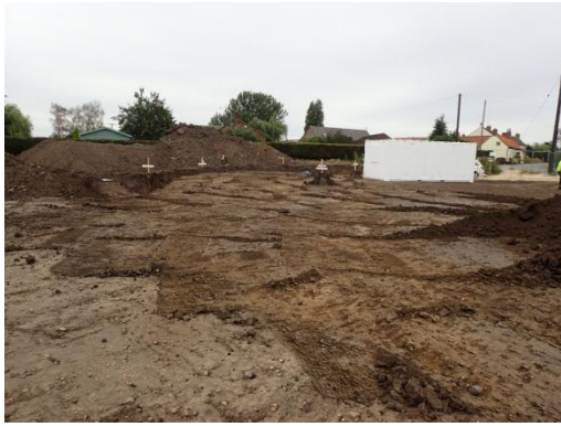
Plate 31: Further ground reduction of site access road, from the south-east
