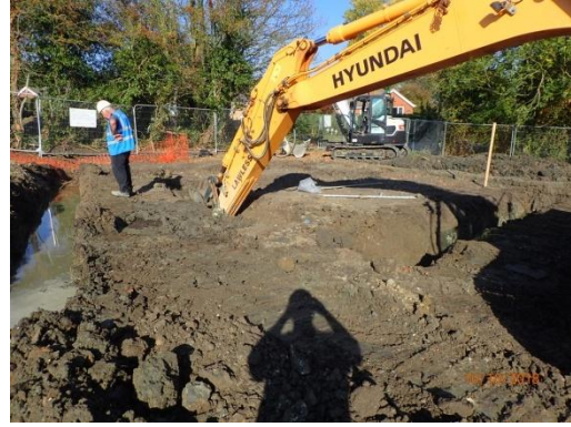
Plate 52: Excavation of the foundations, from the south
