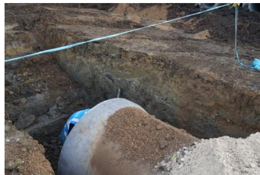
Plate 67: Excavation of the main foul sewer trench, from the north-west
