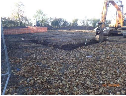
Plate 43: Excavation of the foundations, from the east
