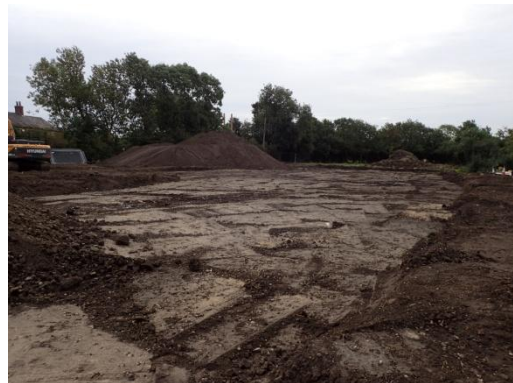
Plate 11: Initial ground reduction, from the south-west
