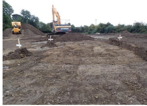
Plate 28: Further ground reduction of site access road, from the north-west
