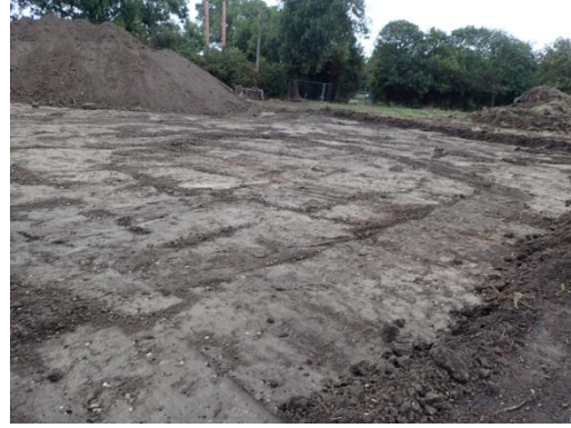
Plate 22: Initial ground reduction, from the north-west
