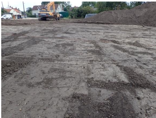
Plate 21: Initial ground reduction, from the south
