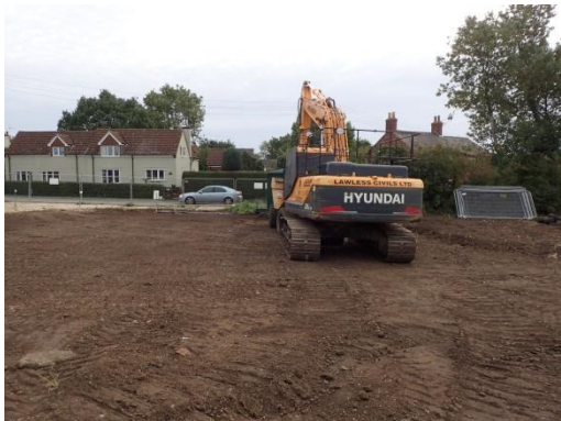
Plate 8: Initial ground reduction, from the south
