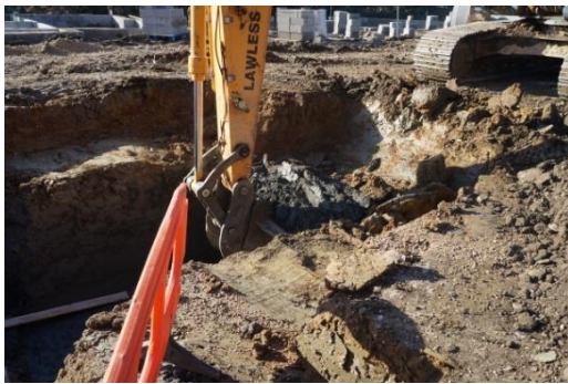
Plate 77: Excavation of the main foul sewer trench, from the east
