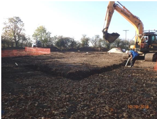
Plate 44: Excavation of the foundations, from the north-east
