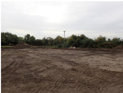
Plate 15: Initial ground reduction, from the north
