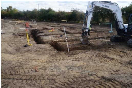
Plate 63: House Plot 13, excavated foundation trenches, from the west
