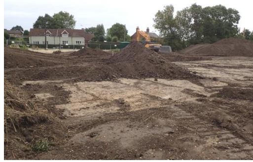
Plate 10: Initial ground reduction, from the south-west
