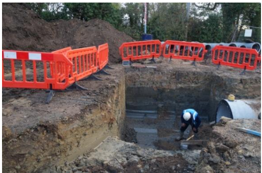
Plate 70: Excavation of the main foul sewer trench, from the south
