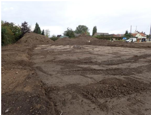
Plate 20: Initial ground reduction, from the west
