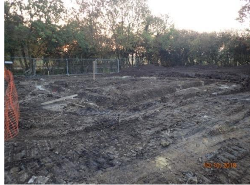
Plate 65: House Plots 6 and 7, excavated foundation trenches, from the west
