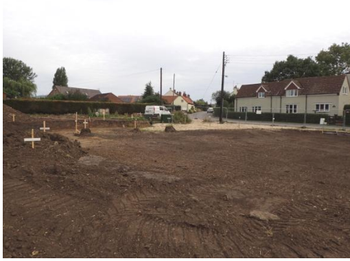
Plate 7: Initial ground reduction, from the south
