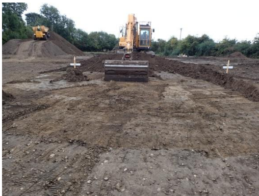
Plate 27: Further ground reduction of site access road, from the north-west
