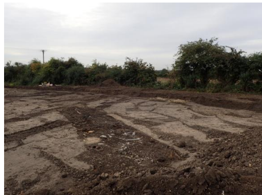
Plate 12: Initial ground reduction, from the west
