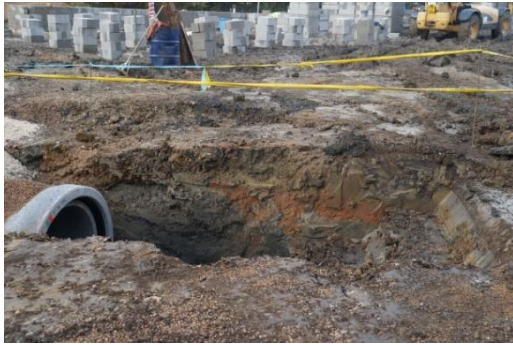
Plate 68: Excavation of the main foul sewer trench, from the north
