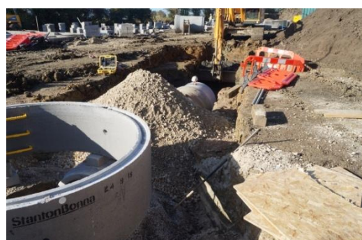
Plate 75: Excavation of the main foul sewer trench, from the east
