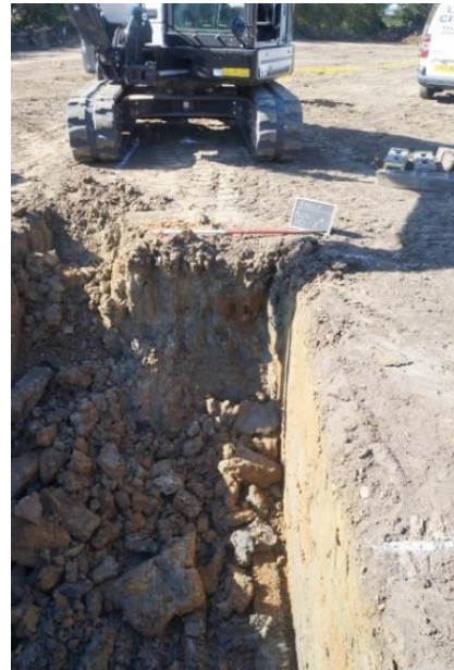
Plate 54: House Plot 10, excavated foundation trench, from the south-east
