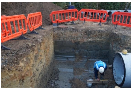
Plate 71: Excavation of the main foul sewer trench, from the south
