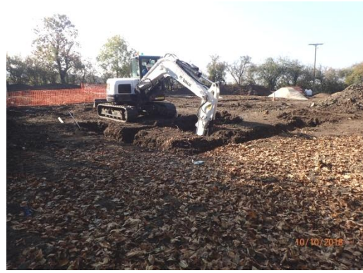
Plate 46: Excavation of the foundations, from the north-east
