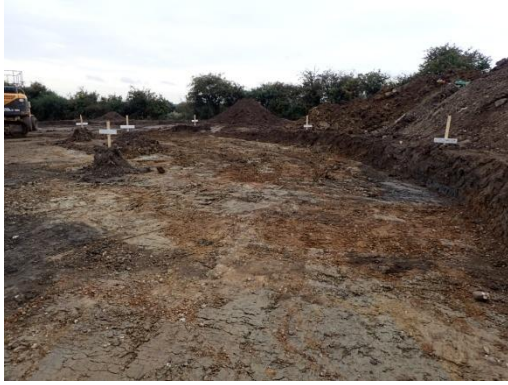
Plate 37: Further ground reduction of site access road, from the south-east
