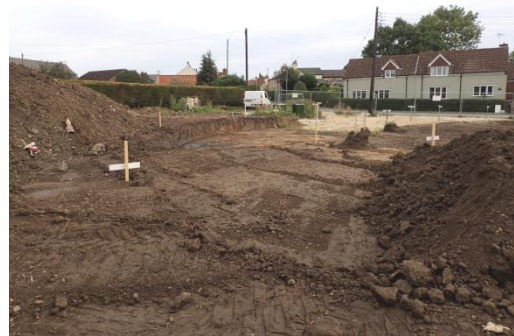
Plate 6: Reduced site access road, from the south-west
