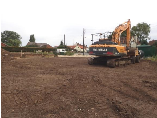
Plate 9: Initial ground reduction, from the south
