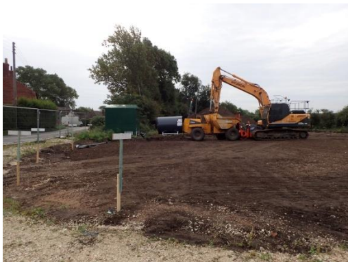
Plate 3: Initial ground reduction, from the north-west
