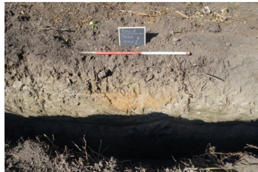
Plate 82: Excavated second service trench, Representative Section 10 , from the south
