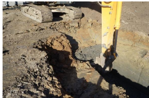
Plate 74: Excavation of the main foul sewer trench, from the south-east
