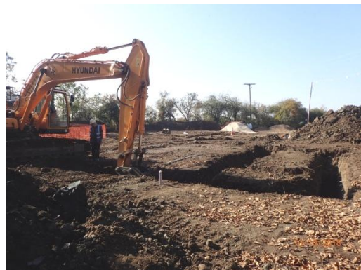
Plate 48: Excavation of the foundations, from the east
