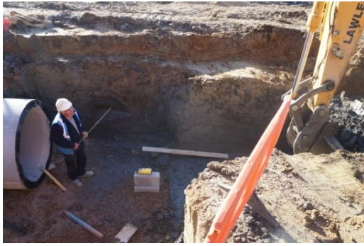
Plate 76: Excavation of the main foul sewer trench, from the south
