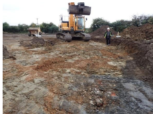
Plate 36: Further ground reduction of site access road, from the south-east
