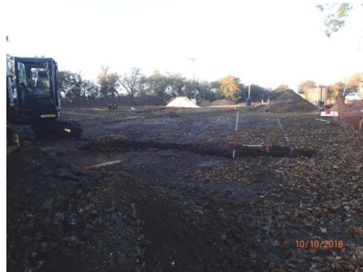
Plate 41: Excavation of the foundations, from the east
