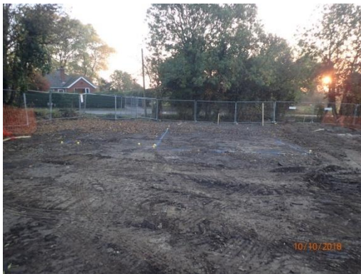
Plate 39: Pre-groundworks, from the west
