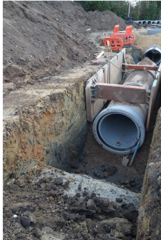
Plate 80: Excavation of the main foul sewer trench, from the west
