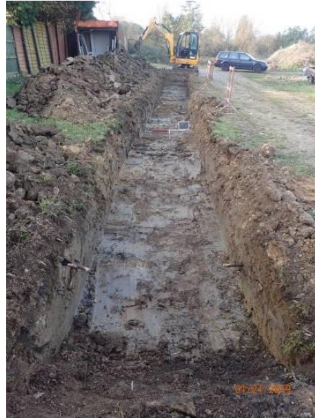
Plate 4: Trench 1 , from the east
