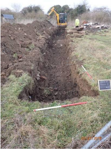
Plate 11: Trench 3, from the south-east
