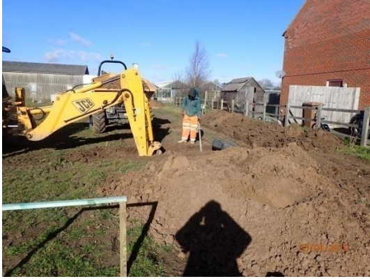
Plate 6: Excavation of the foundations, from the east
