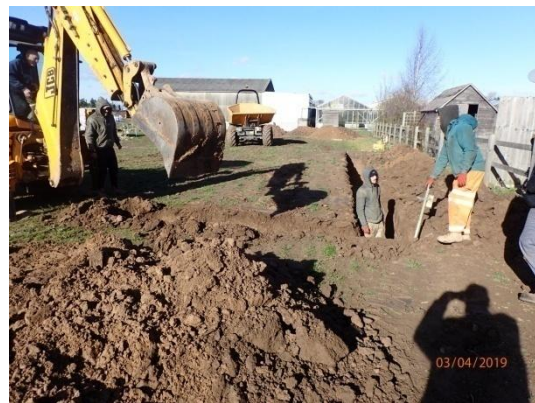
Plate 5: Excavation of the foundations, from the east
