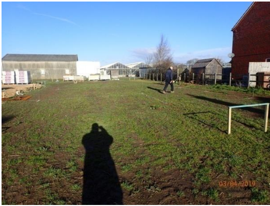
Plate 1: Set out foundations, from the east
