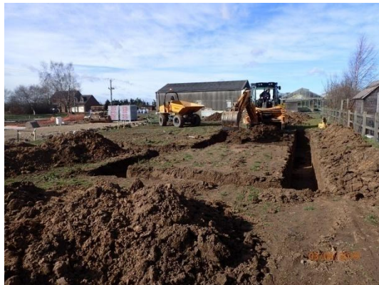
Plate 11: Excavation of the foundations, from the east
