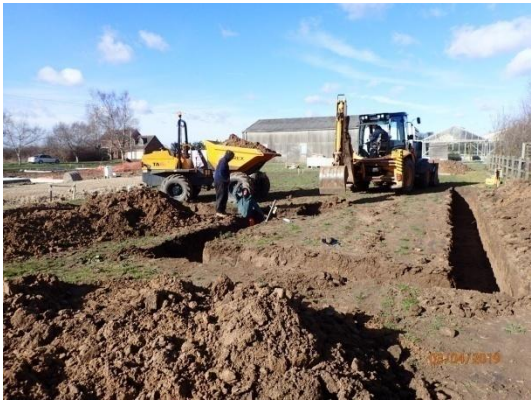
Plate 8: Excavation of the foundations, from the east
