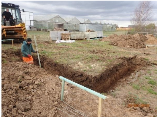
Plate 25: Excavation of the foundations, from the south-east
