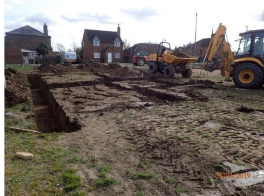
Plate 15: Excavation of the foundations, from the west
