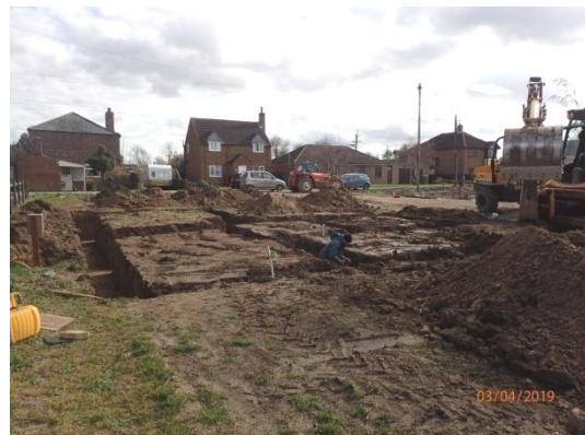
Plate 17: Excavation of the foundations, from the west
