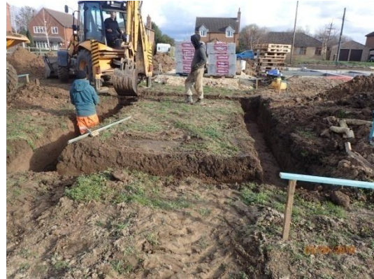
Plate 27: Excavation of the foundations, from the west
