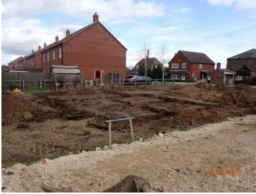
Plate 18: Excavation of the foundations, from the south
