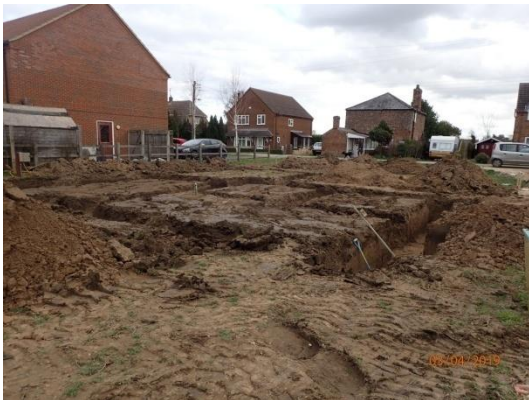
Plate 20: Excavation of the foundations, from the south-west
