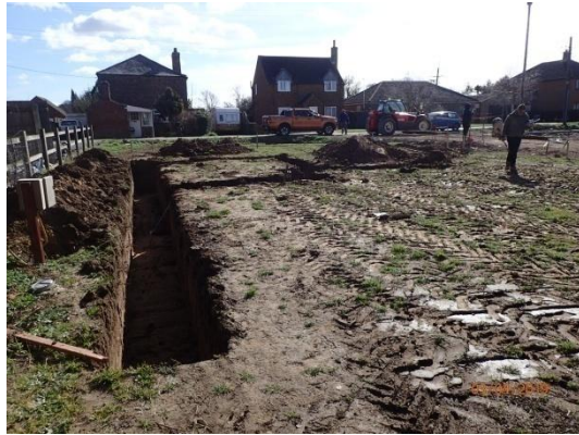
Plate 10: Excavation of the foundations, from the west
