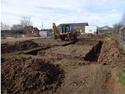
Plate 12: Excavation of the foundations, from the east
