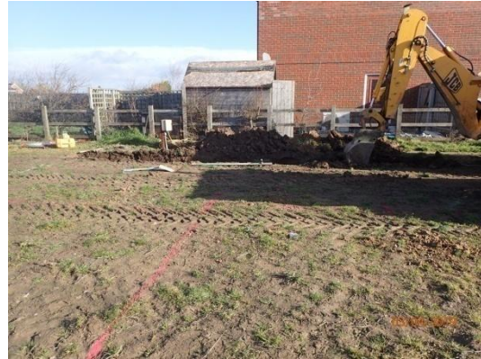
Plate 3: Excavation of the foundations, from the south
