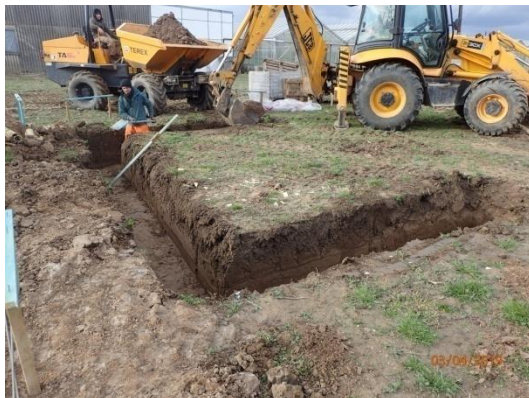
Plate 26: Excavation of the foundations, from the east
