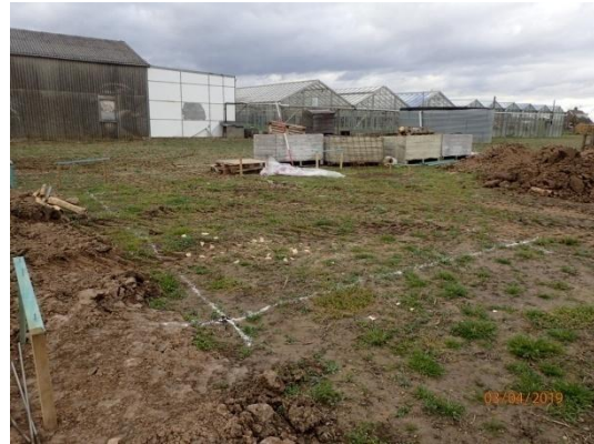
Plate 22: Set out foundations, from the east
