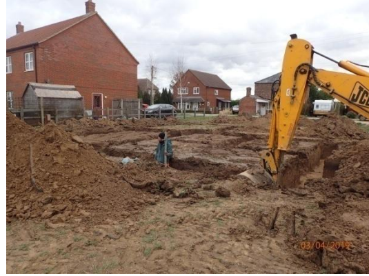
Plate 21: Excavation of the foundations, from the south-west
