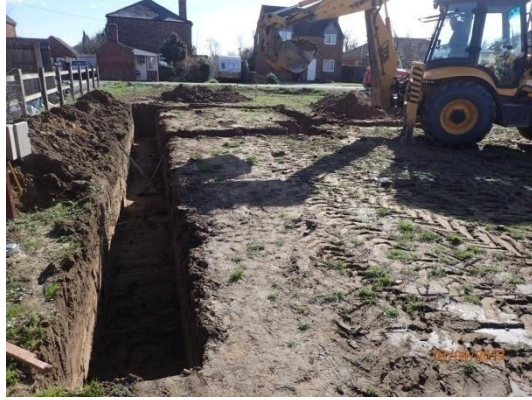
Plate 9: Excavation of the foundations, from the west
