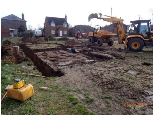
Plate 14: Excavation of the foundations, from the west
