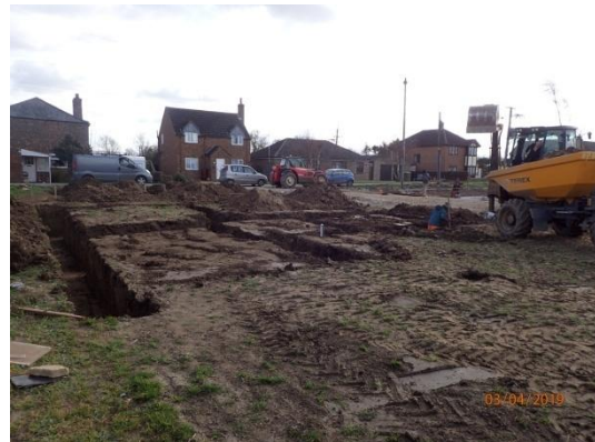
Plate 16: Excavation of the foundations, from the west
