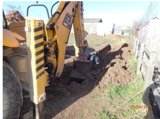
Plate 4: Excavation of the foundations, from the east
