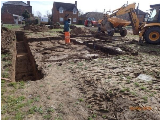
Plate 13: Excavation of the foundations, from the west
