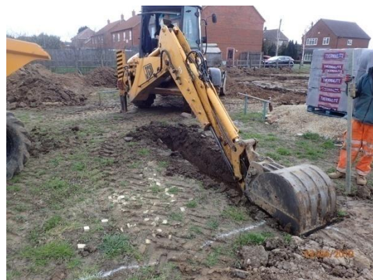
Plate 23: Excavation of the foundations, from the south
