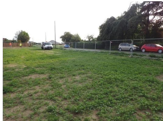
Plate 5: Pre-groundworks, from the south
