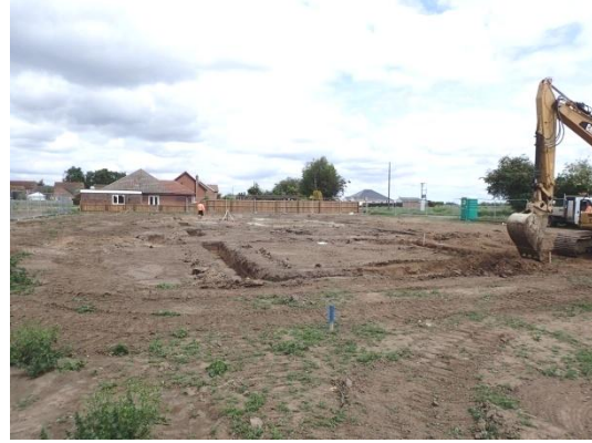
Plate 76: Excavation of the foundations, from the south
