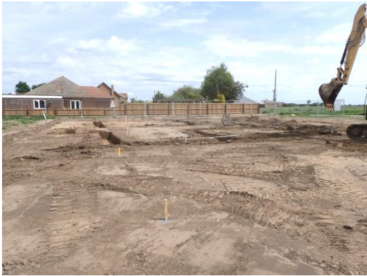
Plate 50: Excavation of the foundations, from the south
