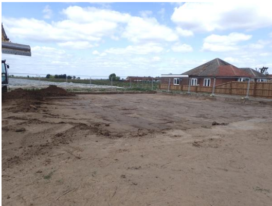
Plate 15: Initial ground reduction, from the south-east
