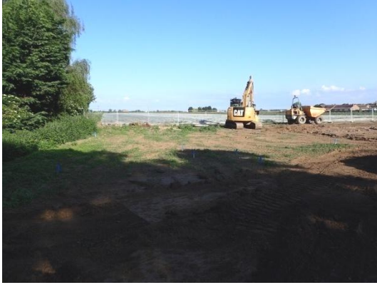
Plate 79: Pre-groundworks, from the east
