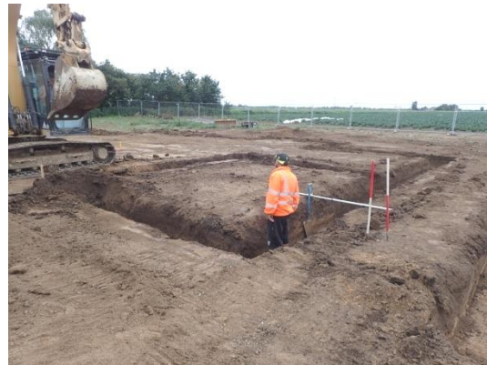
Plate 66: Excavation of the foundations, from the west
