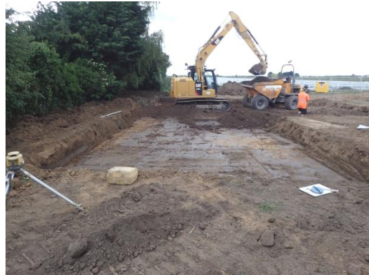
Plate 95: Second phase of mechanical ground reduction, from the east
