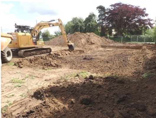
Plate 87: Initial phase of mechanical ground reduction, from the east
