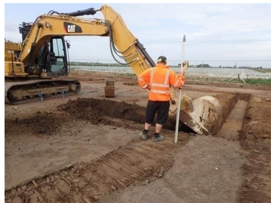
Plate 36: Excavation of the foundations, from the east
