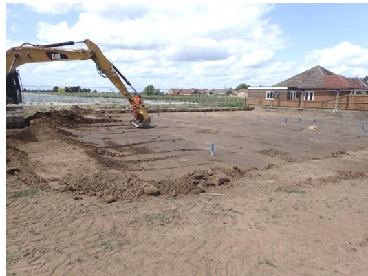
Plate 18: Initial ground reduction, from the east
