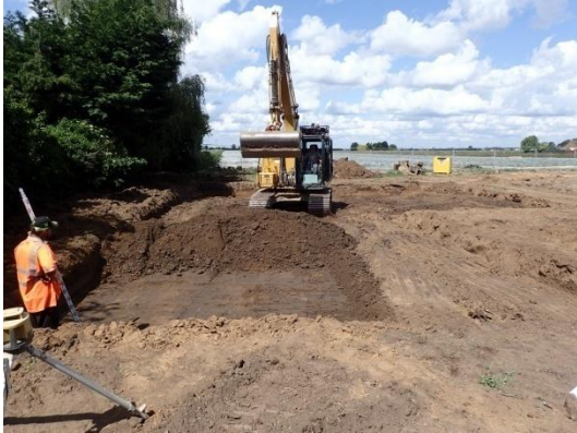
Plate 91: Second phase of mechanical ground reduction, from the east
