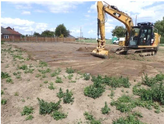
Plate 21: Initial ground reduction, from the south-west
