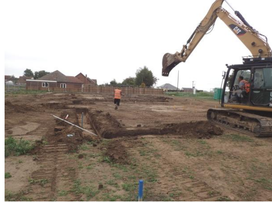
Plate 64: Excavation of the foundations, from the south
