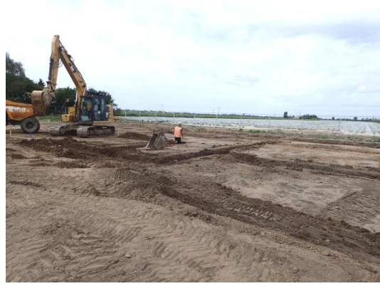
Plate 46: Excavation of the foundations, from the east
