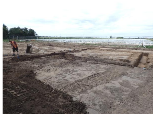
Plate 42: Excavation of the foundations, from the east
