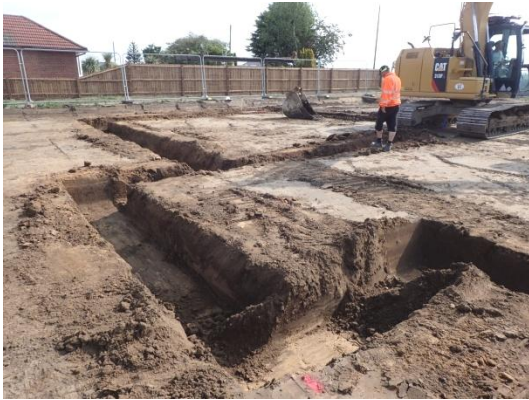
Plate 38: Excavation of the foundations, from the south
