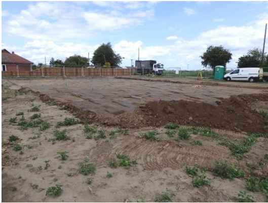
Plate 20: Initial ground reduction, from the south-west
