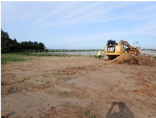
Plate 2: Pre-groundworks, from the east
