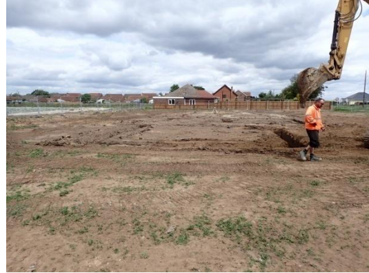
Plate 77: Excavation of the foundations, from the south
