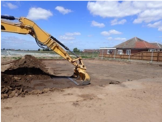
Plate 14: Initial ground reduction, from the east
