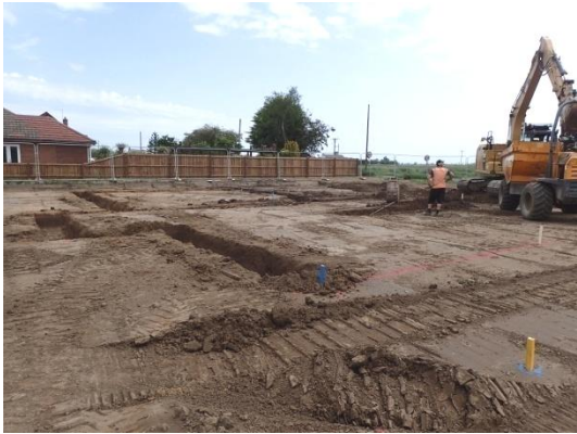
Plate 44: Excavation of the foundations, from the south
