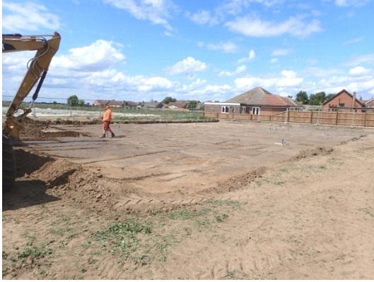
Plate 19: Initial ground reduction, from the south-east
