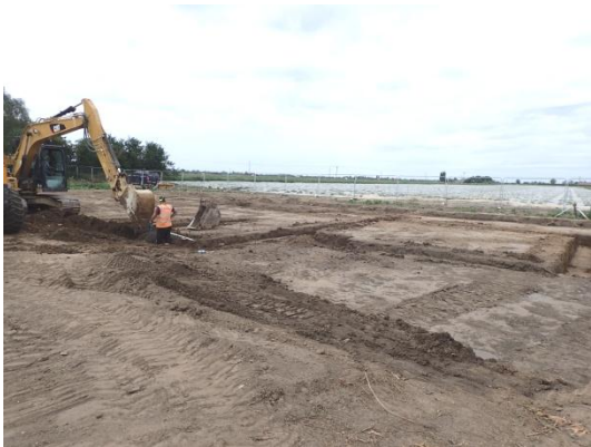
Plate 45: Excavation of the foundations, from the east
