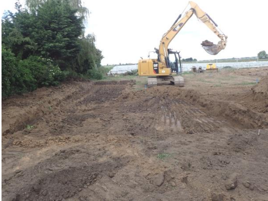
Plate 85: Initial phase of mechanical ground reduction, from the east
