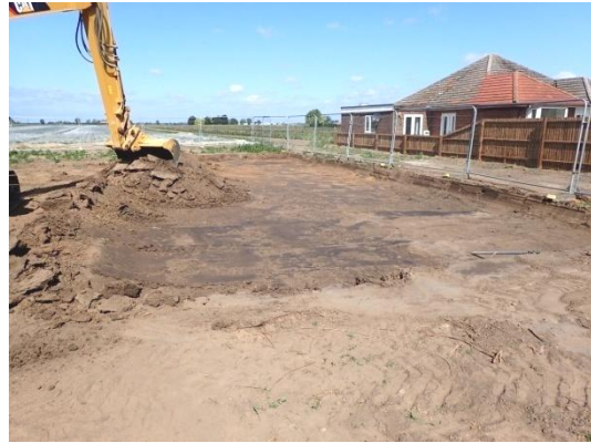
Plate 11: Initial ground reduction, from the east
