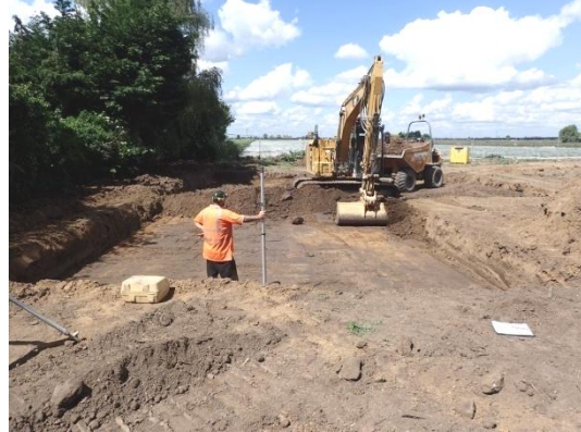
Plate 94: Second phase of mechanical ground reduction, from the east
