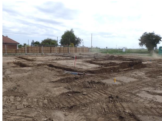
Plate 48: Excavation of the foundations, from the south
