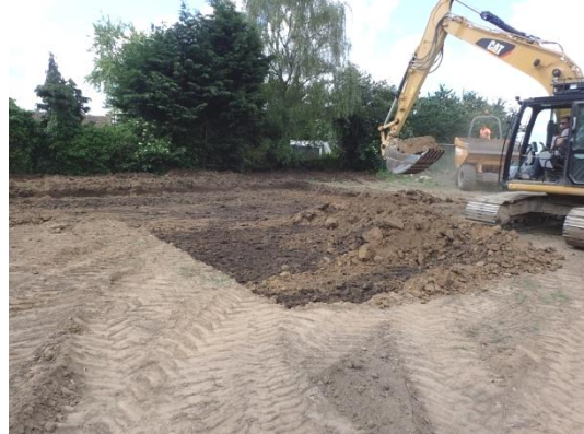
Plate 88: Initial phase of mechanical ground reduction, from the north
