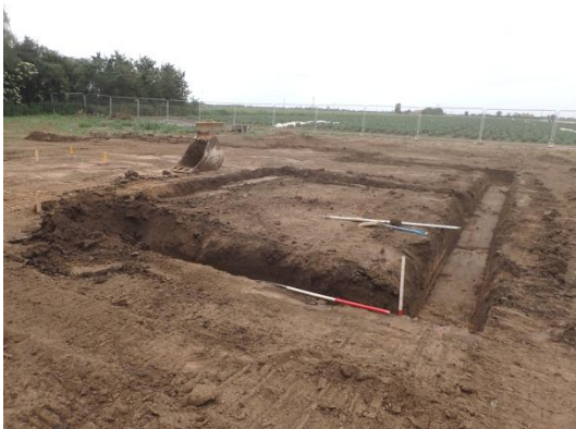
Plate 68: Excavation of the foundations, from the west
