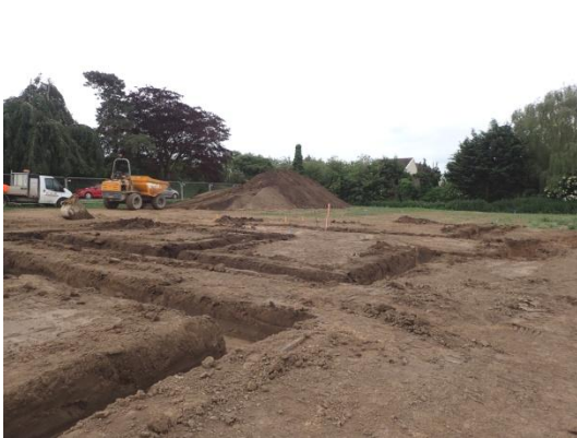
Plate 69: Excavation of the foundations, from the north-west
