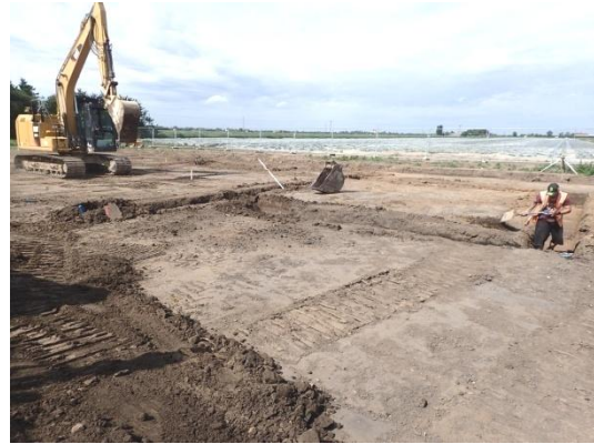
Plate 41: Excavation of the foundations, from the east
