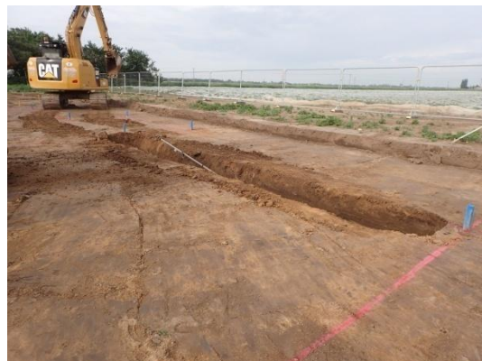
Plate 30: Excavation of the foundations, from the north
