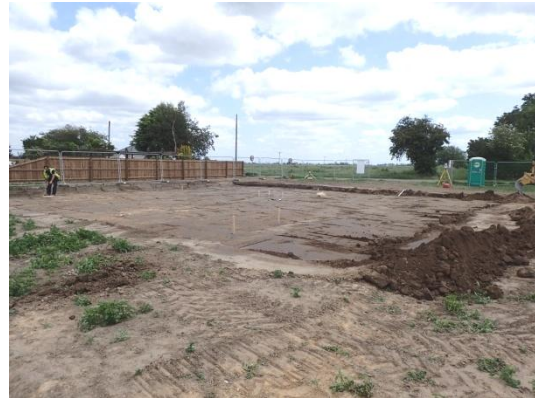
Plate 17: Initial ground reduction, from the west
