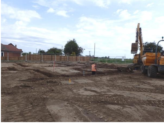
Plate 49: Excavation of the foundations, from the south
