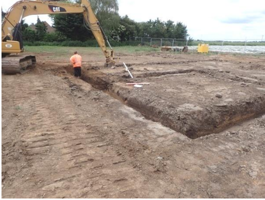
Plate 73: Excavation of the foundations, from the north-east
