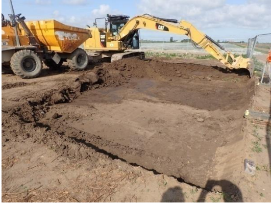
Plate 7: Initial ground reduction, from the east
