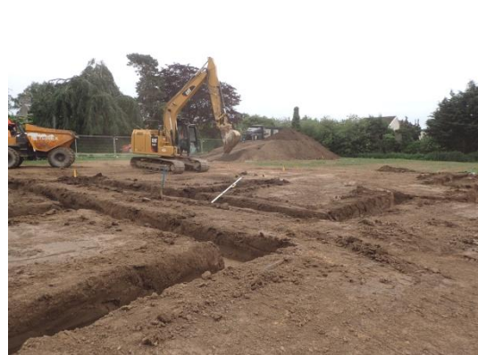
Plate 65: Excavation of the foundations, from the north-west
