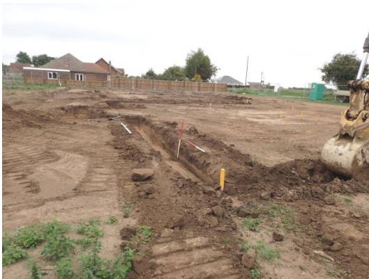
Plate 63: Excavation of the foundations, from the south
