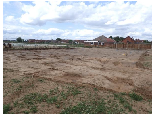
Plate 23: Initial ground reduction, from the south
