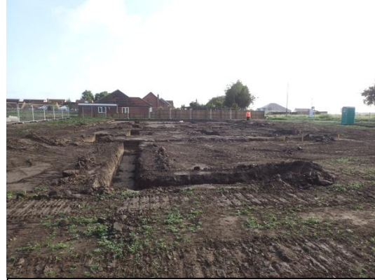
Plate 70: Excavation of the foundations, from the south
