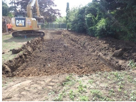
Plate 82: Initial phase of mechanical ground reduction, from the west
