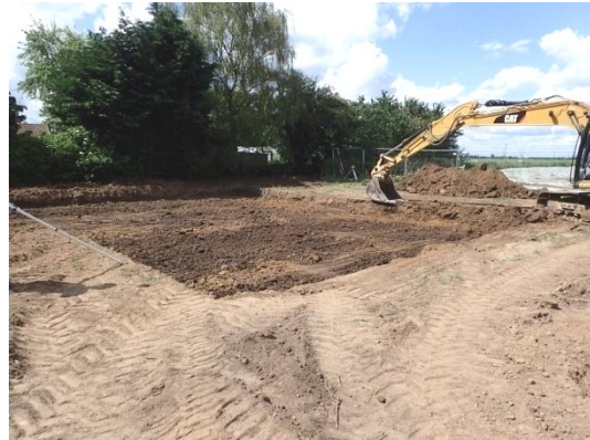
Plate 89: Initial phase of mechanical ground reduction, from the north
