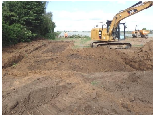
Plate 84: Initial phase of mechanical ground reduction, from the east
