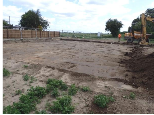
Plate 16: Initial ground reduction, from the west
