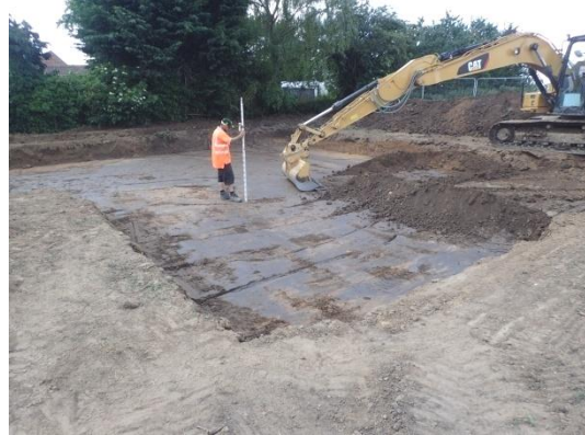
Plate 100: Second phase of mechanical ground reduction, from the north
