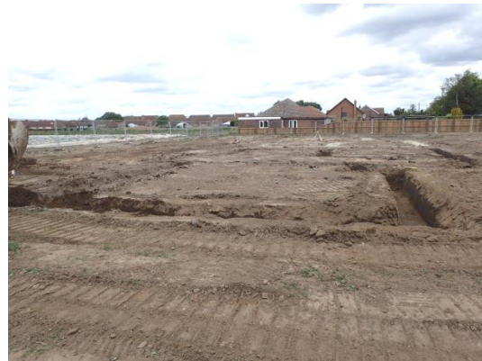
Plate 78: Excavation of the foundations, from the south
