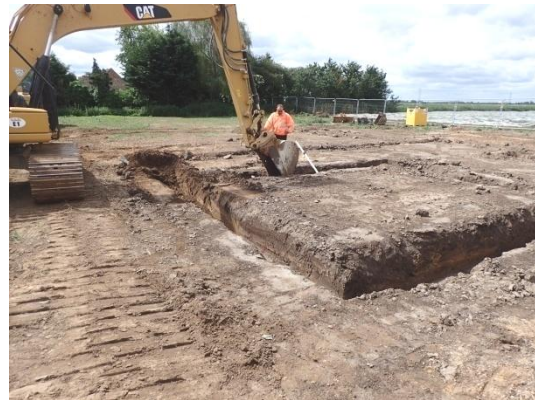
Plate 71: Excavation of the foundations, from the north
