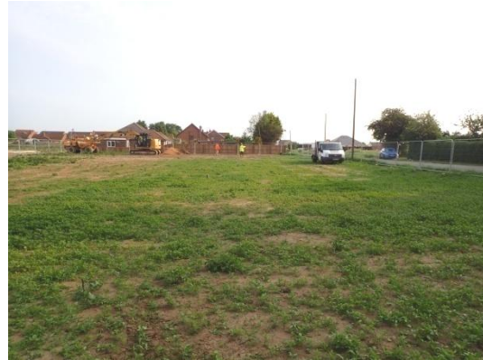
Plate 4: Pre-groundworks, from the south
