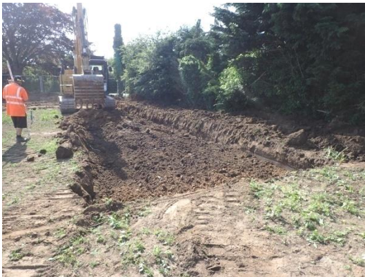
Plate 81: Initial phase of mechanical ground reduction, from the west
