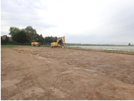
Plate 25: Completed ground reduction, from the north-east
