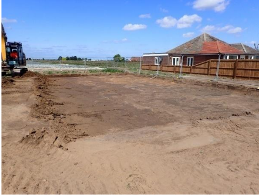
Plate 13: Initial ground reduction, from the east
