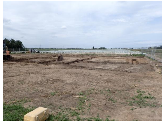
Plate 53: Excavation of the foundations, from the east
