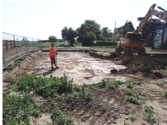
Plate 12: Initial ground reduction, from the west
