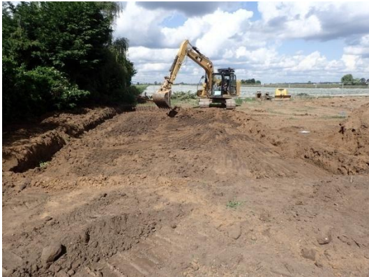
Plate 86: Initial phase of mechanical ground reduction, from the east
