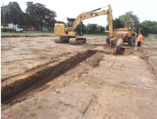
Plate 33: Excavation of the foundations, from the north
