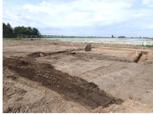
Plate 40: Excavation of the foundations, from the east
