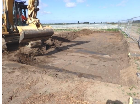
Plate 10: Initial ground reduction, from the east
