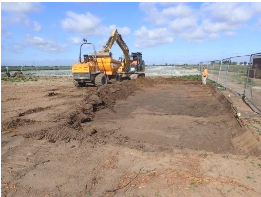
Plate 9: Initial ground reduction, from the east
