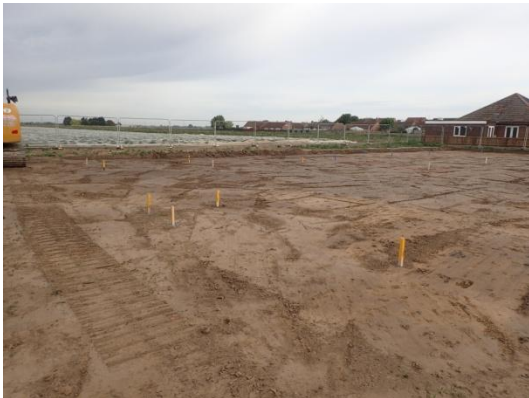
Plate 27: Completed ground reduction, from the east
