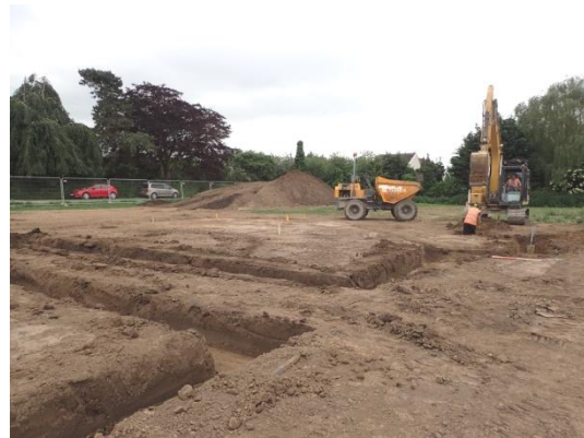
Plate 60: Excavation of the foundations, from the north-west
