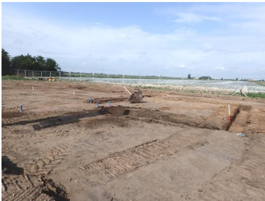
Plate 39: Excavation of the foundations, from the east
