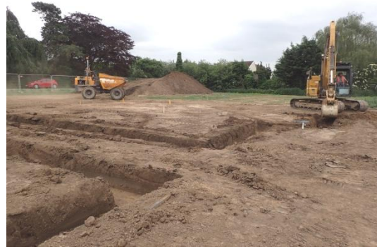
Plate 58: Excavation of the foundations, from the north-west
