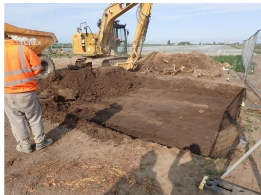
Plate 6: Initial ground reduction, from the east
