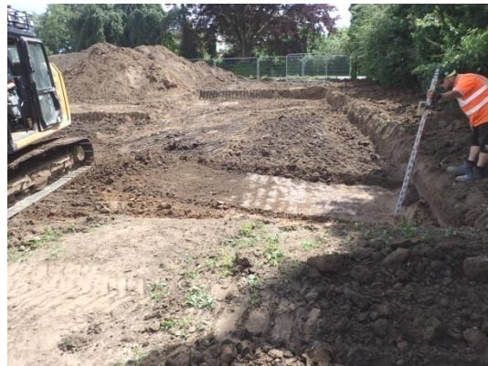
Plate 90: Second phase of mechanical ground reduction, from the west
