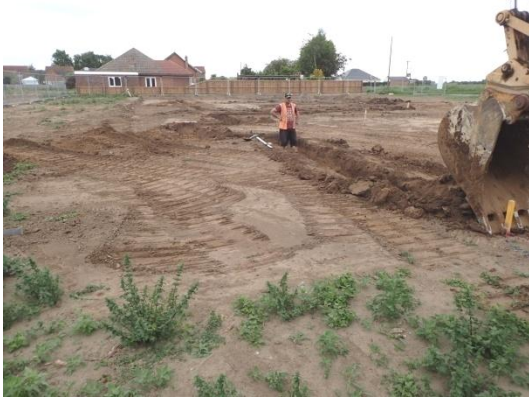
Plate 61: Excavation of the foundations, from the south
