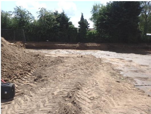
Plate 103: Second phase of mechanical ground reduction, from the north
