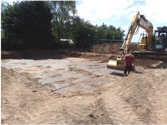
Plate 104: Second phase of mechanical ground reduction, from the north-east
