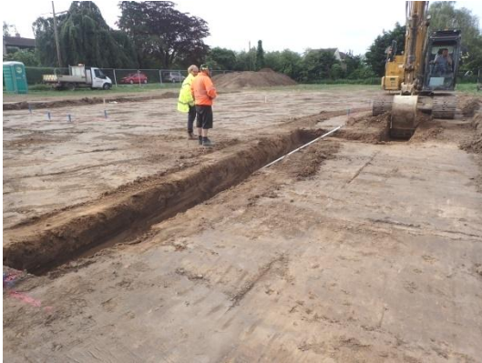
Plate 31: Excavation of the foundations, from the north
