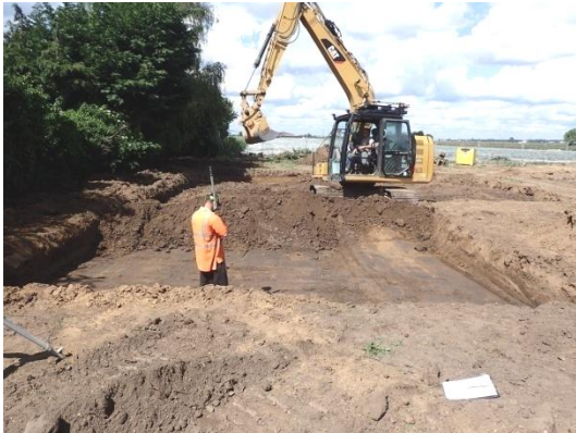
Plate 92: Second phase of mechanical ground reduction, from the east
