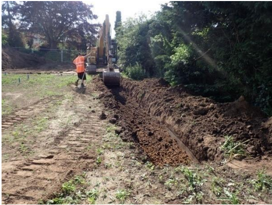
Plate 80: Initial phase of mechanical ground reduction, from the west
