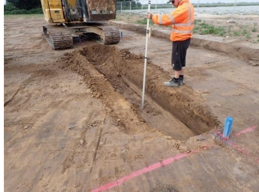
Plate 28: Excavation of the foundations, from the north
