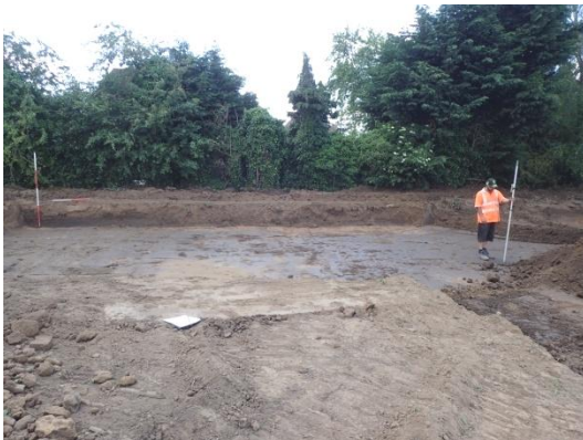
Plate 98: Second phase of mechanical ground reduction, from the north
