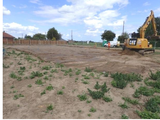
Plate 22: Initial ground reduction, from the south-west
