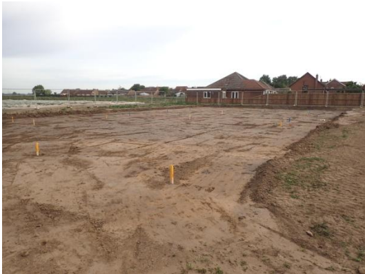
Plate 26: Completed ground reduction, from the south
