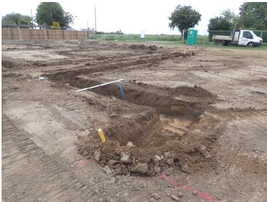
Plate 57: Excavation of the foundations, from the west
