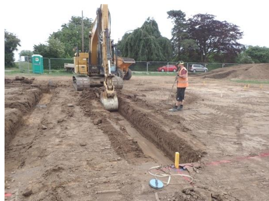
Plate 54: Excavation of the foundations, from the west
