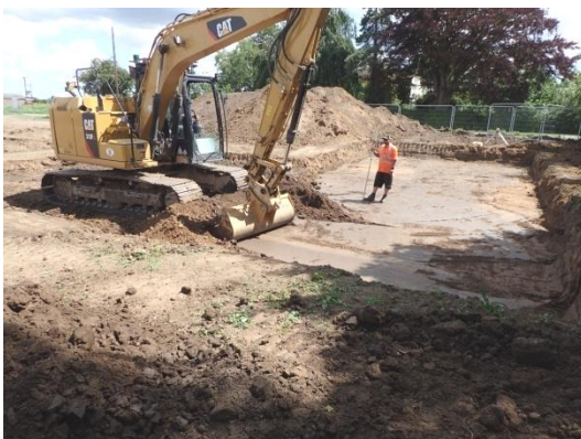
Plate 99: Second phase of mechanical ground reduction, from the west
