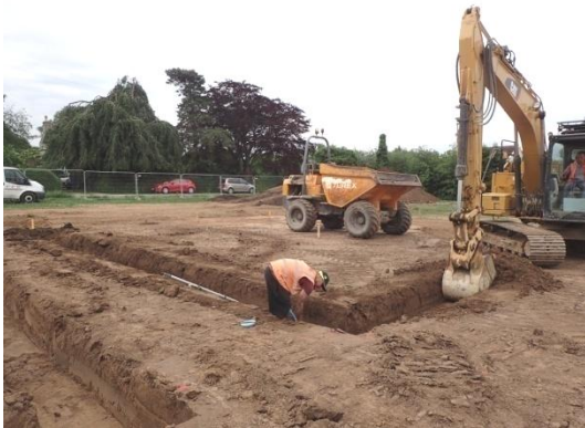
Plate 56: Excavation of the foundations, from the north-west
