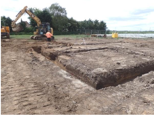
Plate 74: Excavation of the foundations, from the north-east
