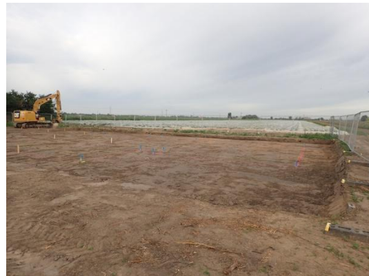
Plate 24: Completed ground reduction, from the east
