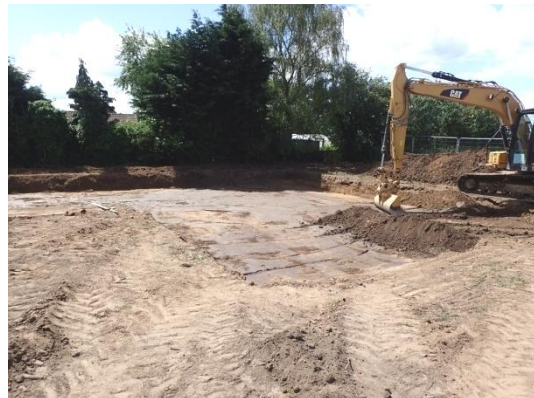
Plate 101: Second phase of mechanical ground reduction, from the north
