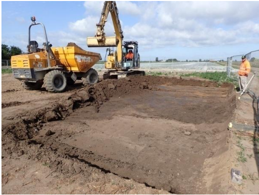
Plate 8: Initial ground reduction, from the east
