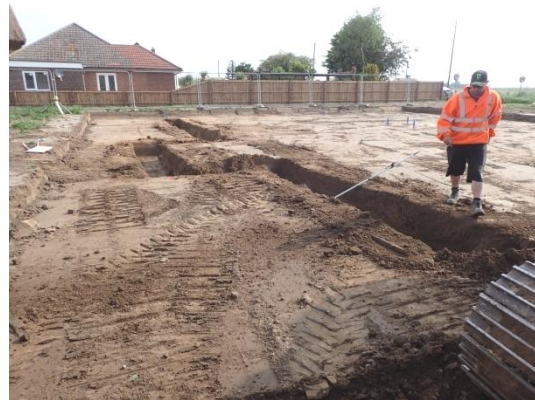
Plate 35: Excavation of the foundations, from the south
