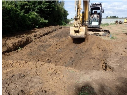
Plate 83: Initial phase of mechanical ground reduction, from the east
