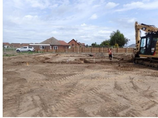
Plate 52: Excavation of the foundations, from the south
