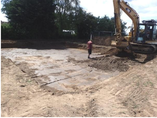
Plate 103: Second phase of mechanical ground reduction, from the north-east
