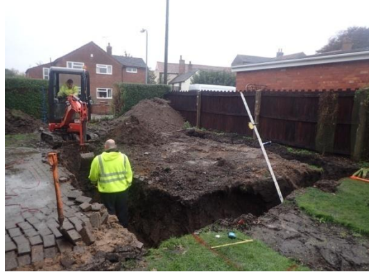
Plate 24: Excavation of the foundations, from the east
