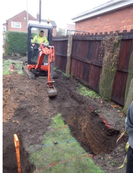
Plate 4: Excavation of the foundations, from the east
