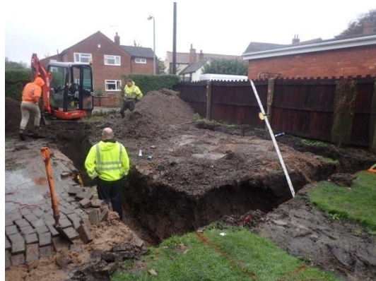
Plate 26: Excavation of the foundations, from the east
