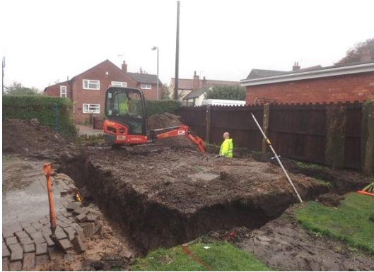
Plate 27: Excavation of the foundations, from the east
