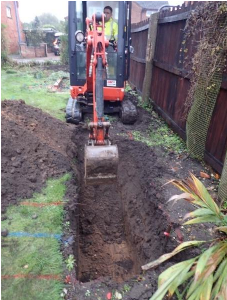
Plate 3: Excavation of the foundations, from the east
