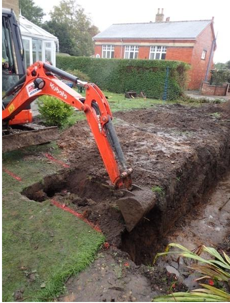
Plate 14: Excavation of the foundations, from the east
