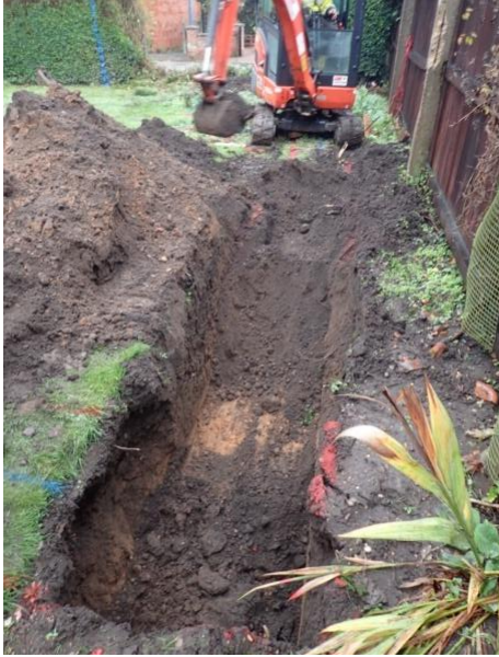
Plate 6: Excavation of the foundations, from the east
