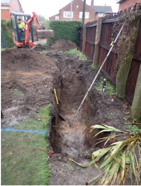
Plate 10: Excavation of the foundations, from the east
