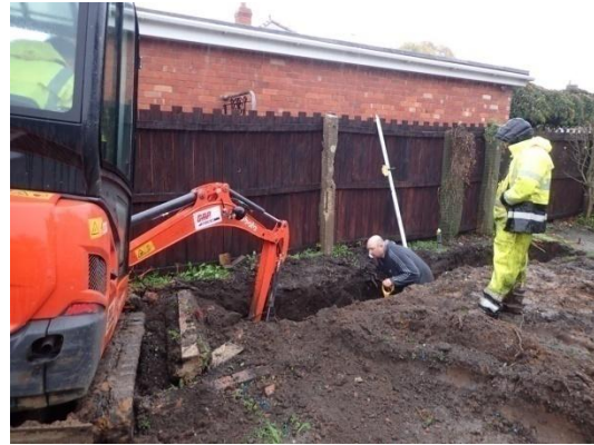
Plate 13: Excavation of the foundations, from the south
