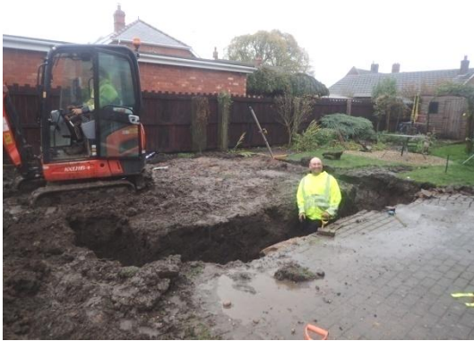
Plate 29: Excavation of the foundations, from the south
