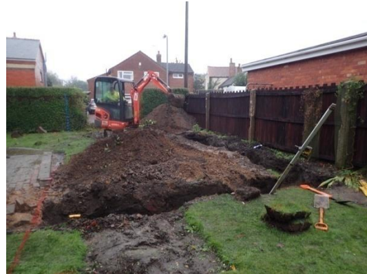
Plate 21: Excavation of the foundations, from the east
