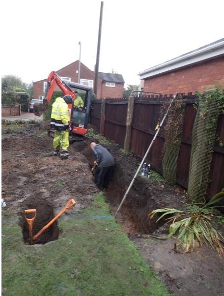
Plate 11: Excavation of the foundations, from the east
