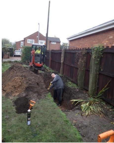
Plate 8: Excavation of the foundations, from the east
