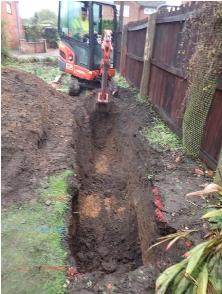
Plate 7: Excavation of the foundations, from the east
