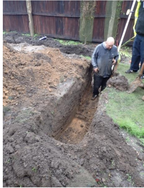
Plate 16: Excavation of the foundations, from the south
