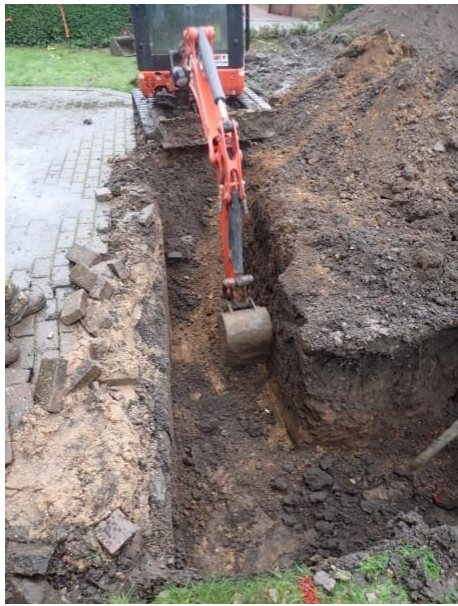
Plate 23: Excavation of the foundations, from the east
