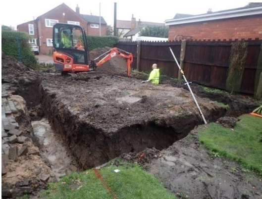
Plate 28: Excavation of the foundations, from the east
