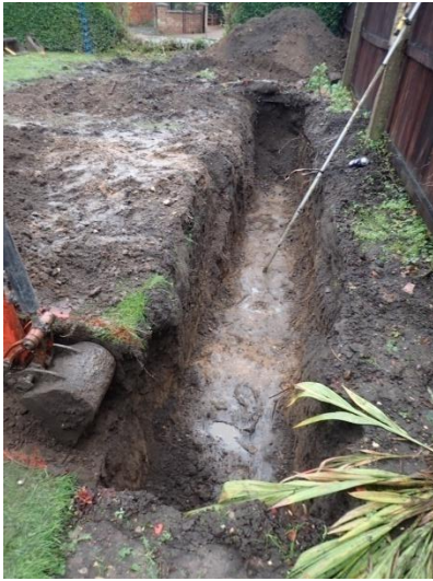
Plate 15: Excavation of the foundations, from the east
