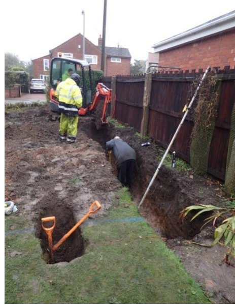
Plate 12: Excavation of the foundations, from the east
