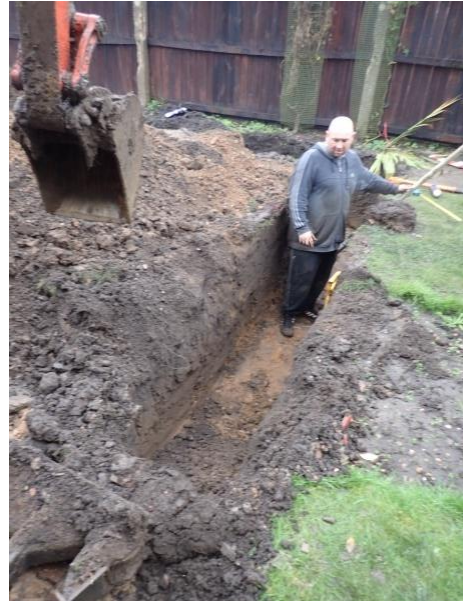
Plate 17: Excavation of the foundations, from the south
