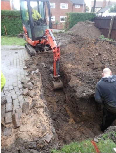
Plate 22: Excavation of the foundations, from the east
