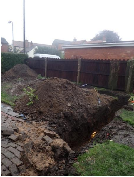
Plate 18: Excavation of the foundations, from the south
