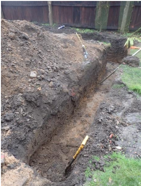
Plate 19: Excavation of the foundations, from the south
