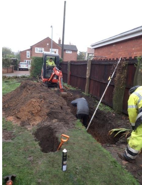
Plate 9: Excavation of the foundations, from the east
