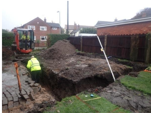
Plate 25: Excavation of the foundations, from the east
