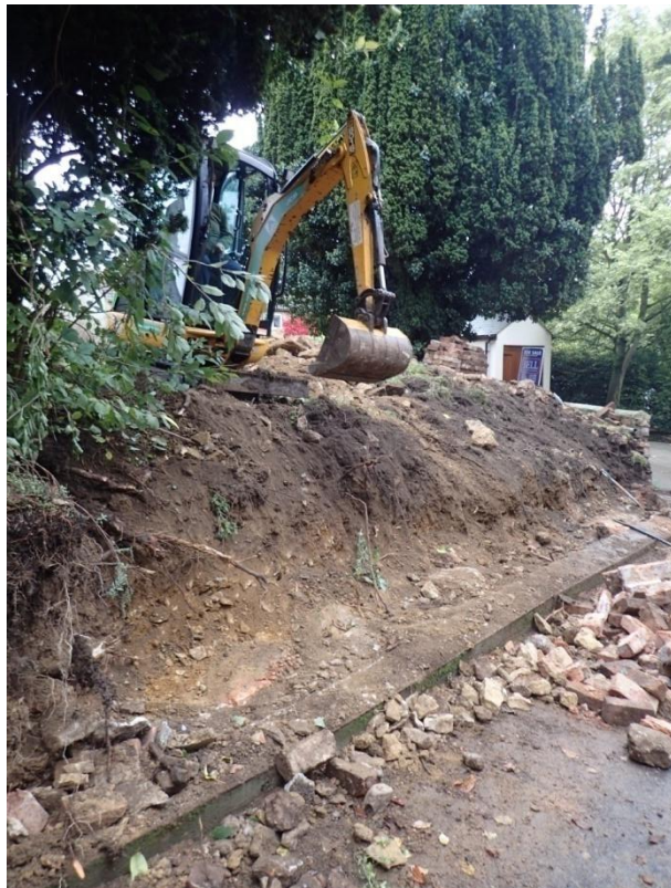
Plate 32: View of the mechanical removal of the earlier mid 19th century churchyard boundary wall, from the north-west
