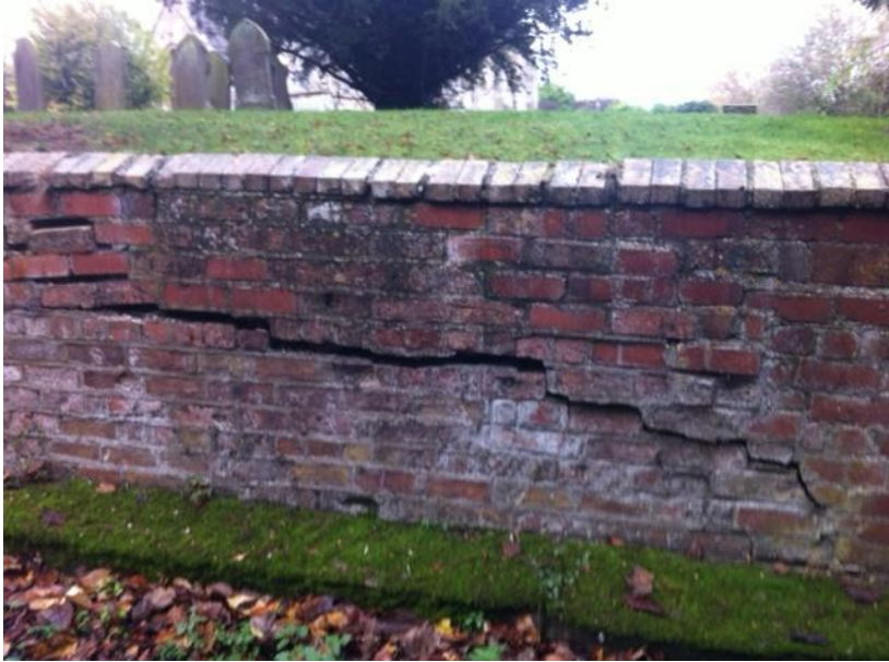
Plate 5: View of the churchyard boundary wall, pre-groundworks, from the west
