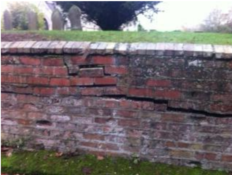
Plate 4: View of the churchyard boundary wall, pre-groundworks, from the west
