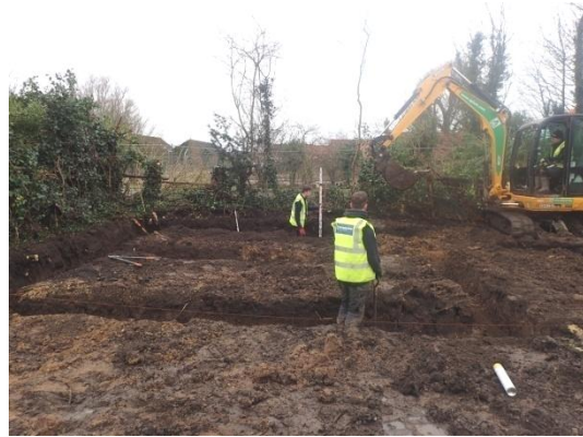
Plate 35: Excavation of the foundations, from the east
