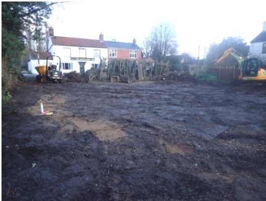
Plate 1: Pre-groundworks, from the south
