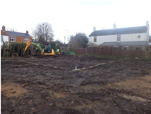
Plate 3: Set out foundations, from the south-west
