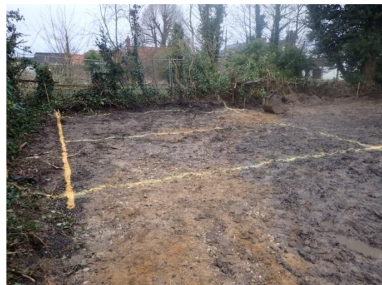
Plate 24: Set out foundations, from the east
