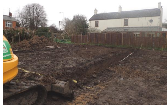
Plate 12: Excavation of the foundations, from the west
