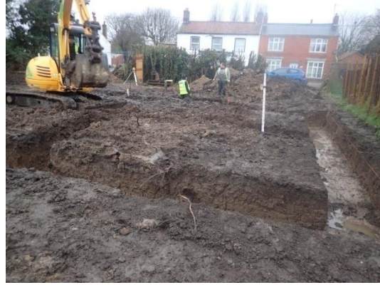
Plate 16: Excavation of the foundations, from the south
