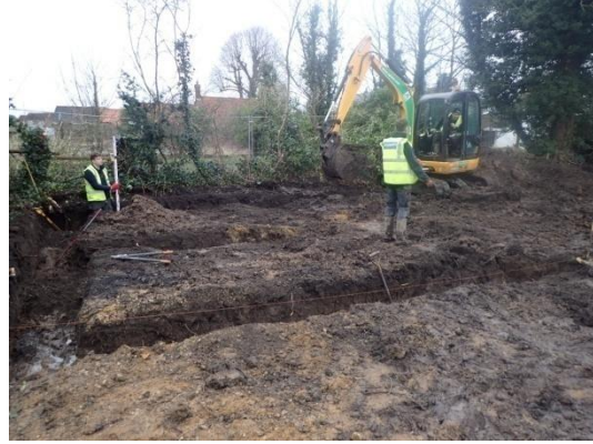
Plate 34: Excavation of the foundations, from the east
