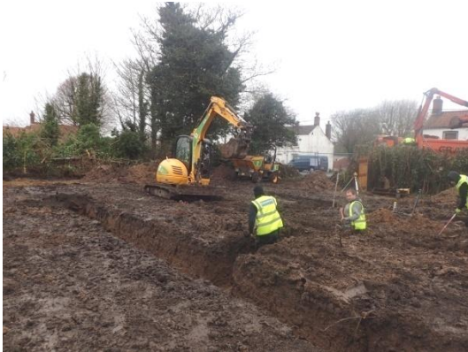
Plate 20: Excavation of the foundations, from the south-east
