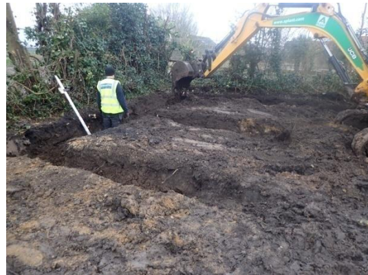
Plate 30: Excavation of the foundations, from the east
