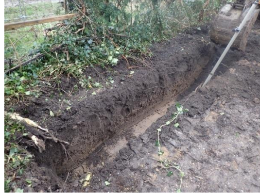
Plate 28: Excavation of the foundations, from the east
