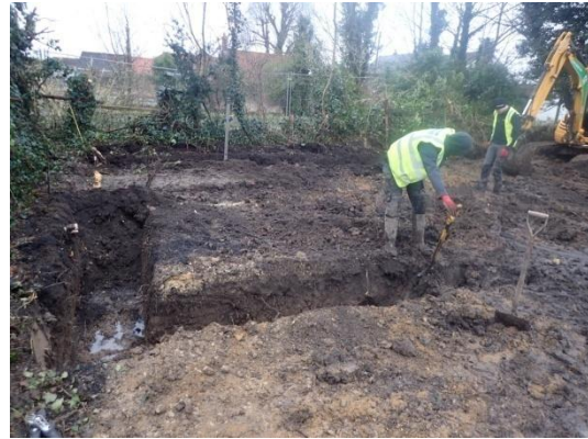
Plate 29: Excavation of the foundations, from the east
