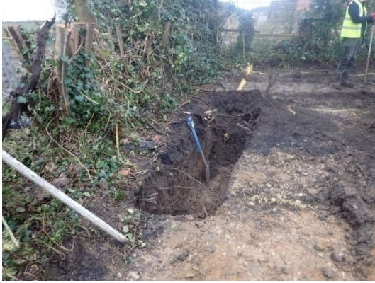
Plate 25: Excavation of the foundations, from the east
