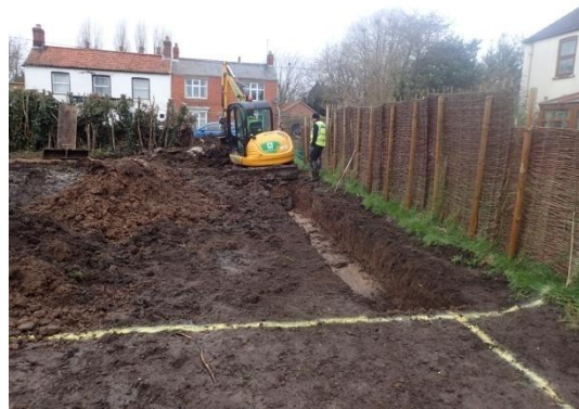
Plate 6: Excavation of the foundations, from the south
