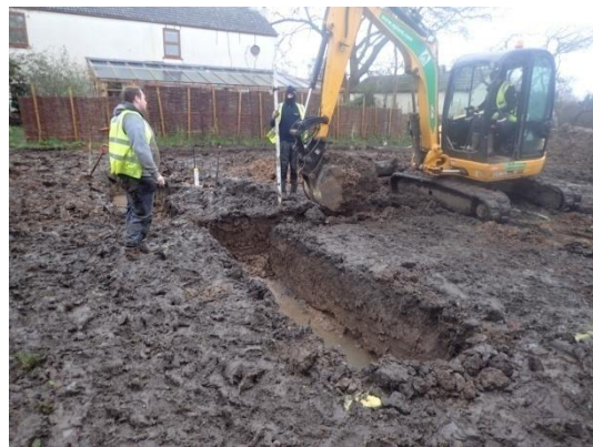
Plate 18: Excavation of the foundations, from the west
