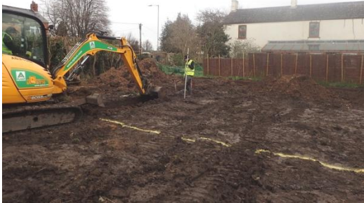
Plate 8: Excavation of the foundations, from the west
