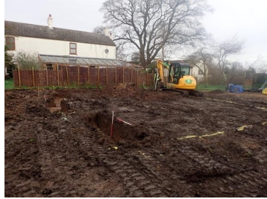
Plate 10: Excavation of the foundations, from the north-west
