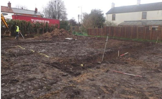
Plate 14: Excavation of the foundations, from the south-west
