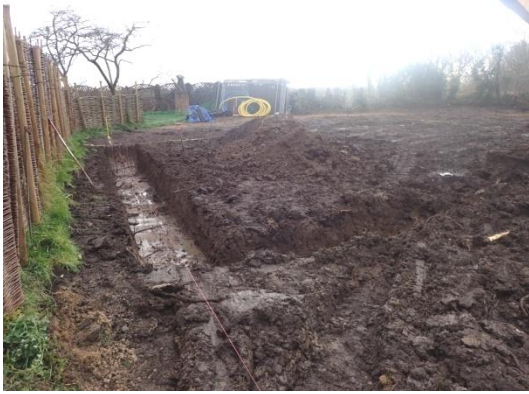
Plate 7: Excavation of the foundations, from the north
