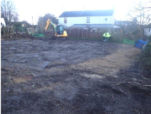
Plate 2: Pre-groundworks, from the west
