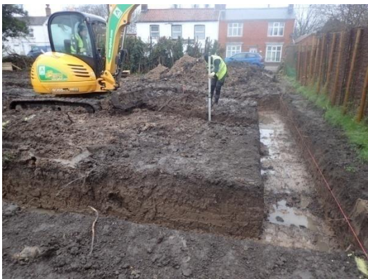
Plate 15: Excavation of the foundations, from the south
