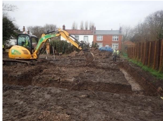
Plate 17: Excavation of the foundations, from the south
