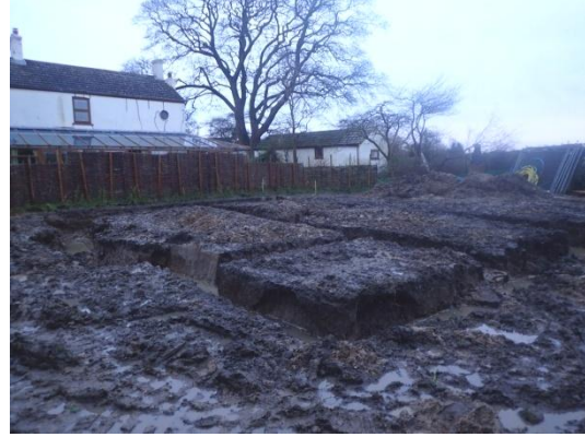
Plate 22: Completed bungalow plot, from the north-west
