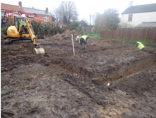
Plate 21: Excavation of the foundations, from the south
