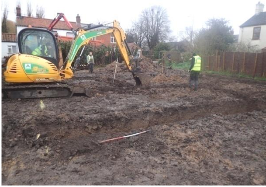
Plate 19: Excavation of the foundations, from the south
