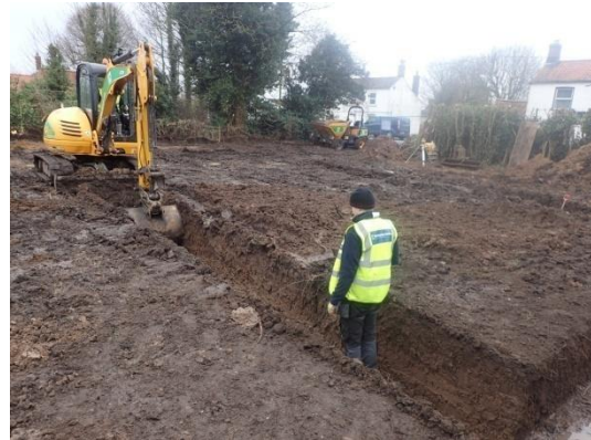
Plate 11: Excavation of the foundations, from the south-east
