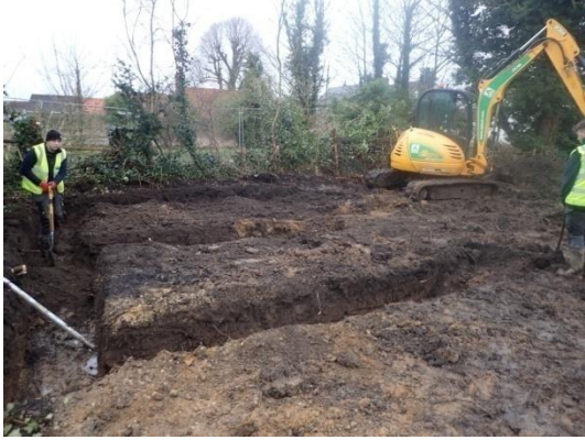
Plate 31: Excavation of the foundations, from the east
