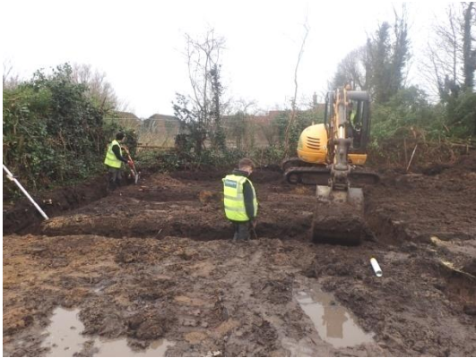
Plate 32: Excavation of the foundations, from the east
