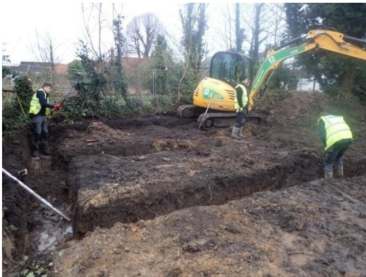
Plate 33: Excavation of the foundations, from the east
