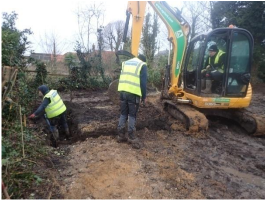
Plate 26: Excavation of the foundations, from the east
