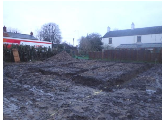
Plate 23: Completed bungalow plot, from the south-west
