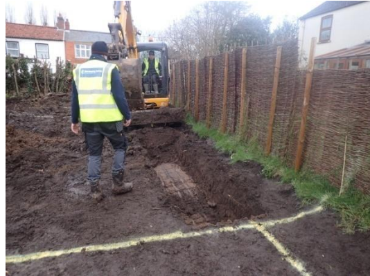
Plate 4: Excavation of the foundations, from the south
