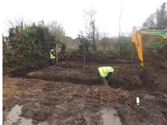
Plate 36: Excavation of the foundations, from the east
