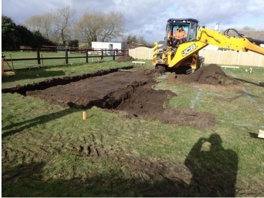
Plate 19: Excavation of the foundations, from the south
