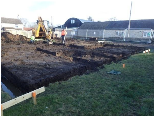
Plate 45: Excavation of the foundations, from the south-west
