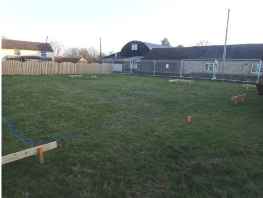
Plate 2: Pre-groundworks, from the south-west
