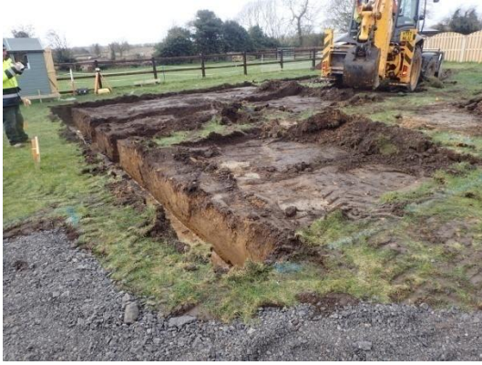
Plate 25: Excavation of the foundations, from the east
