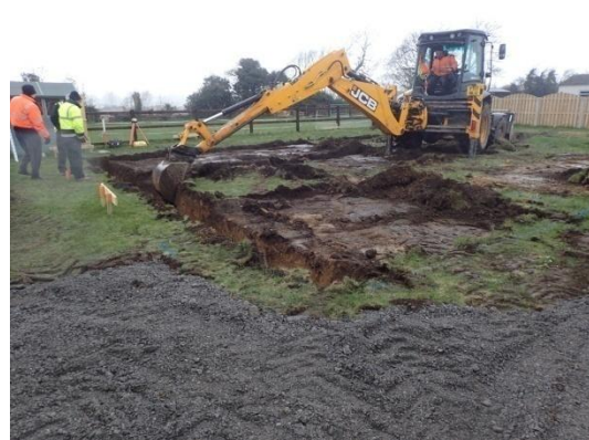
Plate 24: Excavation of the foundations, from the south-east
