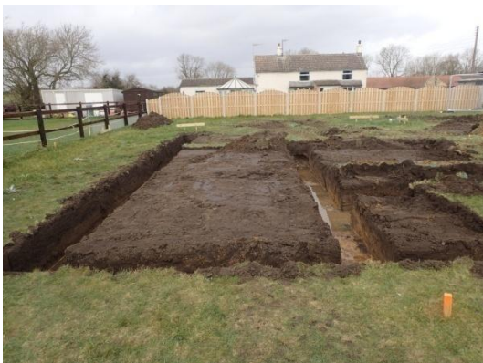
Plate 21: Excavation of the foundations, from the south
