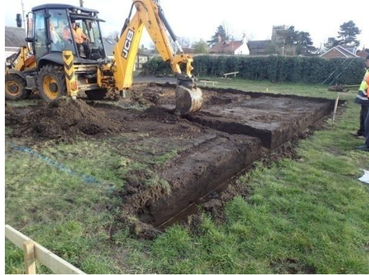
Plate 34: Excavation of the foundations, from the north
