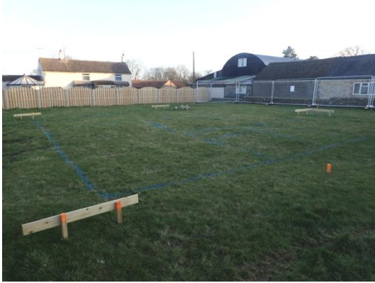
Plate 1: Pre-groundworks, from the south
