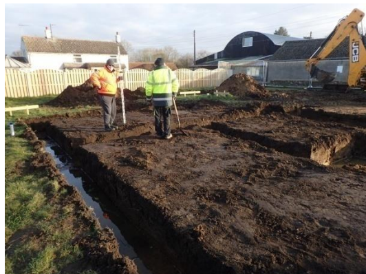
Plate 42: Excavation of the foundations, from the south
