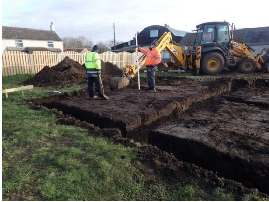
Plate 43: Excavation of the foundations, from the south-west
