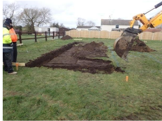
Plate 16: Excavation of the foundations, from the south
