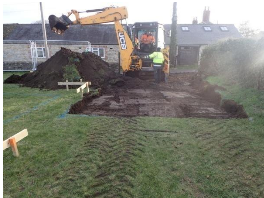
Plate 6: Ground reduction for the new site access, from the west
