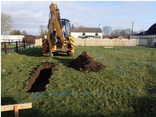
Plate 8: Excavation of the foundations, from the south
