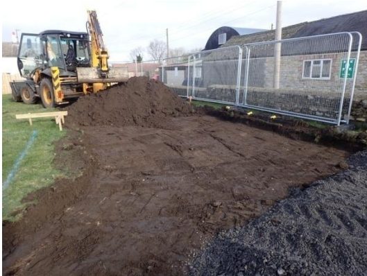
Plate 14: Ground reduction for the new site access, from the south
