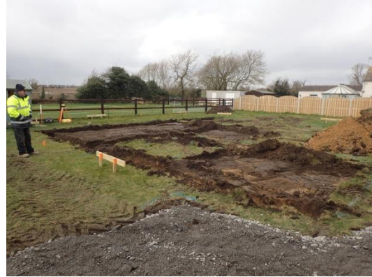
Plate 22: Excavation of the foundations, from the south-east
