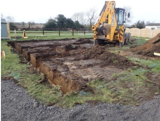
Plate 26: Excavation of the foundations, from the east
