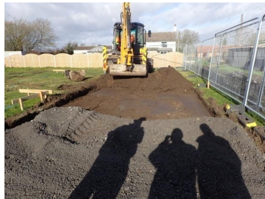
Plate 18: Ground reduction for the new site access, from the south
