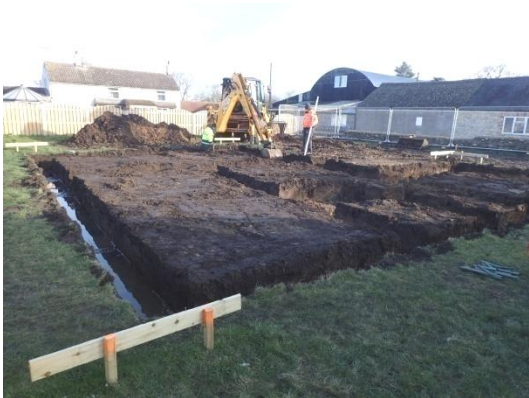
Plate 44: Excavation of the foundations, from the south
