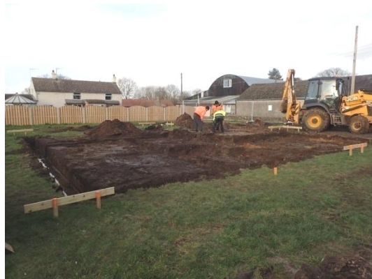
Plate 36: Excavation of the foundations, from the south
