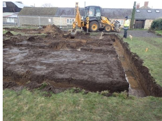
Plate 30: Excavation of the foundations, from the west
