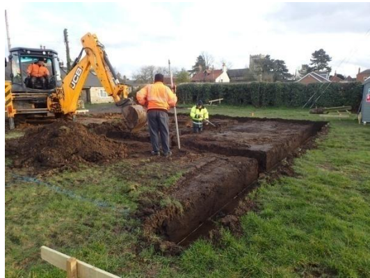
Plate 35: Excavation of the foundations, from the north
