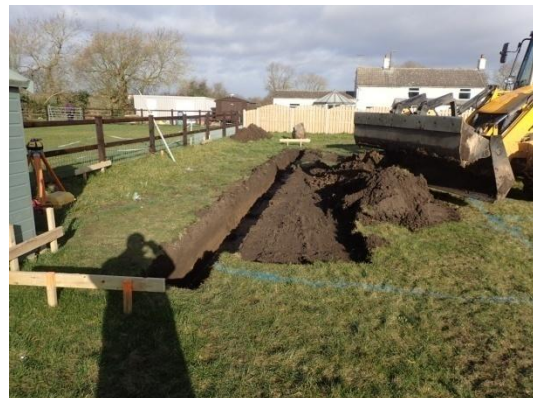
Plate 12: Excavation of the foundations, from the south
