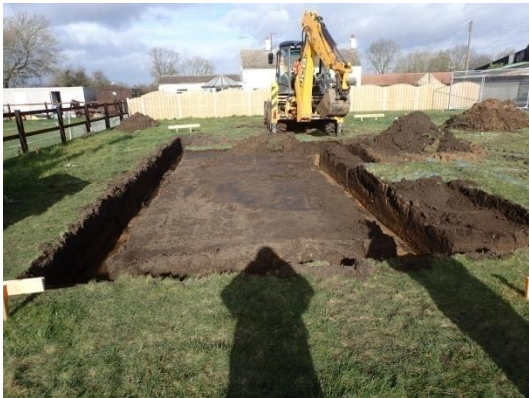
Plate 20: Excavation of the foundations, from the south
