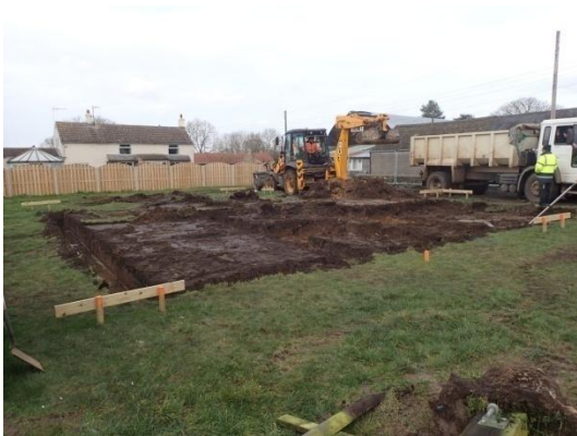
Plate 33: Excavation of the foundations, from the south
