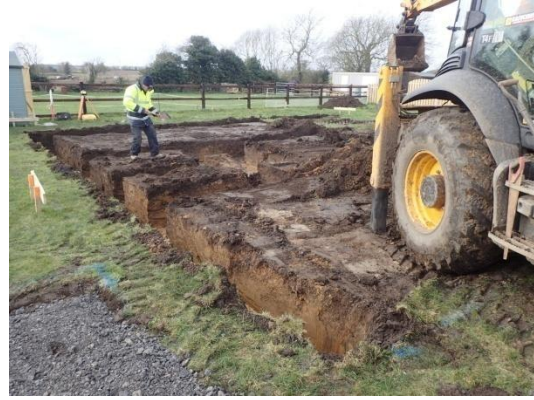
Plate 28: Excavation of the foundations, from the east
