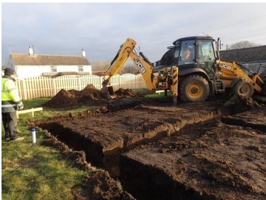
Plate 39: Excavation of the foundations, from the south-west
