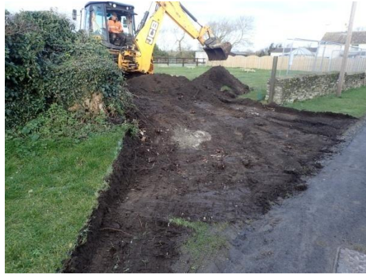
Plate 4: Ground reduction for the new site access, from the south-east
