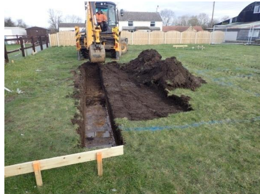
Plate 11: Excavation of the foundations, from the south
