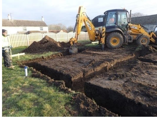
Plate 40: Excavation of the foundations, from the south-west
