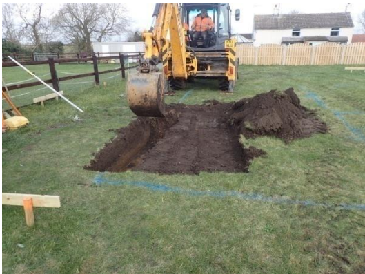
Plate 9: Excavation of the foundations, from the south
