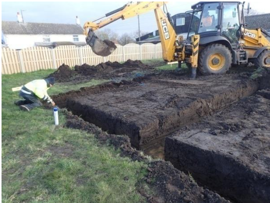
Plate 38: Excavation of the foundations, from the south-west
