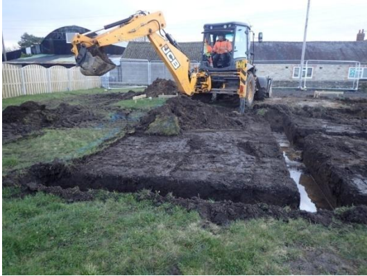
Plate 37: Excavation of the foundations, from the west
