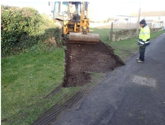
Plate 3: Ground reduction for the new site access, from the south-east
