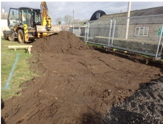
Plate 15: Ground reduction for the new site access, from the south
