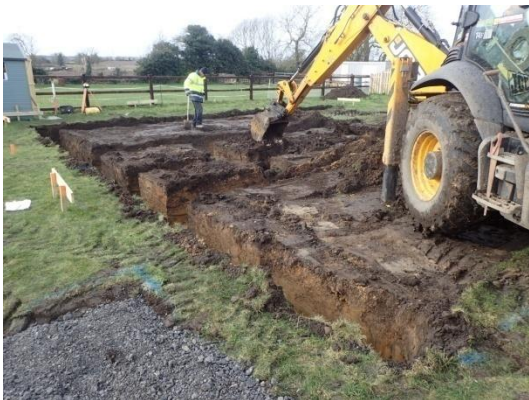
Plate 27: Excavation of the foundations, from the east
