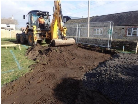
Plate 13: Ground reduction for the new site access, from the south-west
