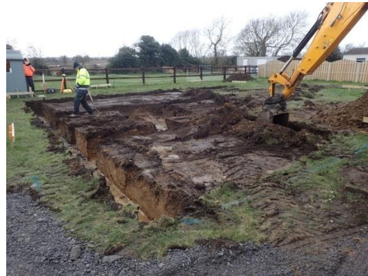
Plate 29: Excavation of the foundations, from the east
