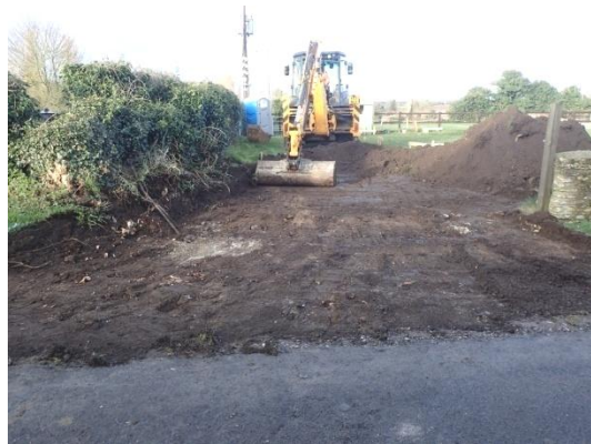
Plate 5: Ground reduction for the new site access, from the east
