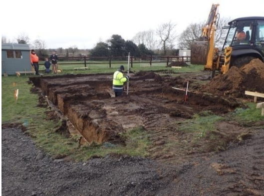
Plate 32: Excavation of the foundations, from the east
