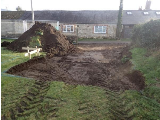
Plate 7: Ground reduction for the new site access, from the west
