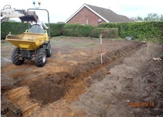
Plate 11: Excavation of the foundations, from the south
