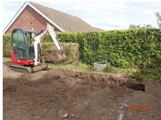
Plate 4: Excavation of the foundations, from the south
