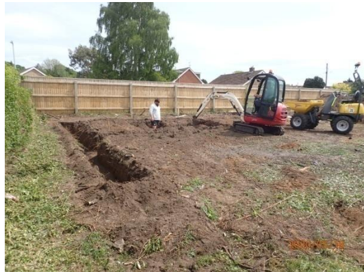
Plate 17: Excavation of the foundations, from the west
