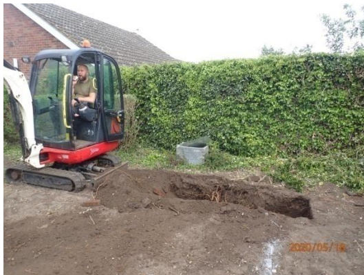
Plate 3: Excavation of the foundations, from the south
