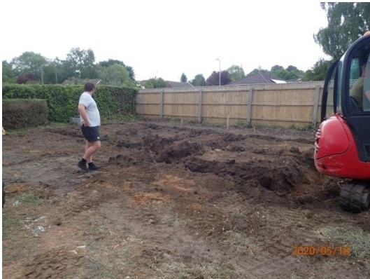
Plate 26: Excavation of the foundations, from the west
