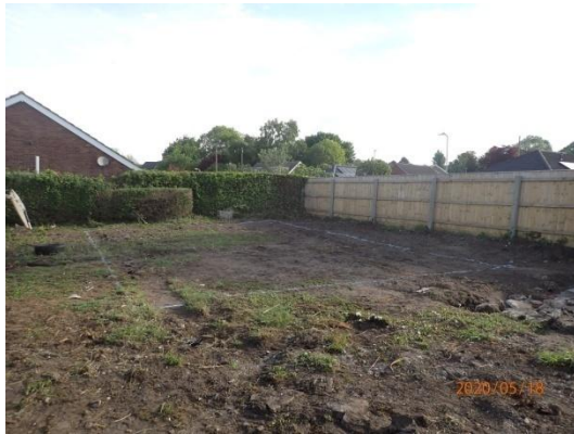
Plate 1: Pre-groundworks, from the south
