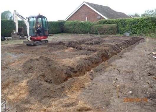
Plate 20: Excavation of the foundations, from the south
