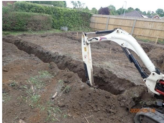
Plate 29: Excavation of the foundations, from the south-west
