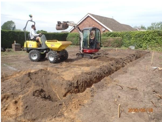
Plate 15: Excavation of the foundations, from the south
