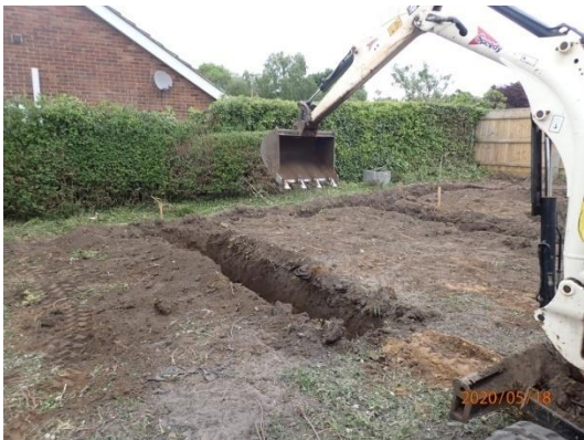
Plate 27: Excavation of the foundations, from the south
