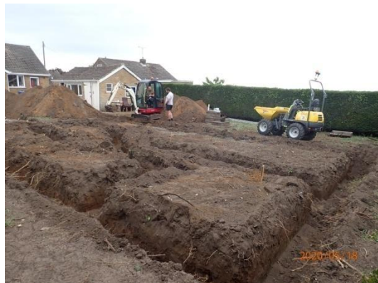
Plate 30: Excavation of the foundations, from the north-east
