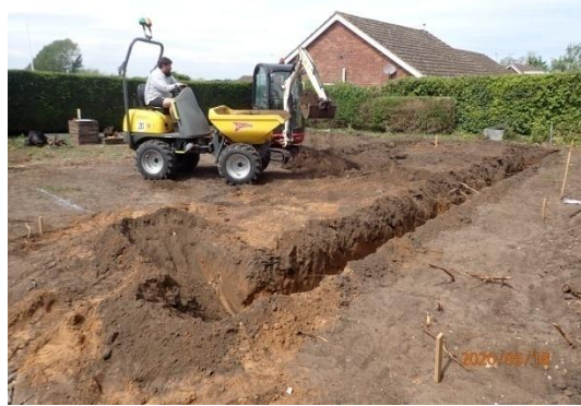
Plate 16: Excavation of the foundations, from the south
