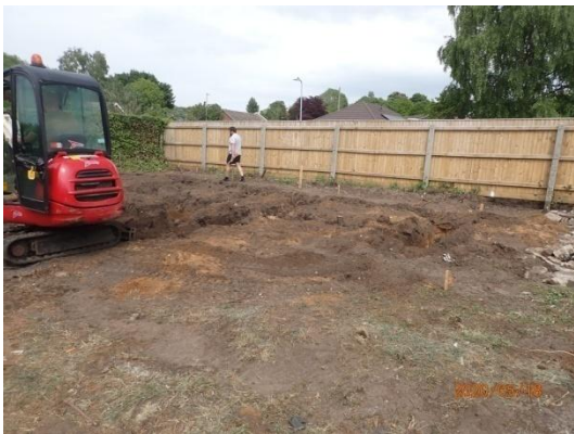
Plate 21: Excavation of the foundations, from the west
