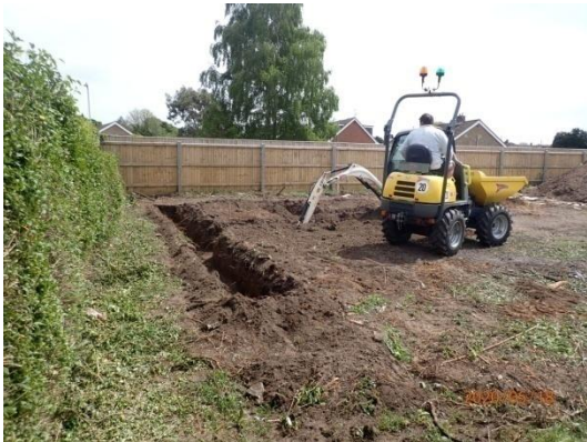
Plate 14: Excavation of the foundations, from the west
