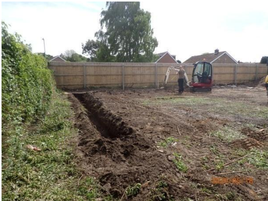
Plate 8: Excavation of the foundations, from the west
