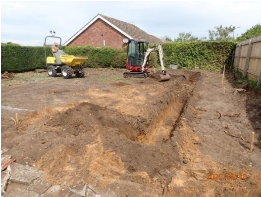
Plate 12: Excavation of the foundations, from the south
