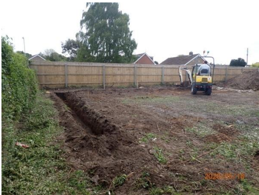
Plate 9: Excavation of the foundations, from the west
