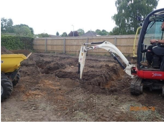
Plate 25: Excavation of the foundations, from the west
