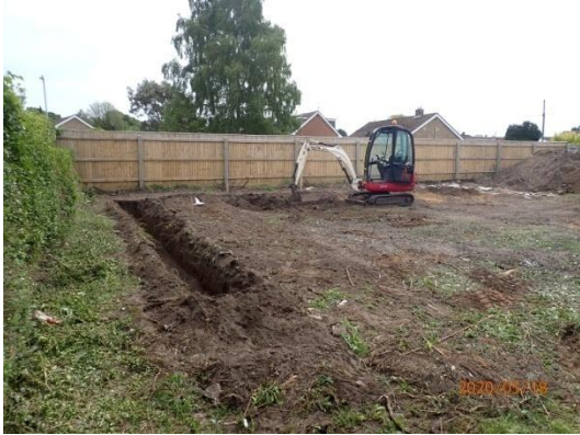
Plate 13: Excavation of the foundations, from the west
