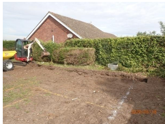
Plate 6: Excavation of the foundations, from the south
