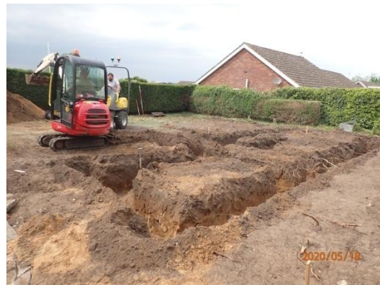
Plate 24: Excavation of the foundations, from the south
