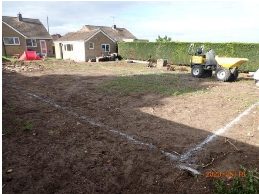
Plate 2: Pre-groundworks, from the north-east
