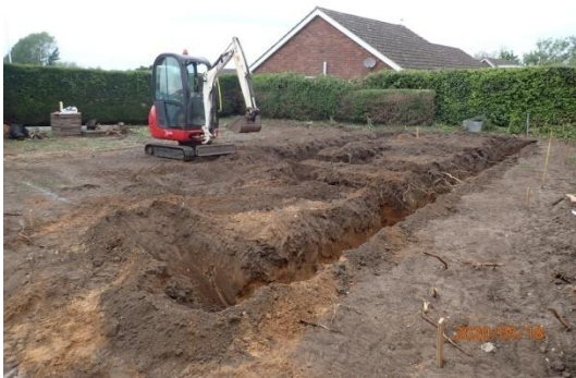
Plate 19: Excavation of the foundations, from the south
