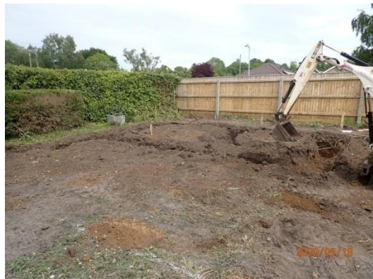
Plate 18: Excavation of the foundations, from the west
