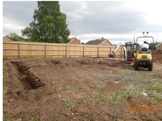
Plate 23: Excavation of the foundations, from the west
