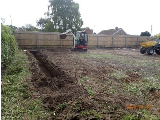
Plate 7: Excavation of the foundations, from the west
