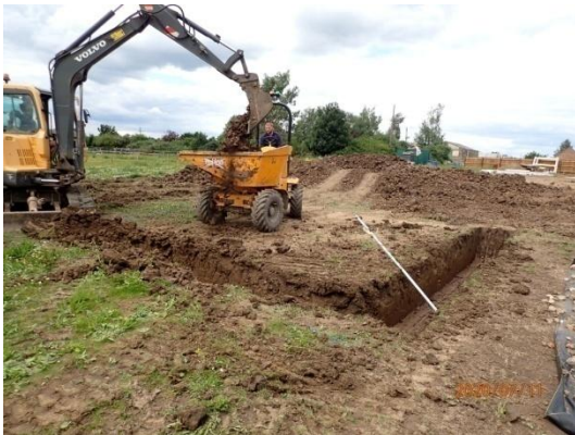
Plate 38: Excavation of the foundations, from the west
