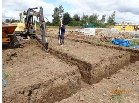
Plate 22: Excavation of the foundations, from the south-east
