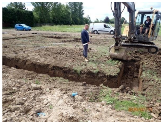
Plate 18: Excavation of the foundations, from the north
