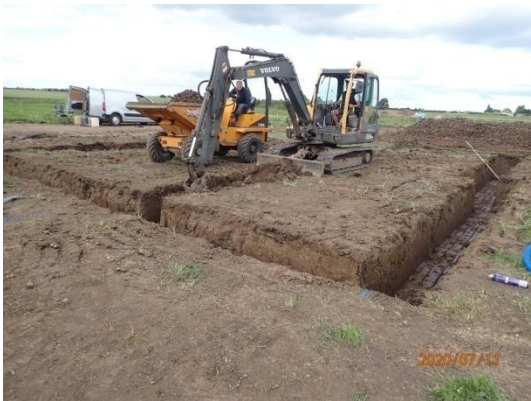
Plate 21: Excavation of the foundations, from the north-east
