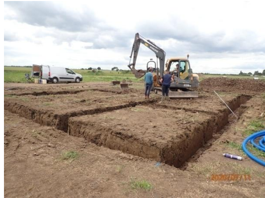
Plate 23: Excavation of the foundations, from the north-east
