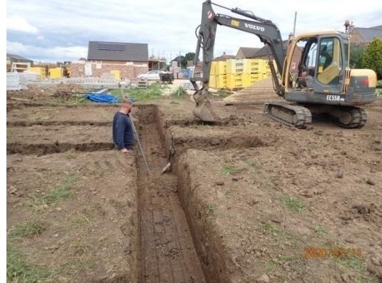
Plate 34: Excavation of the foundations, from the south
