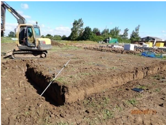
Plate 9: Excavation of the foundations, from the south-east
