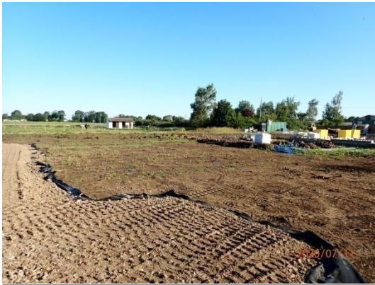
Plate 1: Pre-groundworks, from the south-east
