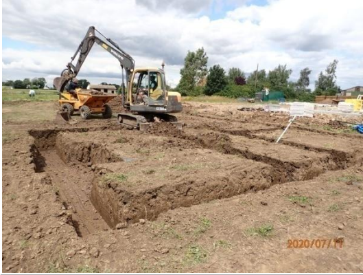
Plate 25: Excavation of the foundations, from the south-east
