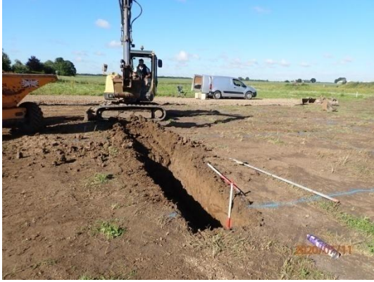
Plate 7: Excavation of the foundations, from the east
