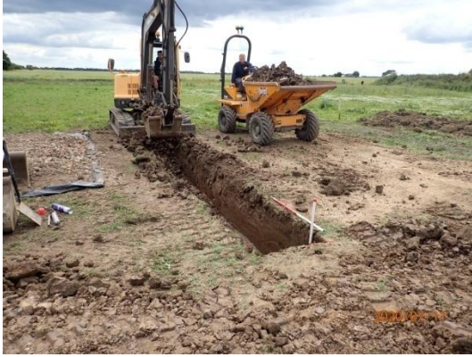
Plate 37: Excavation of the foundations, from the north-east
