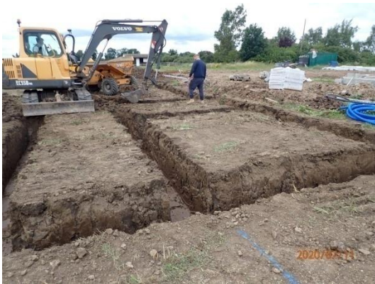
Plate 26: Excavation of the foundations, from the east
