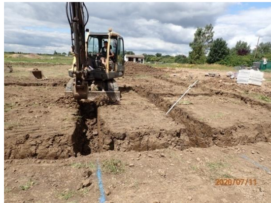
Plate 24: Excavation of the foundations, from the east
