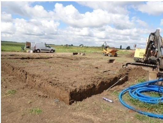
Plate 14: Excavation of the foundations, from the north-east
