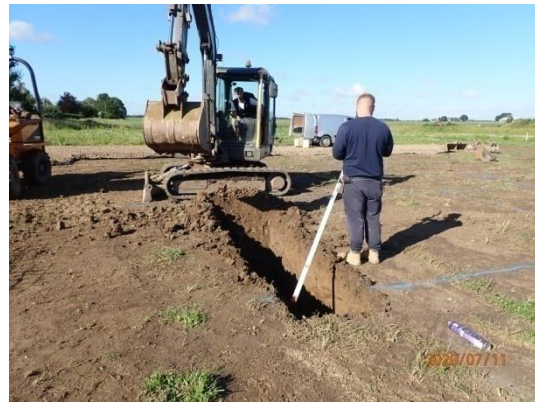
Plate 5: Excavation of the foundations, from the east
