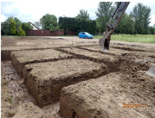
Plate 27: Excavation of the foundations, from the north
