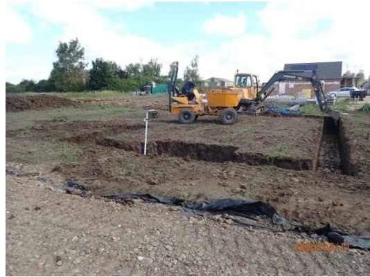
Plate 11: Excavation of the foundations, from the south
