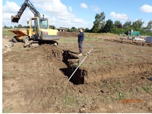
Plate 10: Excavation of the foundations, from the east
