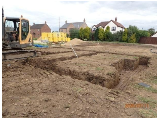
Plate 29: Excavation of the foundations, from the south-west
