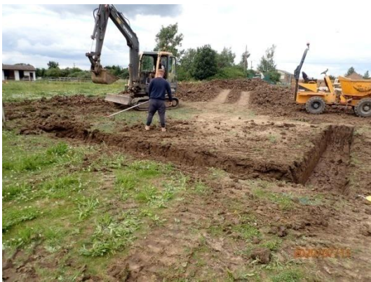
Plate 39: Excavation of the foundations, from the west
