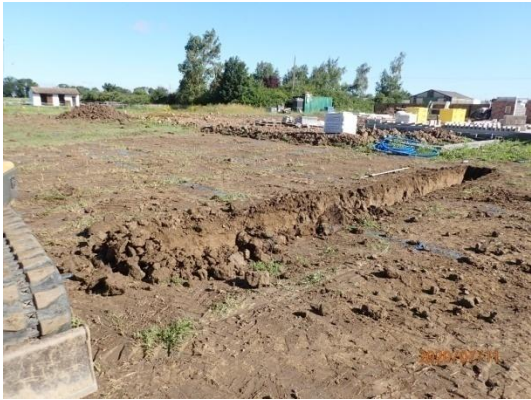
Plate 8: Excavation of the foundations, from the south-west
