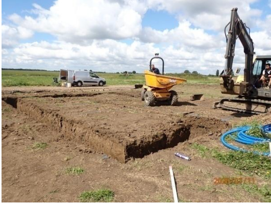
Plate 13: Excavation of the foundations, from the north-east
