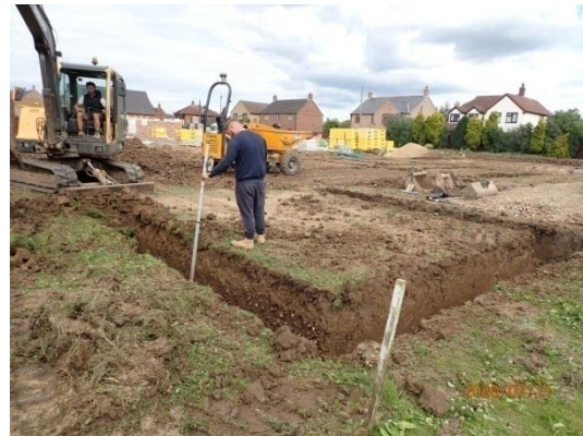
Plate 41: Excavation of the foundations, from the north-west
