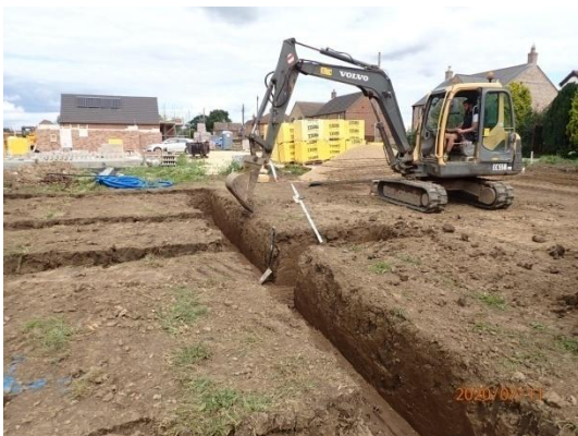
Plate 33: Excavation of the foundations, from the south
