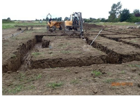
Plate 28: Excavation of the foundations, from the east
