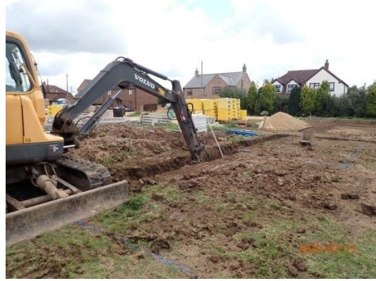
Plate 16: Excavation of the foundations, from the south-west
