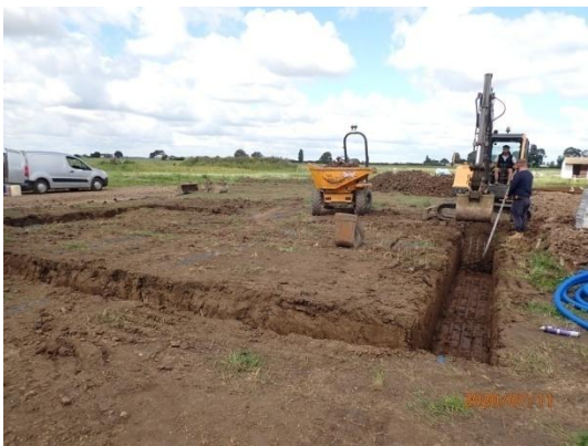
Plate 15: Excavation of the foundations, from the east
