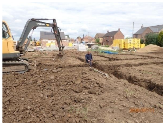
Plate 30: Excavation of the foundations, from the south
