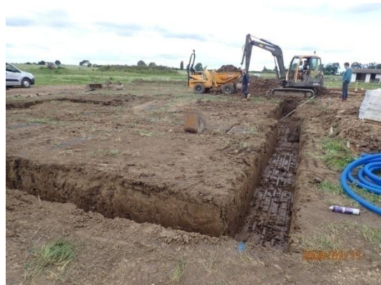
Plate 17: Excavation of the foundations, from the east
