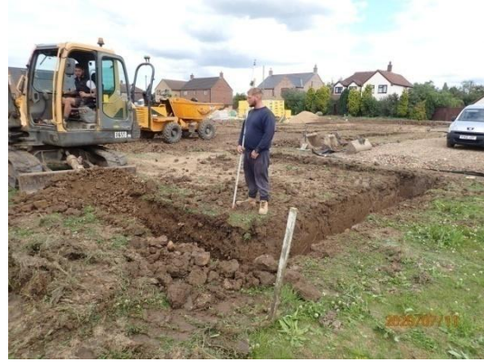
Plate 40: Excavation of the foundations, from the north-west
