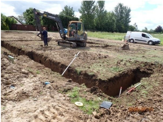
Plate 20: Excavation of the foundations, from the north-west
