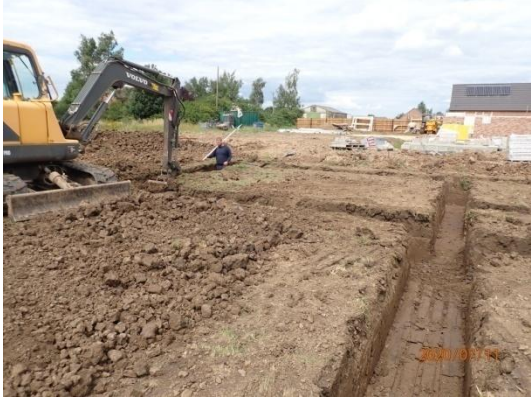
Plate 31: Excavation of the foundations, from the south
