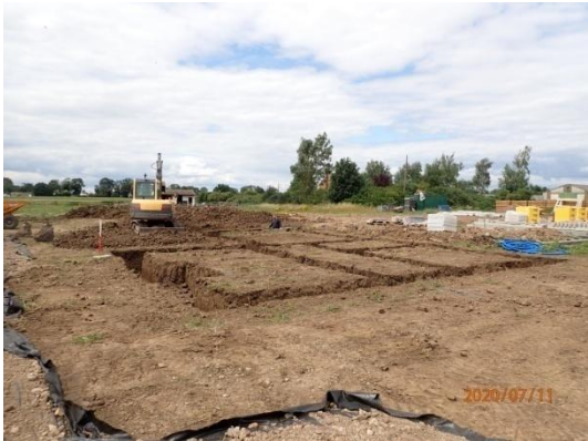
Plate 32: Excavation of the foundations, from the south-east
