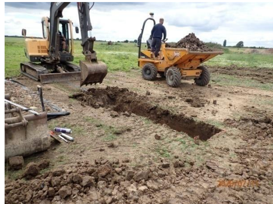
Plate 35: Excavation of the foundations, from the north-east
