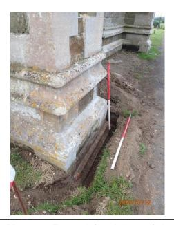
**Plate 12:** Exposed foundations of the north-western buttress of the West Tower, from the north
