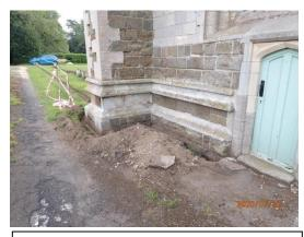
**Plate 5:** Hand excavated section of the cable trench around the north-western buttress of the West Tower & the West Tower, from the south
