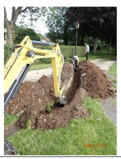
**Plate 18:** Excavation of the cable trench, from the south
