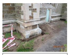
Plate 4: Hand excavated section of the cable trench around the north-western buttress of the West Tower, from the north-west
