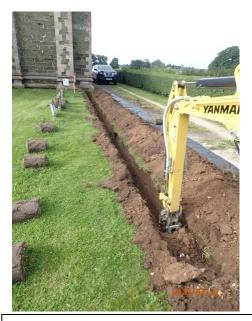
**Plate 26:** Excavation of the cable trench, from the north
