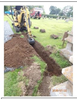
**Plate 20:** Excavation of the cable trench, from the south
