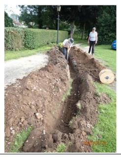
**Plate 19:** Excavation of the cable trench, from the south
