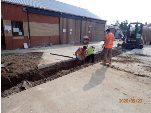
Plate 19: Excavation of the foundations, from the north-west
