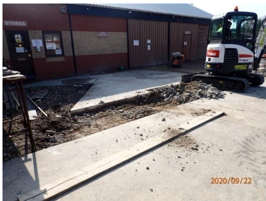
Plate 3: Excavation of the foundations, from the north
