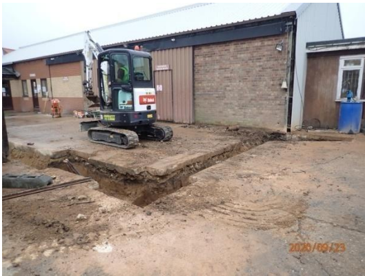
Plate 38: Excavation of the foundations, from the west
