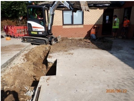
Plate 14: Excavation of the foundations, from the south-west
