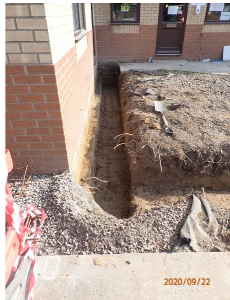
Plate 18: Excavation of the foundations, from the north
