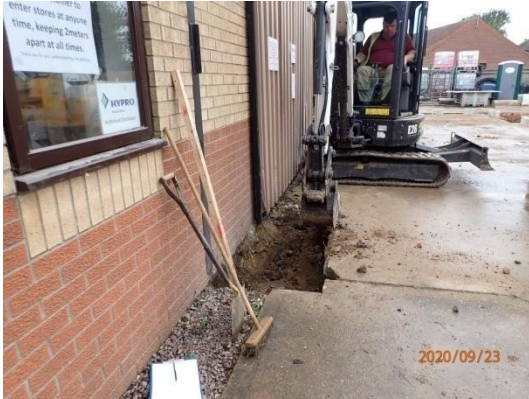
Plate 49: Excavation of the foundations, from the north-east
