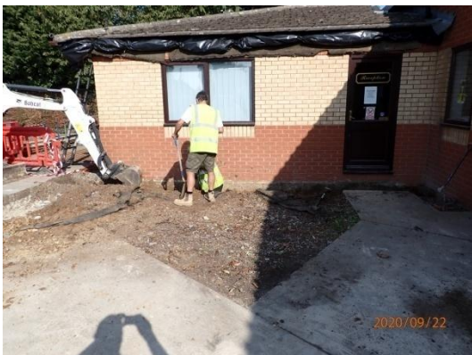
Plate 15: Excavation of the foundations, from the west
