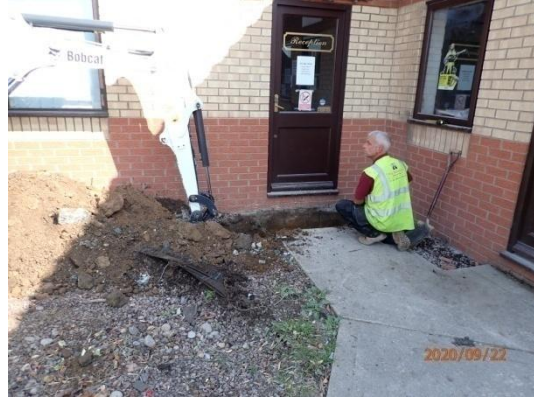
Plate 10: Excavation of the foundations, from the west
