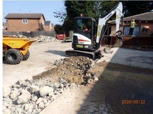
Plate 4: Excavation of the foundations, from the south-west
