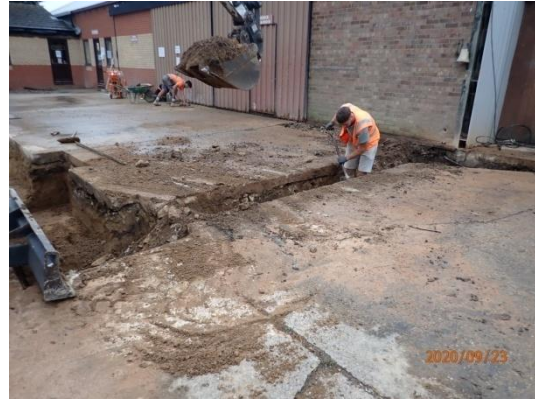
Plate 34: Excavation of the foundations, from the south-west
