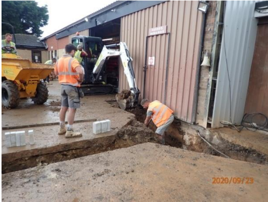
Plate 43: Excavation of the foundations, from the west
