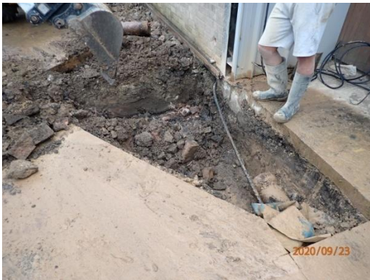
Plate 32: Excavation of the foundations, from the west
