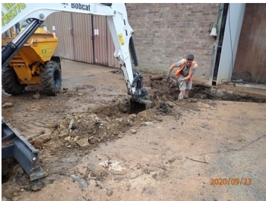
Plate 33: Excavation of the foundations, from the north-west
