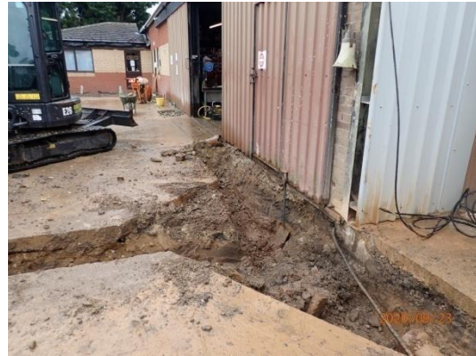
Plate 41: Excavation of the foundations, from the south-west
