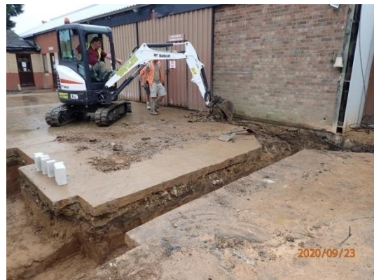
Plate 42: Excavation of the foundations, from the west
