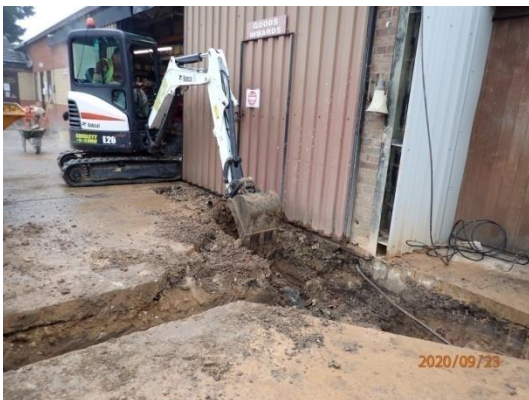
Plate 39: Excavation of the foundations, from the west
