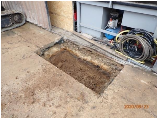
Plate 51: Excavation of the foundations, from the north-west
