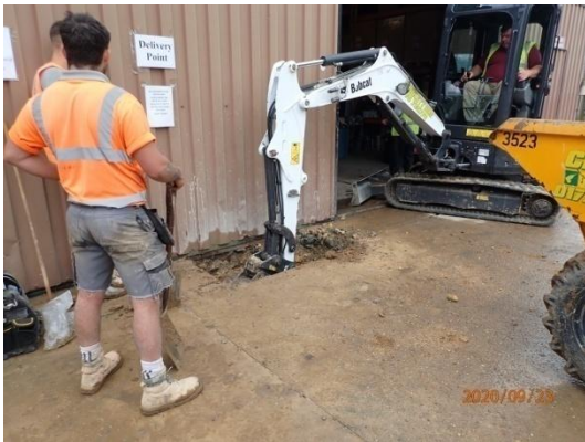
Plate 44: Excavation of the foundations, from the north-west
