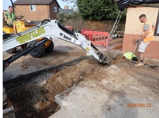
Plate 16: Excavation of the foundations, from the south-west
