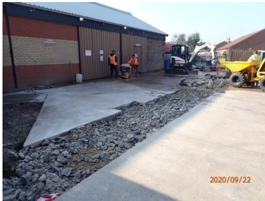
Plate 2: Pre-groundworks, from the north
