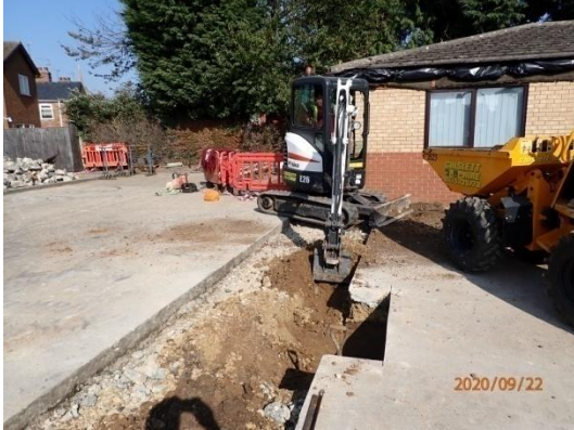
Plate 13: Excavation of the foundations, from the south-west
