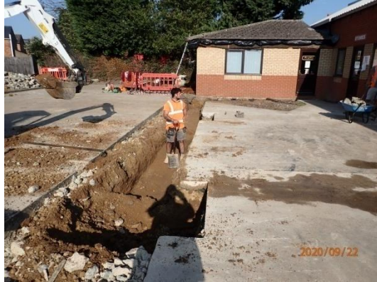
Plate 22: Excavation of the foundations, from the south-west
