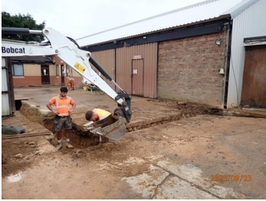
Plate 37: Excavation of the foundations, from the west
