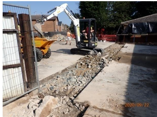
Plate 5: Excavation of the foundations, from the south-west
