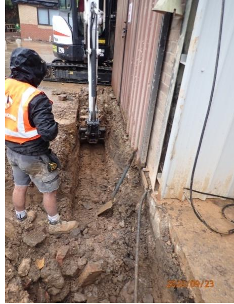
Plate 40: Excavation of the foundations, from the south-west
