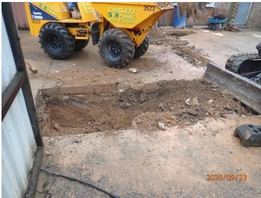
Plate 26: Excavation of the foundations, from the north-west
