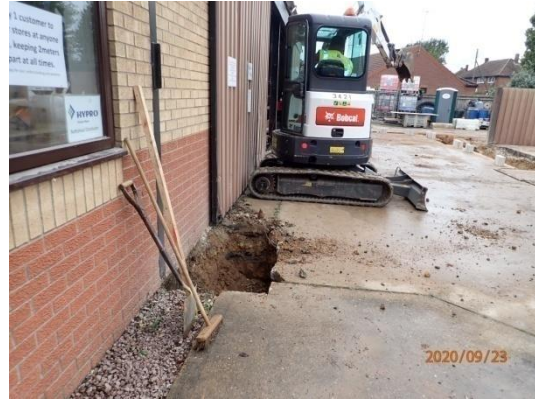
Plate 52: Excavation of the foundations, from the north-east
