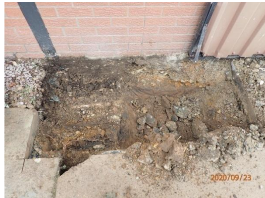
Plate 47: Excavation of the foundations, from the north-west
