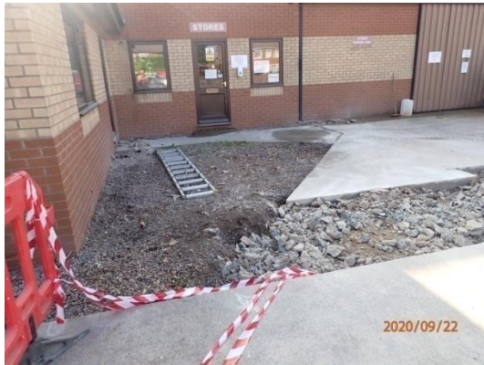
Plate 1: Pre-groundworks, from the north-west
