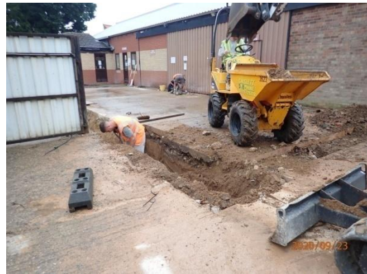
Plate 29: Excavation of the foundations, from the south-west
