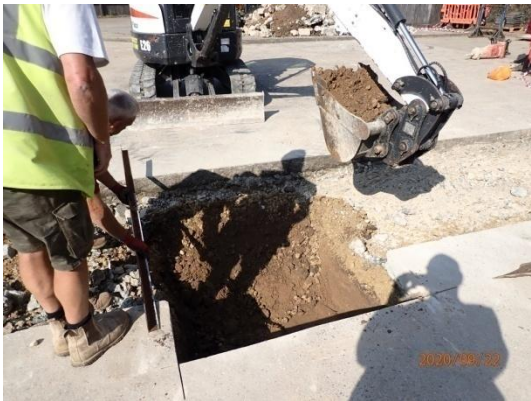
Plate 9: Excavation of the foundations, from the south-east
