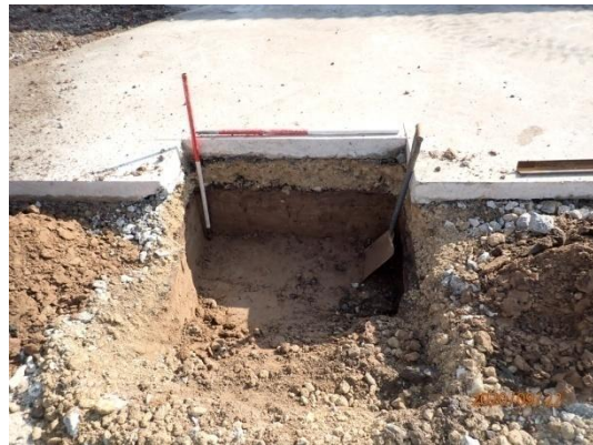
Plate 12: Representative Section 1, from the north-west
