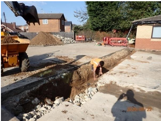
Plate 21: Excavation of the foundations, from the south-west
