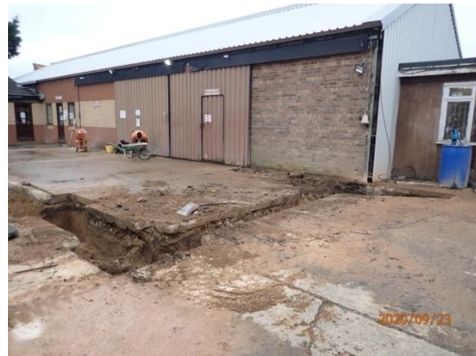
Plate 35: Excavation of the foundations, from the south-west
