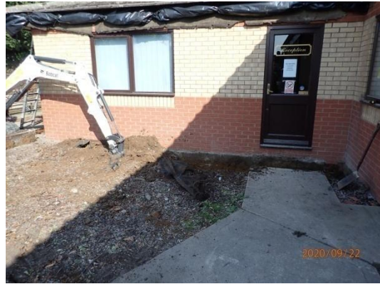
Plate 11: Excavation of the foundations, from the west
