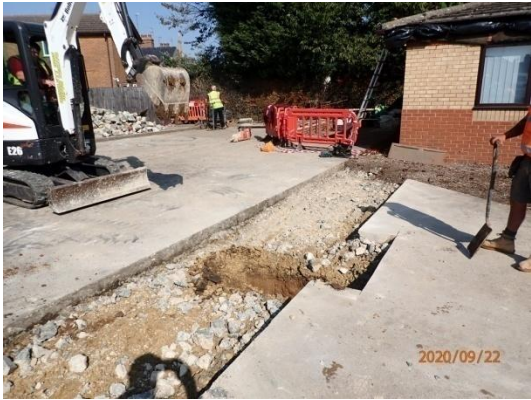
Plate 8: Excavation of the foundations, from the south-west
