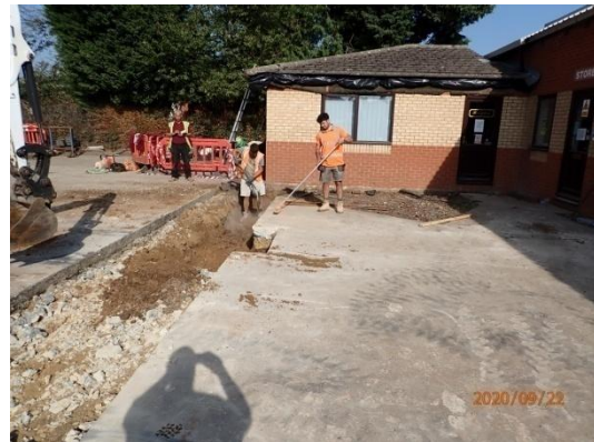
Plate 17: Excavation of the foundations, from the south-west
