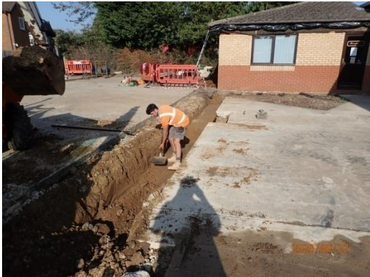
Plate 20: Excavation of the foundations, from the south-west
