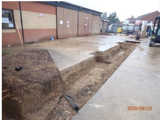
Plate 24: Excavation of the foundations, from the north
