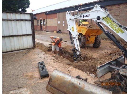
Plate 28: Excavation of the foundations, from the south-west
