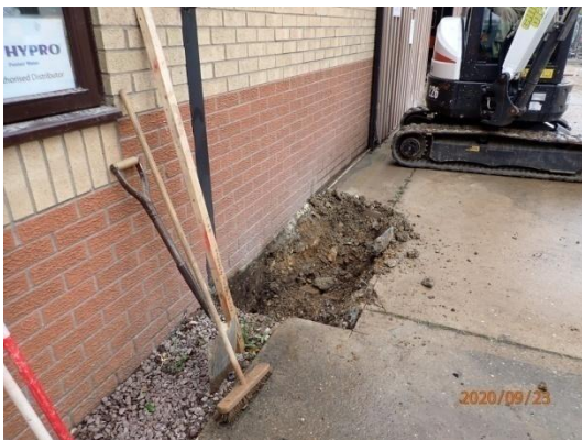
Plate 45: Excavation of the foundations, from the north-east
