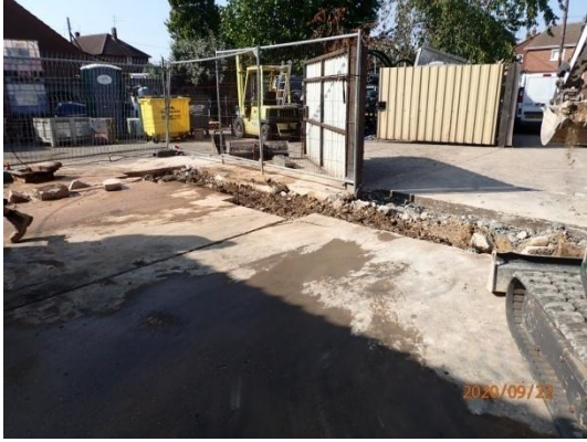
Plate 7: Excavation of the foundations, from the south-east
