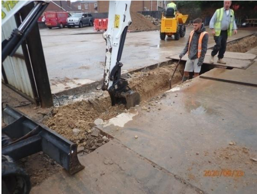
Plate 25: Excavation of the foundations, from the south-east
