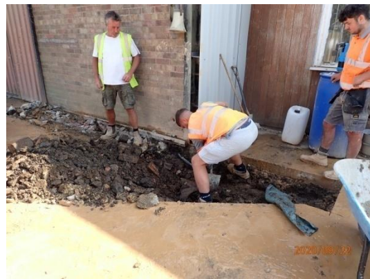
Plate 6: Hand excavations around the area of a modern drain, from the north
