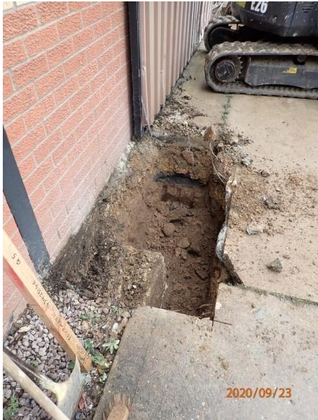
Plate 50: Excavation of the foundations, from the north-east
